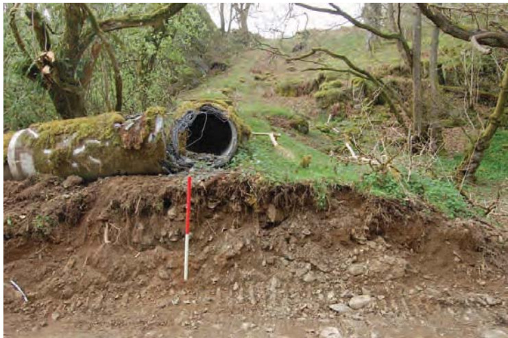
late . isused surge pipe F bro en through to allo access to borehole
