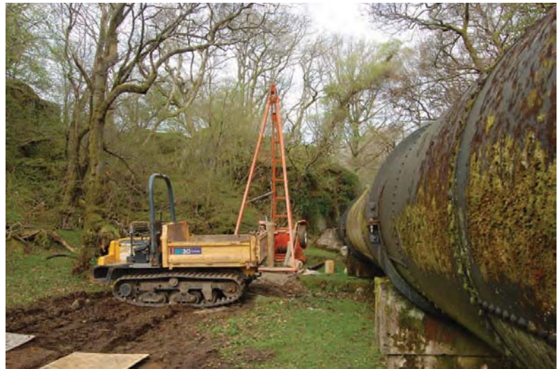
late . able percussi e borehole rig in place on
