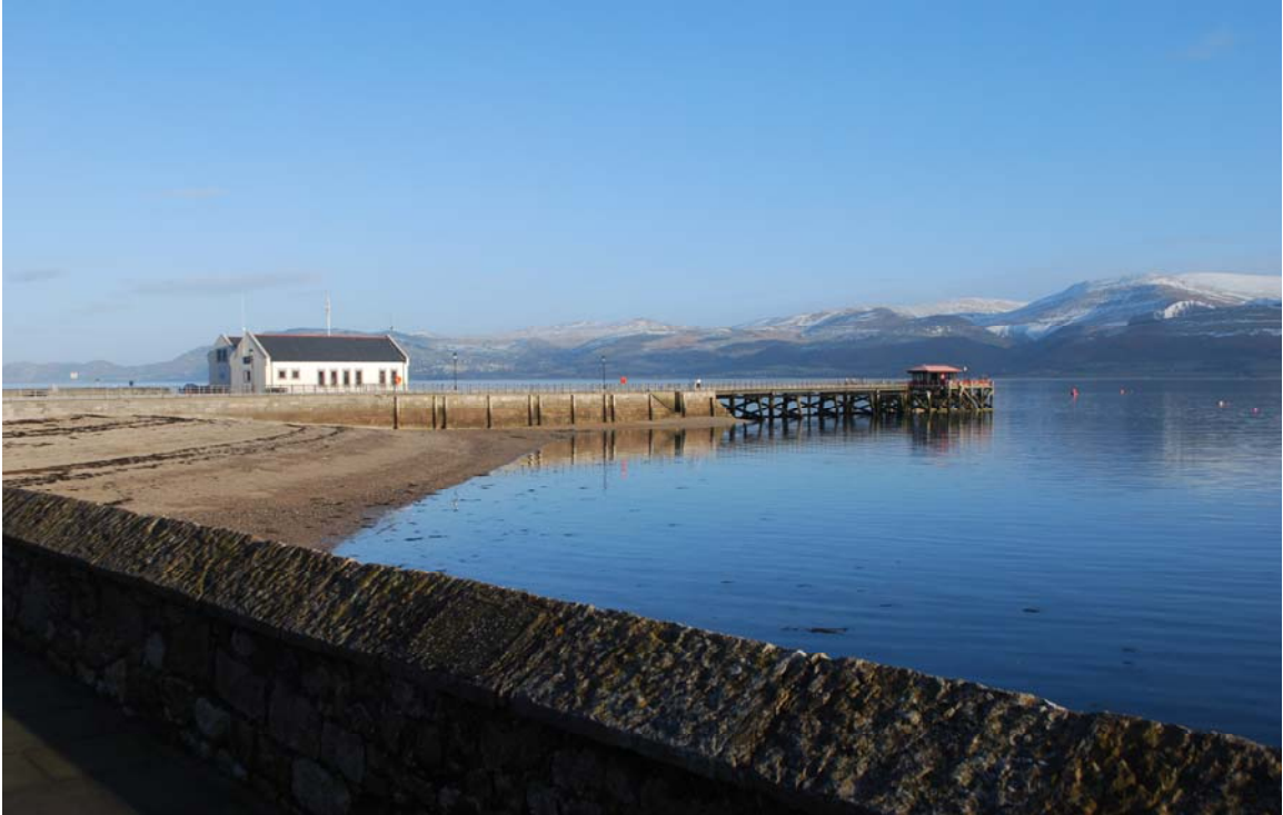
Plate 1 Beaumaris Pier from the west, showing stone and timber sections
