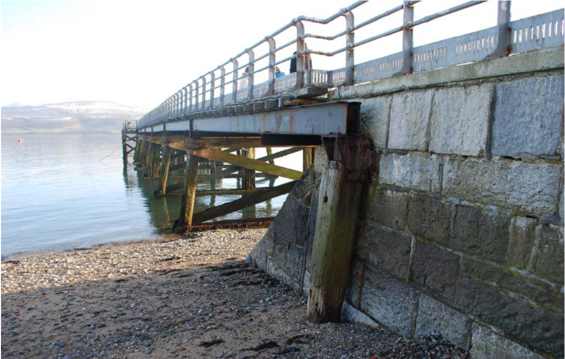
Plate 5 Detail showing the junction of the stone and wooden pier sections, from the north north east
