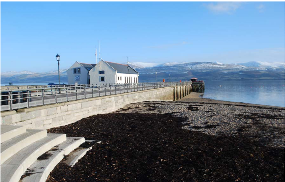
Plate 2 Beaumaris Pier from the north west, showing the lifeboat station
