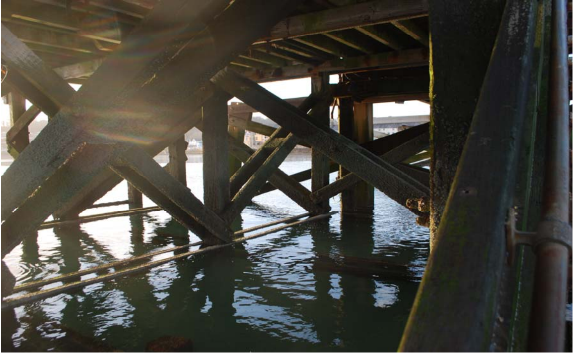
Plate 9 Detail showing the construction technique at the pier head
