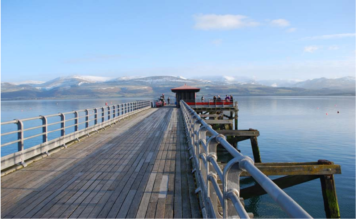
Plate 7 The timber decking with the shelter and landing stage at the southern end of the pier
