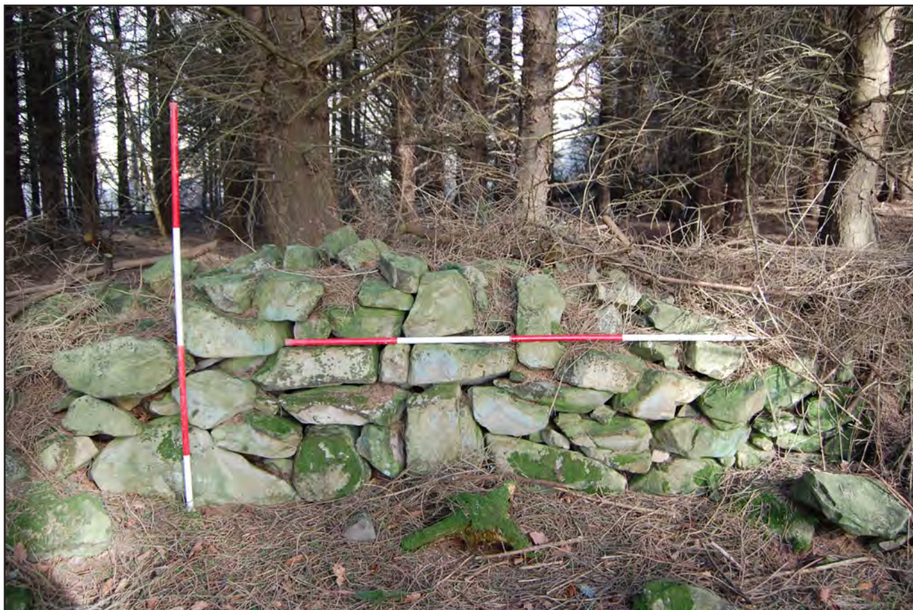
Plat 03: Darn o'r mur i'r de o'r bylchiad o'r uchder ac y lled gwreiddiol. Graddfa 2x2m. Plate 03: Section of wall south of breach which survives to the original height and width. Scale 2x2m.
