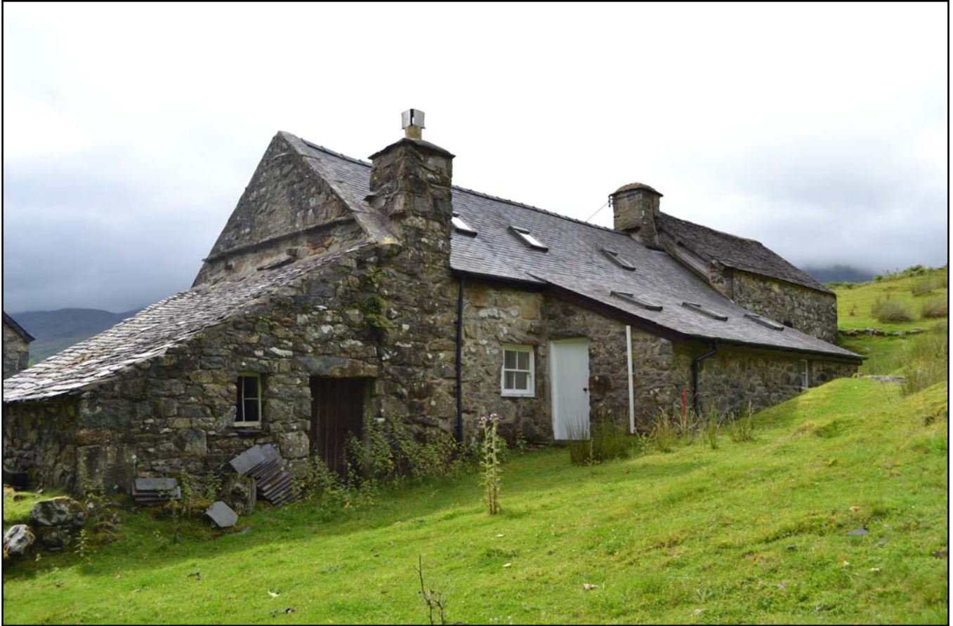
Plate 3: Northwest facing external elevation
