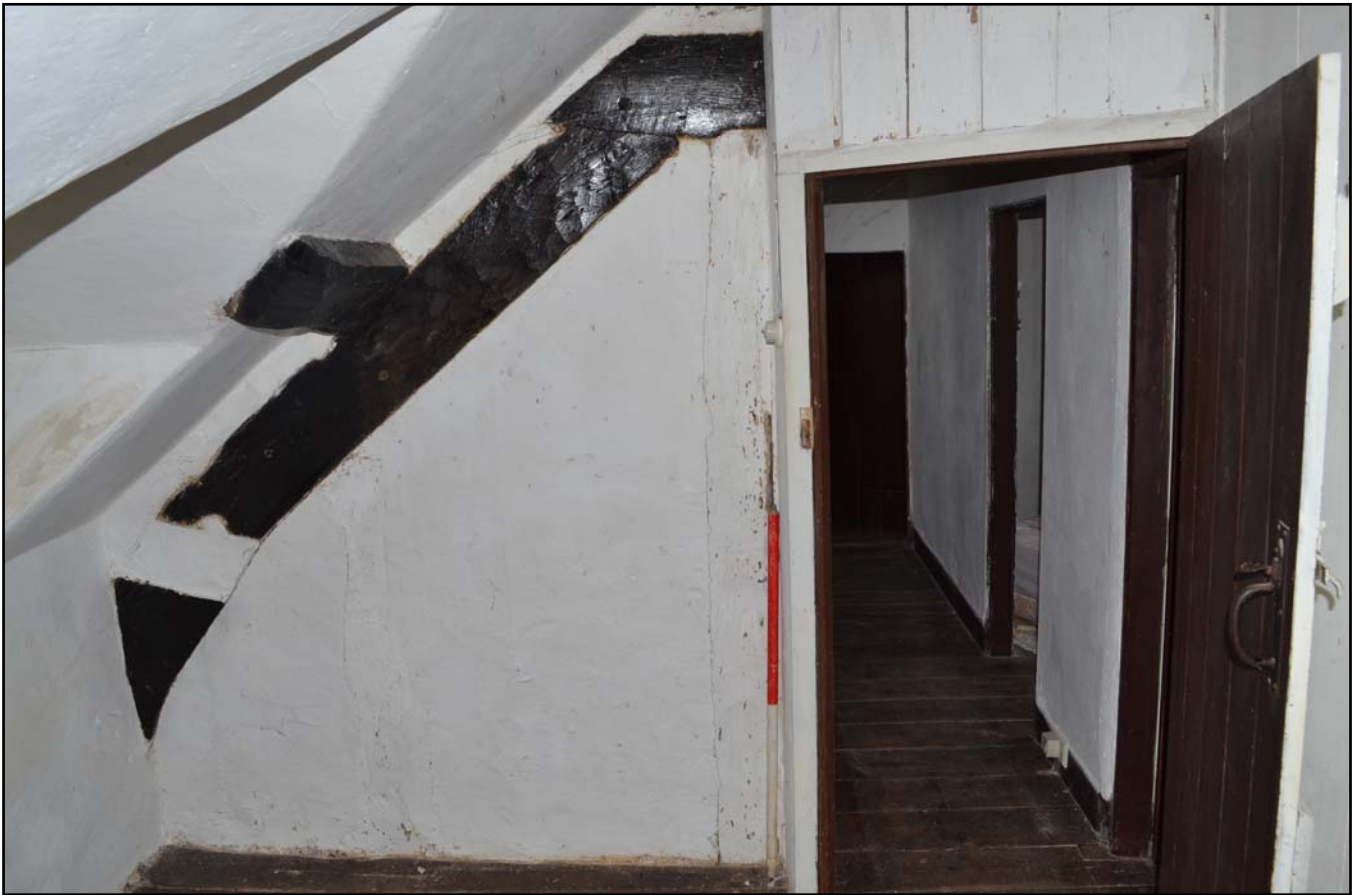
Plate 17: Bedroom 5 showing roof truss from the northeast
