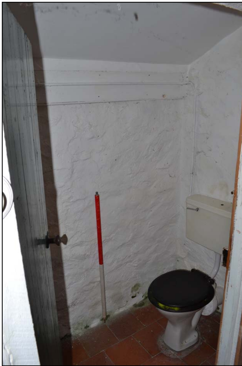
Plate 9: Toilet from the south
