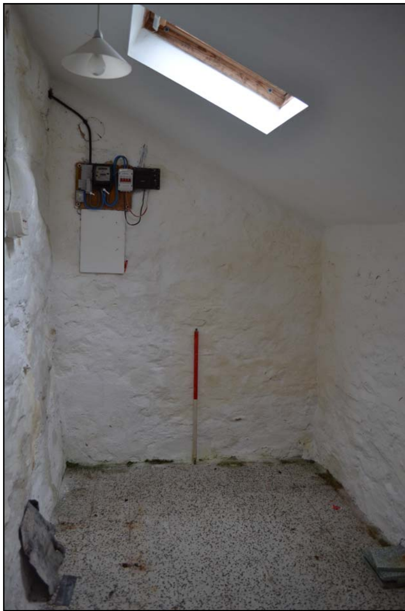
Plate 7: Kitchen from the southwest
