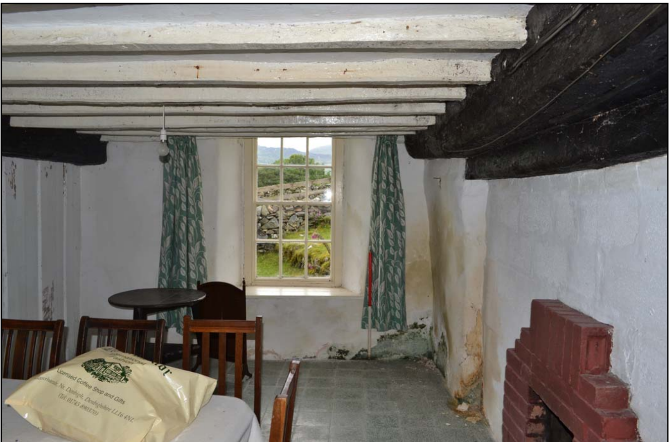
Plate 6: Former Hall from the northwest
