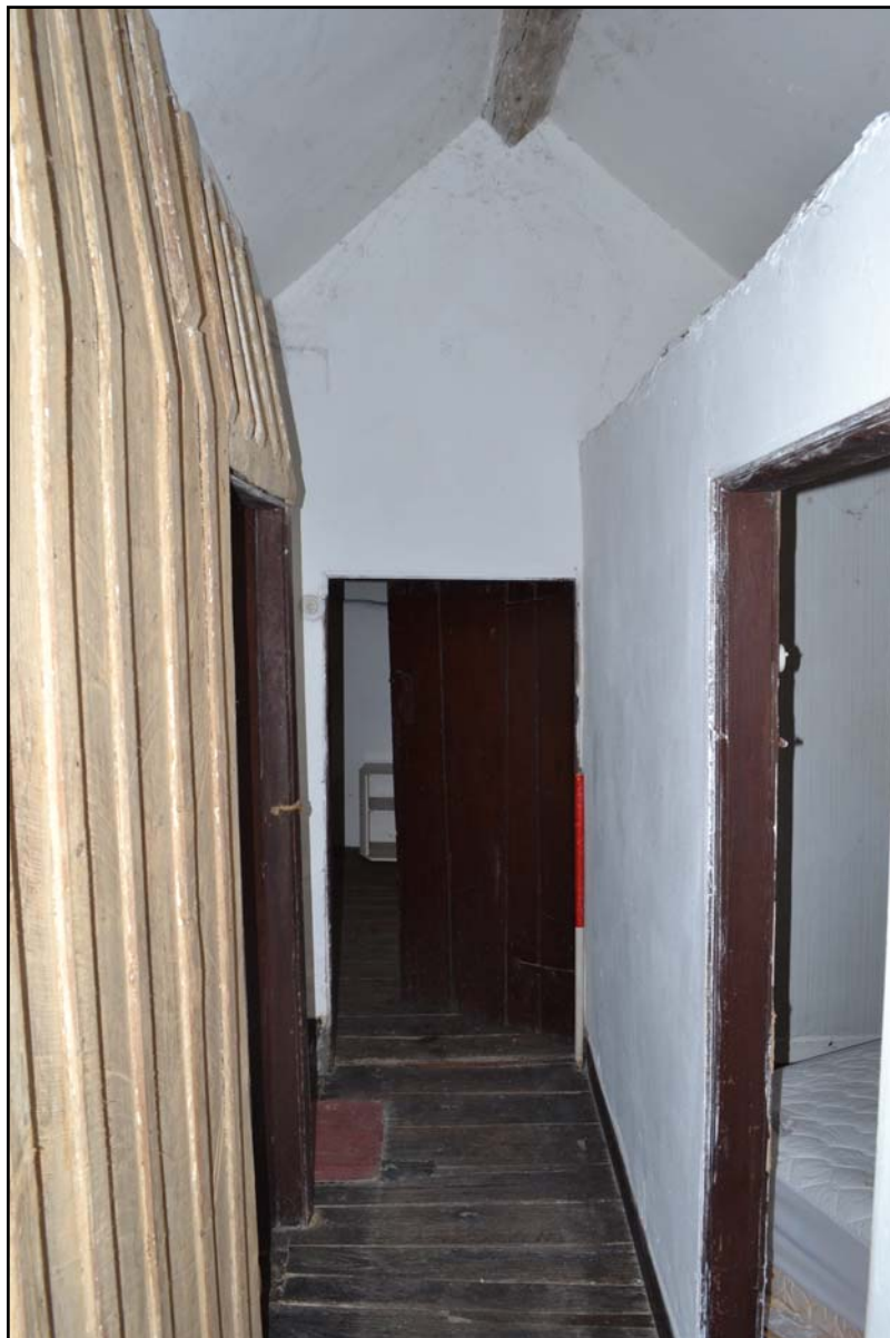
Plate 12: Upstairs landing from the southwest
