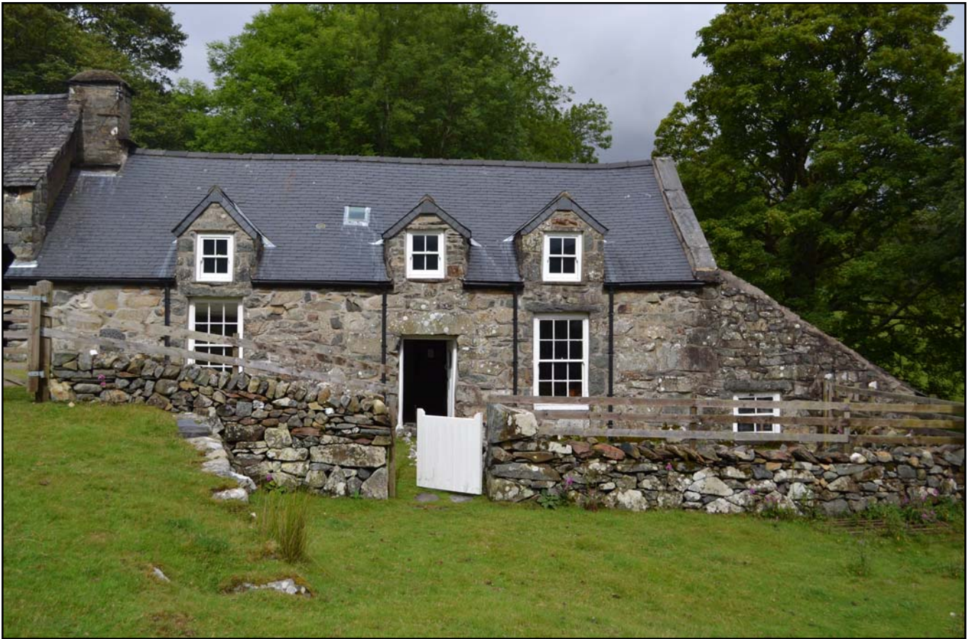
Plate 1: Southeast facing external elevation
