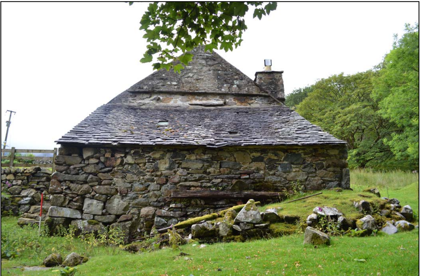
Plate 2: Northeast external elevation showing waterwheel pit
