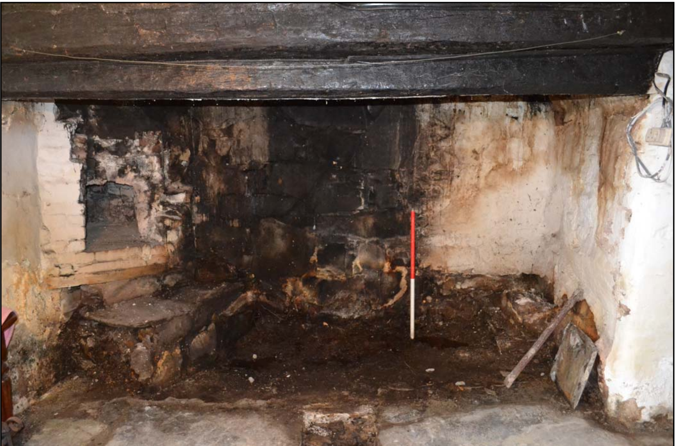
Plate 20: Former Hall inglenook fireplace revealed, from the southeast
