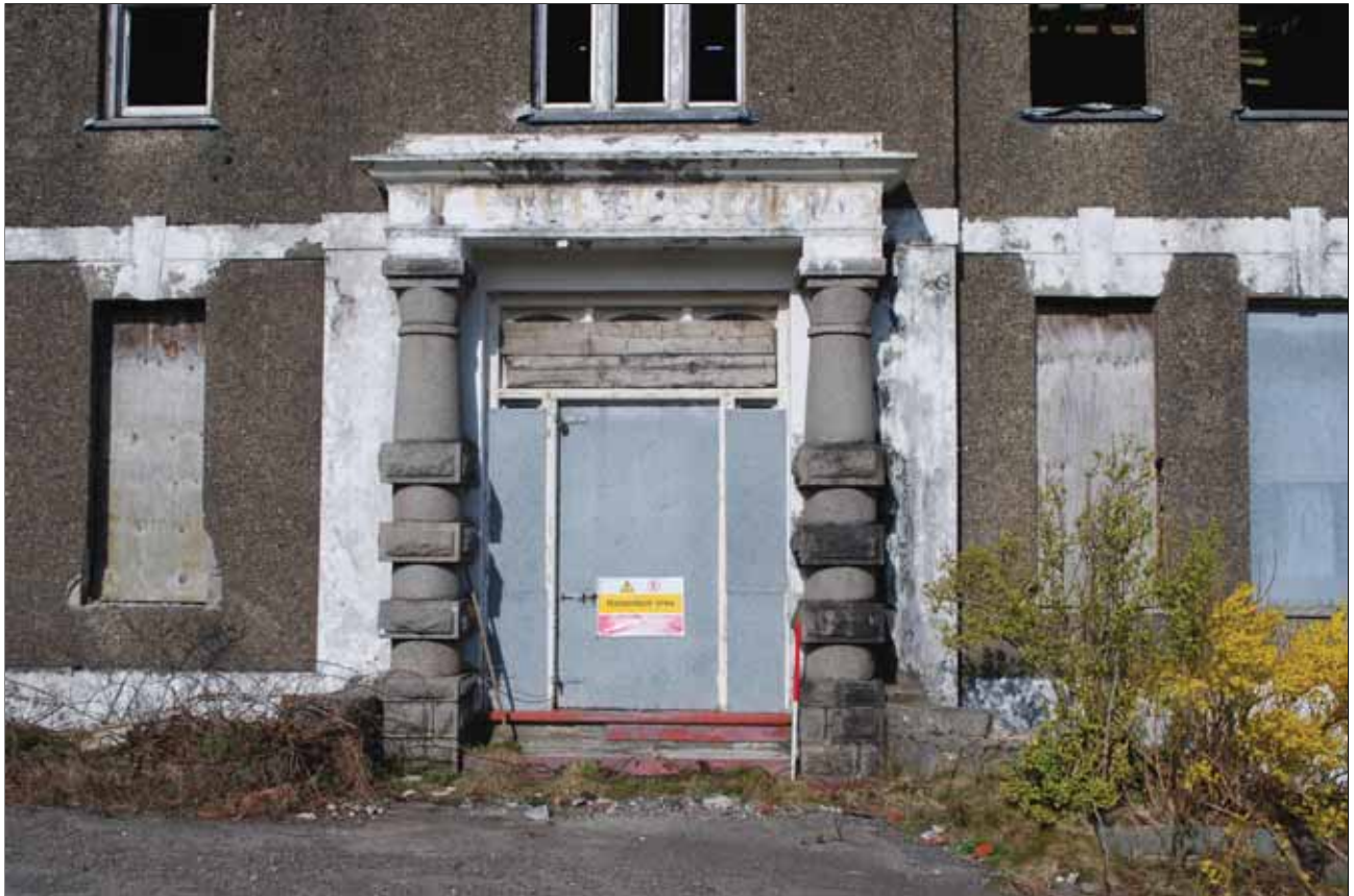
Plate 6 View of snecked granite columns at Plas Pistill from the south east. Scale 1m
