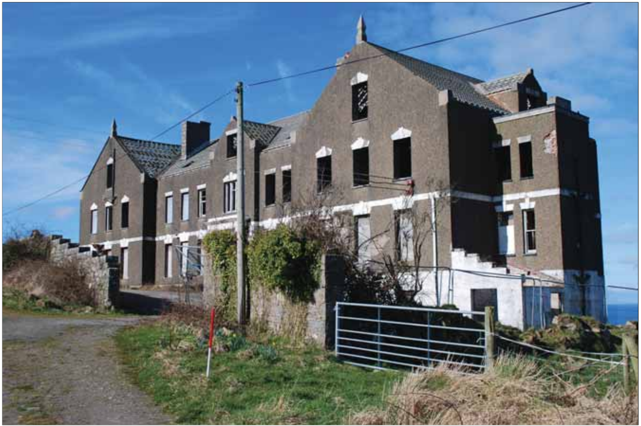
Plate 5 Plas Pistyll from the south east. Scale 1m
