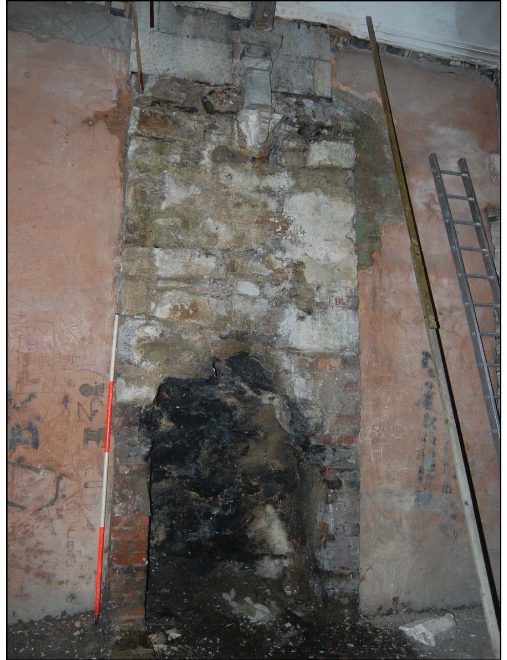
Plate 12. Ysgol Jones Bach fireplace, south elevation (internal)
