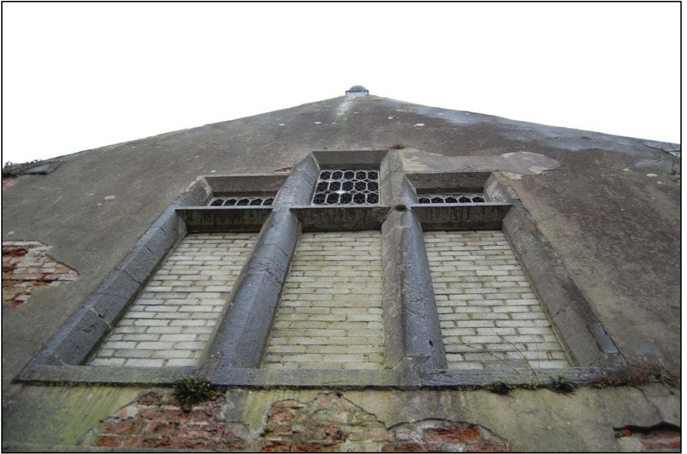
Plate 5. Ysgol Jones Bach west elevation (external)
