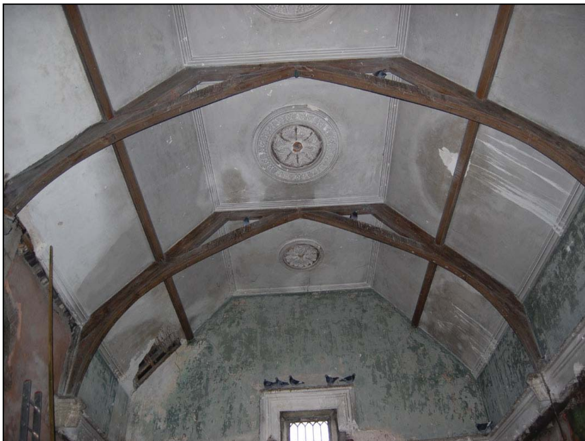
Plate 14 . Ysgol Jones Bach hammer-beam trusses, west elevation (internal).
