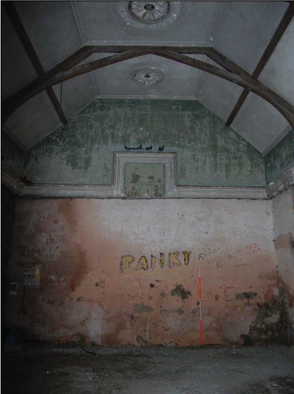
Plate 7. Ysgol Jones Bach east elevation (internal)
