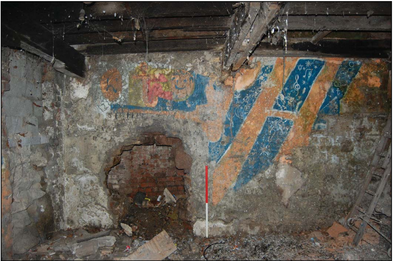
Plate 17. Ysgol Jones Bach, sub-level north elevation (internal)
