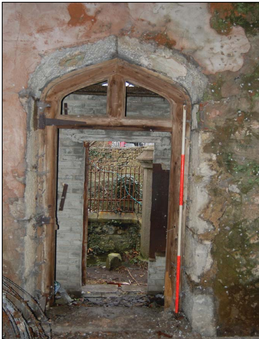
Plate 10. Ysgol Jones Bach door frame, north elevation (internal).
