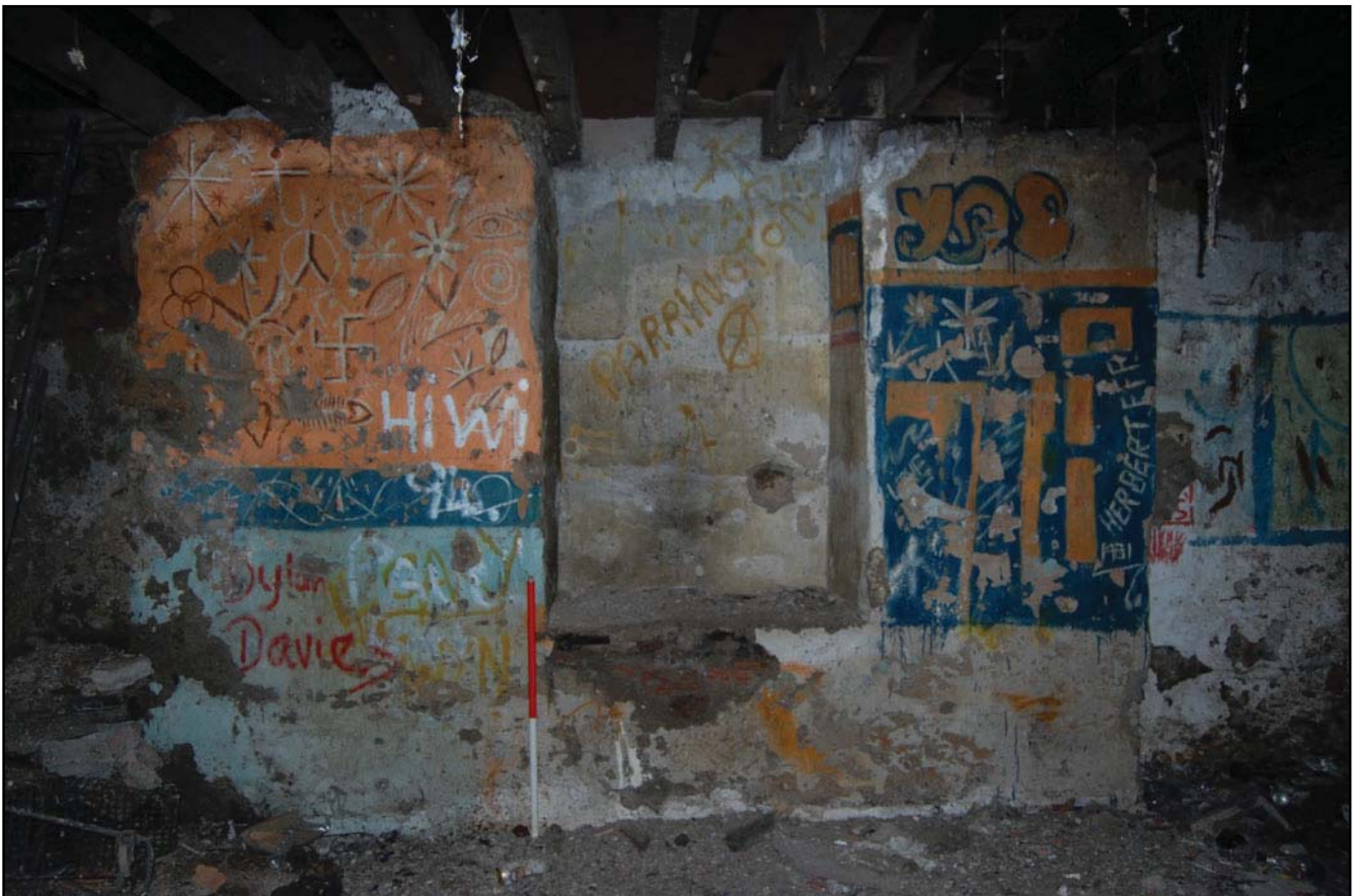
Plate 18. Ysgol Jones Bach, sub-level east elevation (internal)
