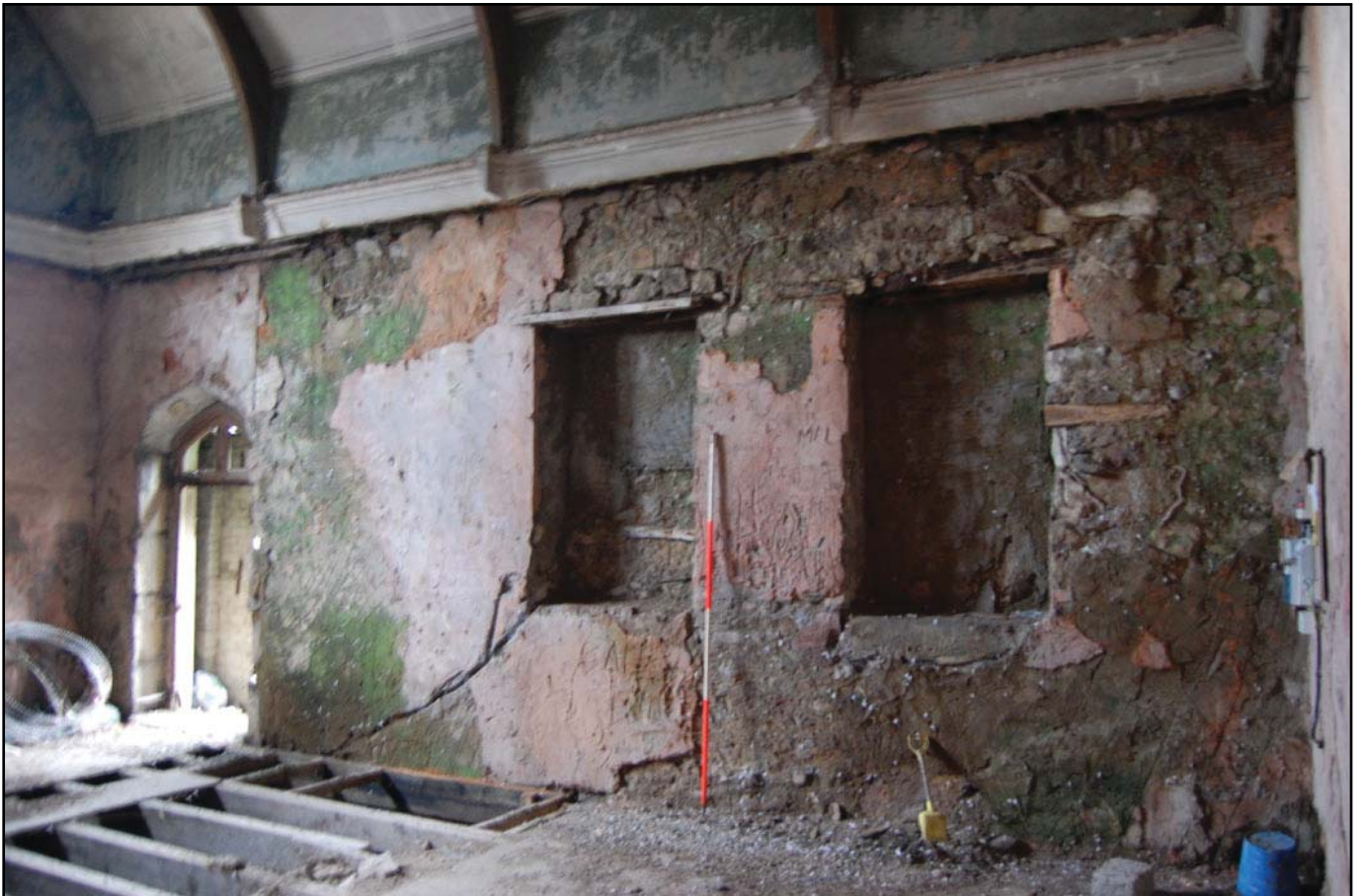
Plate 6. Ysgol Jones Bach north elevation (internal)
