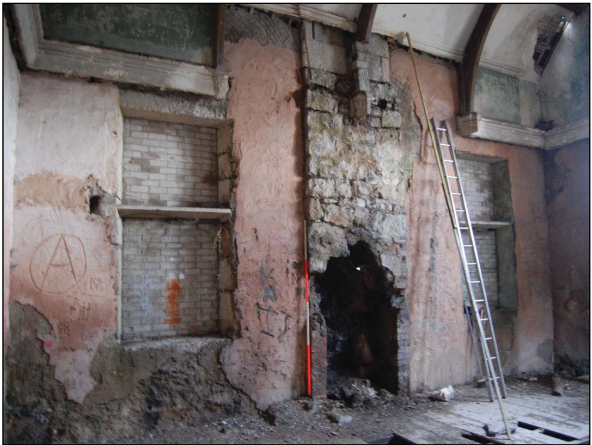
Plate 9. Ysgol Jones Bach south elevation (internal).
