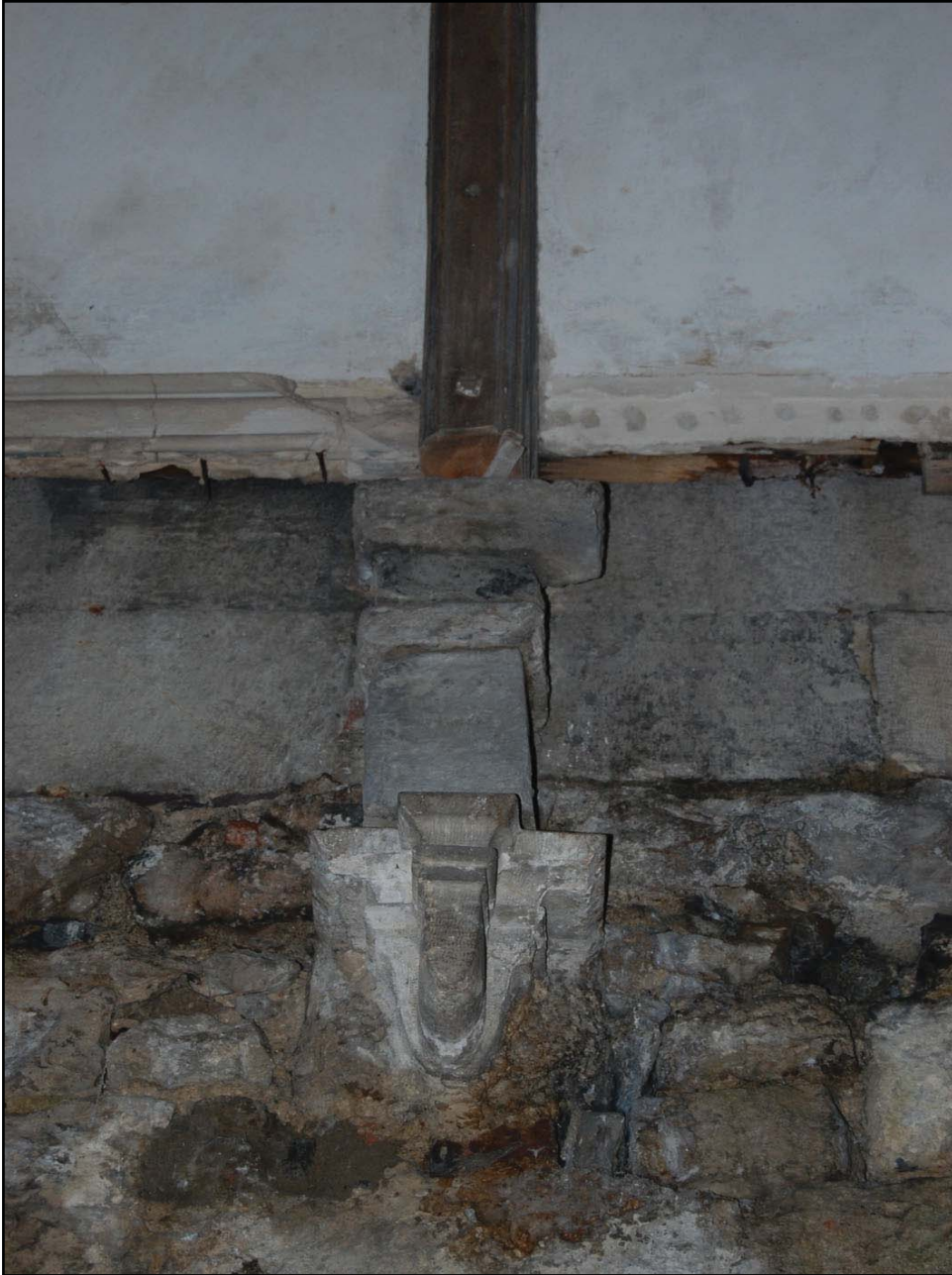
Plate 11. Ysgol Jones Bach decorated corbel stone, south elevation (internal)
