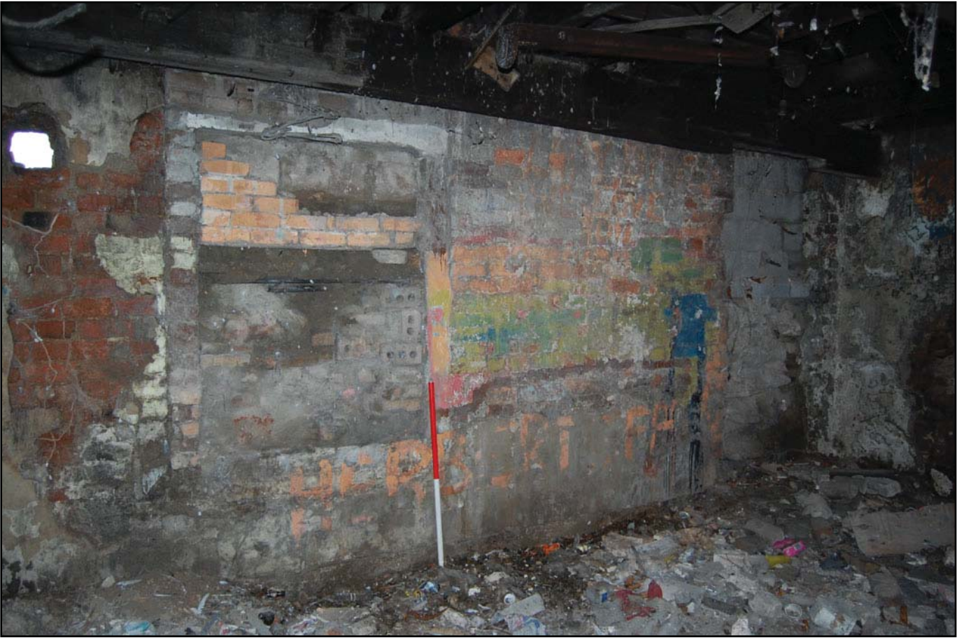
Plate 19. Ysgol Jones Bach, sub-level west elevation (internal)
