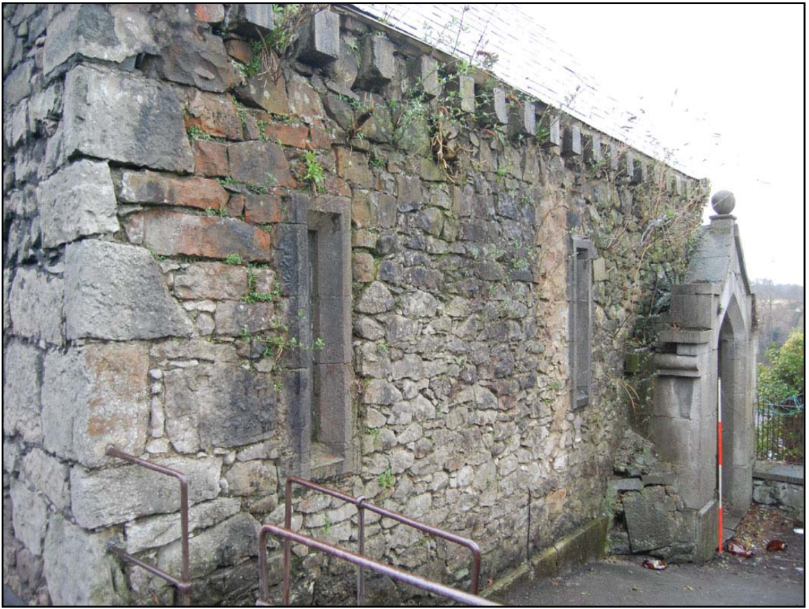
Plate 1. Ysgol Jones Bach north elevation (external).
