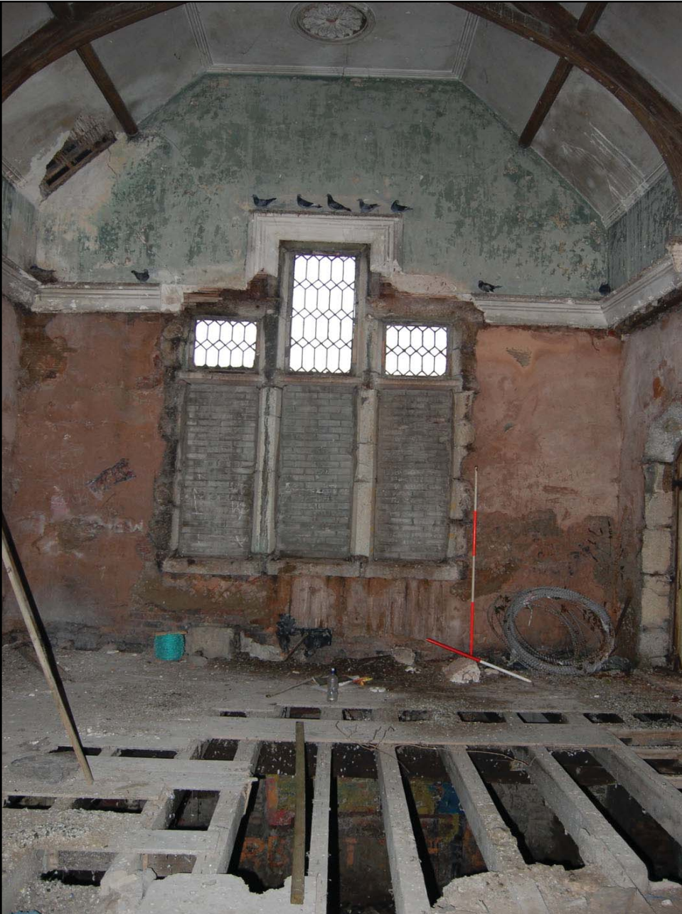
Plate 8. Ysgol Jones Bach west elevation (internal)
