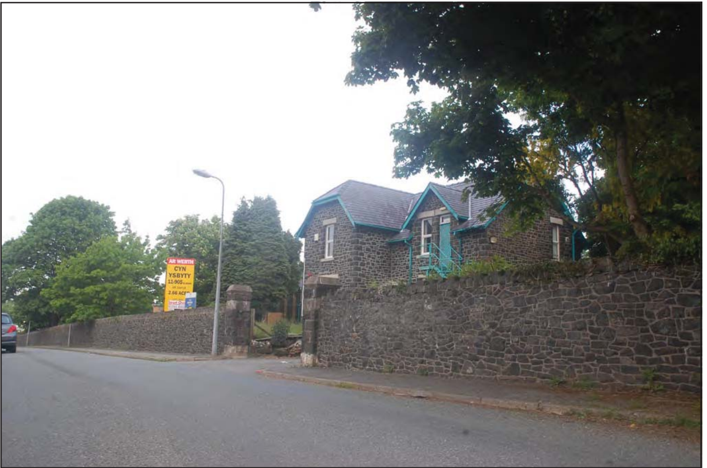
Plate 01: View west of main entrance and boundary wall along Hendrewen Road. The administration block is visible behind the boundary wall.
