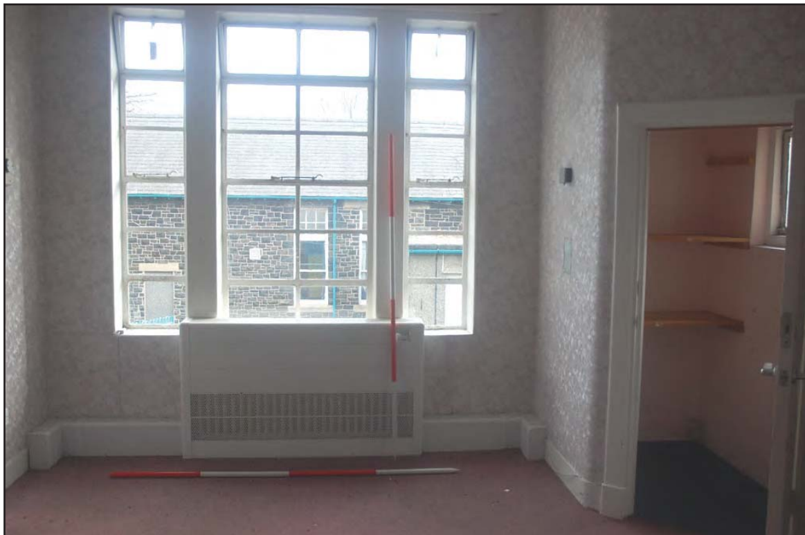
Plate 26: Short Stay Unit (Internal): view south of Room G01, detailing large casement window and internal structural and decorative features, including storage cubby (cf. Plate 25), door moulding and bullnose skirtings. Note the rear elevation of the Long Stay Unit visible through the window
