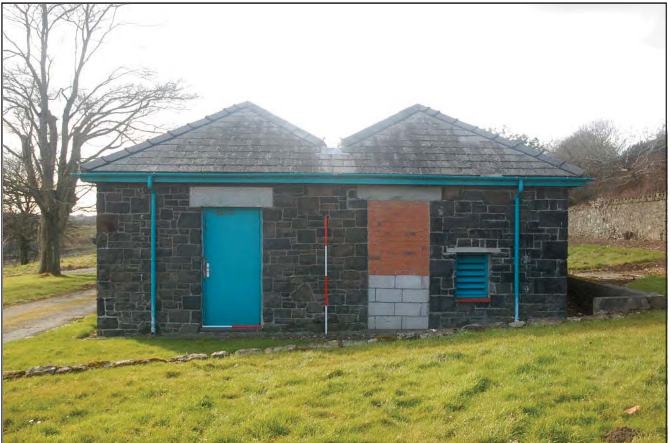
Plate 58: Generator Room: Southeast facing elevation detailing side entrance (blue door) and blocked entrance next to louvred vent. Double hip gable roof. The generator room was built between 1900 and 1914. The extension is indicated where the gables meet in the middle. (Scale: 1 x 2.0m; 1 x 1.0m)
