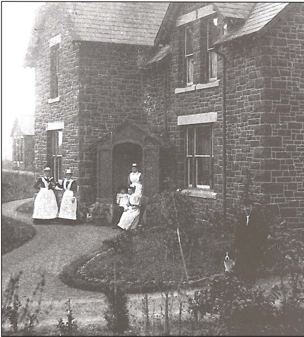
Plate 67: Administration Block - archive image from the nineteenth/early twentieth century detailing main entrance. The entrance porch has since been removed (cf. Plate 42); the front garden and path have been replaced with tarmacadam; the windows with modern sash replicas. A modern fire escape stairwell is now present linking the first floor parallel sash windows to the ground level; one of the two windows is now a fire escape door (Source: Roberts & Evans, 1995)
