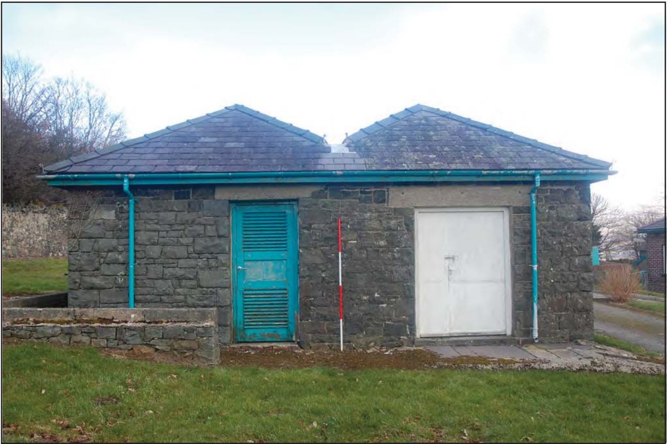
Plate 57: Generator Room: Northwest facing elevation detailing main entrance (large door) and louvred entrance. Double hip gable roof. The generator room was built between 1900 and 1914. An extension was later added, indicated by where the gables meet in the middle. The stonework on the left side of image is slightly different in appearance to the right side, indicating the extended portion. (Scale: 1 x 2.0m)
