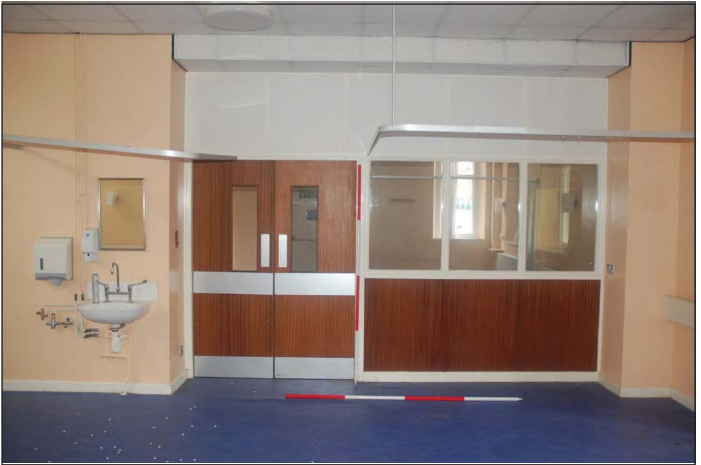
Plate 15: Long Stay Unit (Internal): Room G11 - view northeast of former female ward, detailing entrance via fire doors. Bullnose skirting boards are visible. Note Room G12 visible through the doors and screen (Scales: 2 x 2.0m)
