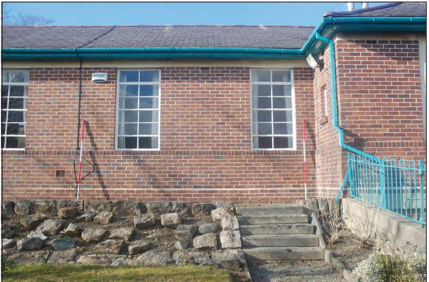
Plate 20: Short Stay Unit : Southeast facing elevation. Built from brick and not stone as the original buildings. Hip gable roof visible along with casement windows (Rooms G06 to G8). The courtyard separating the Long and Short Stay Units are visible in the foreground; the day room wing (Room G01) is visible to the right of the image (Scales: 2 x 2.0m)
