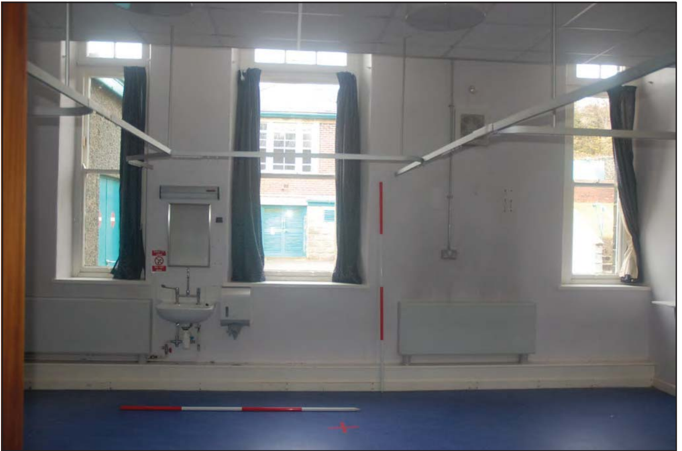
Plate 13: Long Stay Unit (Internal): Room G05 - view northwest detailing former male ward. All doors are fire doors. Bullnose skirting boards are visible. Note the Short Stay Unit visible through the windows as a brick-built structure (Scales: 2 x 2.0m)
