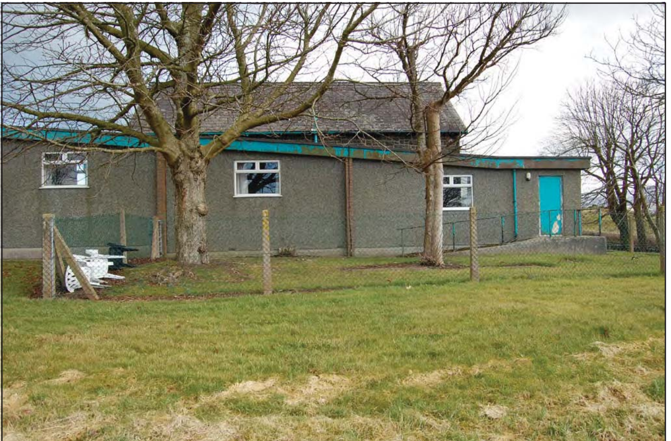
Plate 38: Link Corridor connecting Long and Short Stay Units: View east. Built 1991. Pebbledashed fronted with a box gutter and awning windows. Provides access to respective units; effectively masks the southwest facing elevations of both. Male ward wing of the Long Stay Unit is visible in the background as a slated pitched roof
