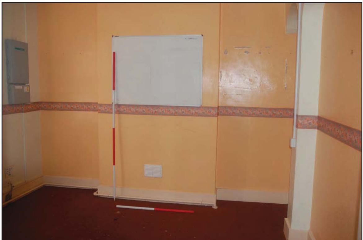
Plate 46: Administration Block (Internal): View southwest of former matron's office (Room G03) detailing redundant fireplace and current decor. Scales: 1 x 2.0m and 1 x 1.0m
