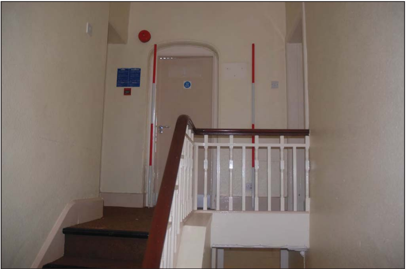
Plate 49: Administration Block (Internal): View northeast of first floor stairs leading to Rooms F02, F03 and F05. Room F03 is located at the centre of the image: the curved door arch is clearly visible. The staircase has a moulded rail with turned balusters; the tread and risers are carpeted. (Scales: 2 x 2.0m).
