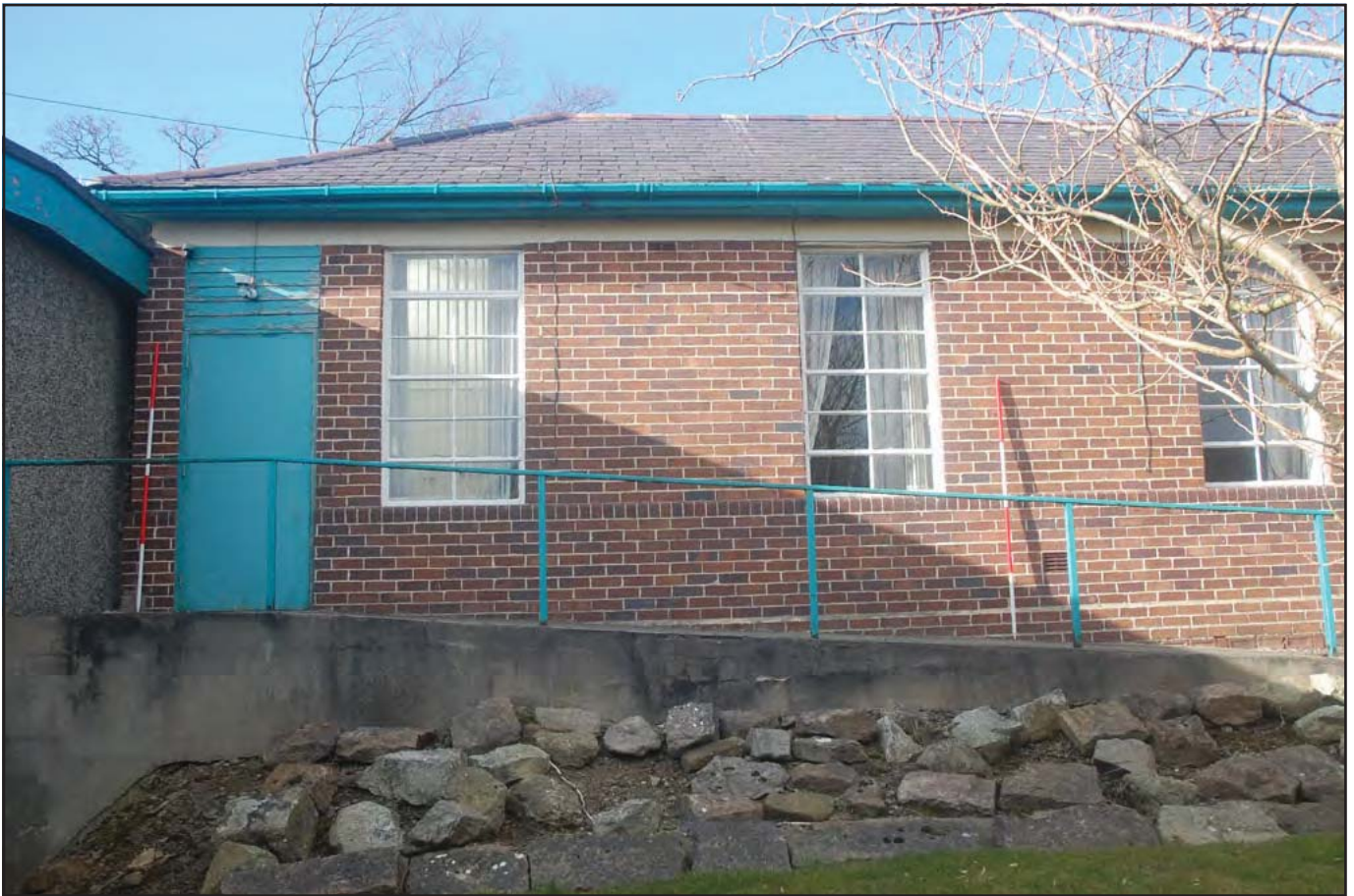
Plate 19: Short Stay Unit : Southeast facing elevation. Built from brick and not stone as the original buildings. Hip gable roof visible along with casement windows (Rooms G09, G10 & G13) and disabled access into G13. The courtyard separating the Long and Short Stay Units are visible in the foreground; the Link Corridor is visible to the left of the image (Scales: 2 x 2.0m)
