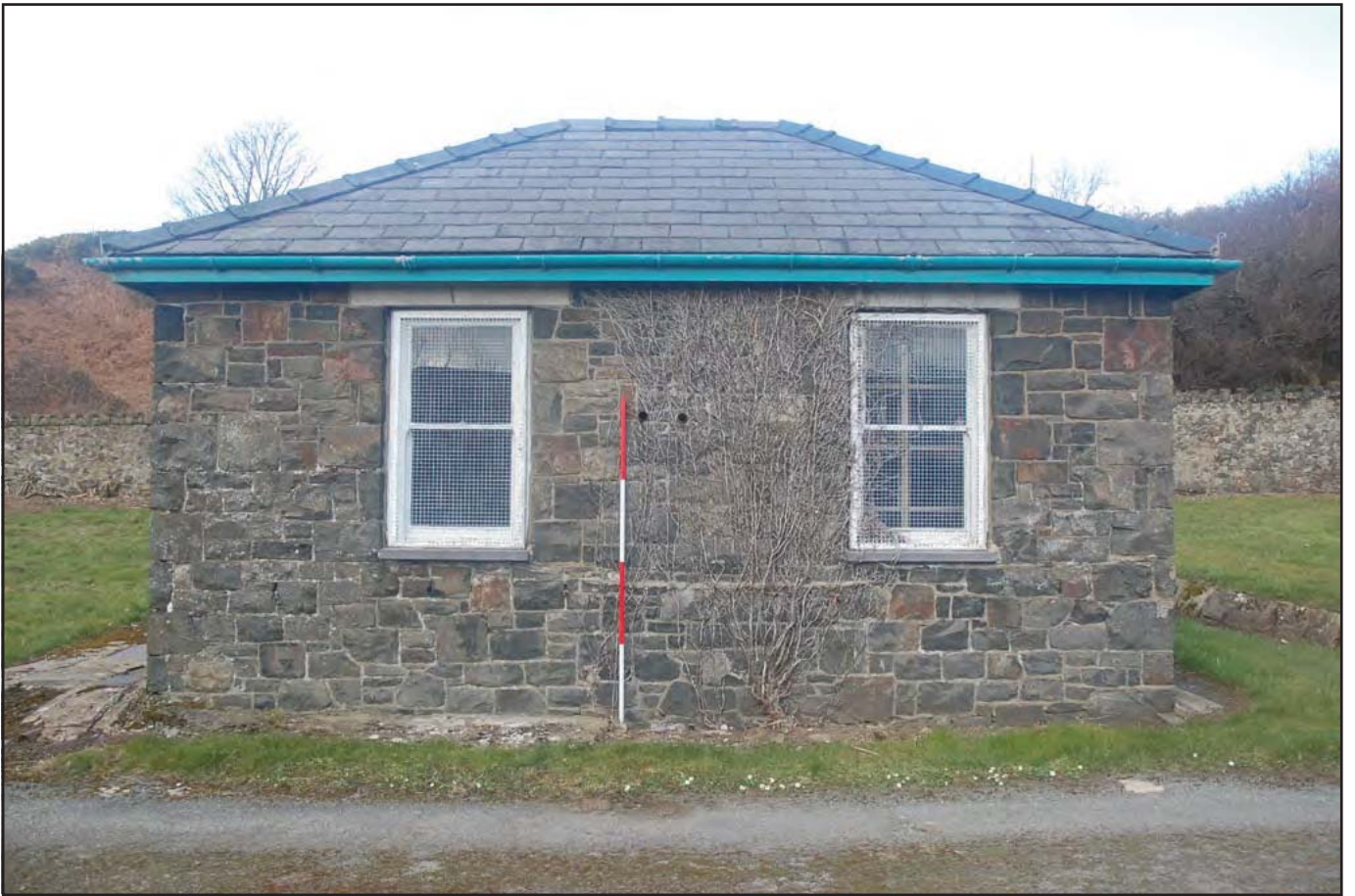
Plate 59: Generator Room: Southeast facing elevation detailing hip gable roof. The generator room was built between 1900 and 1914. An extension was later added (not visible). Stone lintel and quoins are present reflecting original building style for the hospital complex. (Scale: 1 x 2.0m)
