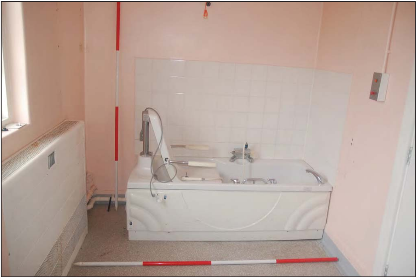
Plate 29: Short Stay Unit (Internal): View northeast of Room G05 detailing current use as a bathroom. Originally two rooms: sluice and bathroom, which were combined into a single room; original visible fittings limited to the casement window (left of image) (Scales: 2 x 2.0m)
