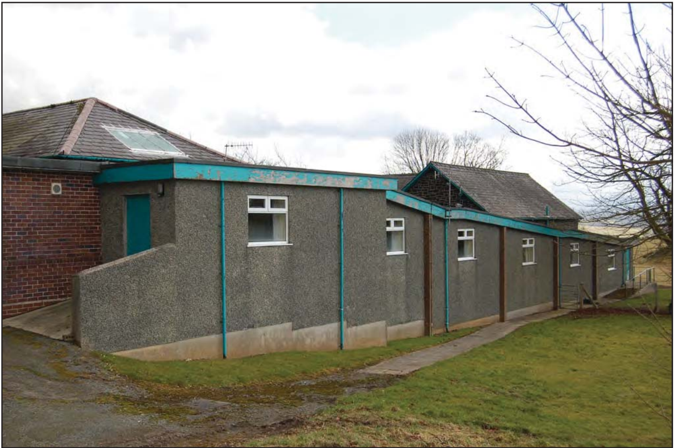
Plate 37: Link Corridor connecting Long and Short Stay Units: View south. Built 1991. Pebbledashed fronted with a box gutter and awning windows. Provides access to respective units; effectively masks the southwest facing elevations of both.
