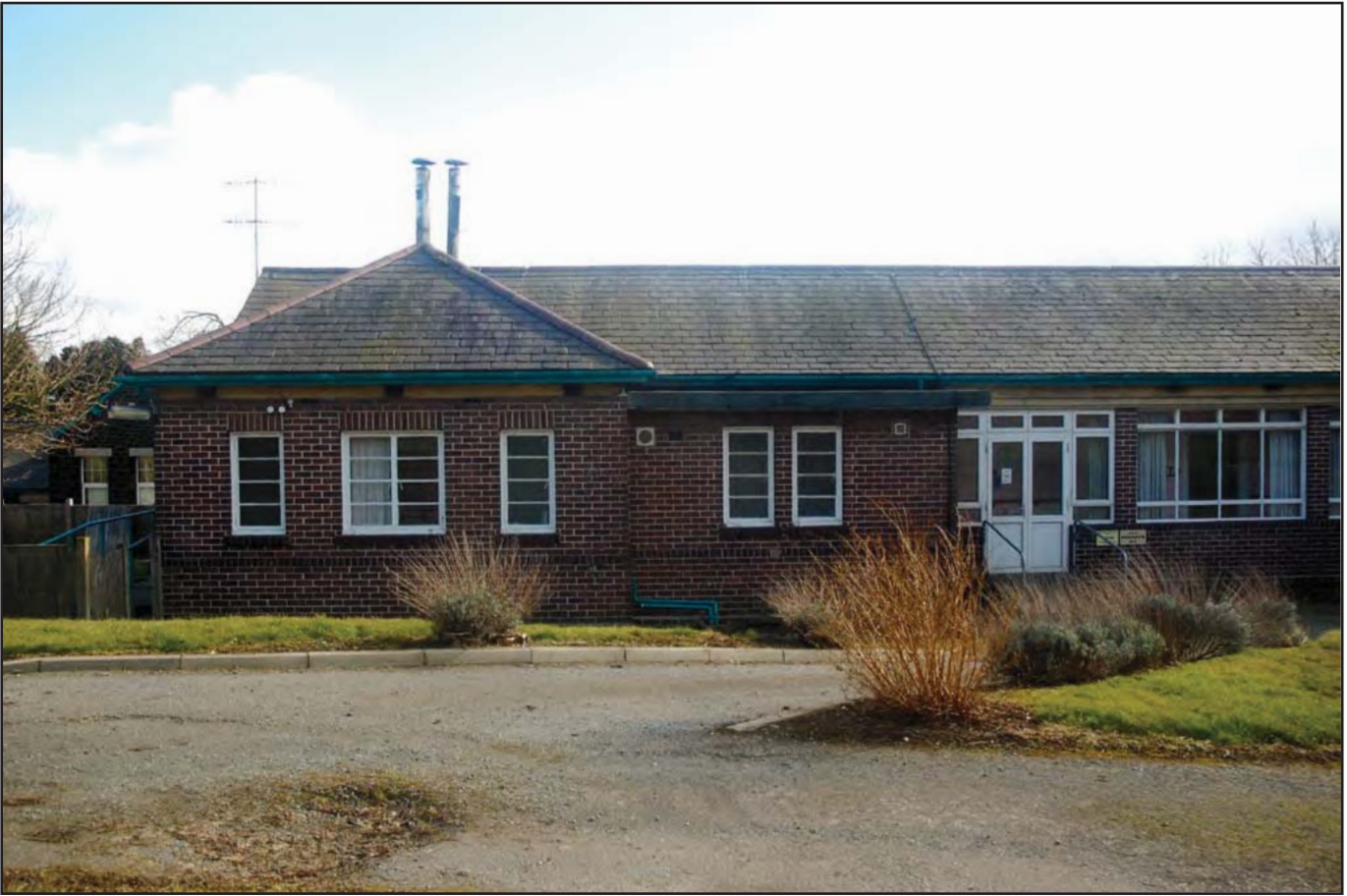
Plate 23: Short Stay Unit: Northwest facing elevation - Rooms G02 to G05 and main entrance; detailing English Garden Wall bond brick style and casement windows
