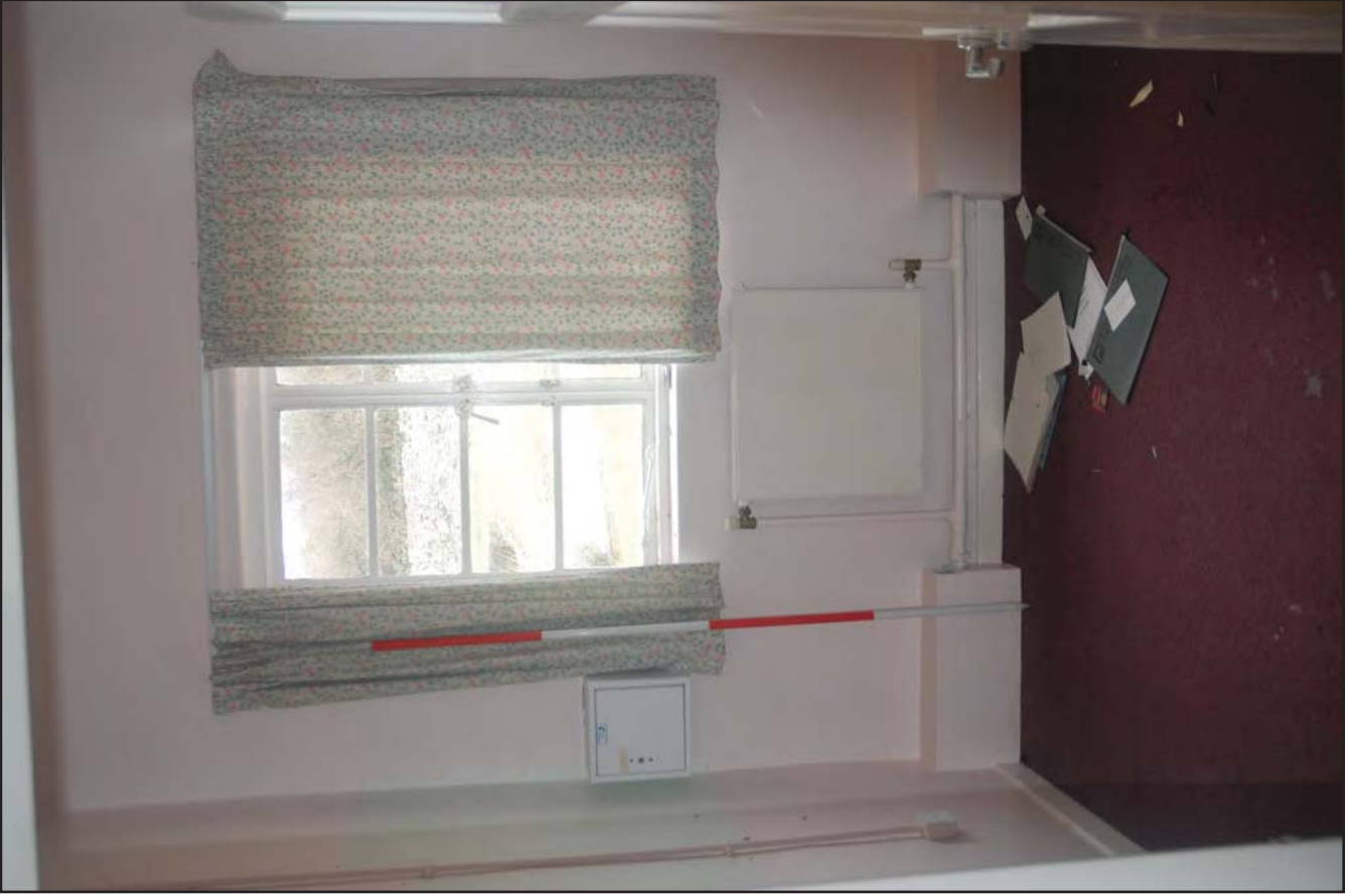
Plate 27: Short Stay Unit (Internal): view northwest of Room G03, detailing casement window and bullnose skirtings. Note moulded panel entrance door and not fire door as used in the Long Stay Unit (Scale: 1 x 2.0m)
