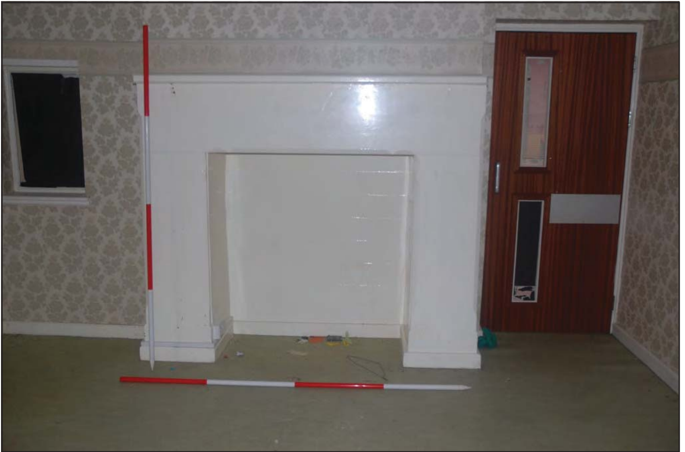
Plate 11: Long Stay Unit (Internal): Room G02 - view southwest detailing former ward kitchen fireplace current decorative styles and features. All doors are fire doors. Bullnose skirting boards are visible.
