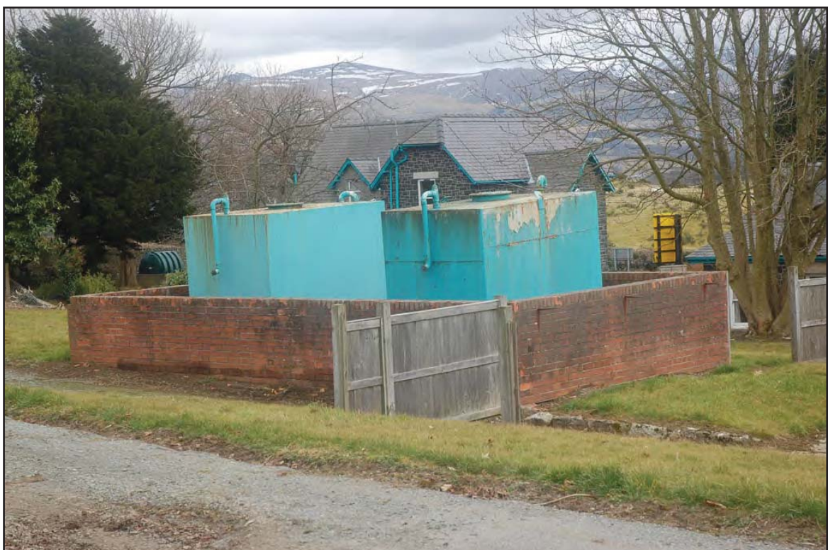
Plate 62: Oil Tanks: View southeast of oil tanks located towards rear of property. Enclosed by a low brick wall (Dearnes/Rat trap Bond). Accessed via site road that links all buildings within complex. Note administration block towards centre of image and views from the hospital site towards Snowdownia.
