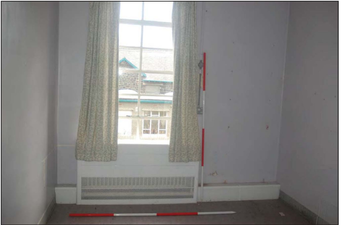
Plate 31: Short Stay Unit (Internal): View southeast of Room G07 detailing former use as a ward. Storage heater visible below original casement window, with boxed in plumbing (Scales: 2 x 2.0m)
