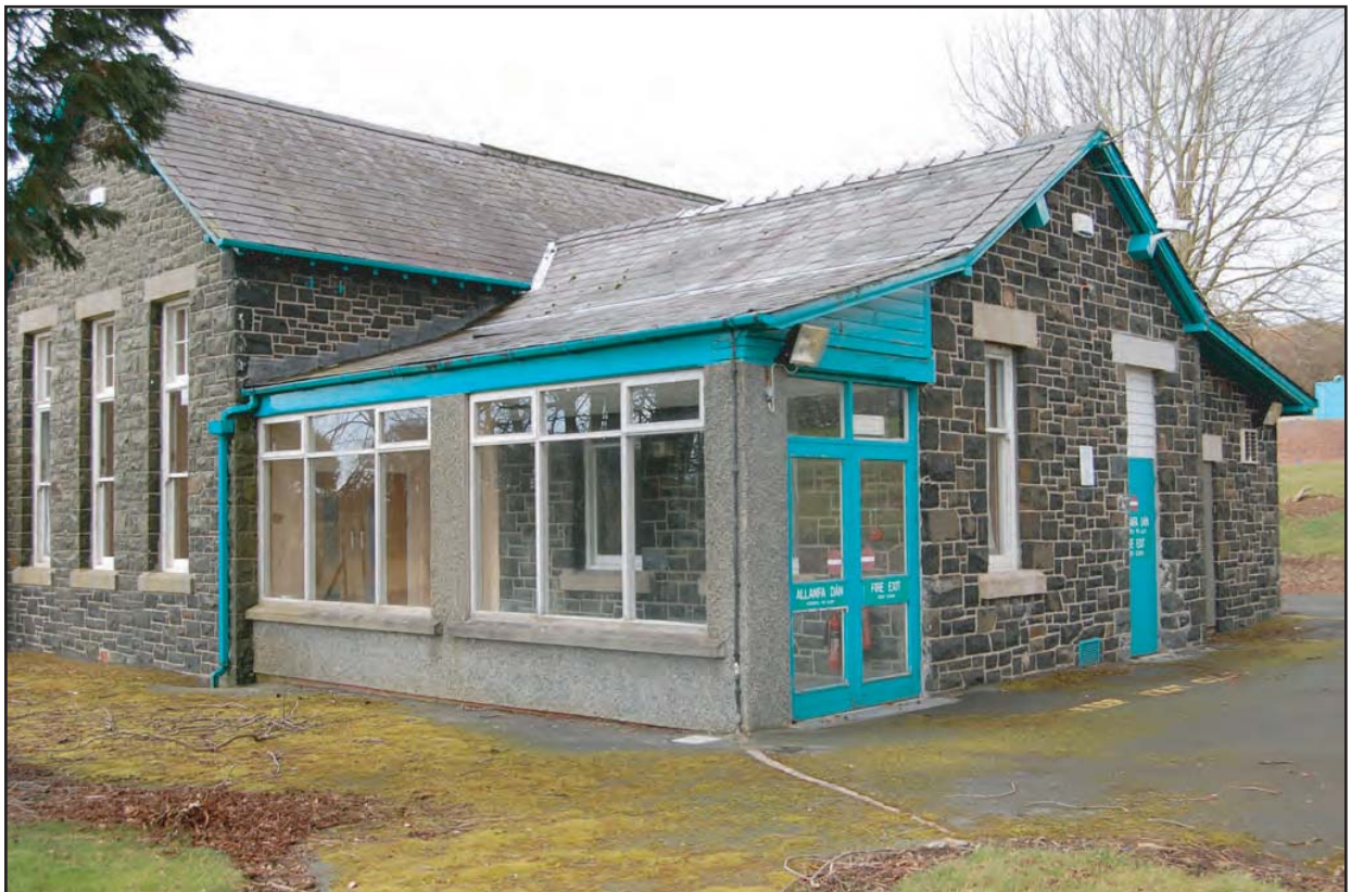
Plate 06: Long Stay Unit (External): Southeast and northeast facing elevations detailing original female wing (Room G11) and later extension (Room G12). The later extension was constructed between 1900 and 1914.
