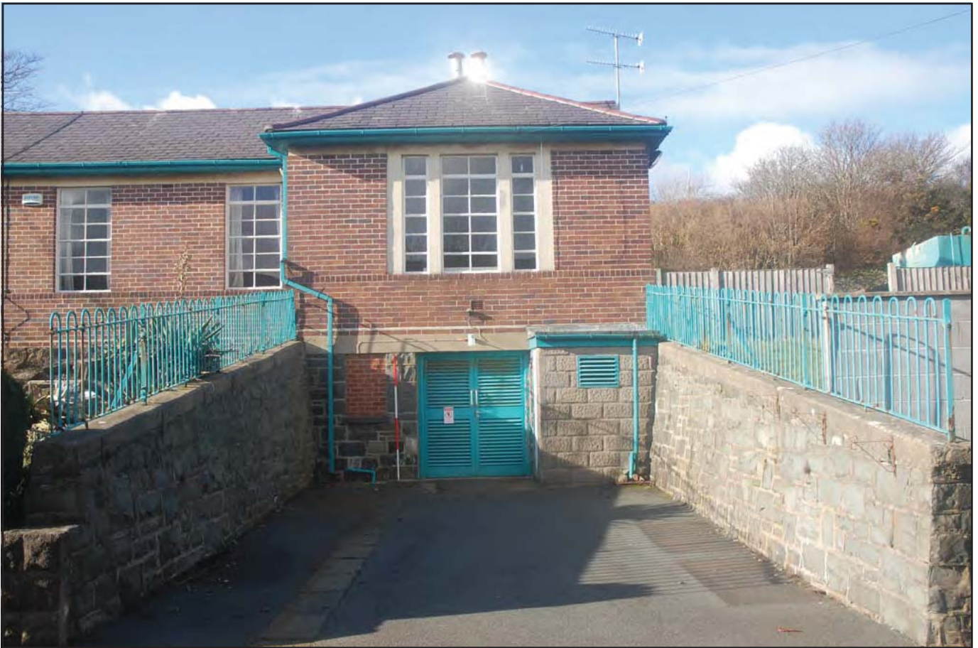
Plate 21: Short Stay Unit : Southeast facing elevation - Former Day Room (Room G01) and basement level boiler house; the latter includes a lean to annexe with a louvred window. The courtyard separating the Long and Short Stay Units is to the left of the image (Scale: 1x 2.0m)
