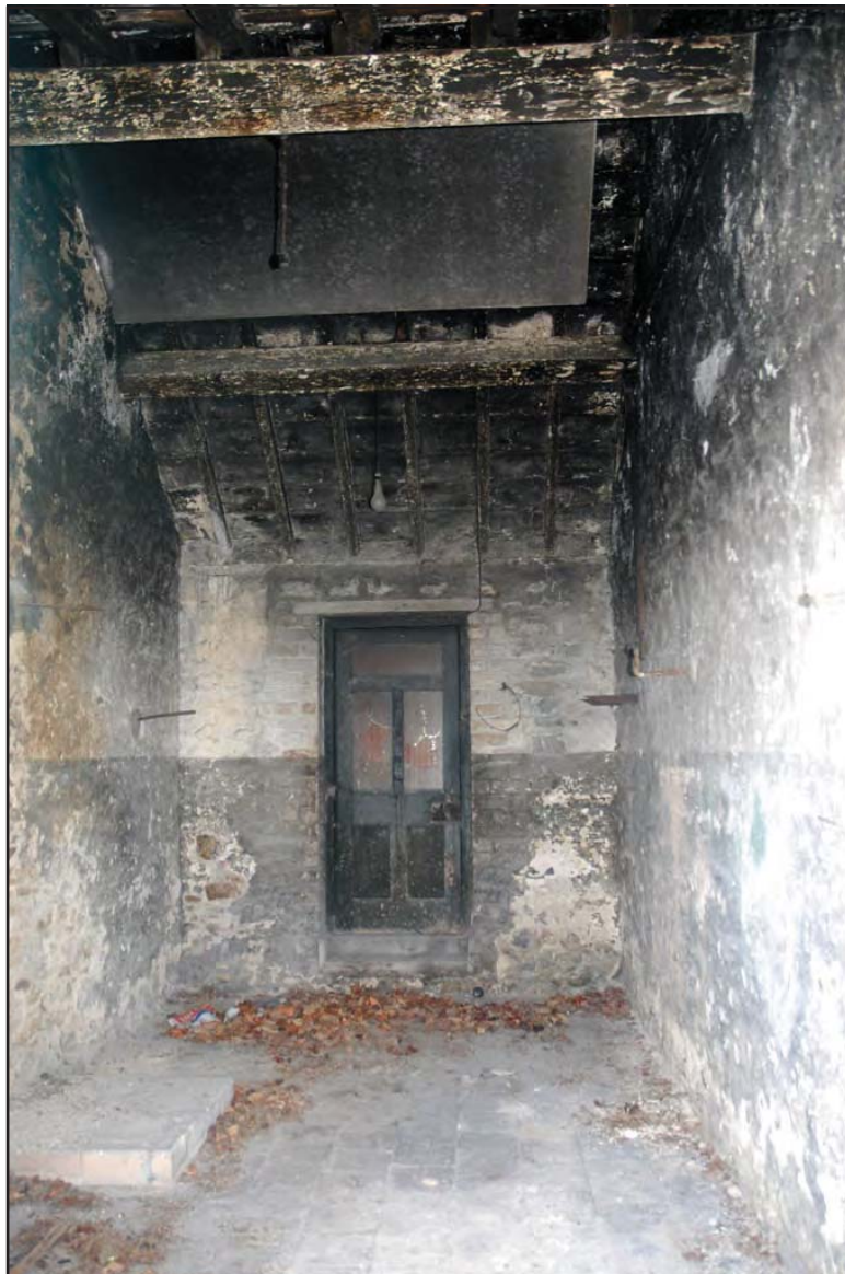
Plate 56: Garage (Internal): View northwest of main room interior detailing decor and usage: quarry tile floor, fireplace (?) plinth and roughcast walls. Rear door visible brick repair surround suggesting the door/entrance has been rebuilt or reused.
