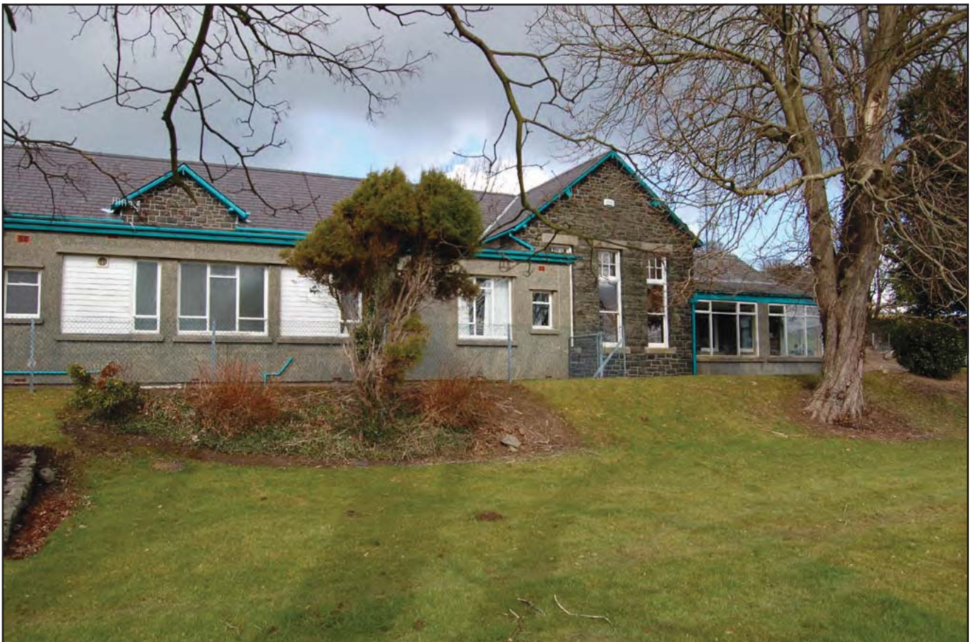
Plate 04: Long Stay Unit (External): Southeast facing elevation detailing late twentieth century flat roof extensions to the original structure. The Link Corridor is in the left foreground of image. The gable end of the female wing is also visible, detailing original structural style.
