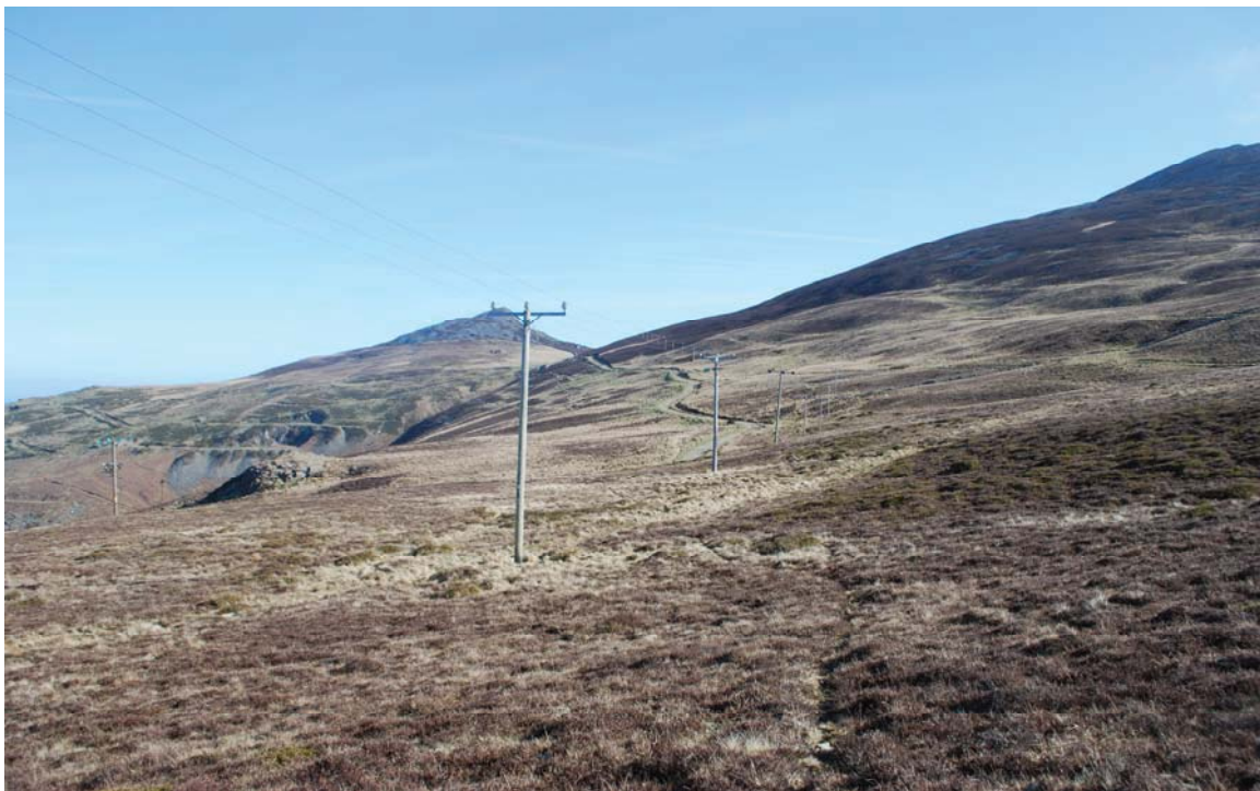
Plate 14 A general view of the current overhead cable route looking north towards Yr Eifl quarry
