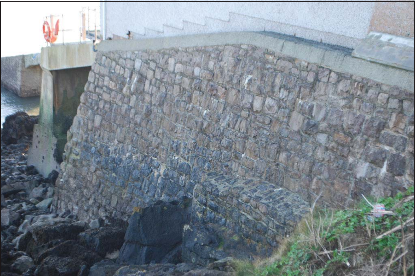
Plate 10 – The 1992 plinth extension to the north of the lifeboat house
