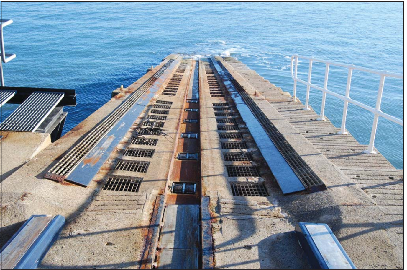
Plate 19 – The slipway, taken from the boat house
