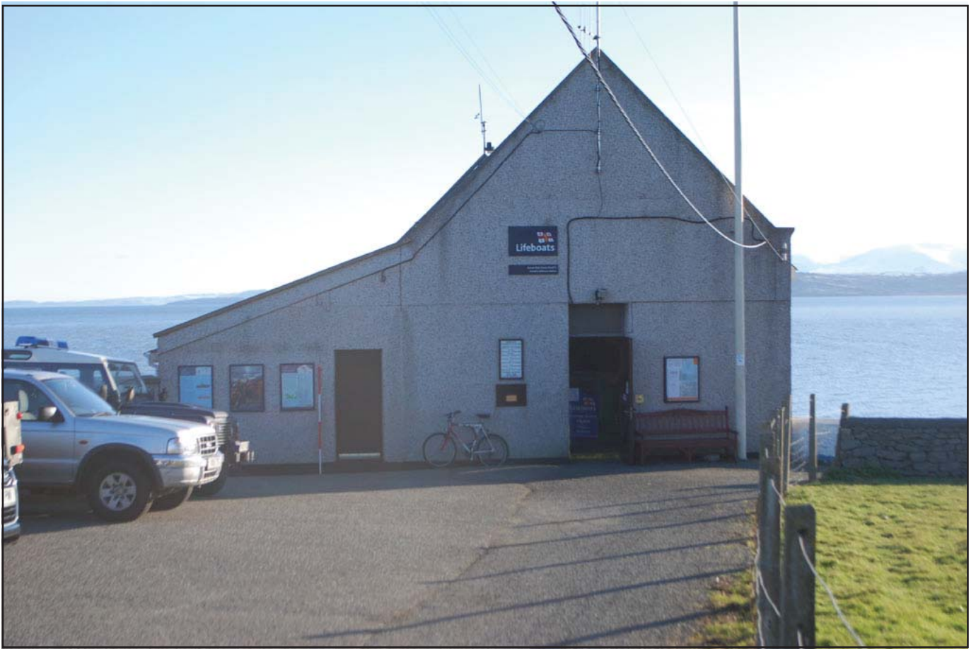
Plate 01 – Lifeboat station from the northeast
