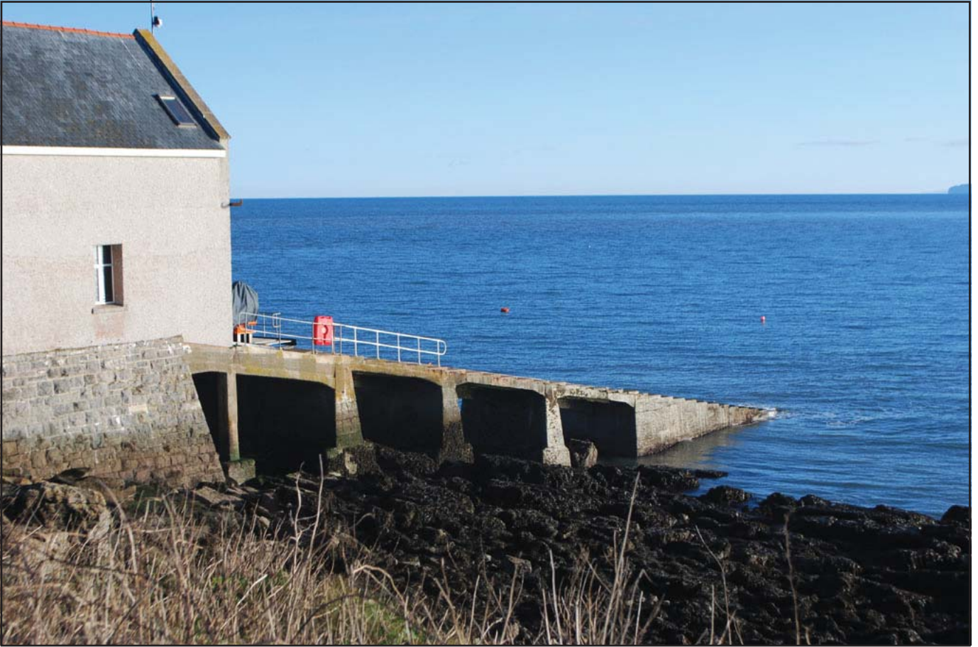
Plate 06 – Detail of concrete construction of slipway
