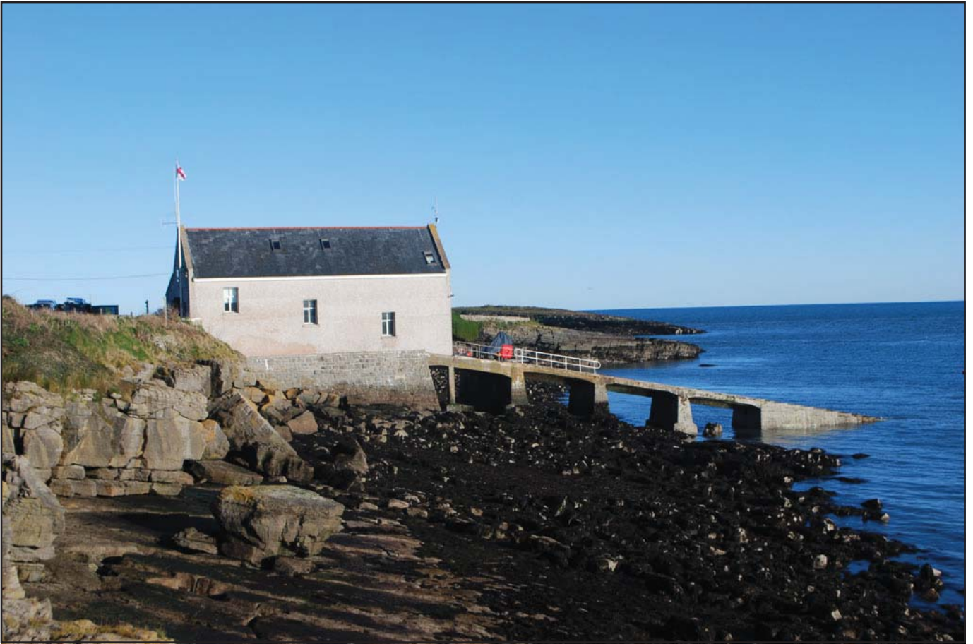
Plate 05 – The lifeboat station from the south; the 1983 adaption can be seen in the extension of the building in the first few metres of the slipway
