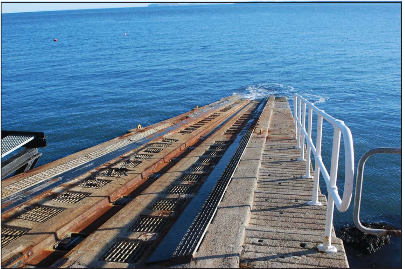
Plate 07 – The slipway from the west
