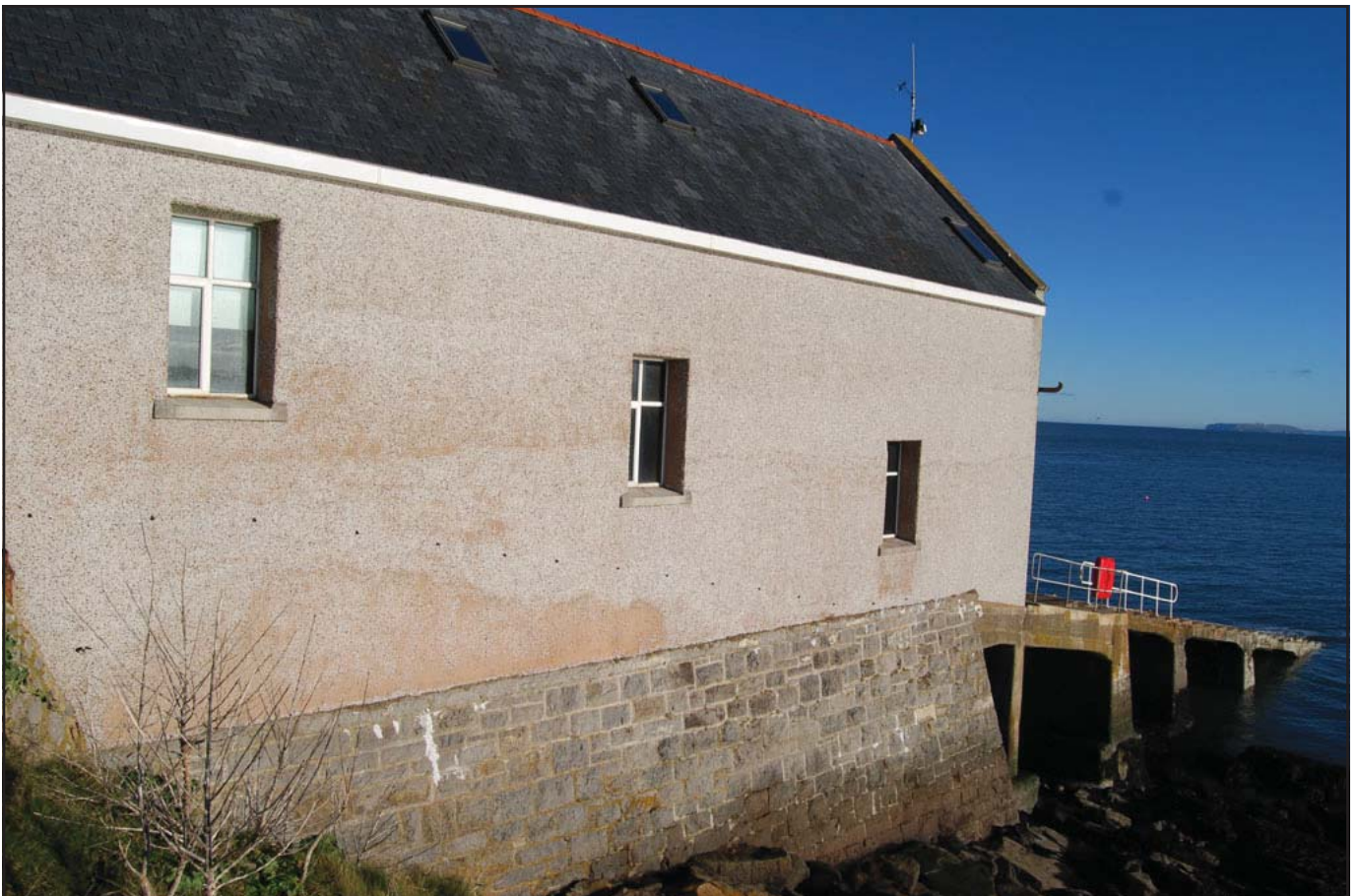
Plate 04 – 1909 plinth and later slipway of lifeboat house; the slope is reflected in the positioning of the lifeboat house windows
