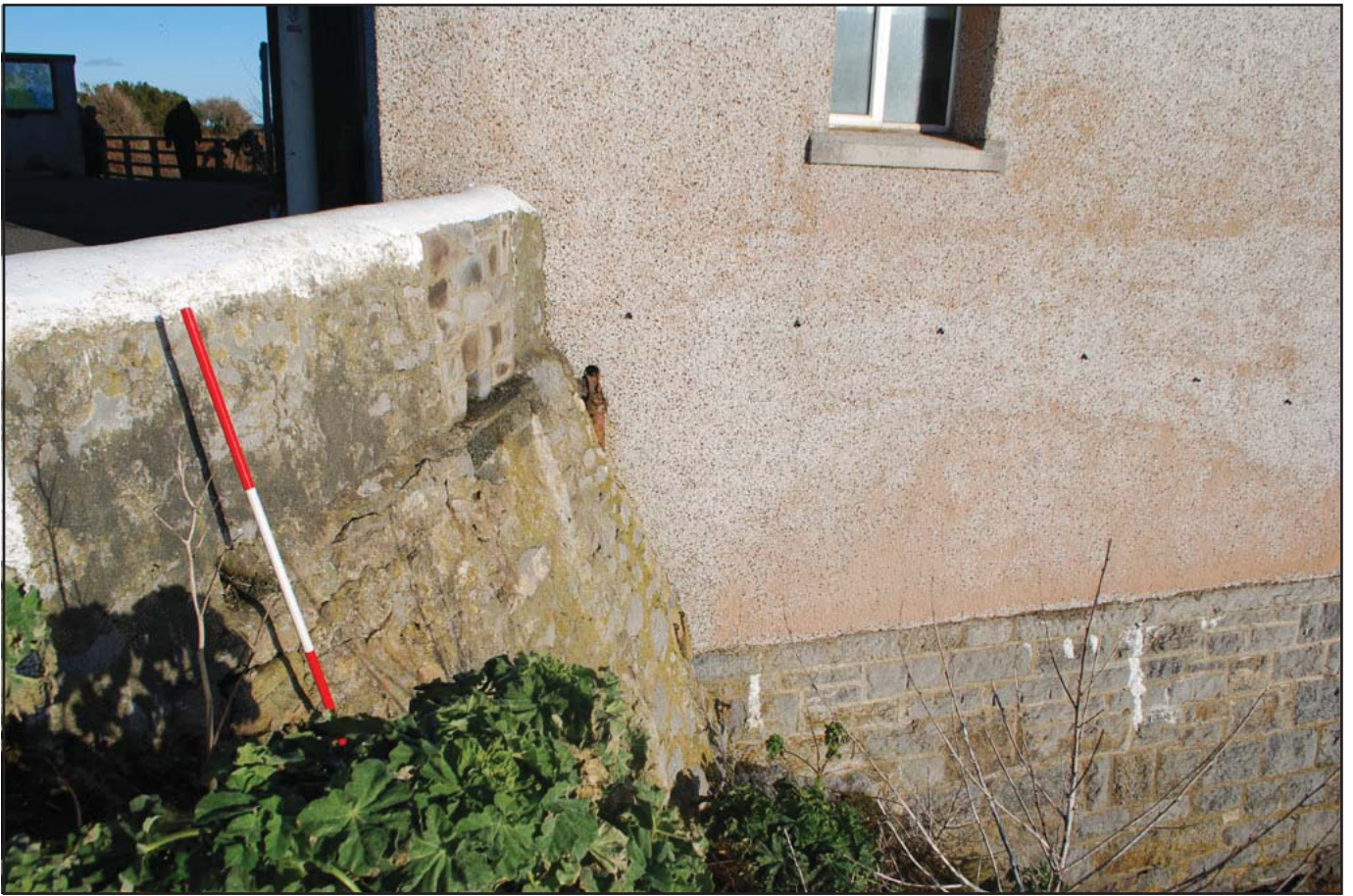
Plate 03 – Detail showing retaining wall south of lifeboat station; scale 2.0m
