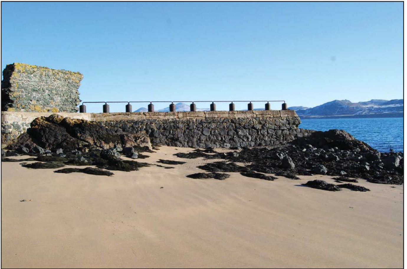
Plate 11 - Southwest oriented angle in breakwater, built 1918-1927
