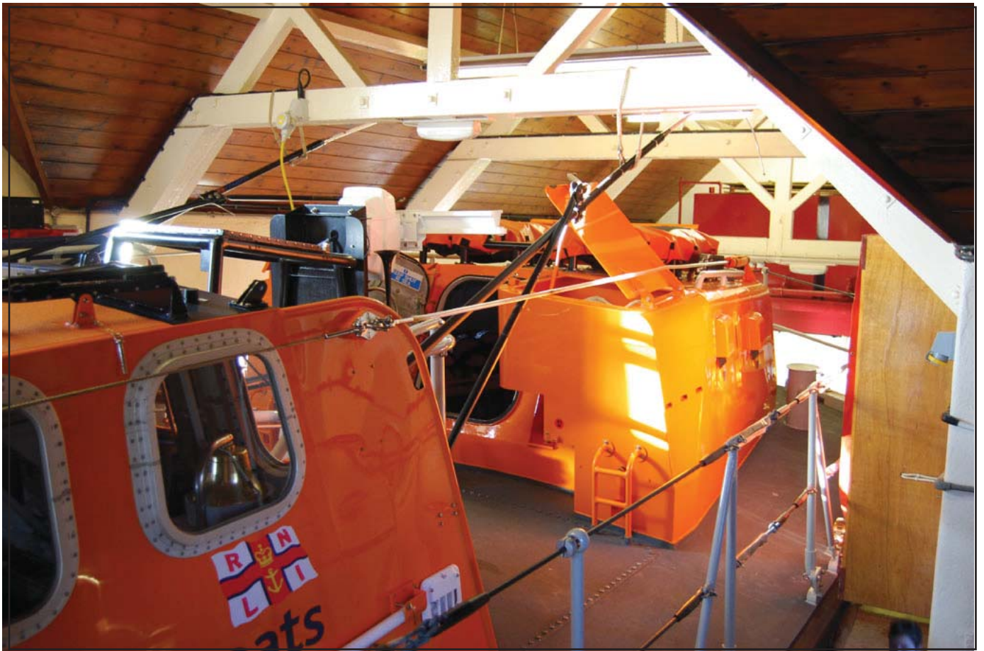
Plate 15 – Detail showing roof trusses
