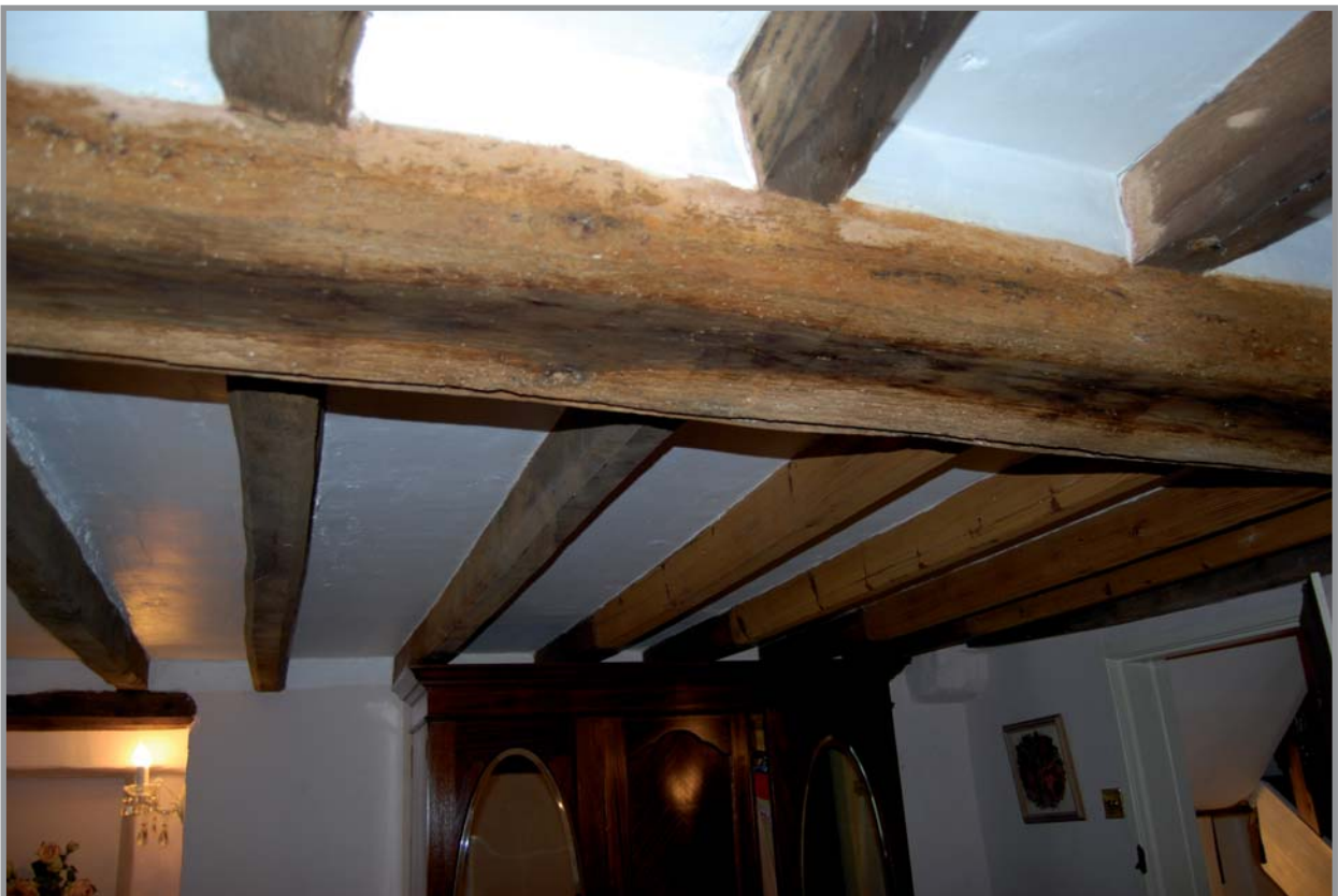
Plate 16: Front bedroom, showing chamfered beam. Facing south
