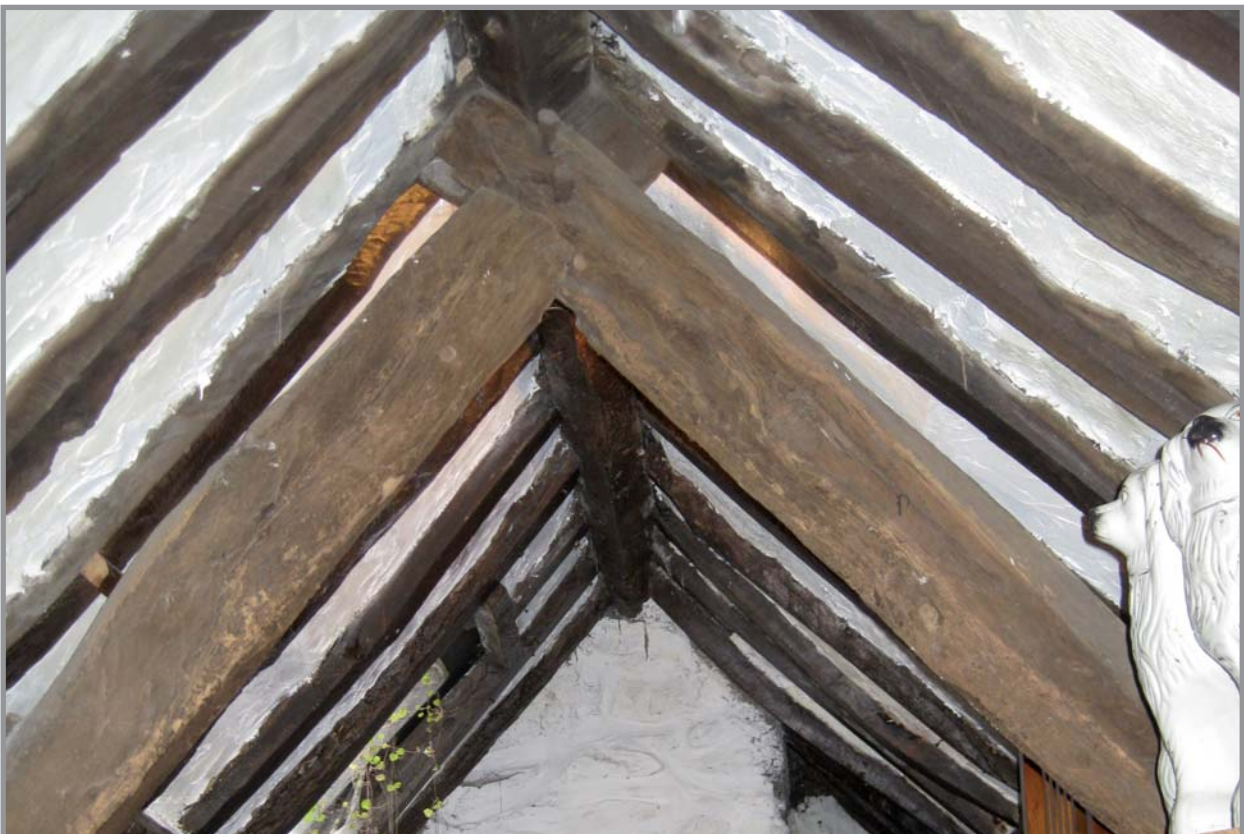
Plate 22: Truss 2 in attic room. Facing south-west
