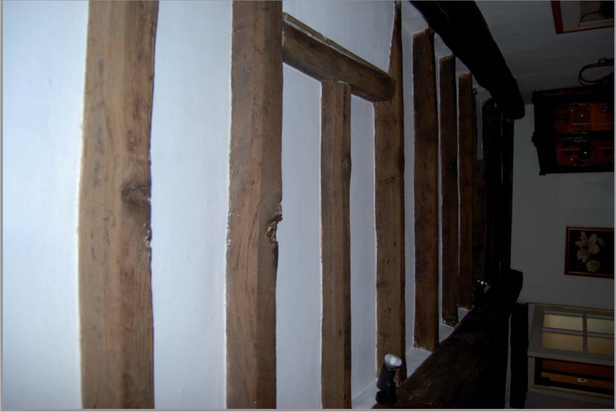
Plate 3: Ground floor living room, showing ceiling timbers. Facing north-west
