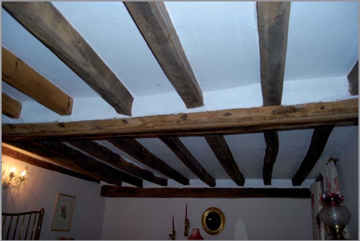
Plate 15: Front bedroom, showing ceiling timbers. Facing North-east
