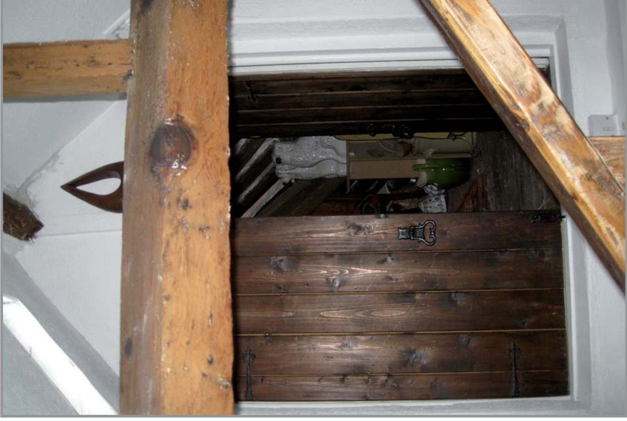
Plate 18: Door leading into attic, showing staircase to first floor. Facing north-west
