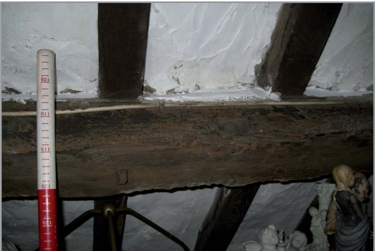
Plate 24: Attic room, showing timber detail. Facing north-west
