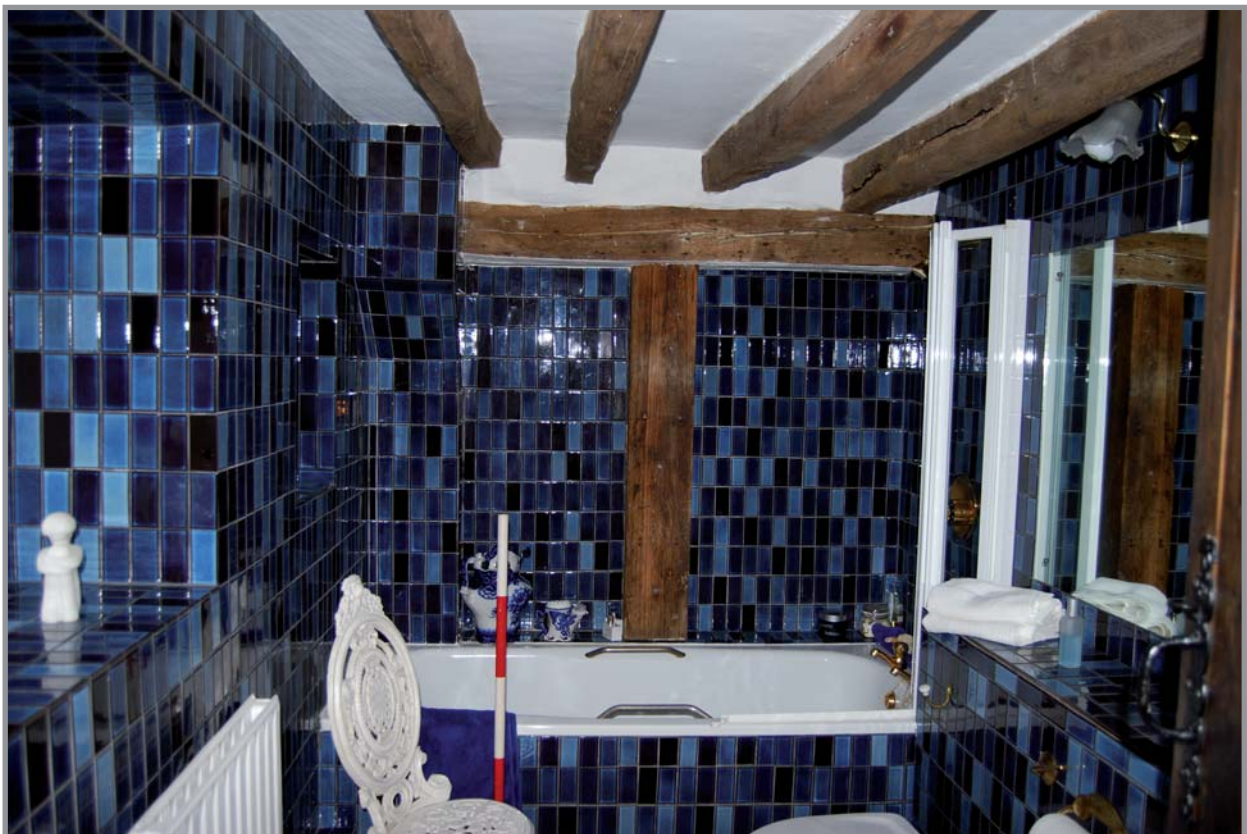
Plate 12: Bathroom, showing timbers. Facing north-west
