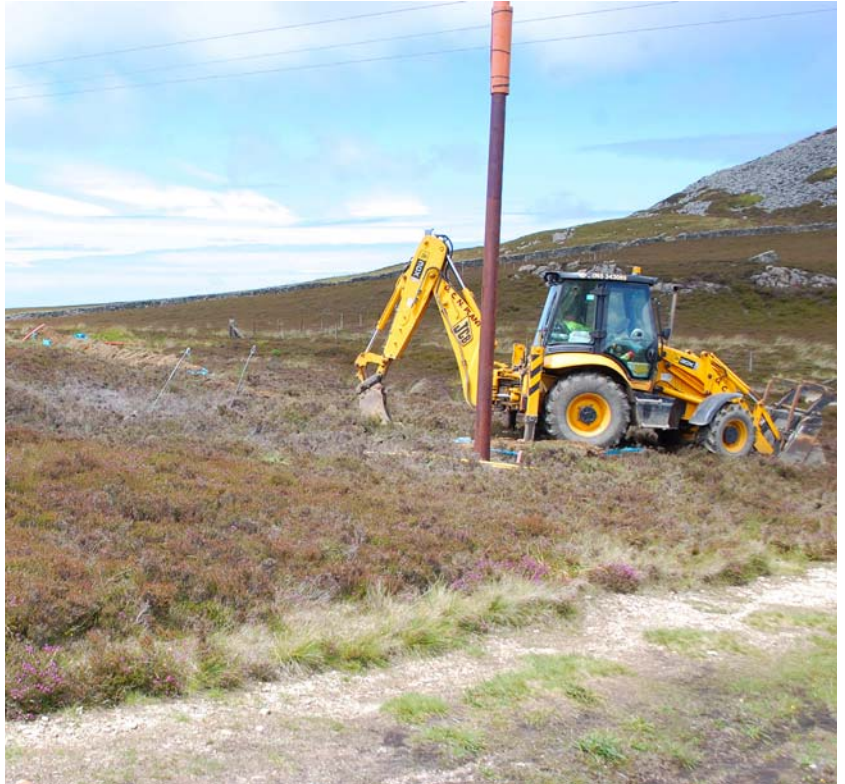
Above: Plate 06 - Excavation of footings for new pole 25A, about 30m from site 06. View from the north
