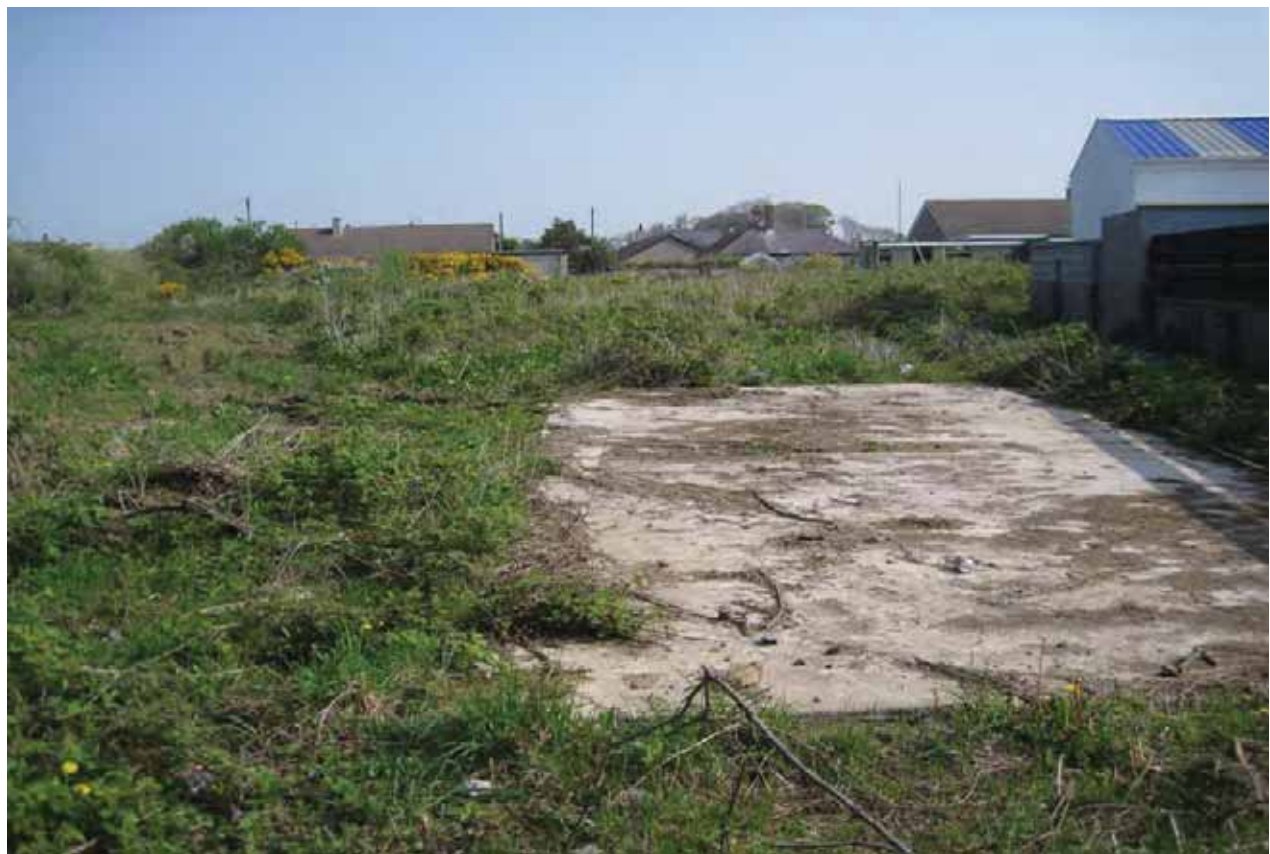
Fig. 10 A concrete pad within the development area, possibly a base for a former POW camp structure
