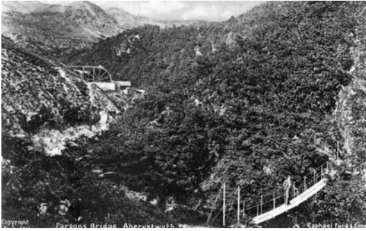
01) Temple Mine, old Parson's Bridge in foreground 1890
