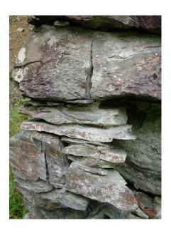
10) 40 foot wheel-pit - damaged stone southeastern corner (close up)
