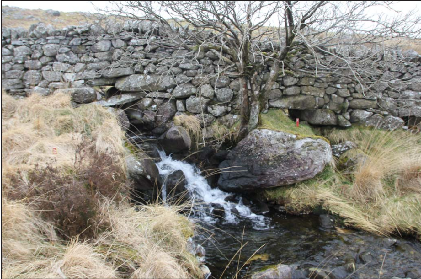
Plate 01: View of proposed hydro intake weir, from the northeast.
