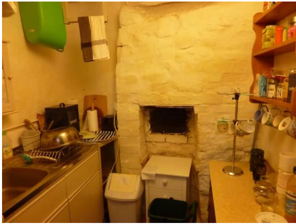
Fig.3 bread oven in cross wall between cottage and meeting room; inside the oven (right)
