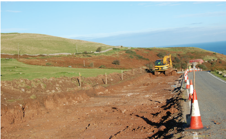
Plate 3: Trench dug for car park foundations, from SE
