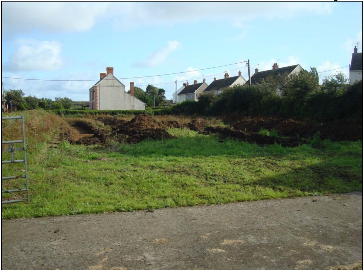
Plate 4: AS04 - Mechanically excavated trenches, looking south southeast
