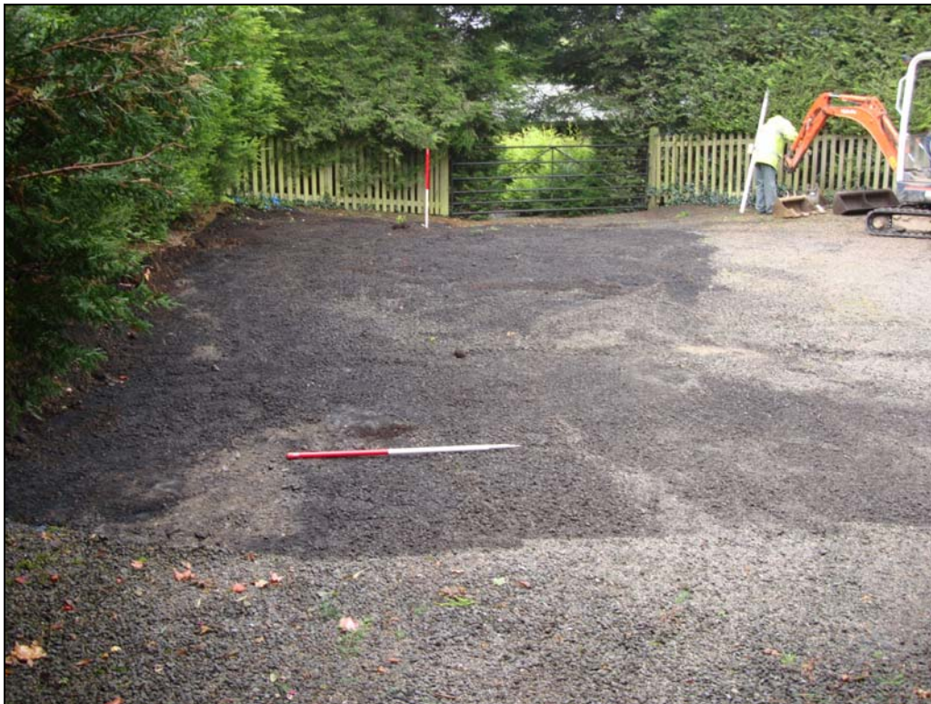
Plate 2: CBB002 – Initial levelling of the area, looking southwest.
