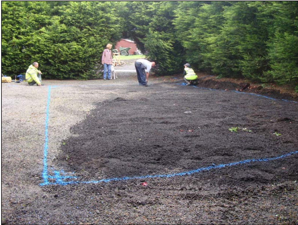
Plate 3: CBB003 – Marking out the trenches, looking east northeast.
