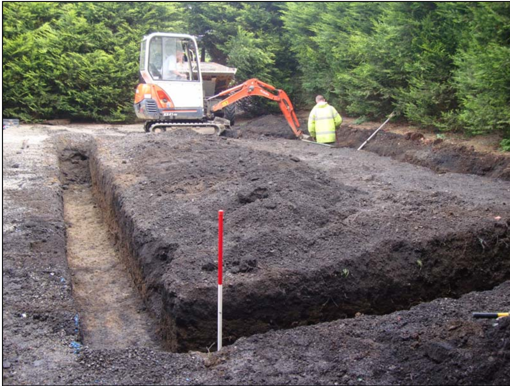
Plate 7: CBB007 – Trenches almost completed, looking east northeast
