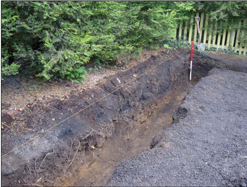
Plate 5: CBB005 – Trench section A to B, looking south southwest.
