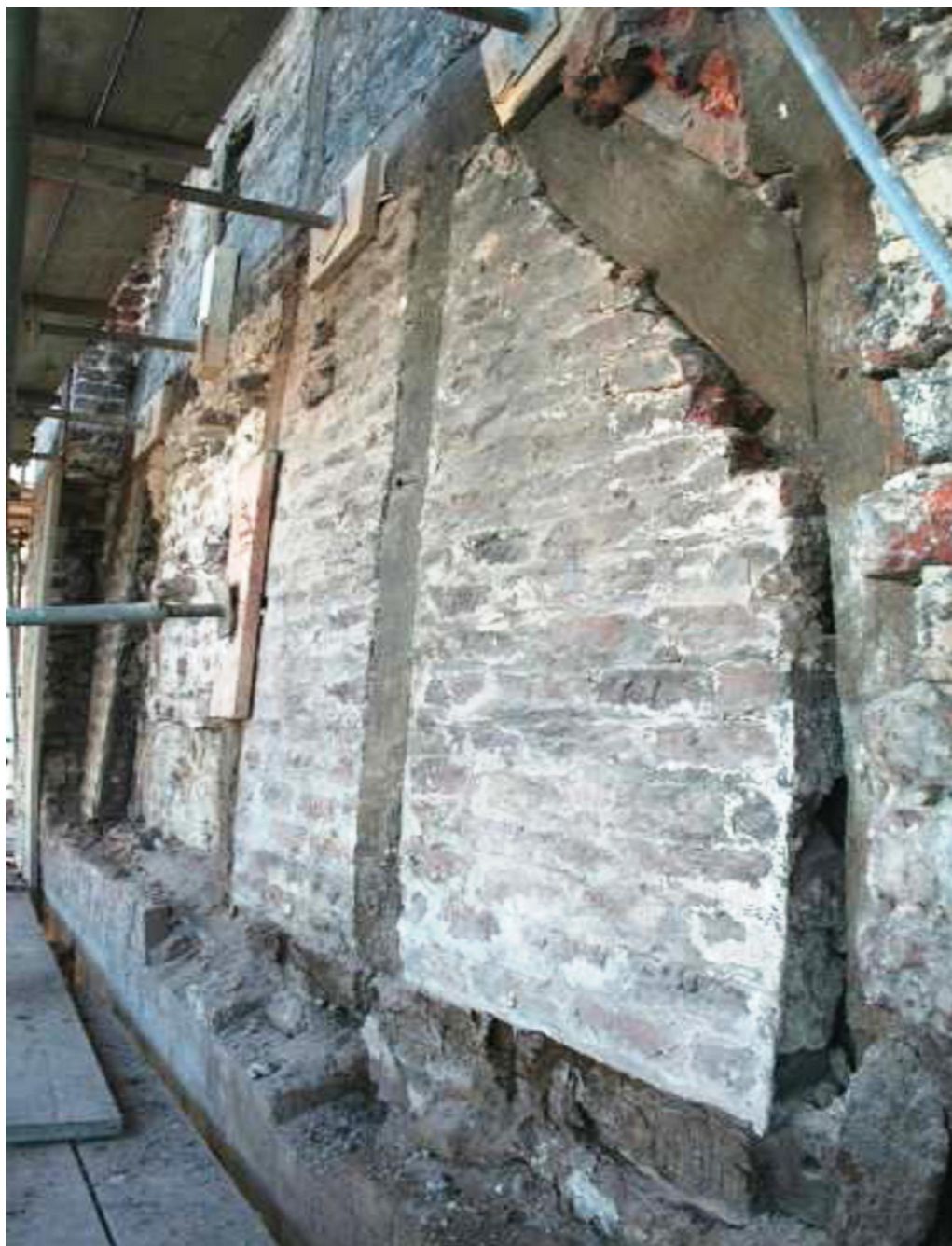
Fig. 8, Timber-framed truss-partition between tie-beam & girding-beam
