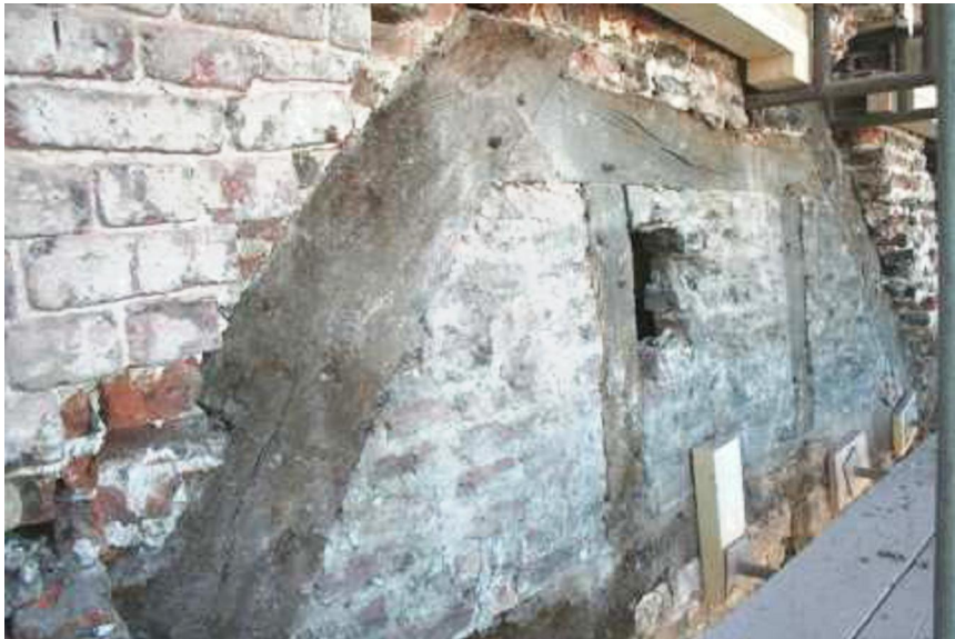
Fig. 7, Framed truss- partition between collar and tie-beam
