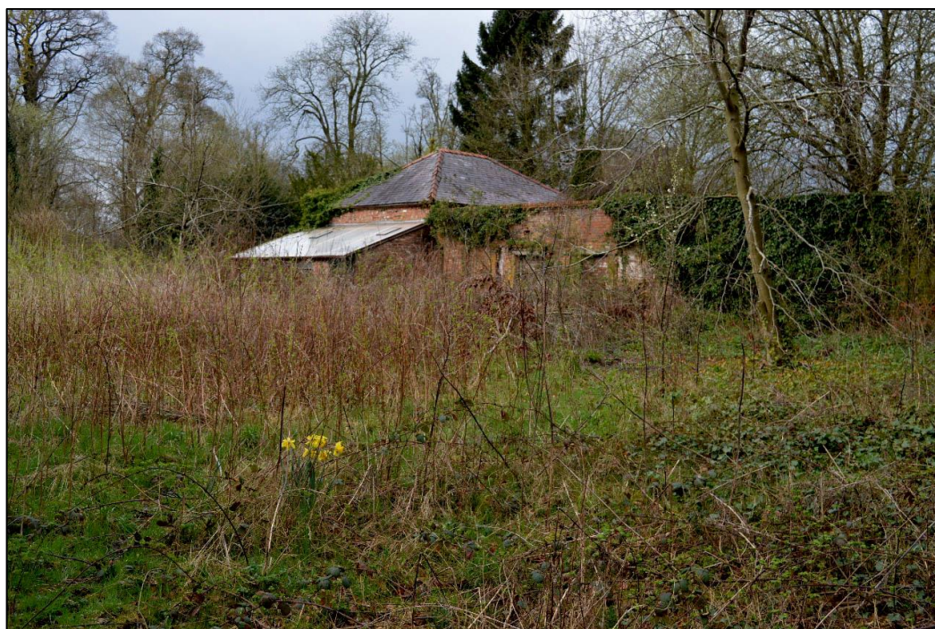
Fig. 6 View from the north-east across the former site of the hall showing the housekeeper's cottage and surviving west wall Photo CPAT 4486-0038
