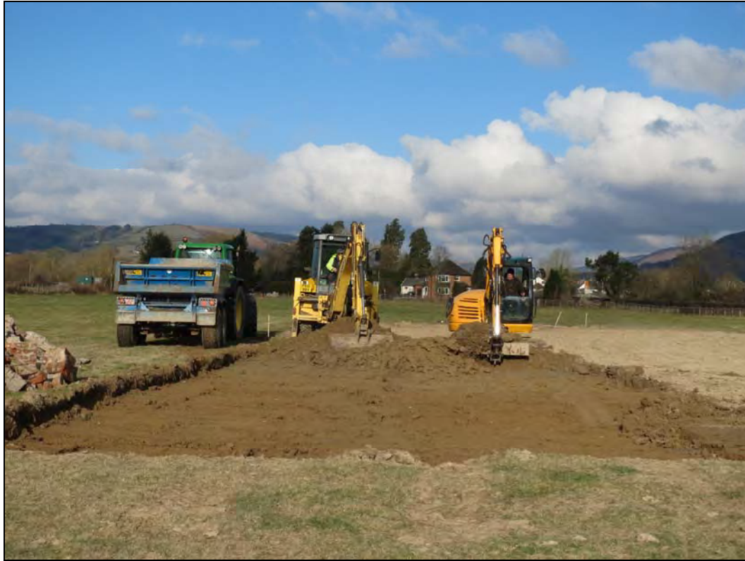
Plate 1. Soil strip at the southern corner of the site. Looking northwest.
