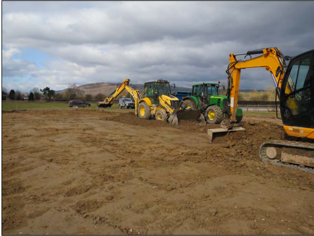
Plate 3. Soil strip across the central part of the site. Looking north.
