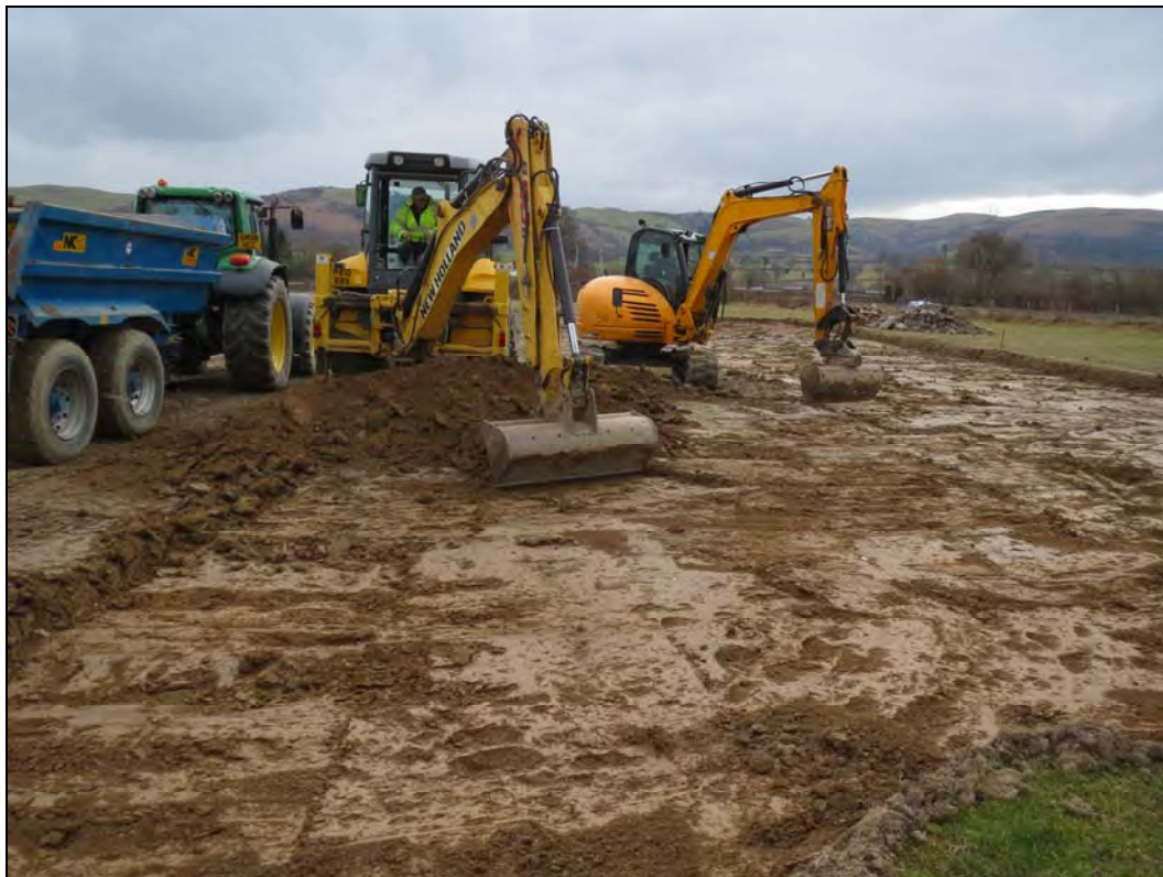
Plate 2. Soil strip within the northwest part of the site. Looking southeast.
