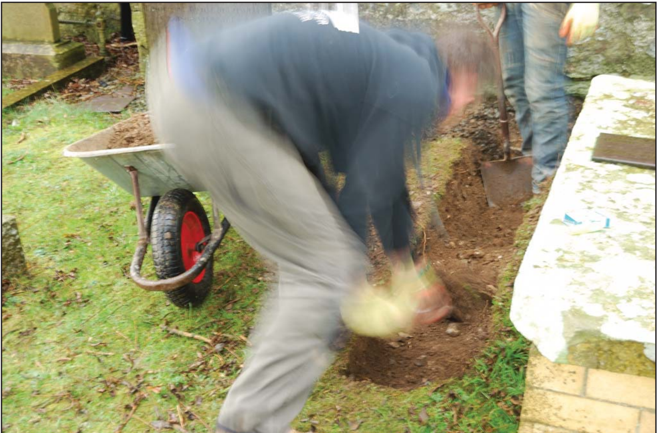
Plate 02: Manual excavation of pipe trench. (photographic archive ref. G2488_003)
