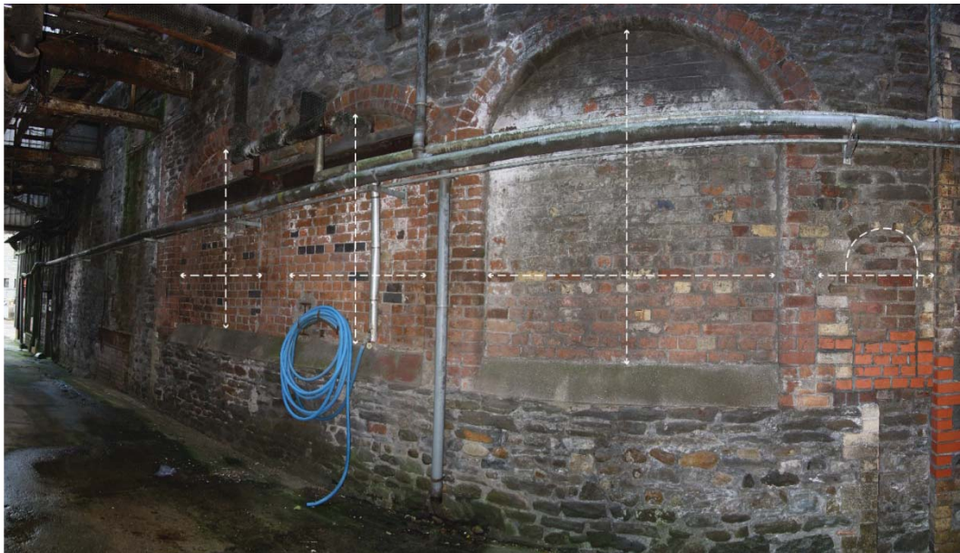
Figure 4.1 Infilled openings to northern facade (stitched photo)
