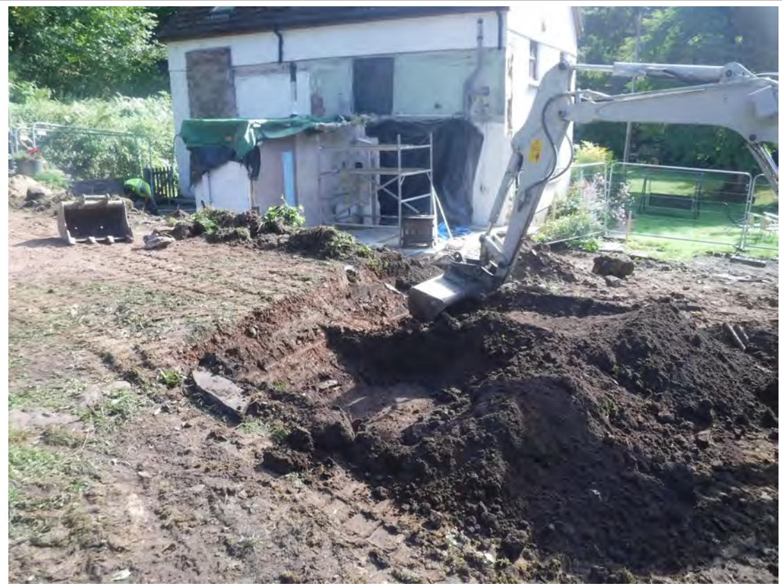
Plate 1. Overview of Retaining Wall Area.
