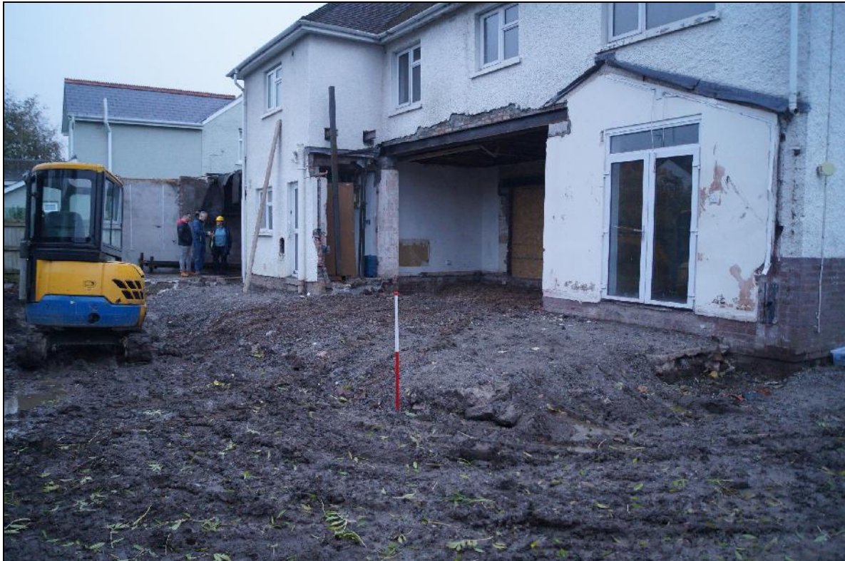
Plate 3: RCH2018_103, General view of the development area, looking southeast.
