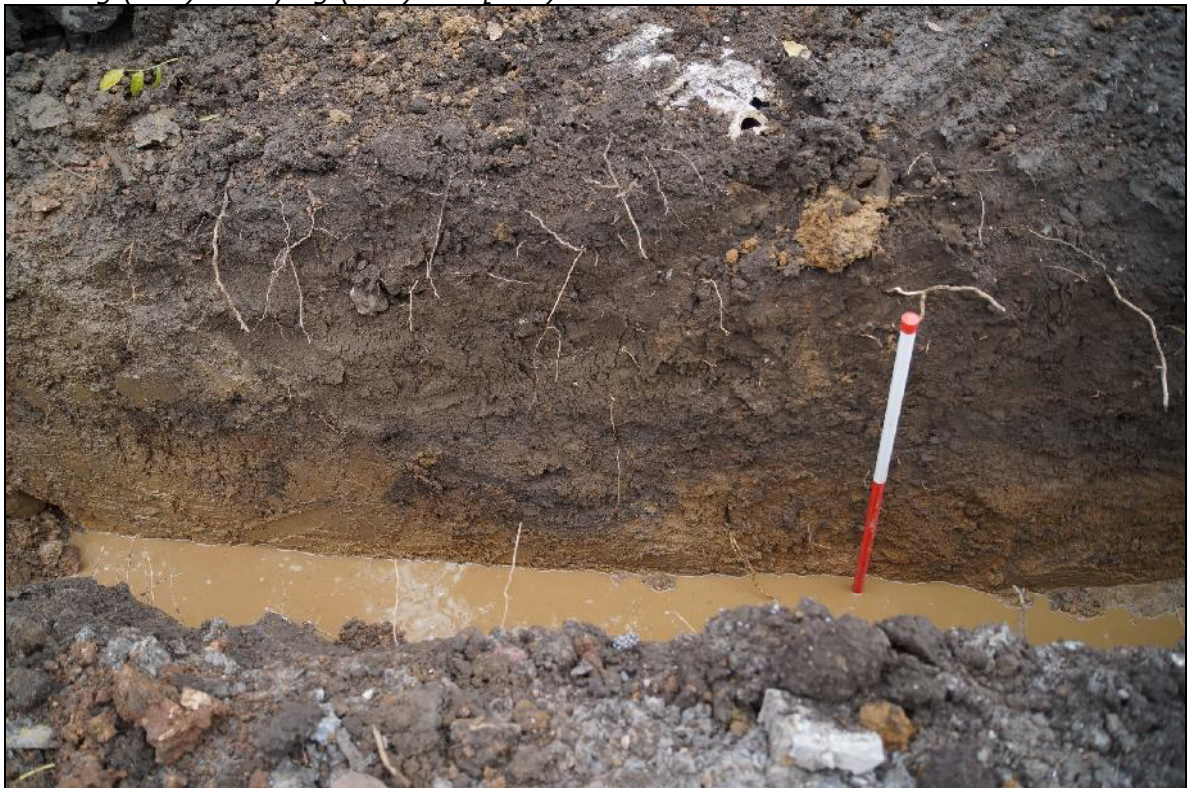
Plate 8: RCH2018_108, Northern part of the foundation trench, looking northeast showing (005) and [006] and subsoil (009). Contexts (002) and (001) overlying.
