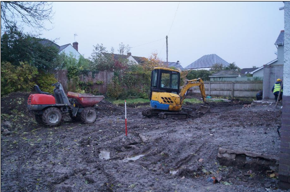
Plate 2: RCH2018_102, General view of the development area, looking east.
