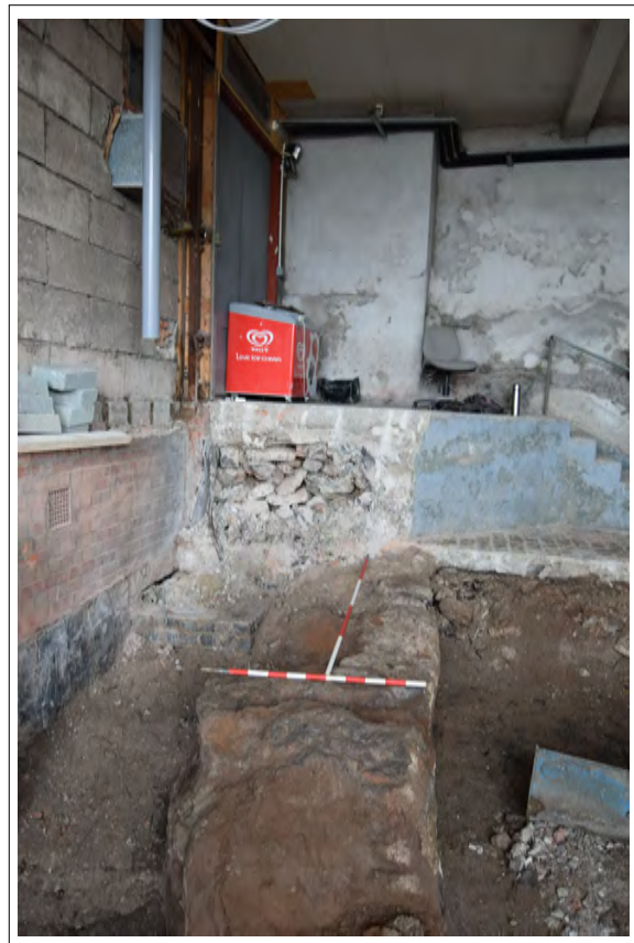
Plate 6. View of Wall (001). Looking south-southwest. Scales 1m & 2m
