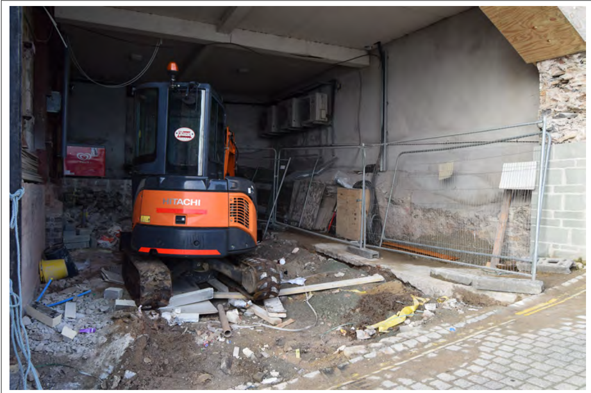
Plate 1. The Site, works commencing. Looking southwest.
