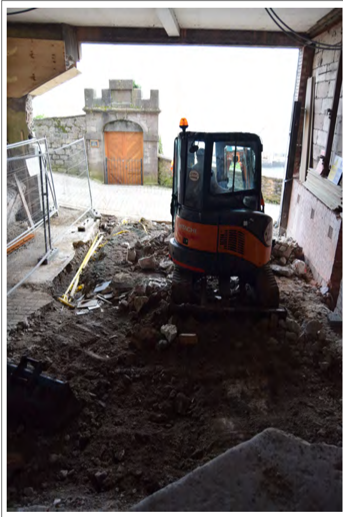
Plate 3. Discovery of Wall (001). Looking north-northeast.
