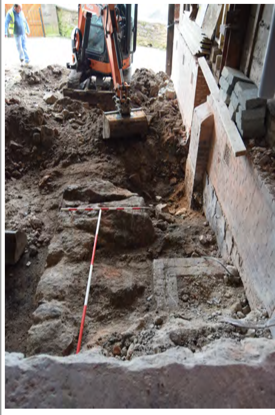
Plate 5. View of Wall (001). Looking north-northeast. Scales 1m & 2m
