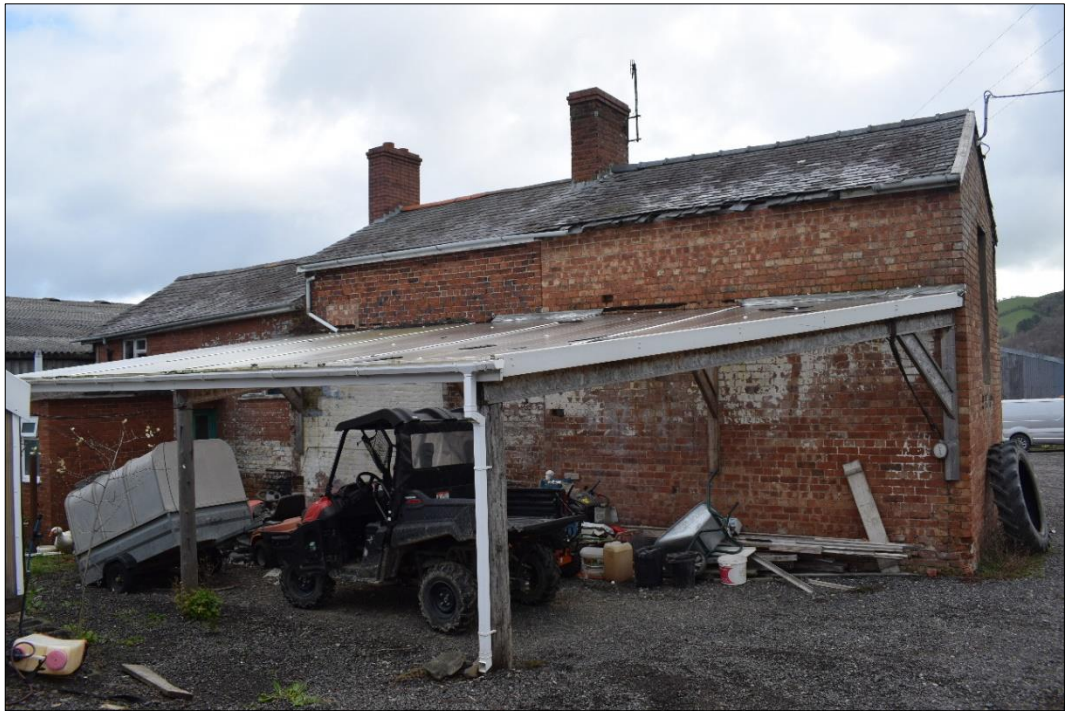
Fig. 11 The western elevation. Photo CPAT 4630-0006
