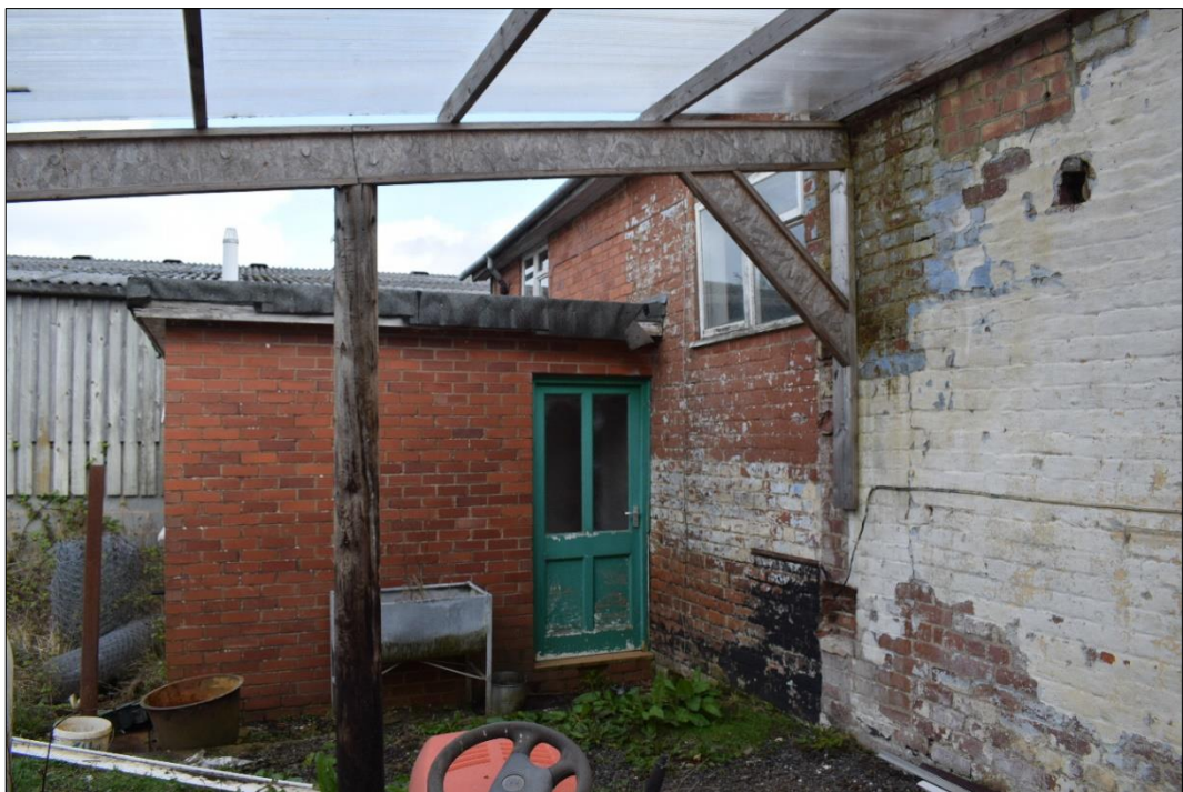
Fig. 12 The western elevation, showing the extension and blocked first-floor window on the landing. Photo CPAT 4630-0011
