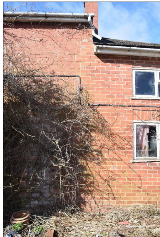
Figs 9 and 10. The eastern elevation showing the joints between the original house and the store (left) and later rebuild (right). Photos 4630-0014 and 15
