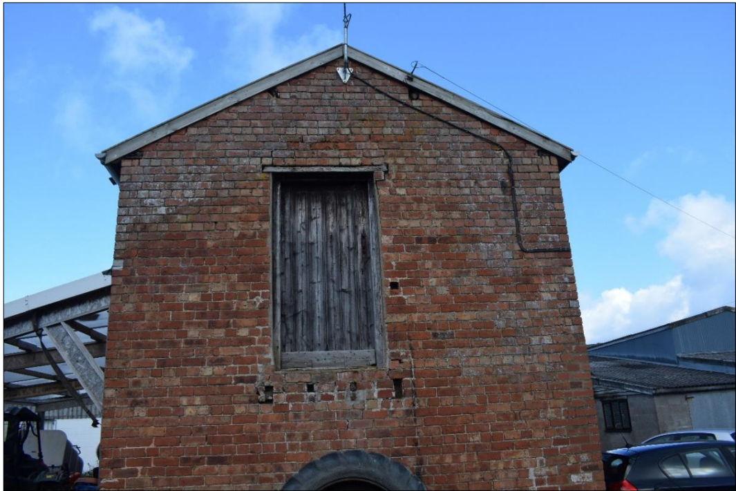
Fig. 13 The southern gable end showing the first-floor access and sockets for landing and handrail. Photo CPAT 4630-0013
