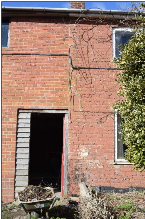
Figs 9 and 10. The eastern elevation showing the joints between the original house and the store (left) and later rebuild (right). Photos 4630-0014 and 15
