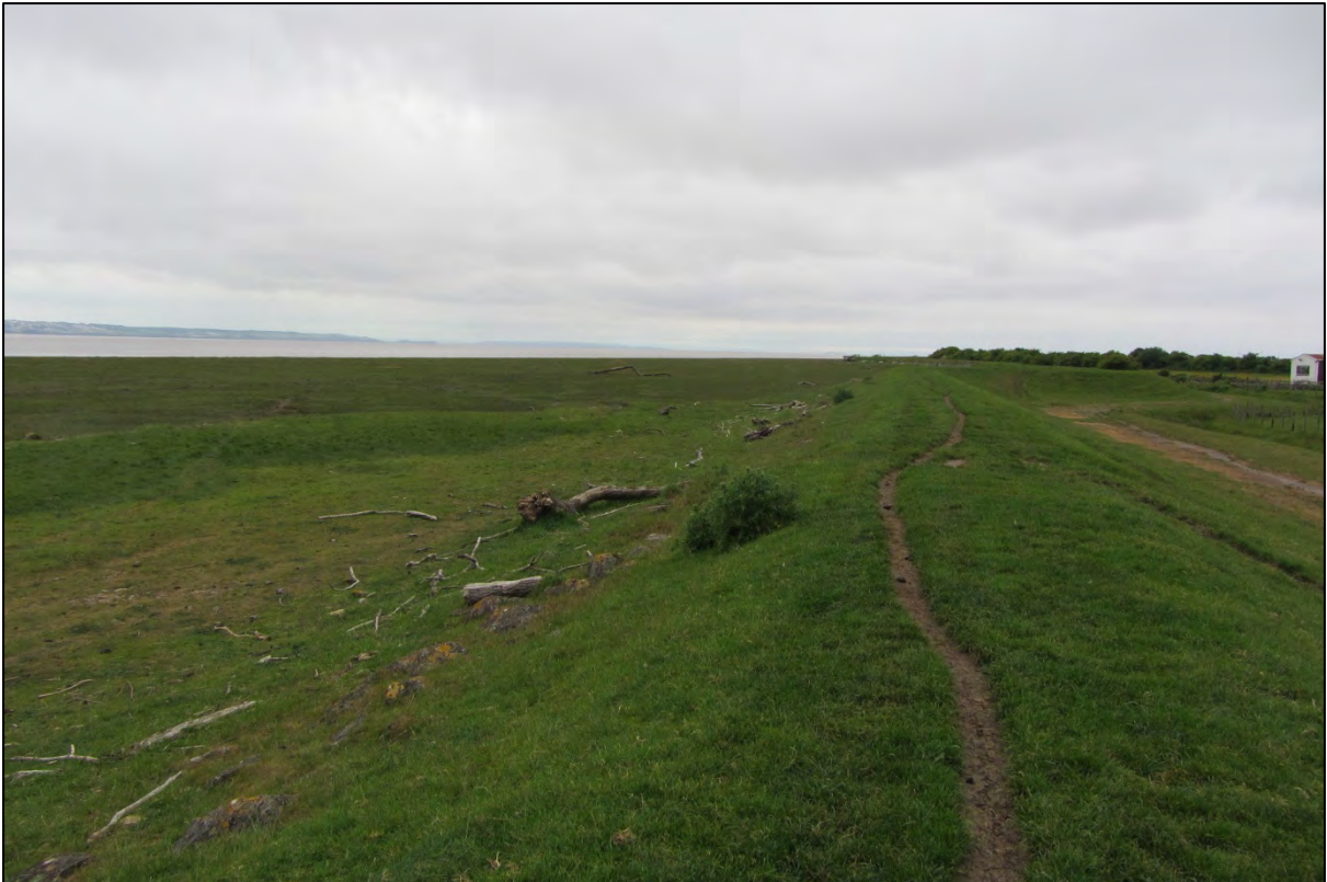
Photo 0-1 Existing embankment at Portland Grounds (looking West)
