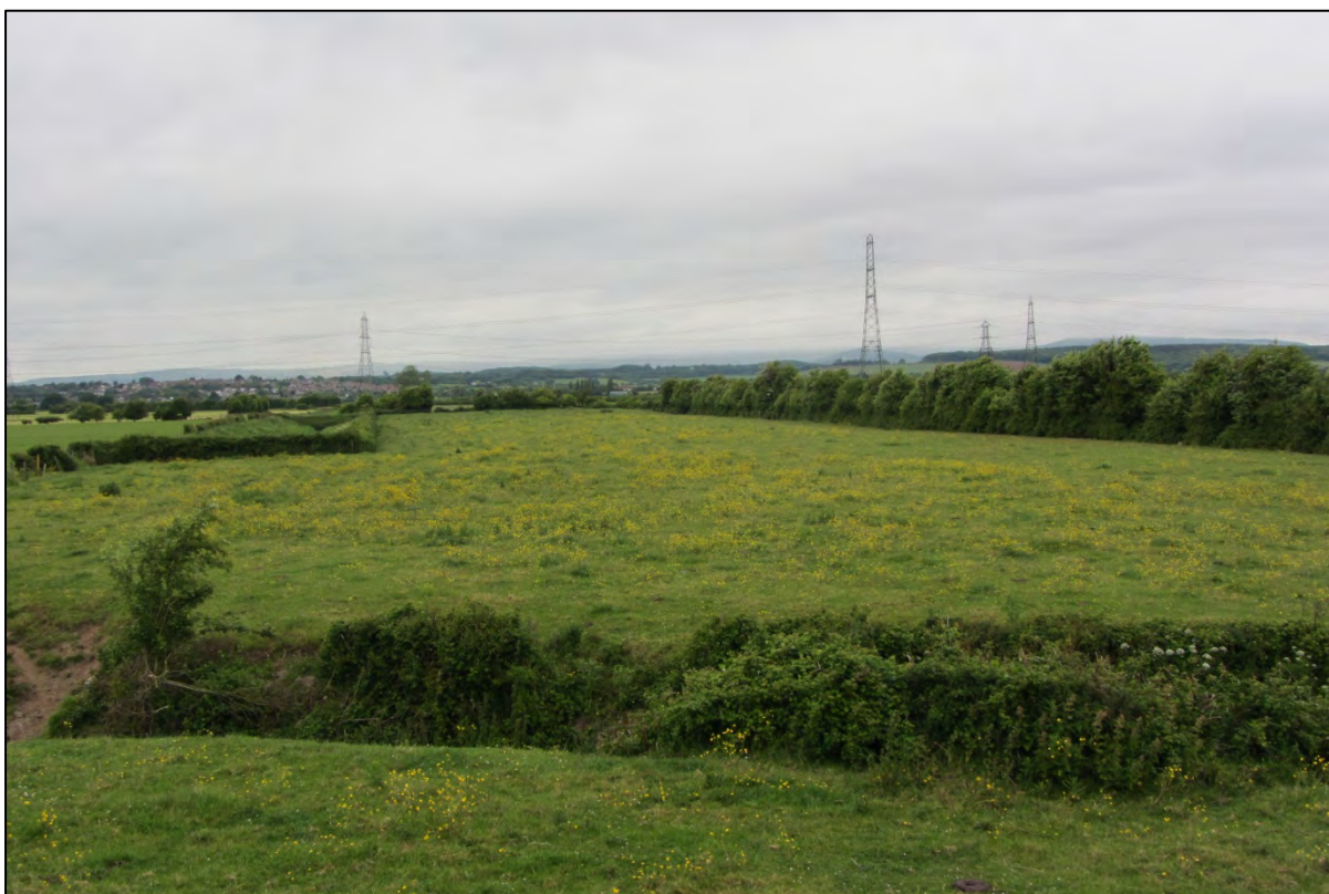
Photo 8-2 View of the landward side of the Portland Grounds embankment.
