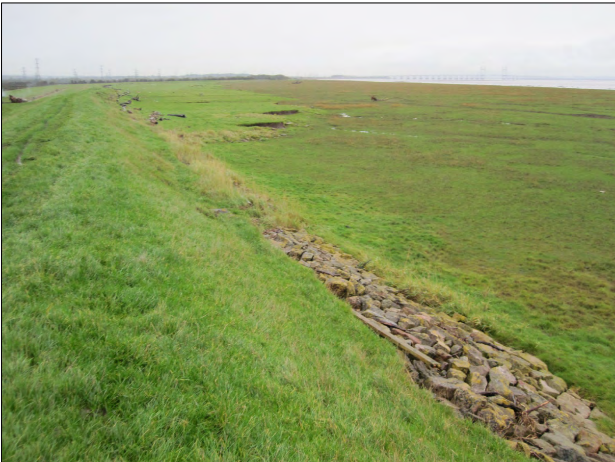
Photo 8-1 View of the seaward side of the embankment at Portland Grounds
