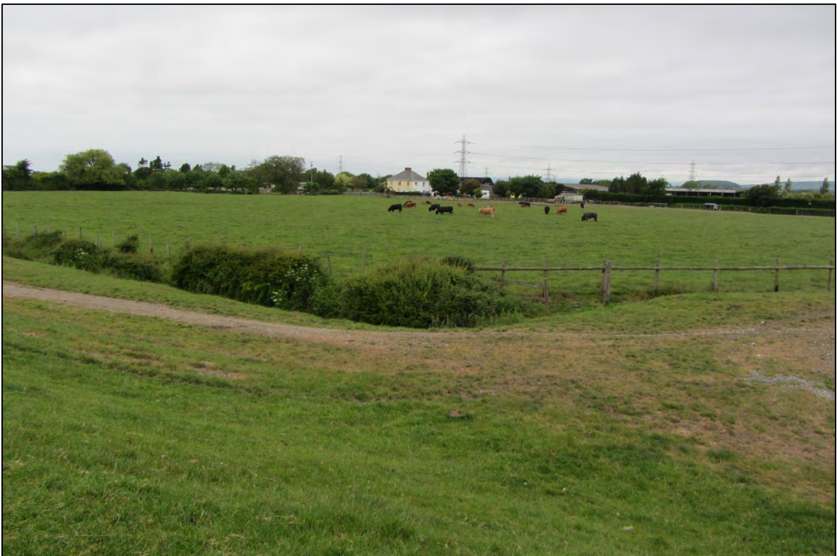
Photo 0-2 Inland of the embankment at Portland Grounds
