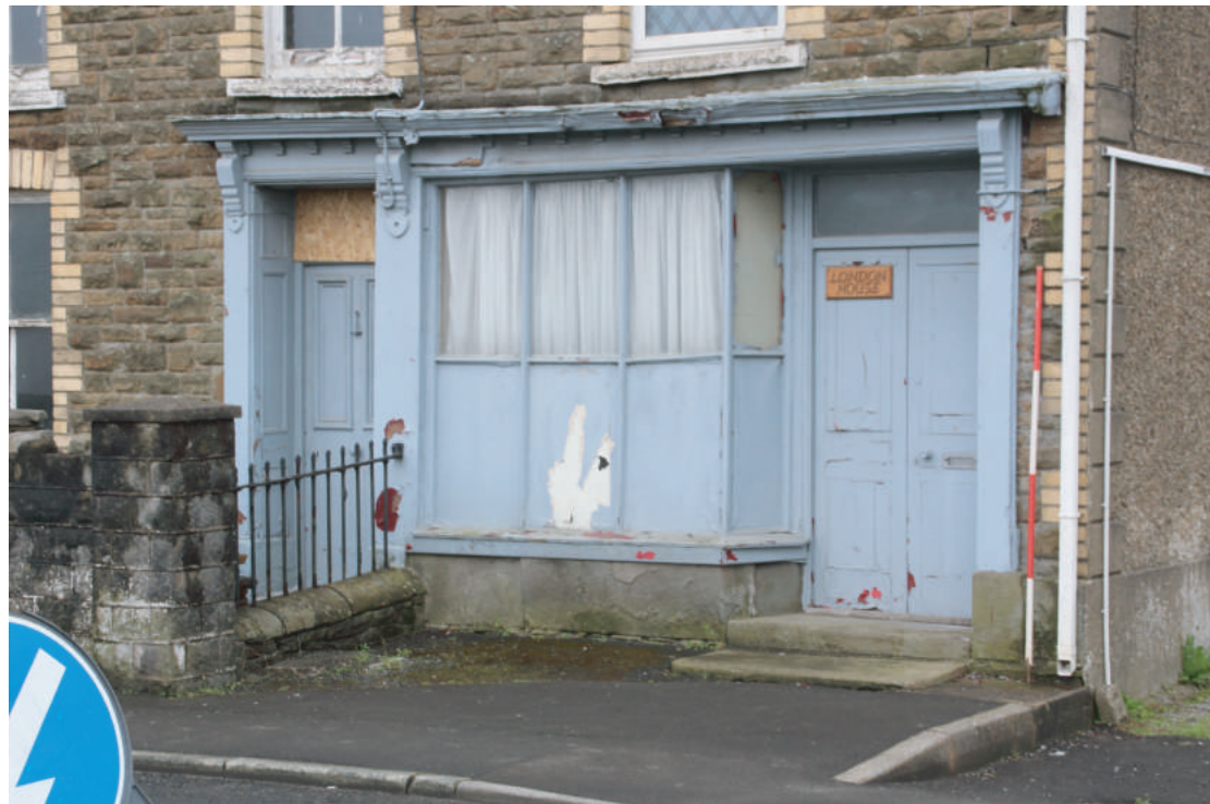
Plate 10. London House, Beach Road, Penclawdd. Early shopfront. Looking southeast.
