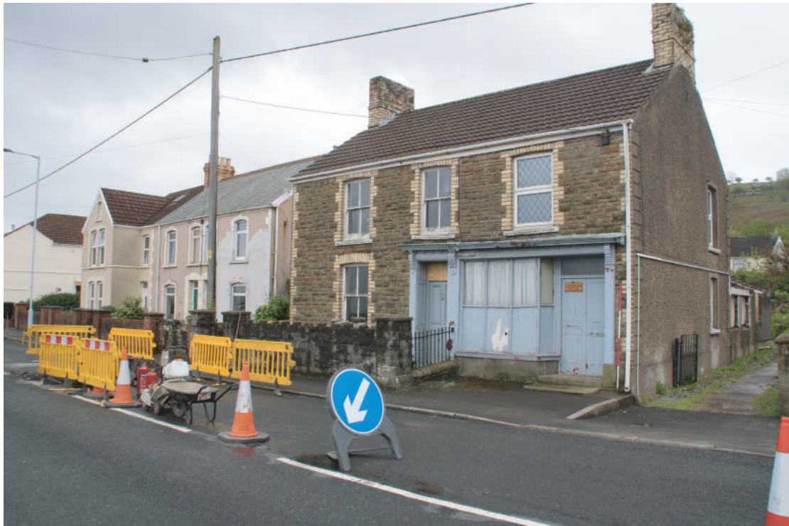
Plate 05. London House, Beach Road, Penclawdd. Looking southeast.
