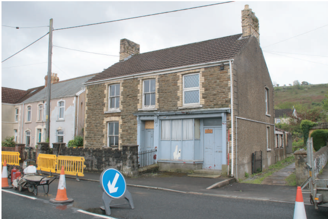
Plate 07. London House, Beach Road, Penclawdd. Looking southeast.
