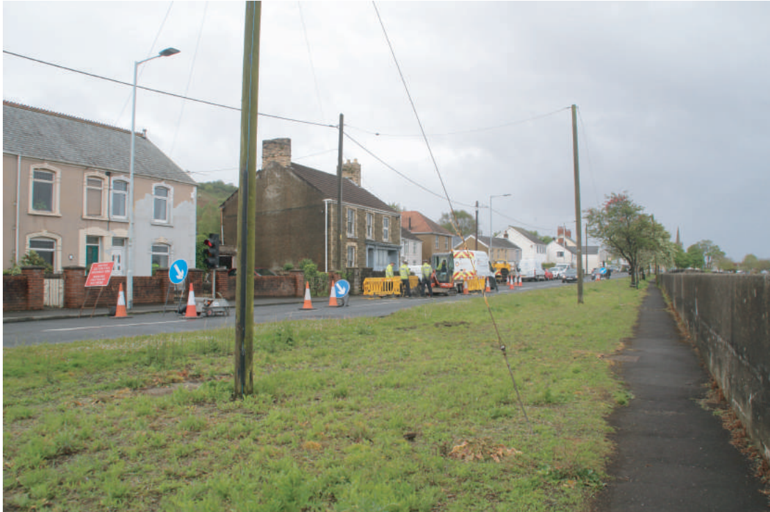
Plate 01. London House, Beach Road, Penclawdd. Looking southwest.
