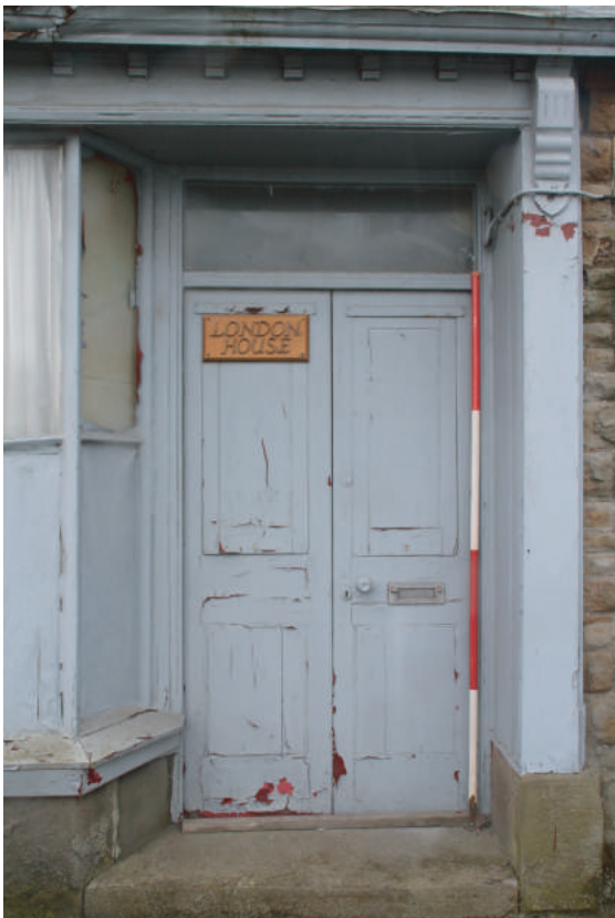
Plate 15. London House, Beach Road, Penclawdd. Shopfront doorway. Oblique view. Looking south.
