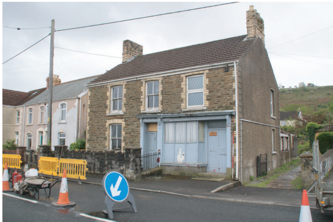
Plate 06. London House, Beach Road, Penclawdd. Looking southeast.
