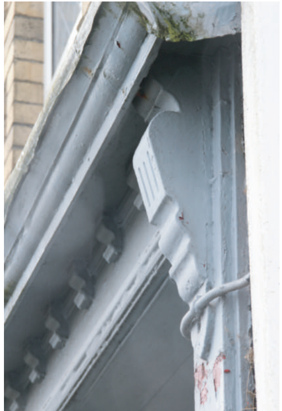
Plate 18. London House, Beach Road, Penclawdd. Detail of moulded corbel on shopfront. Looking southeast.
