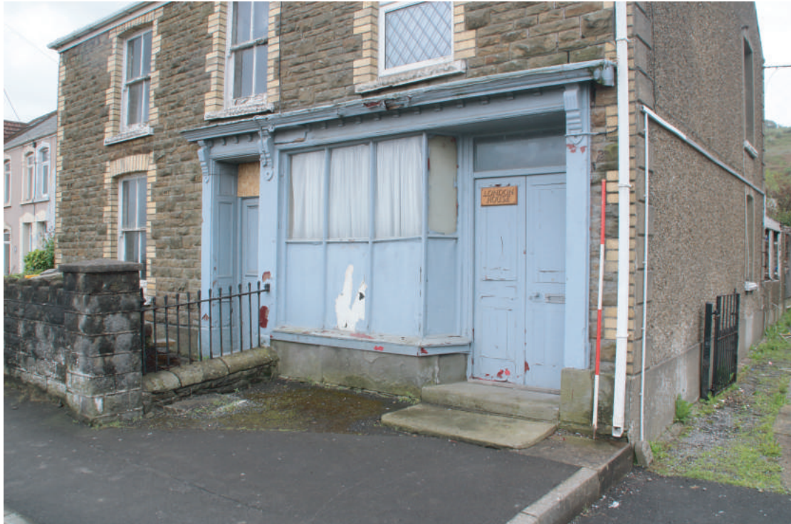
Plate 09. London House, Beach Road, Penclawdd. Looking southeast.
