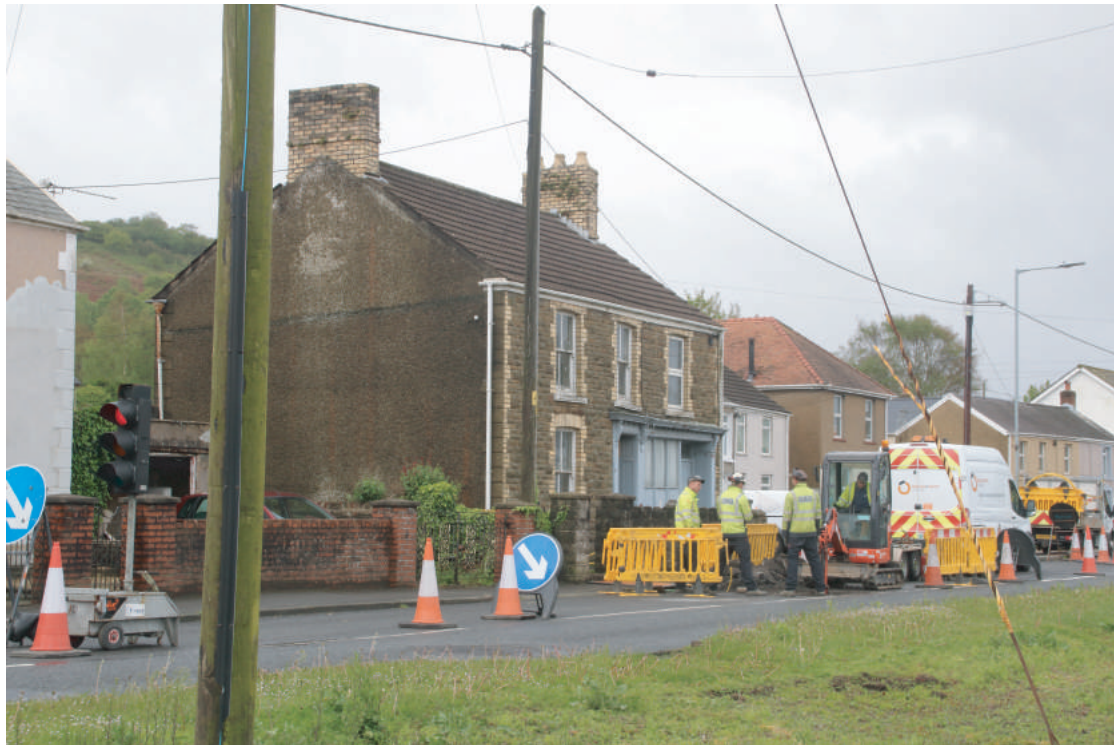
Plate 02. London House, Beach Road, Penclawdd. Looking southwest.
