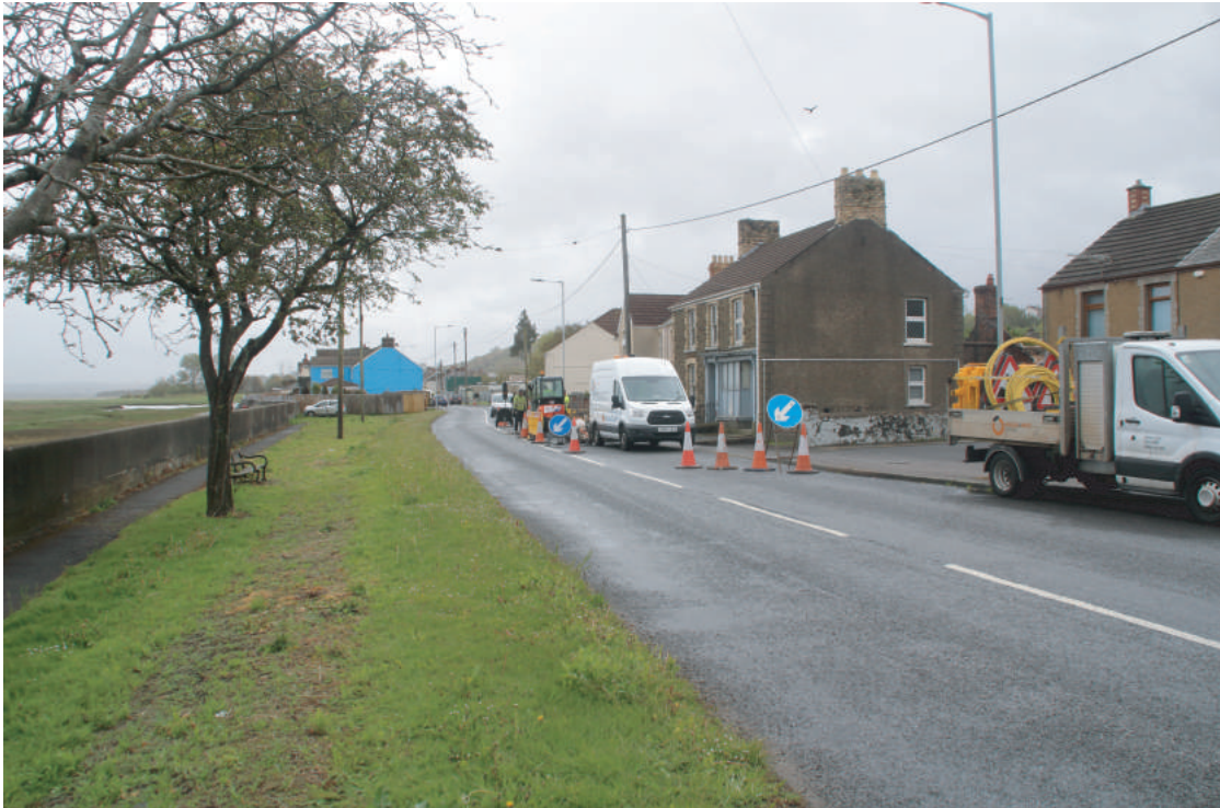
Plate 03. London House, Beach Road, Penclawdd. Looking eastwards.
