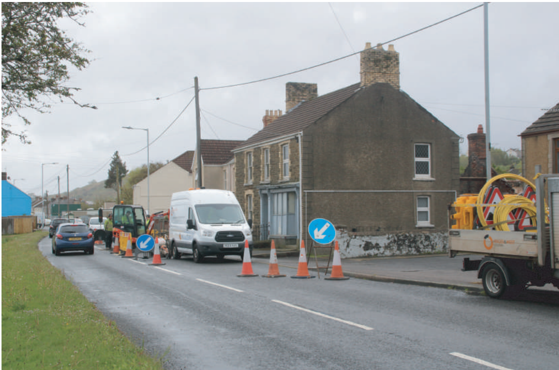
Plate 04. London House, Beach Road, Penclawdd. Looking eastwards.
