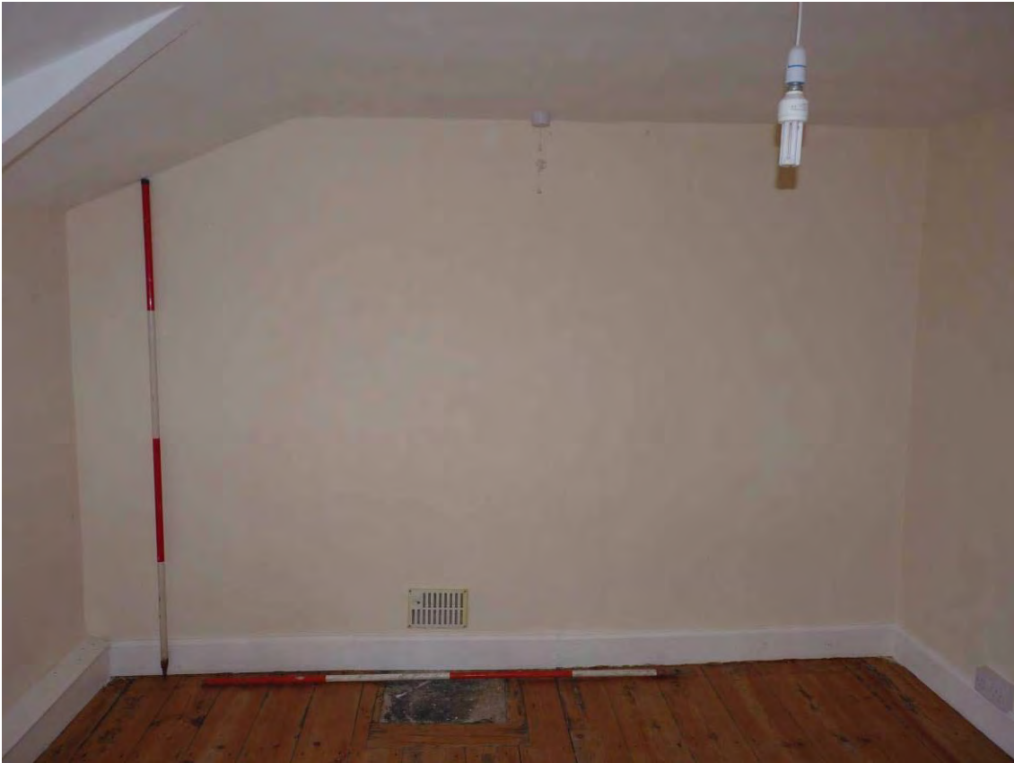
Photo 25: The Farmhouse interior, 1 st floor, Room 7. Looking East. 2m scales.
