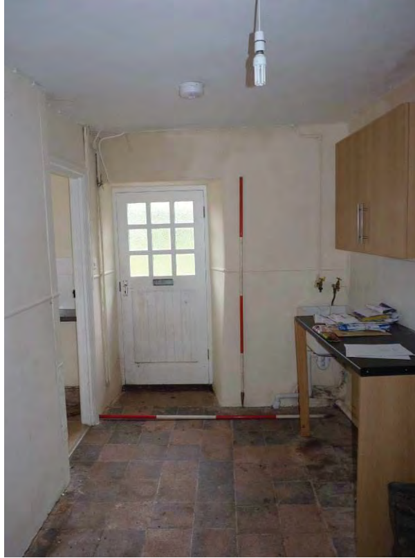
Photo 19: The Farmhouse interior, Room 4. Looking South. 2m scales.
