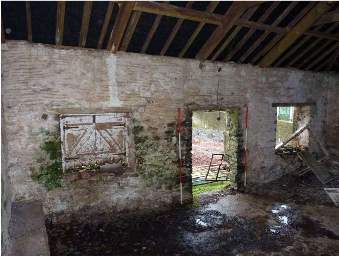
Photo 55: The Cow Shed, northern room. Looking Northwest. 2m scales.
