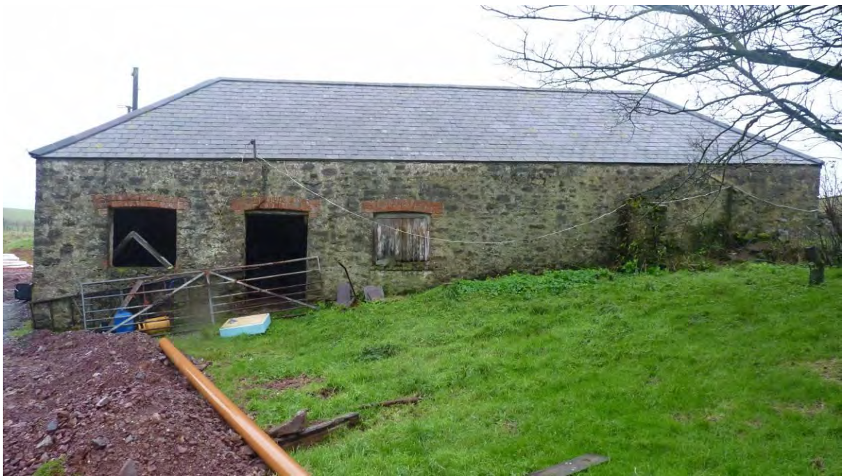
Photo 44: The Cow Shed, western elevation. Looking East.
