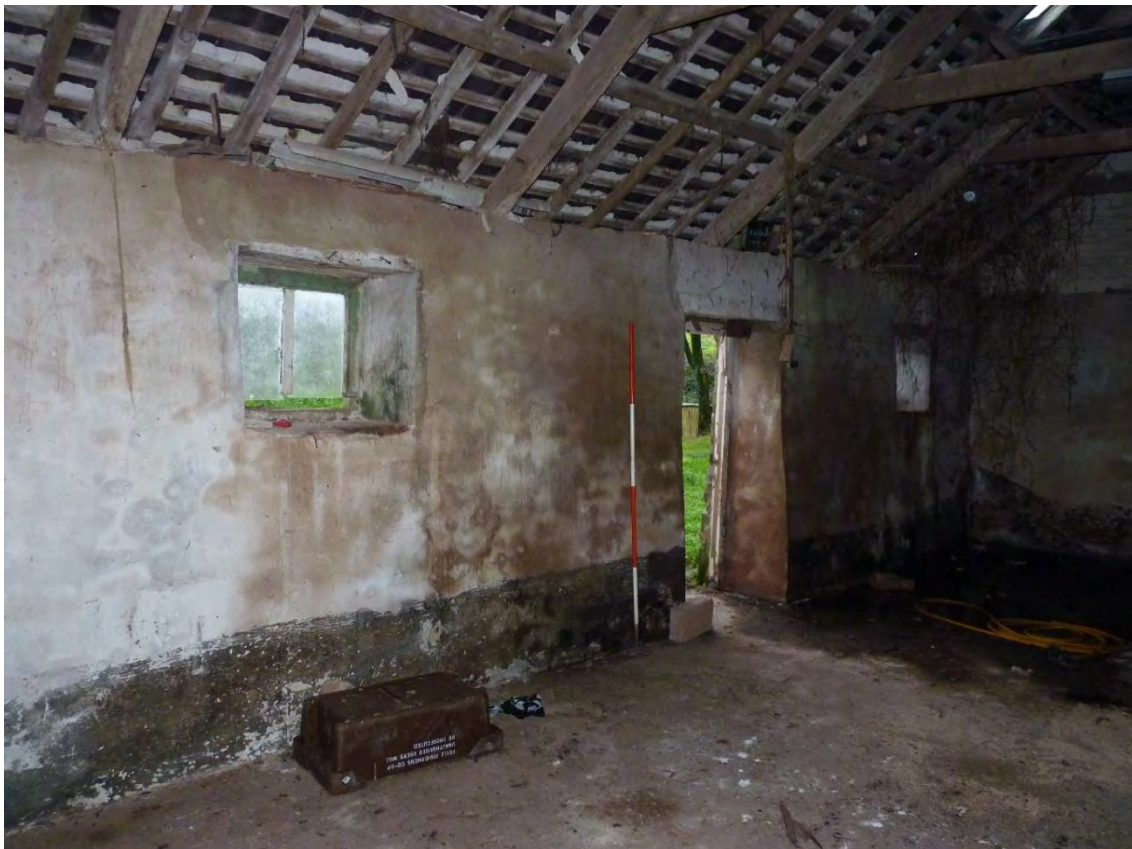
Photo 70: The Cart Shed, interior, northern room. Looking Southeast. 2m scale.
