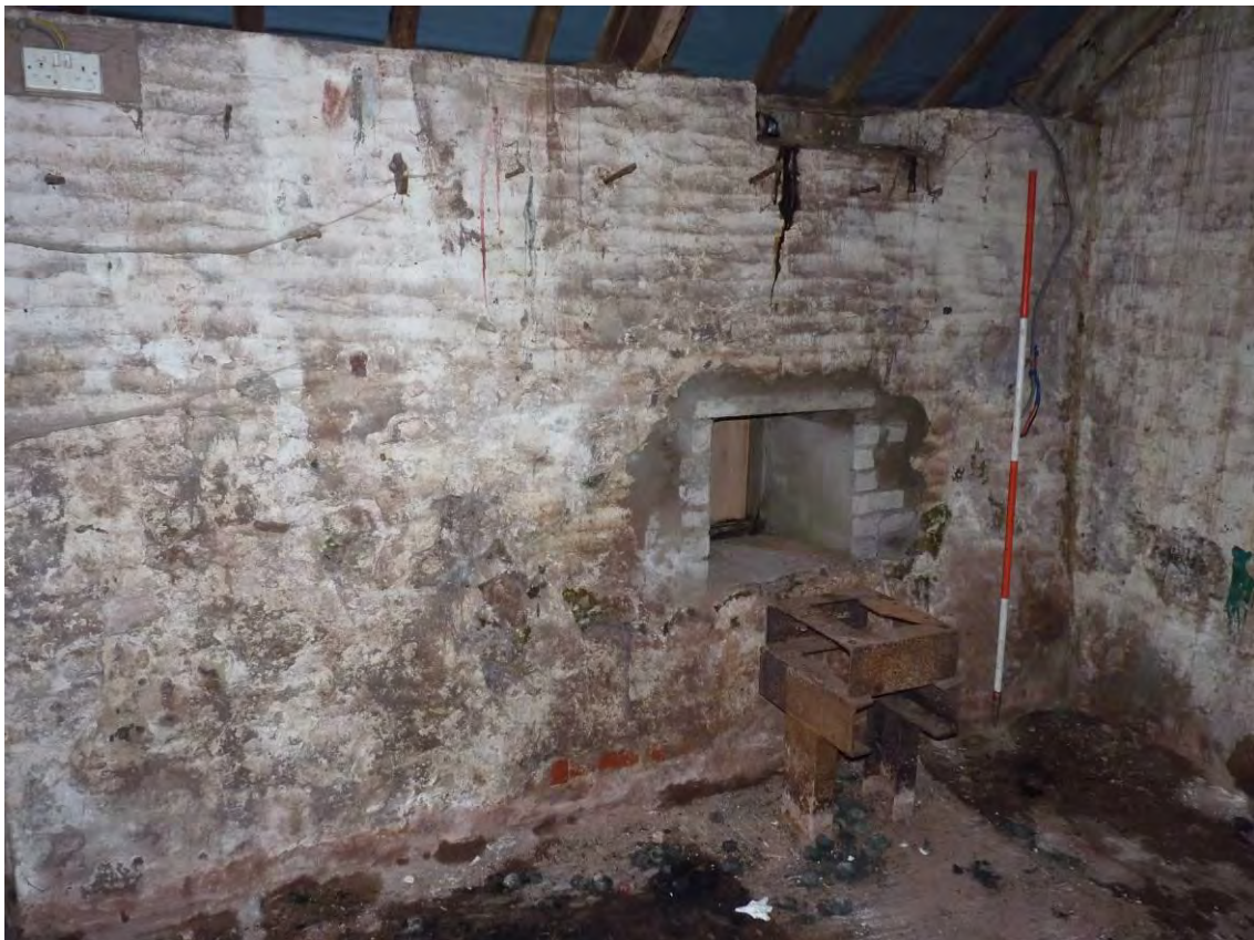
Photo 40: The Lean-to, interior, inserted opening in southern wall. Looking Southwest. 2m scale.
