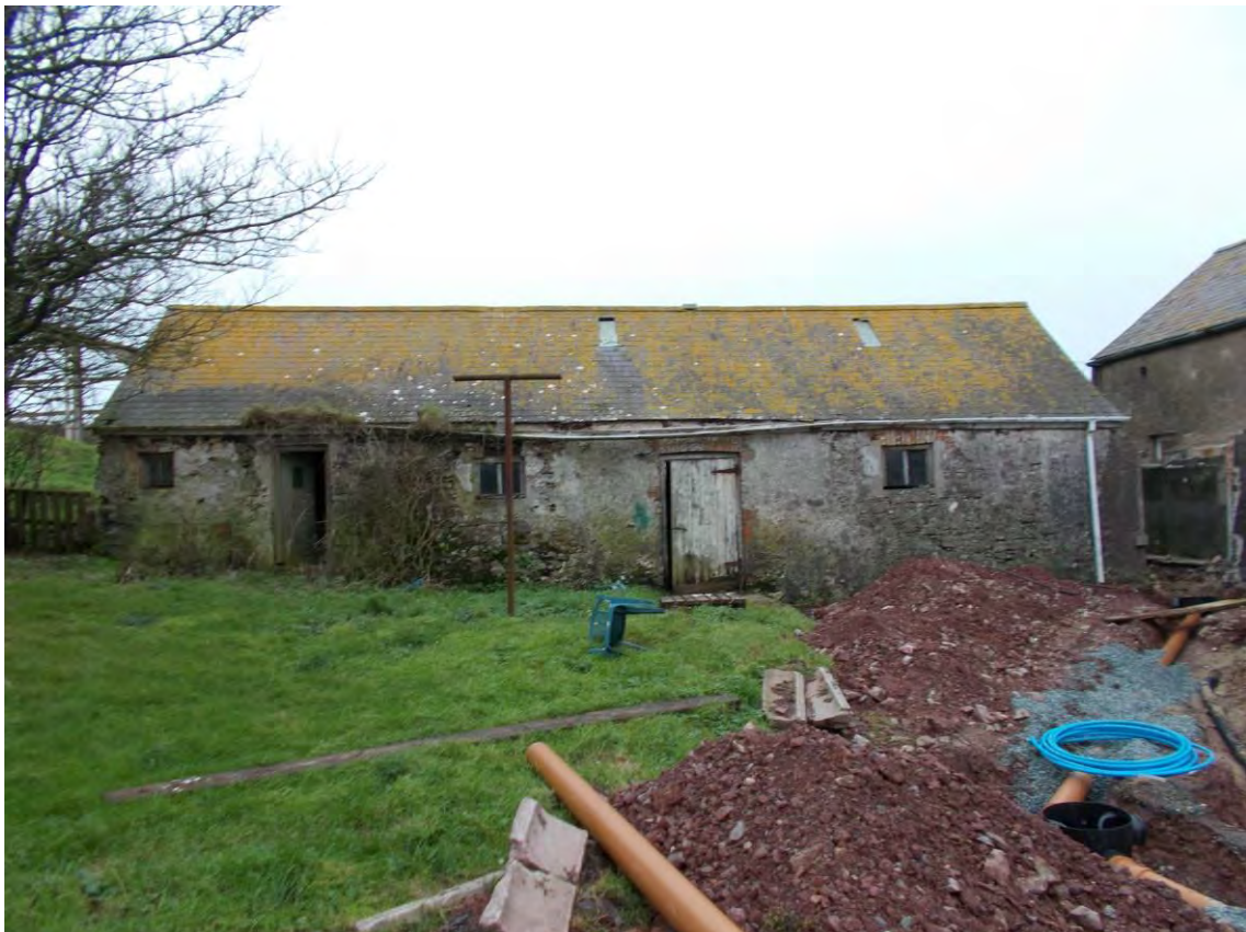
Photo 60: The Cart Shed, eastern elevation. Looking West.
