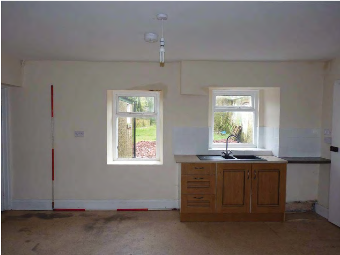
Photo 17: The Farmhouse interior, Room 3. Looking South. 2m scales.
