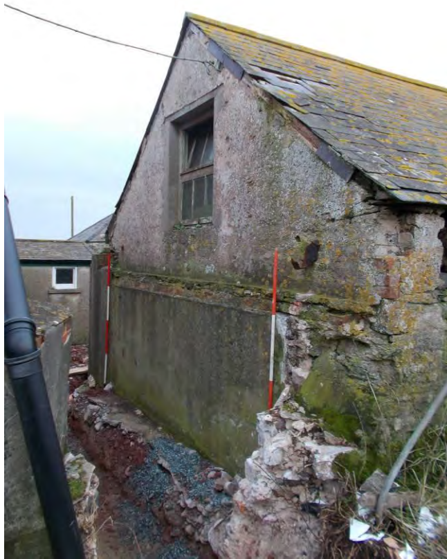
Photo 63: The Cart Shed, northern (gable) elevation. Looking Southeast. 2m scales.
