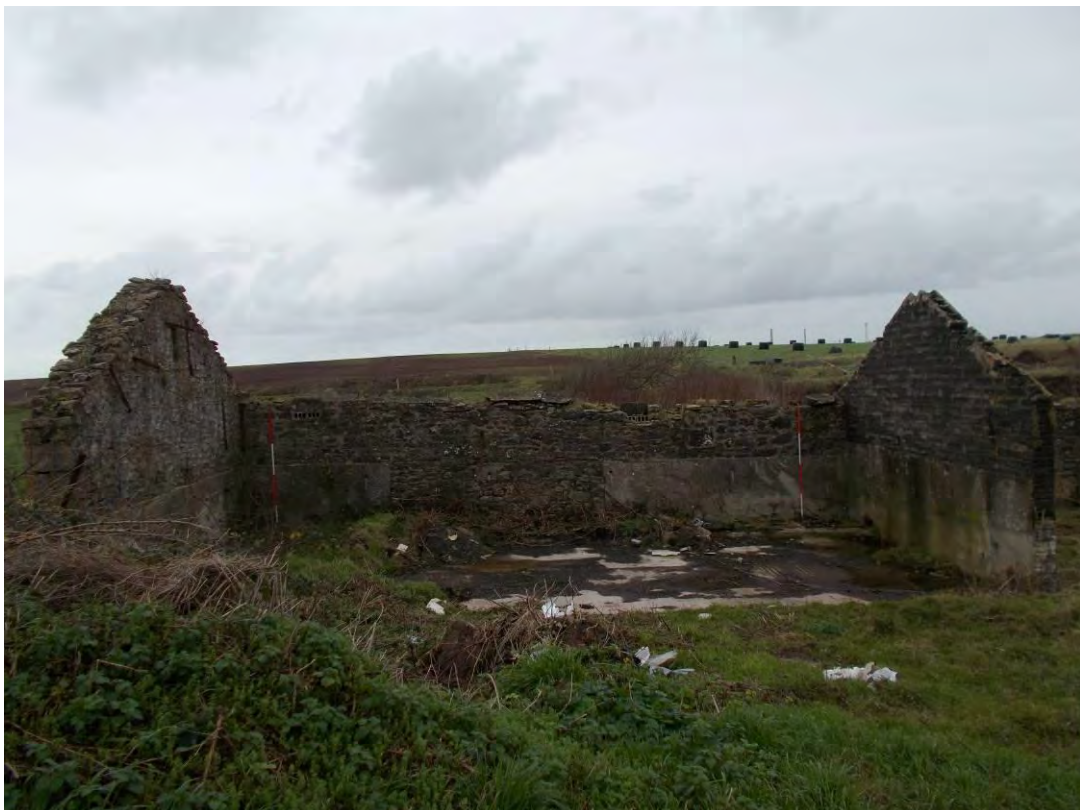
Photo 88: Detached ruinous structure at the western end of the farmstead, interior of western room. Looking North. 2m scales.
