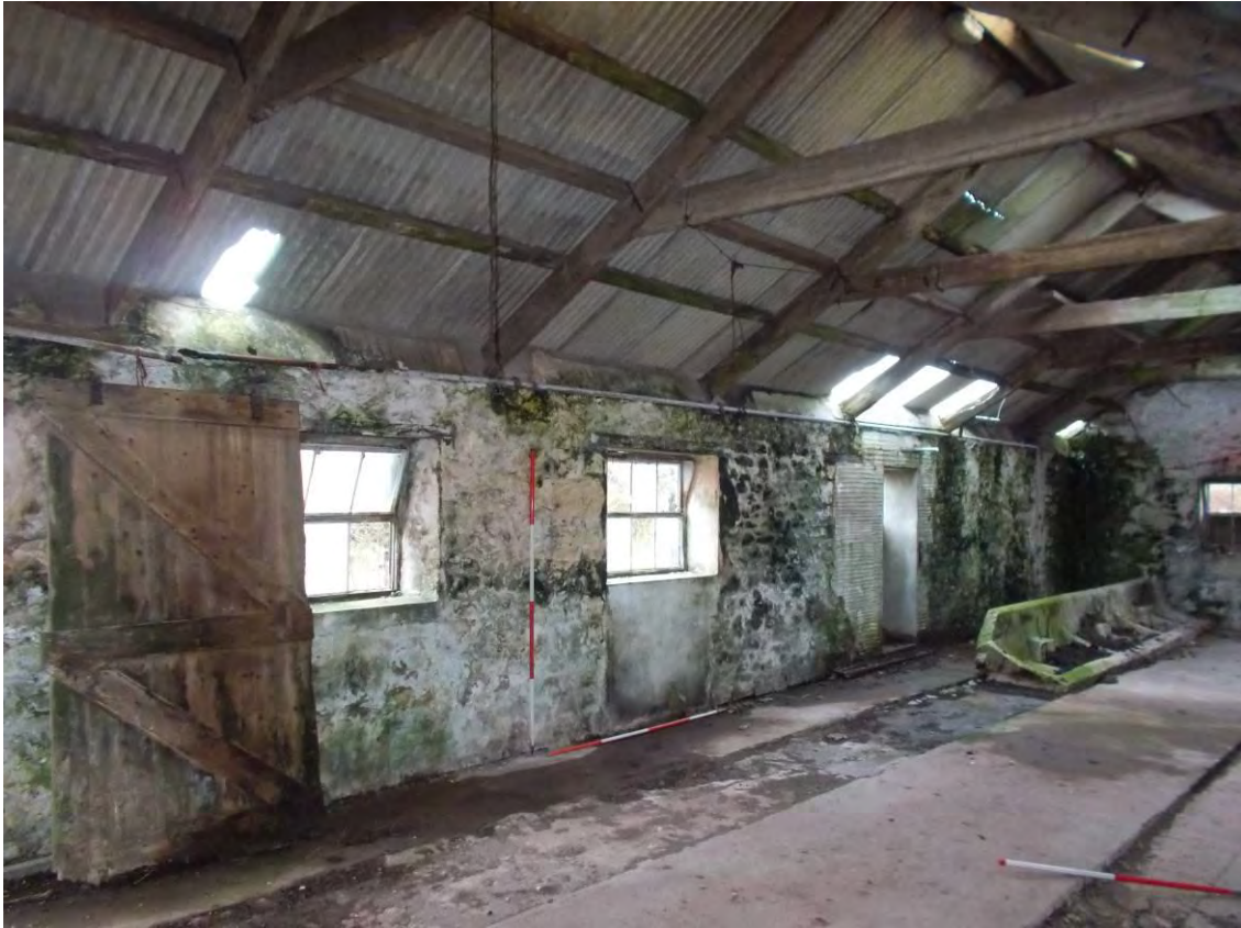
Photo 77: The Milking Parlour, Building 1, interior. Looking Northwest. 1m & 2m scales.
