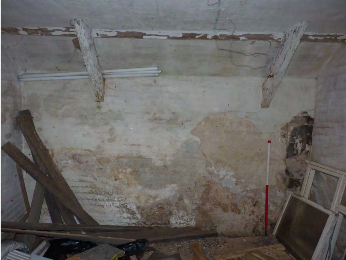
Photo 68: The Cart Shed, interior, southern room. Looking West. 1m scale.
