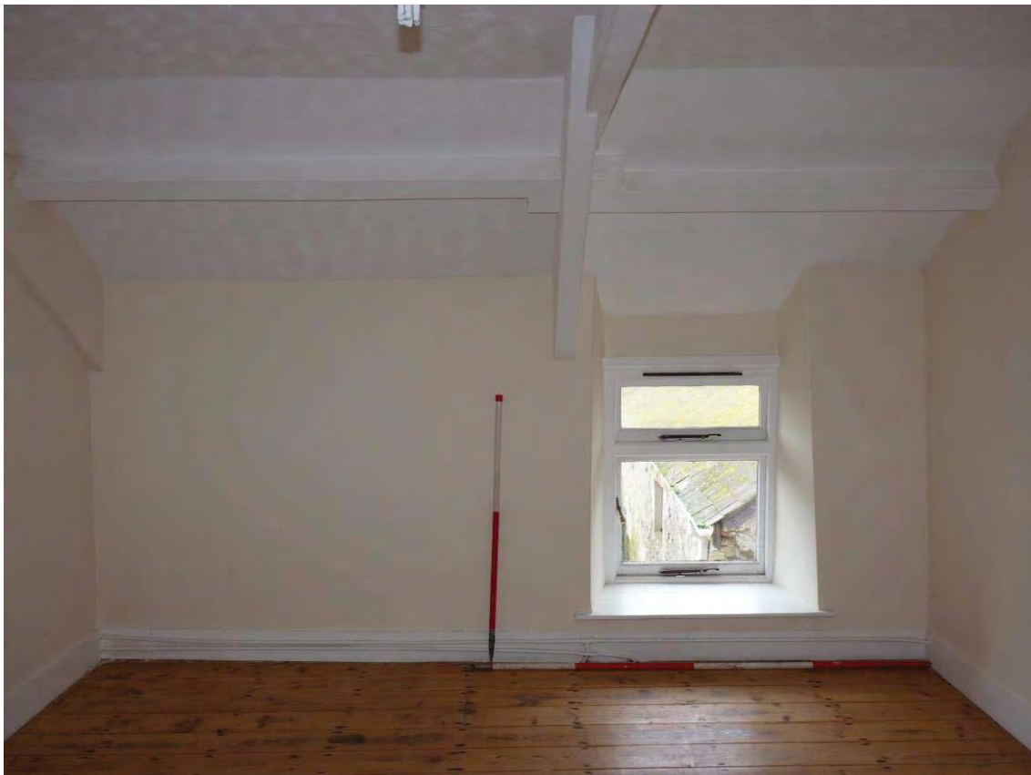
Photo 30: The Farmhouse interior, 1 st floor, Room 9. Looking South. 1m & 2m scales.
