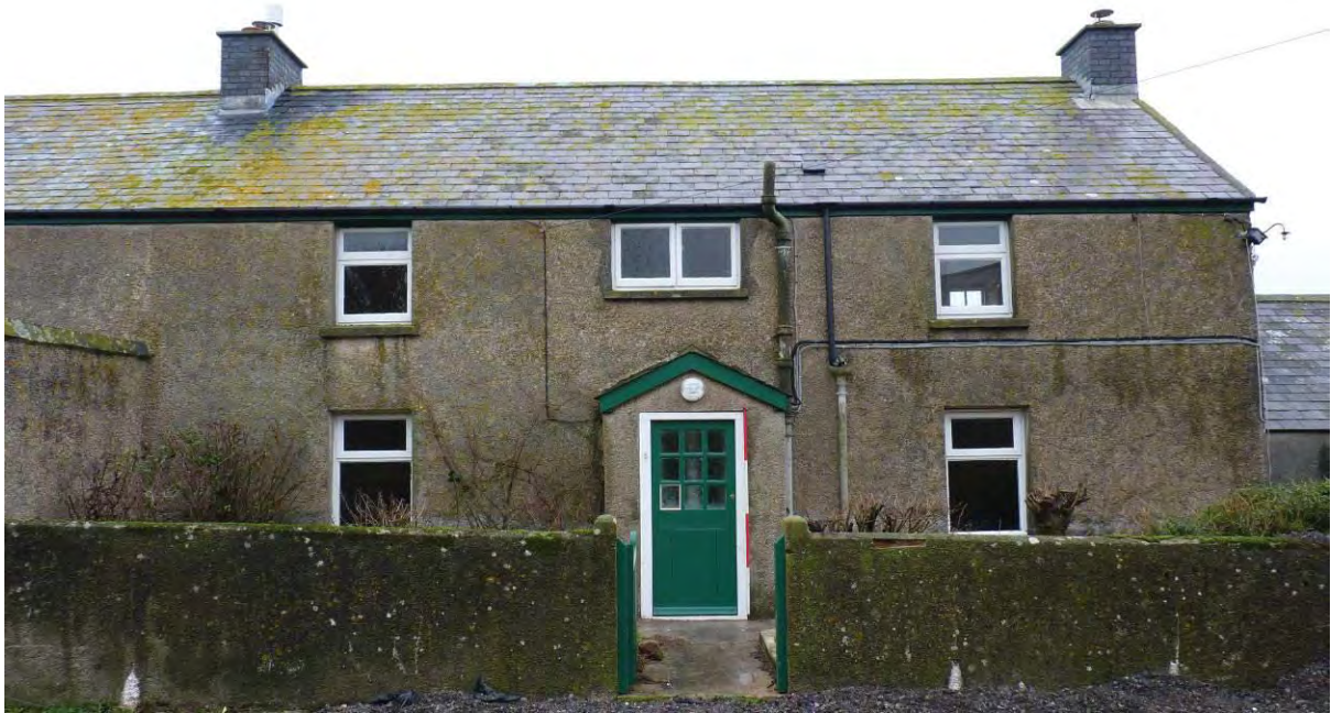
Photo 3: The Farmhouse, southern elevation. Looking north. 2m scale.
