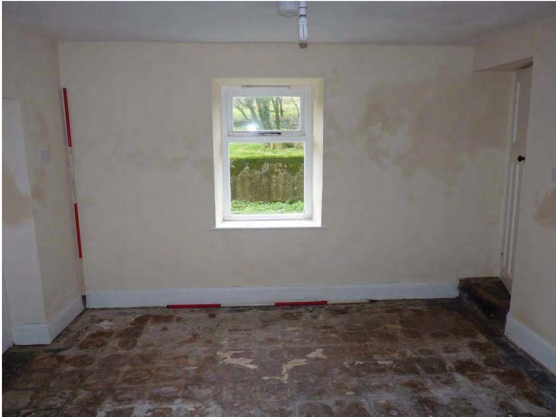
Photo 15: The Farmhouse interior, Room 2. Looking South. 2m scales.
