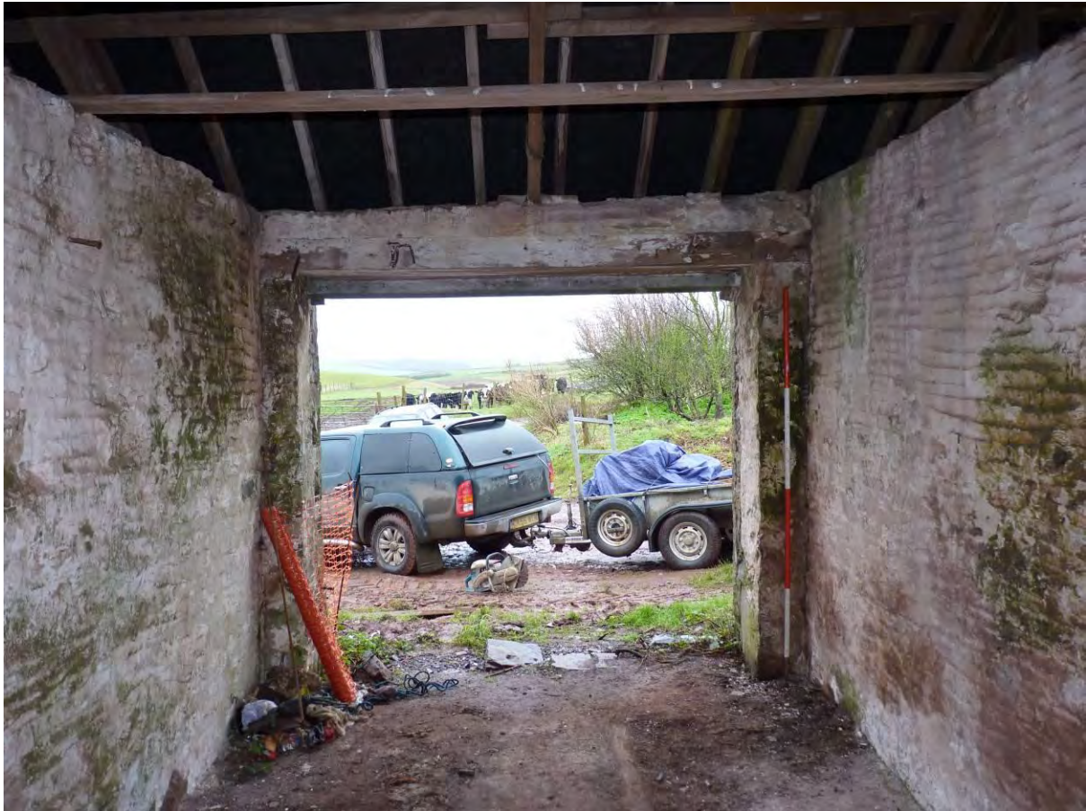
Photo 53: The Cow Shed, central room. Looking East. 2m scale.
