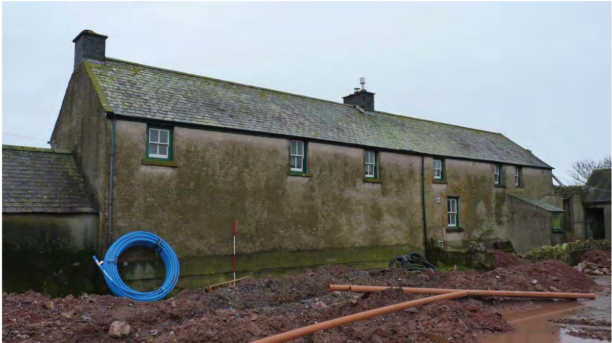
Photo 7: The Farmhouse, northern (rear) elevation. Looking South-southwest. 2m scale.
