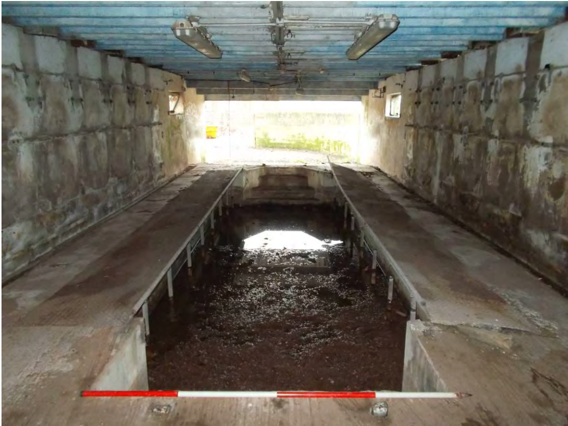
Photo 81: The Milking Parlour, Building 2, interior. Looking East. 2m scale.
