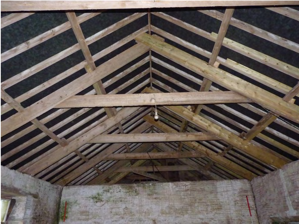
Photo 59: The Cow Shed, northern room, roof structure. Looking South.
