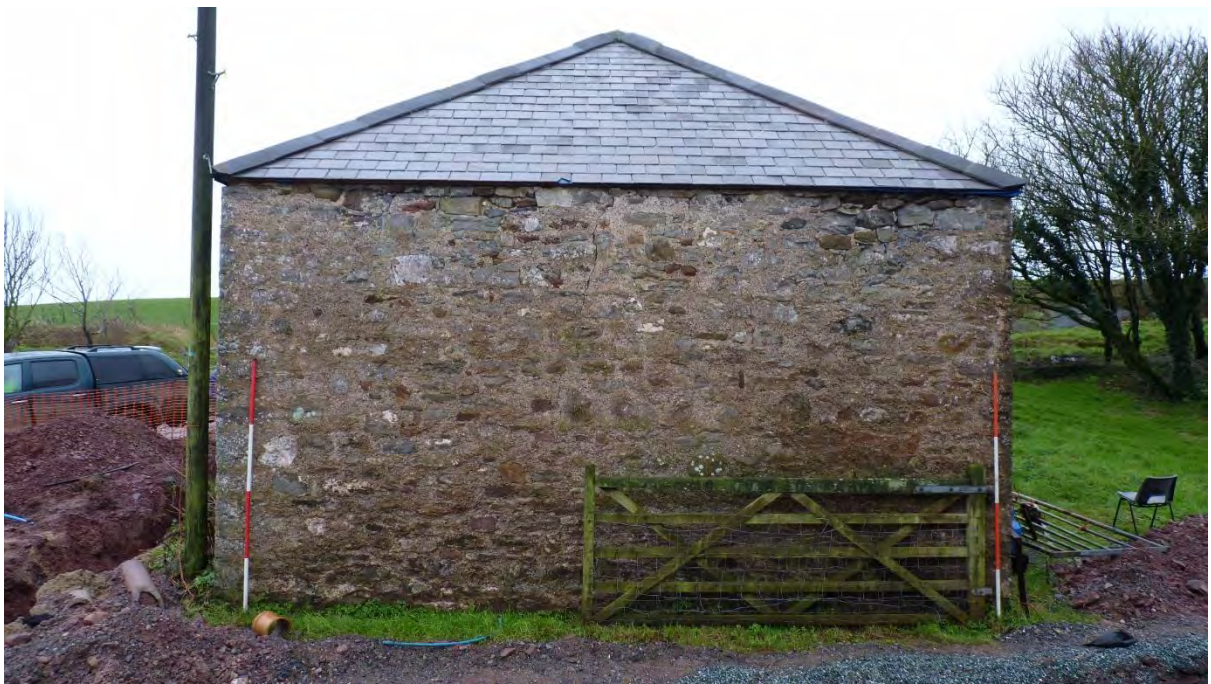
Photo 46: The Cow Shed, northern (gable) elevation. Looking South. 2m scales.
