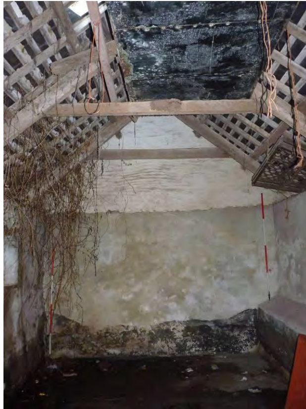
Photo 71: The Cart Shed, interior, northern room. Looking South. 2m scales.
