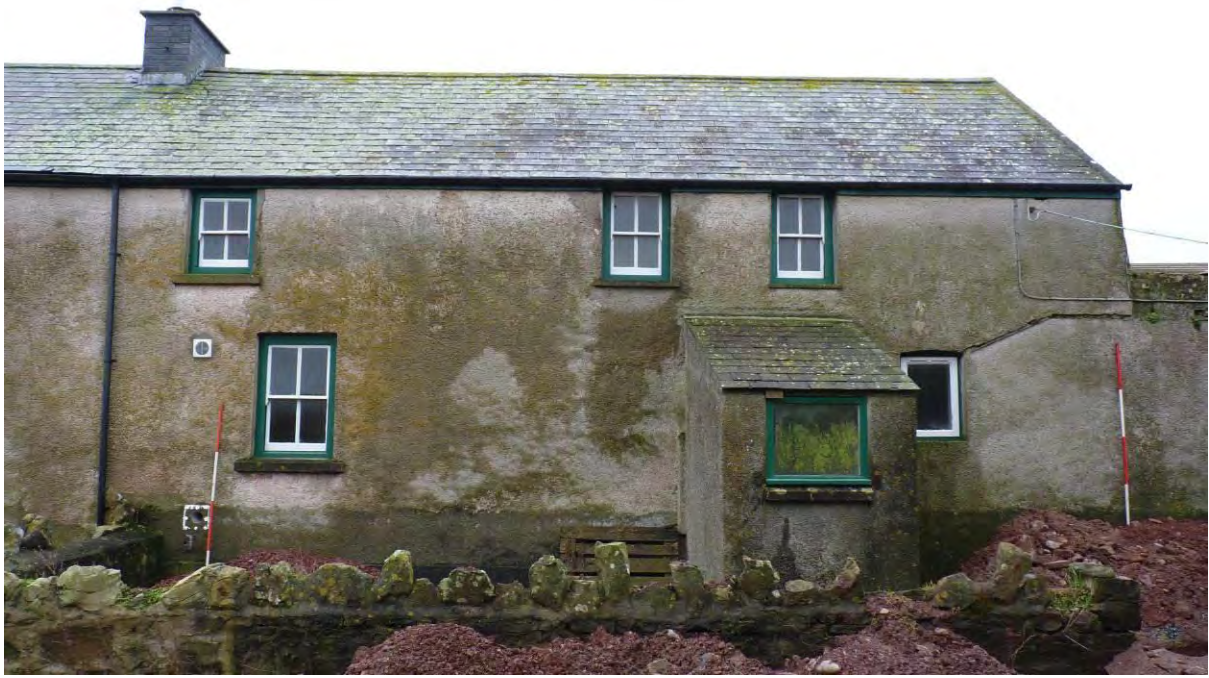
Photo 9: The Farmhouse, northern (rear) elevation. Looking South. 2m scale
