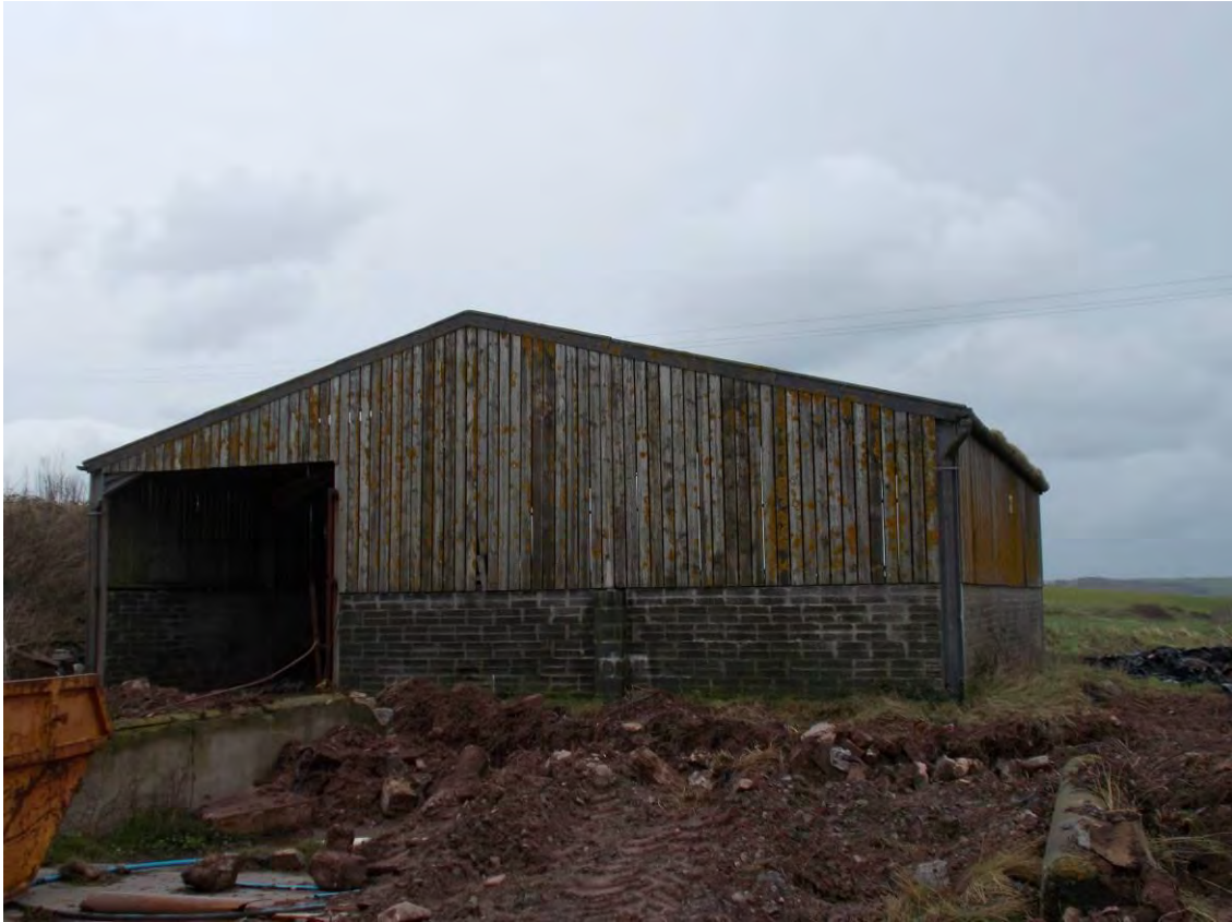
Photo 83: The Workshop, western elevation. Looking East-northeast.
