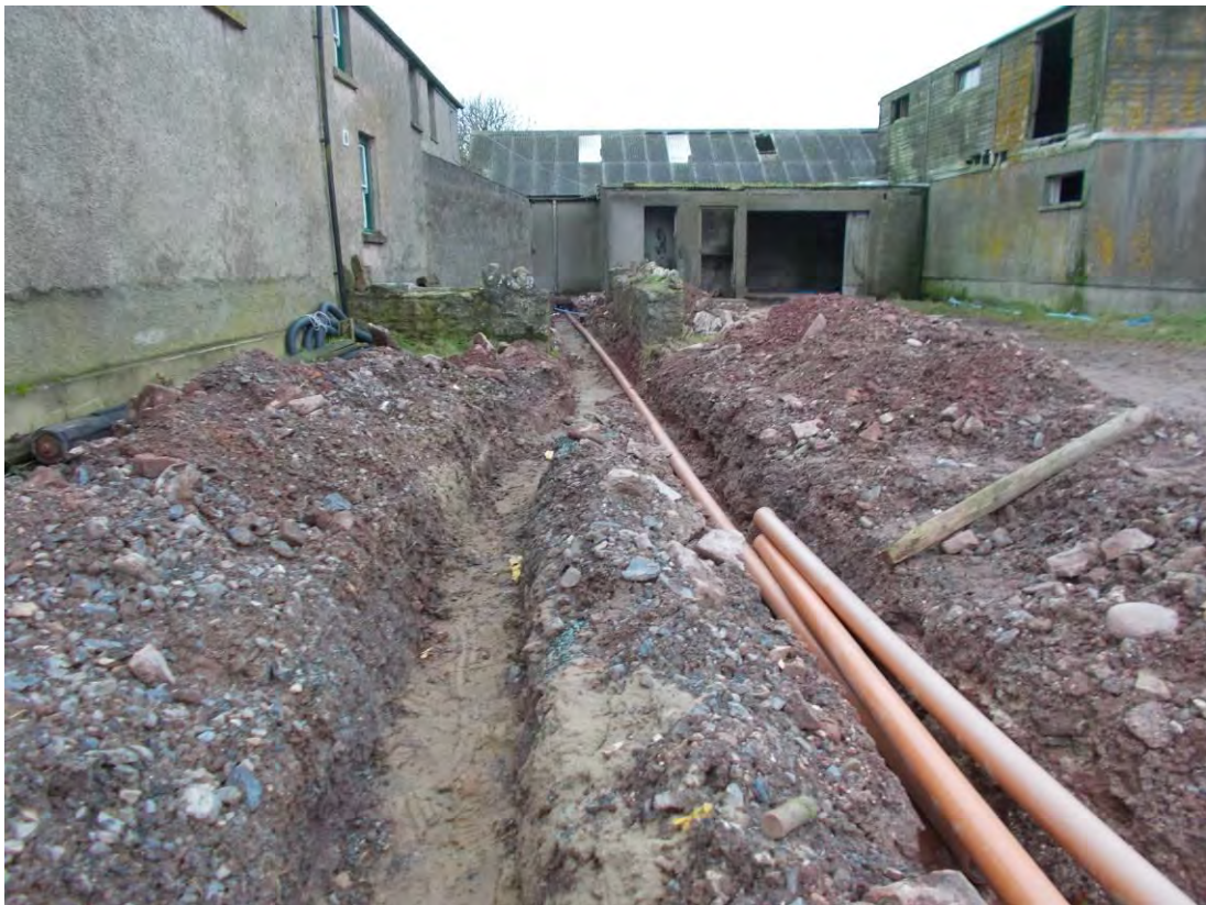
Photo 98: Service trench excavations - trench through northern area.
