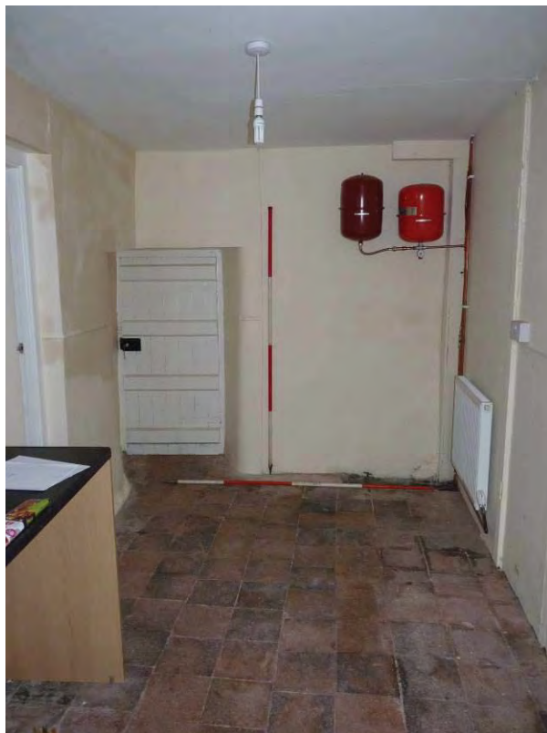
Photo 20: The Farmhouse interior, Room 4. Looking North. 2m scales.
