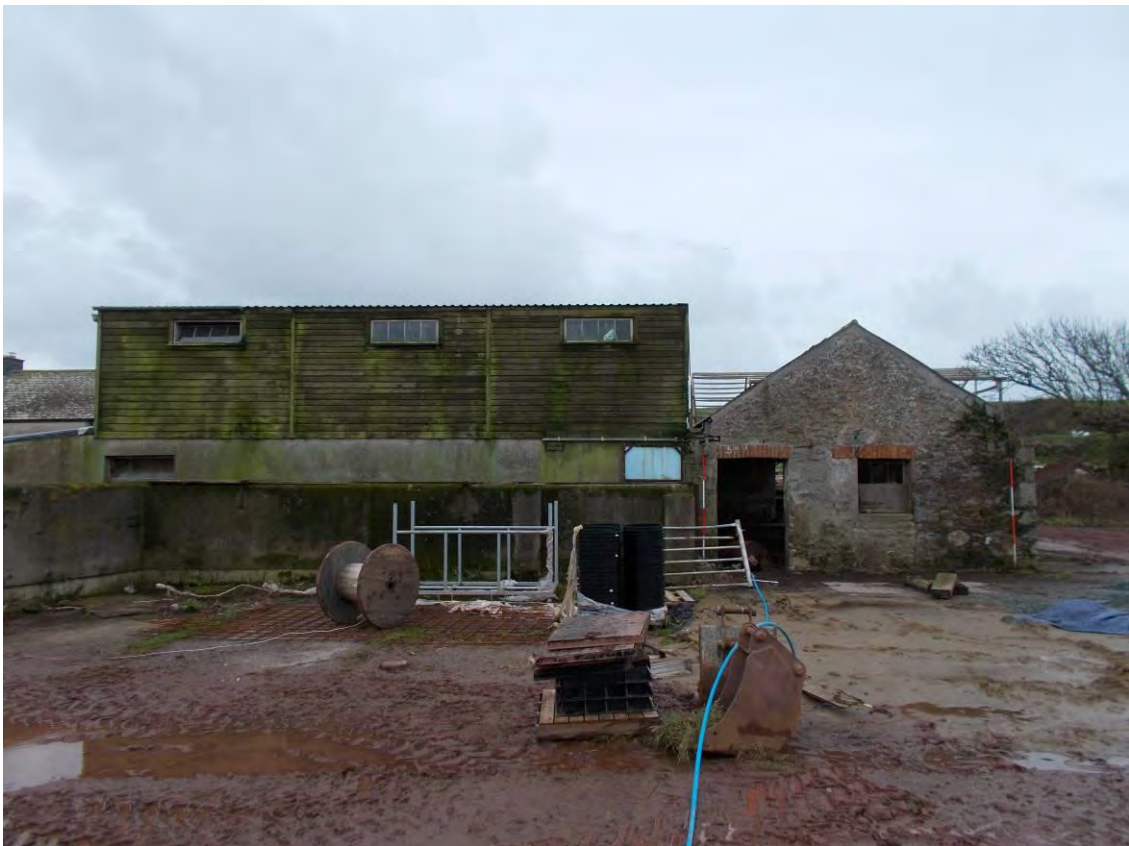
Photo 78: The Milking Parlour, Buildings 1 & 2, northern elevation. Looking South. 2m scales.
