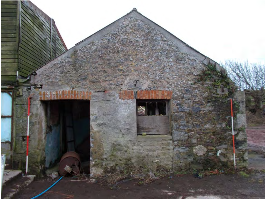
Photo 75: The Milking Parlour, Building 1, northern (gable) elevation. Looking South. 2m scales.
