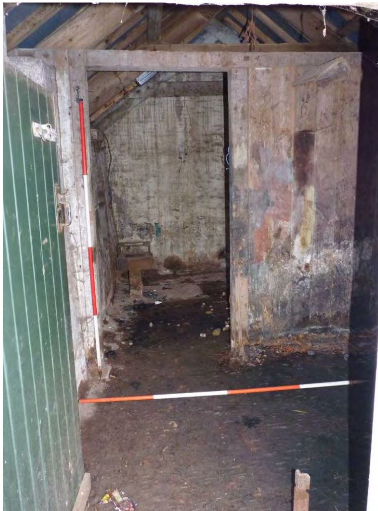
Photo 36: The Lean-to, interior, from the doorway. Looking West. 2m scales.
