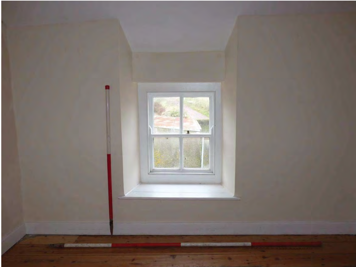
Photo 27: The Farmhouse interior, 1 st floor, Room 8. Looking North. 1m & 2m scales.
