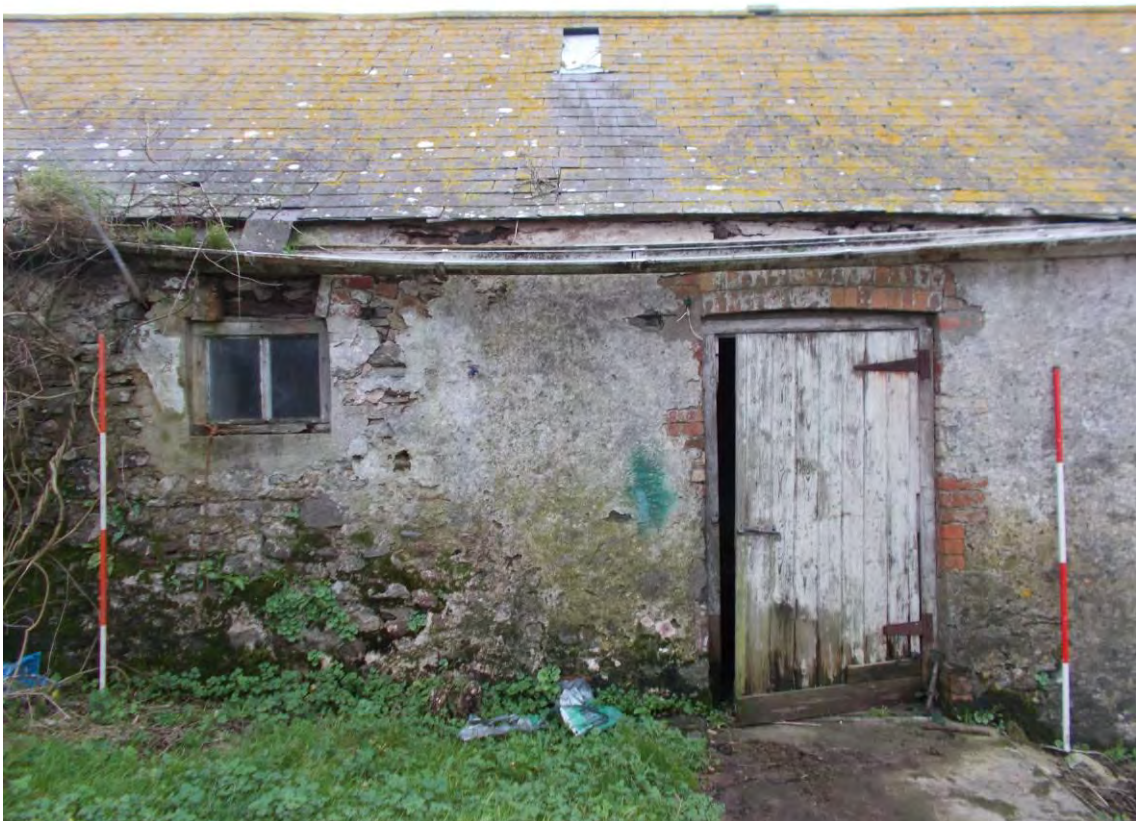
Photo 62: The Cart Shed, eastern elevation. Looking West. 2m scales.
