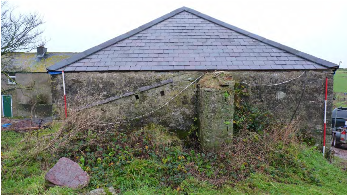
Photo 47: The Cow Shed, southern (gable) elevation. Looking North. 1m & 2m scales.
