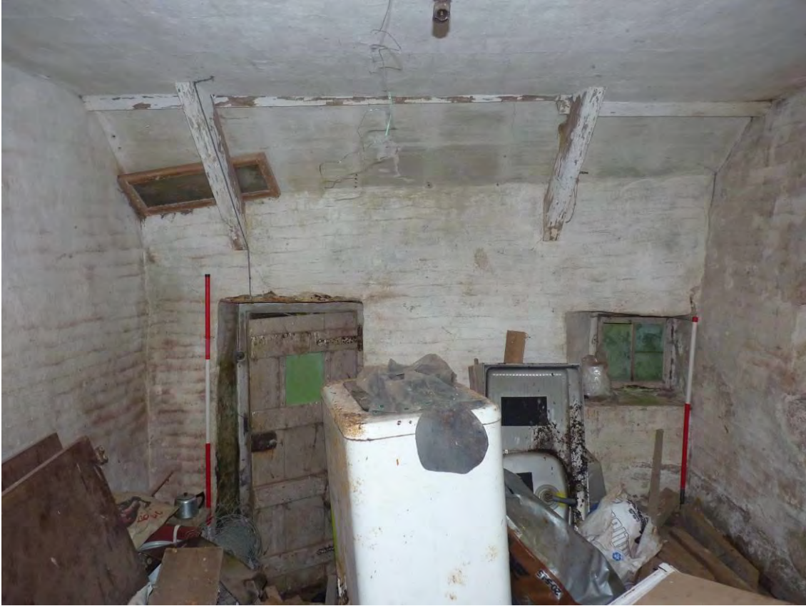
Photo 67: The Cart Shed, interior, southern room. Looking East. 1m & 2m scales.
