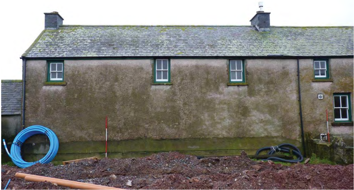
Photo 8: The Farmhouse, northern (rear) elevation. Looking South. 2m scale
