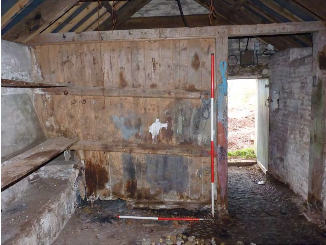
Photo 41: The Lean-to, interior, internal division. Looking East. 1m & 2m scales.
