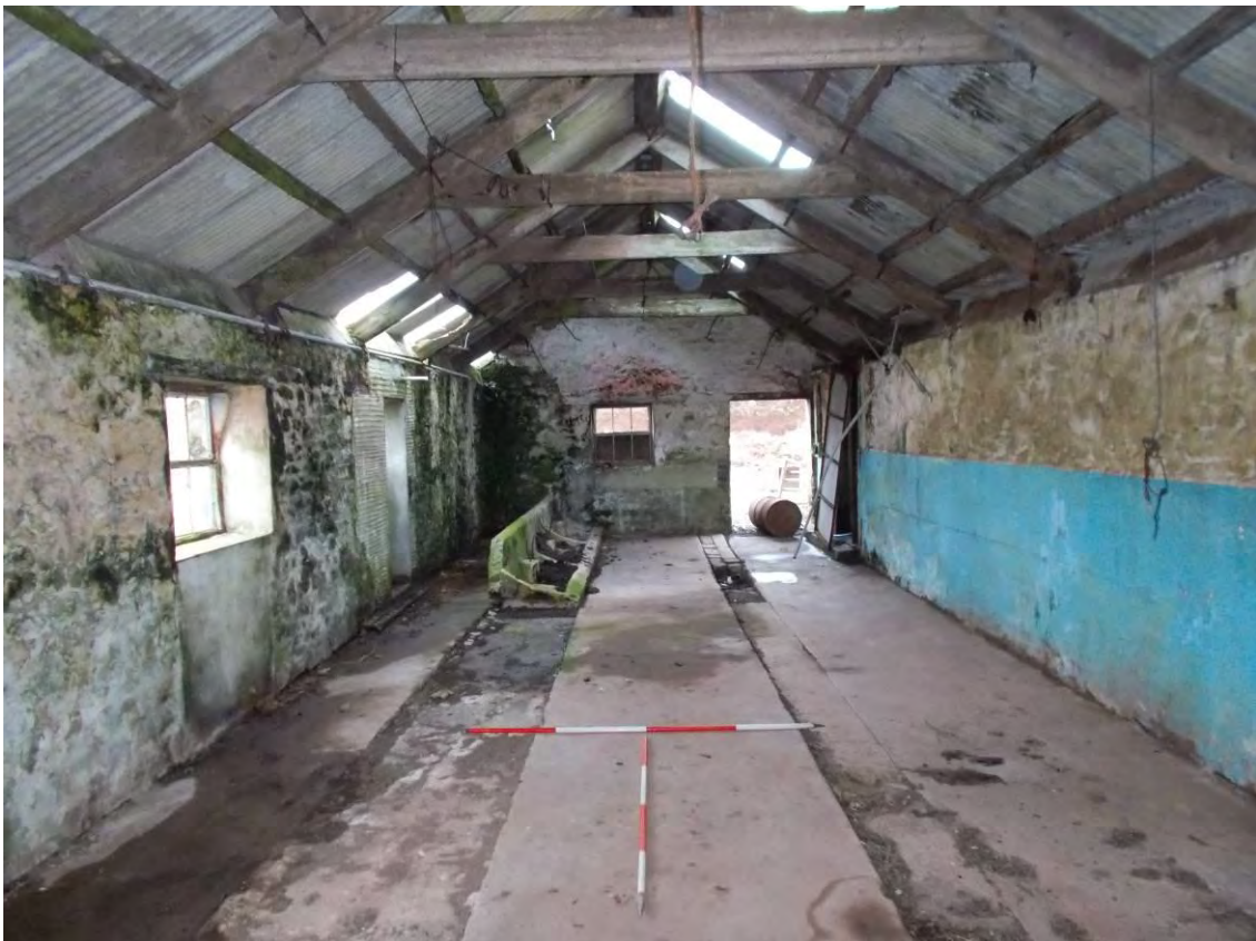
Photo 76: The Milking Parlour, Building 1, interior. Looking North. 2m scales.
