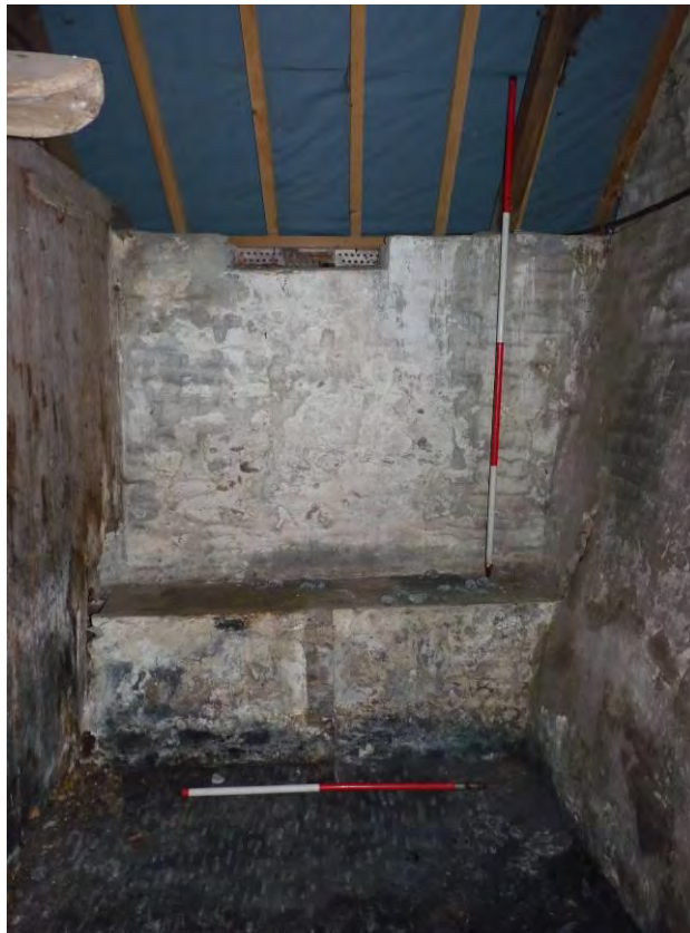
Photo 38: The Lean-to, interior, eastern compartment. Looking North. 1m & 2m scales.
