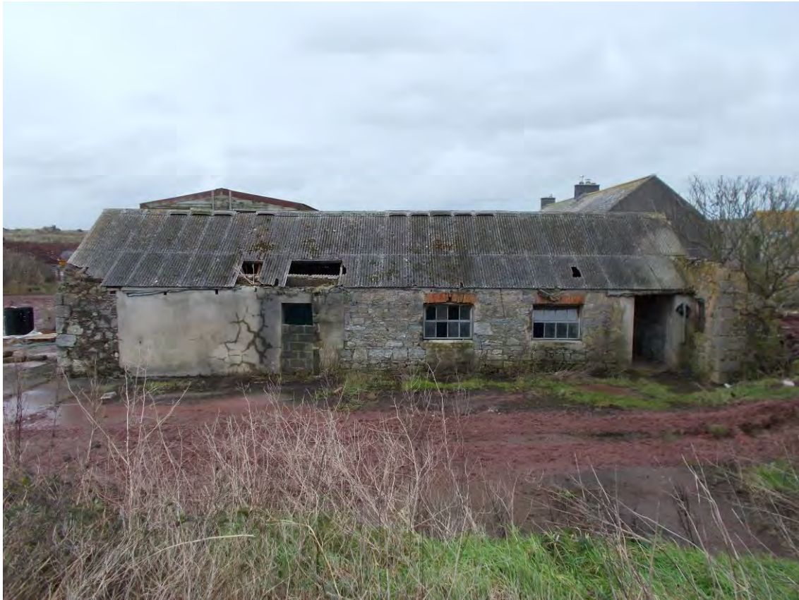
Photo 73: The Milking Parlour, Building 1, western elevation. Looking East.
