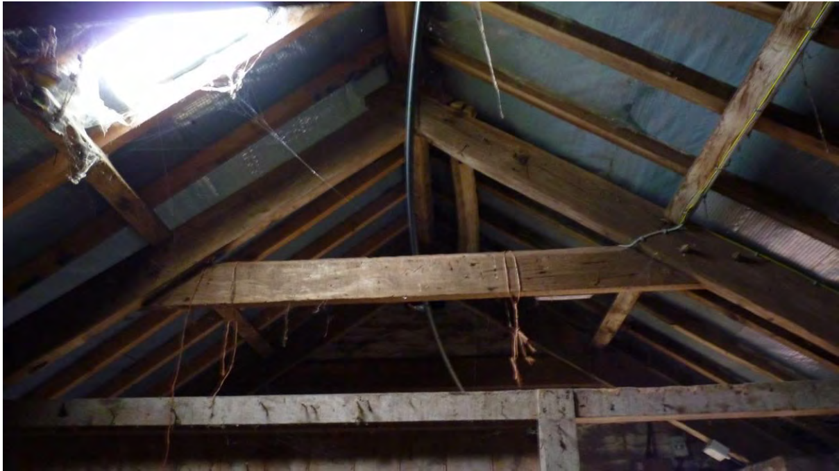
Photo 43: The Lean-to, interior, roof structure. Looking East.
