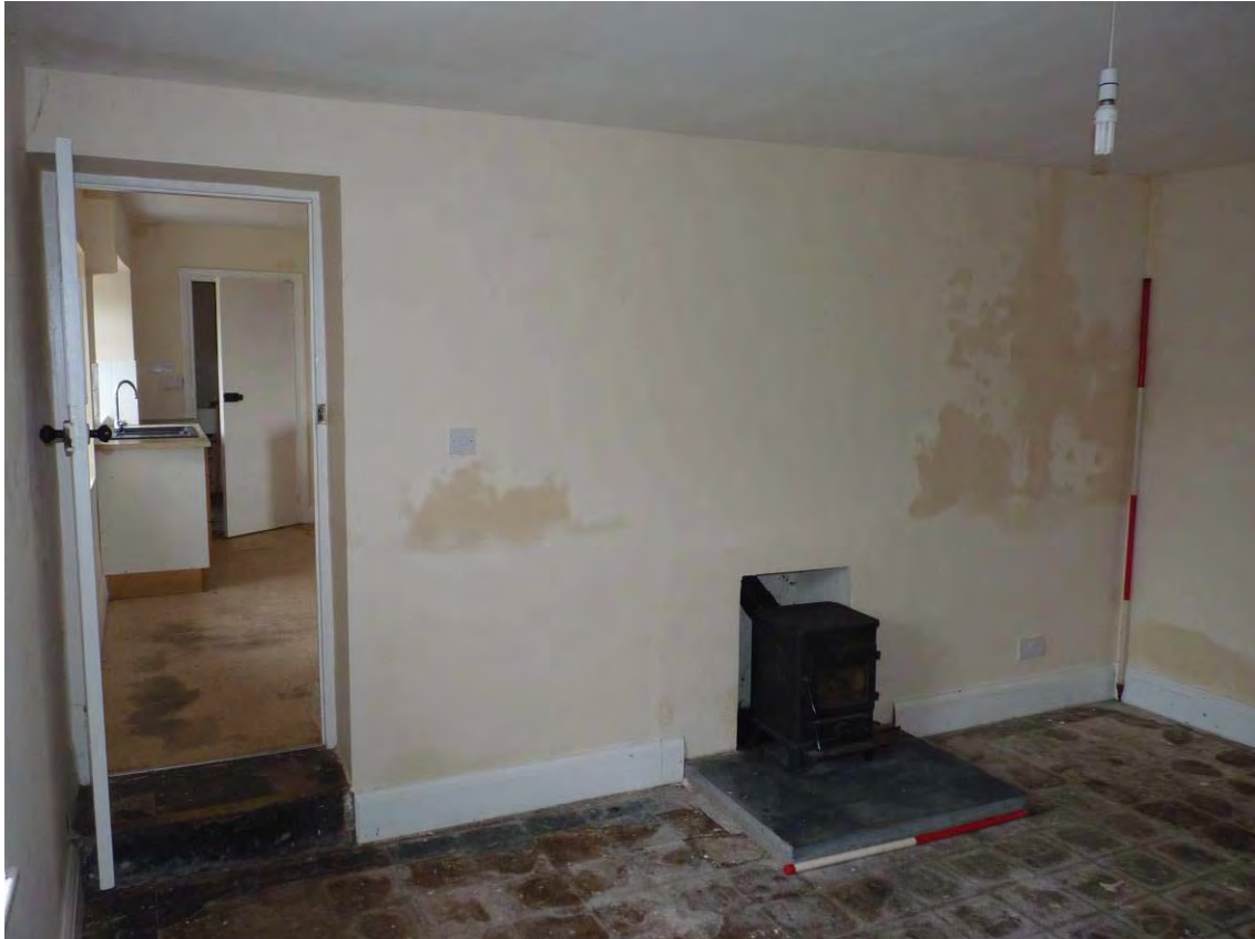
Photo 16: The Farmhouse interior, Room 2. Looking West-northwest. 1m & 2m scales.
