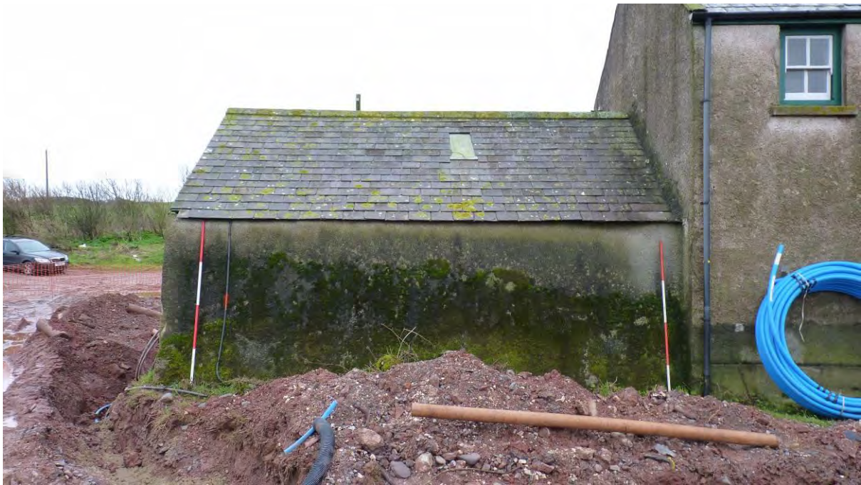
Photo 34: The Lean-to, northern elevation. Looking South. 2m scales.
