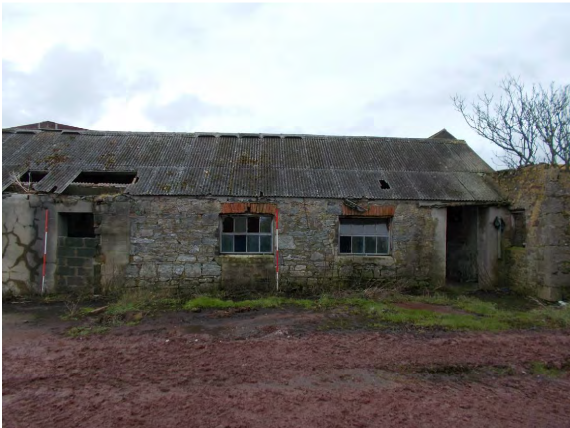
Photo 74: The Milking Parlour, Building 1, western elevation. Looking East. 2m scales.
