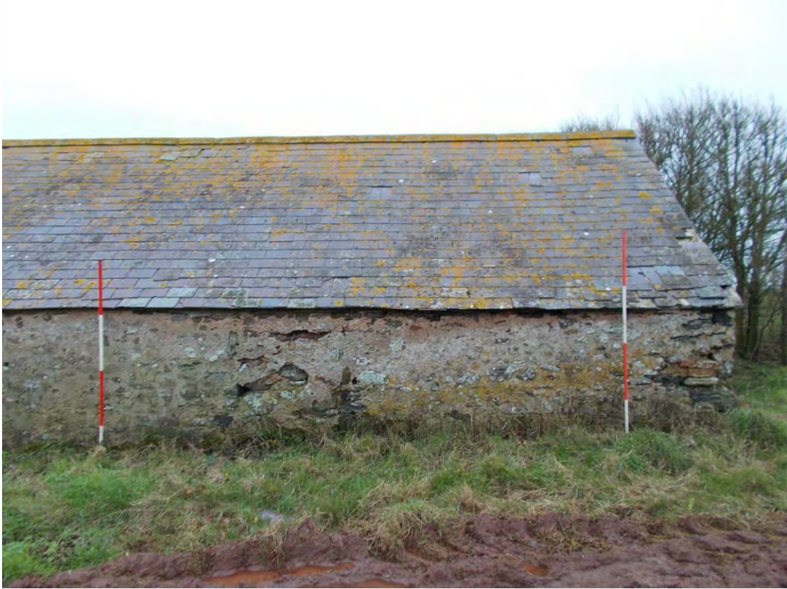
Photo 65: The Cart Shed, western elevation. Looking East. 2m scales.
