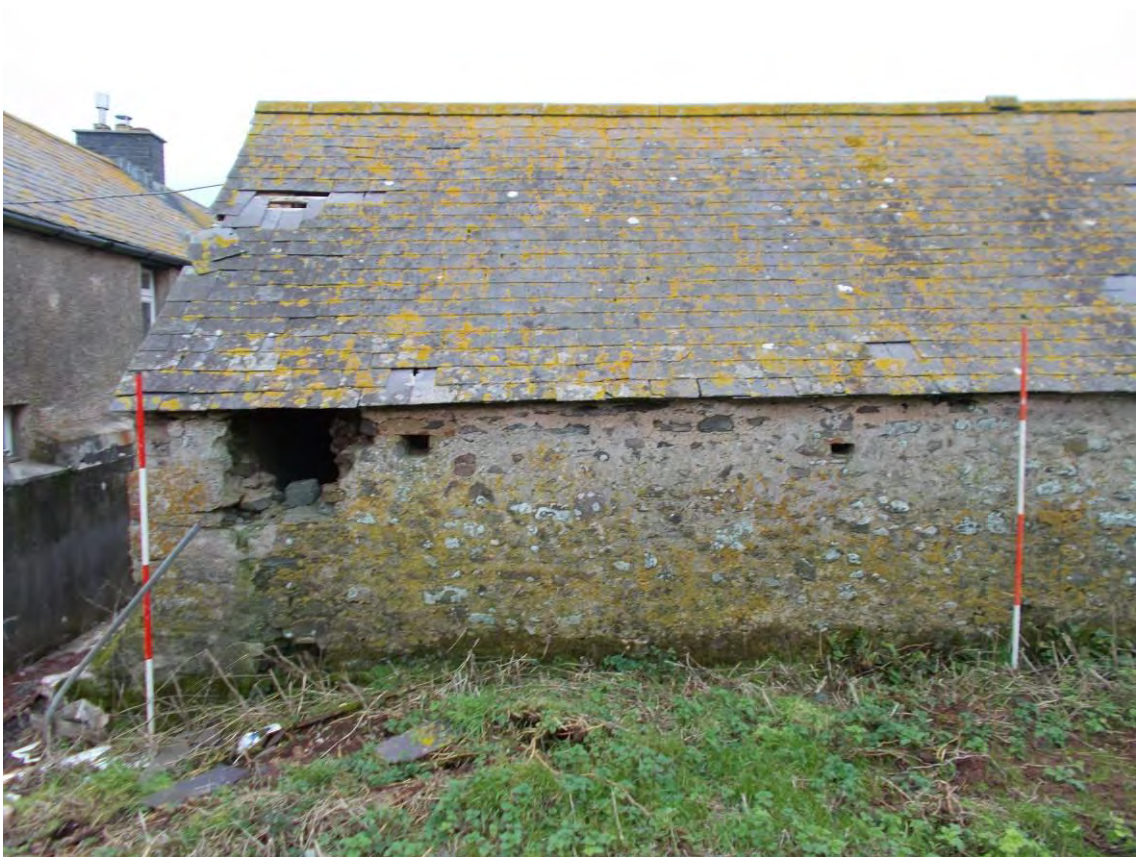
Photo 64: The Cart Shed, western elevation. Looking East. 2m scales.
