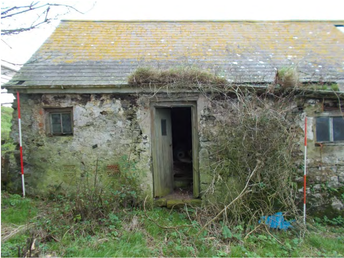
Photo 61: The Cart Shed, eastern elevation. Looking West. 2m scales.
