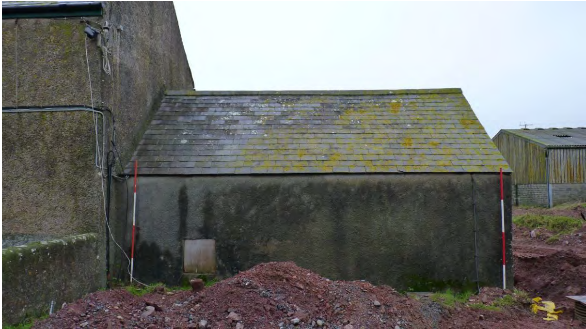
Photo 33: The Lean-to, southern elevation. Looking North. 2m scales.
