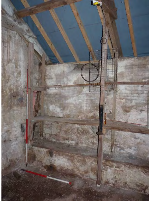
Photo 39: The Lean-to, interior, western compartment. Looking North-northwest. 1m & 2m scales.
