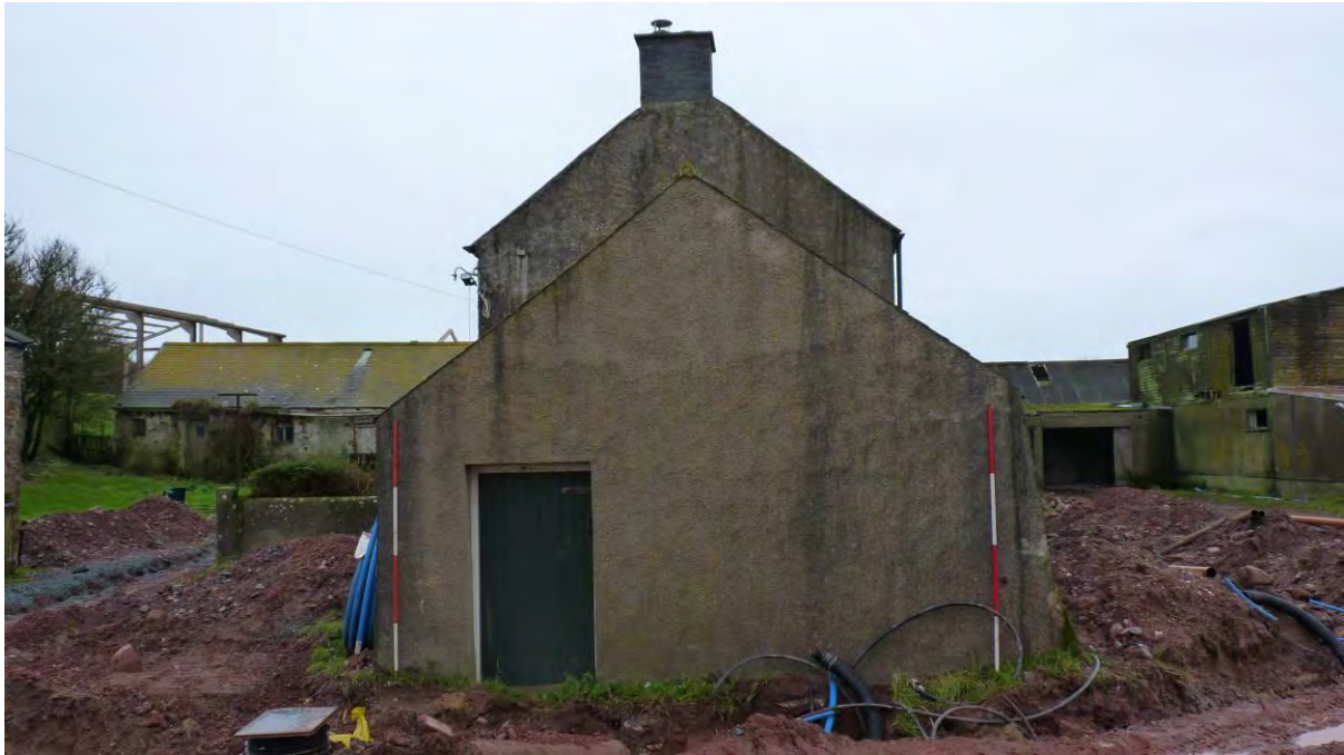
Photo 35: The Lean-to, eastern (gable) elevation. Looking West. 2m scales.
