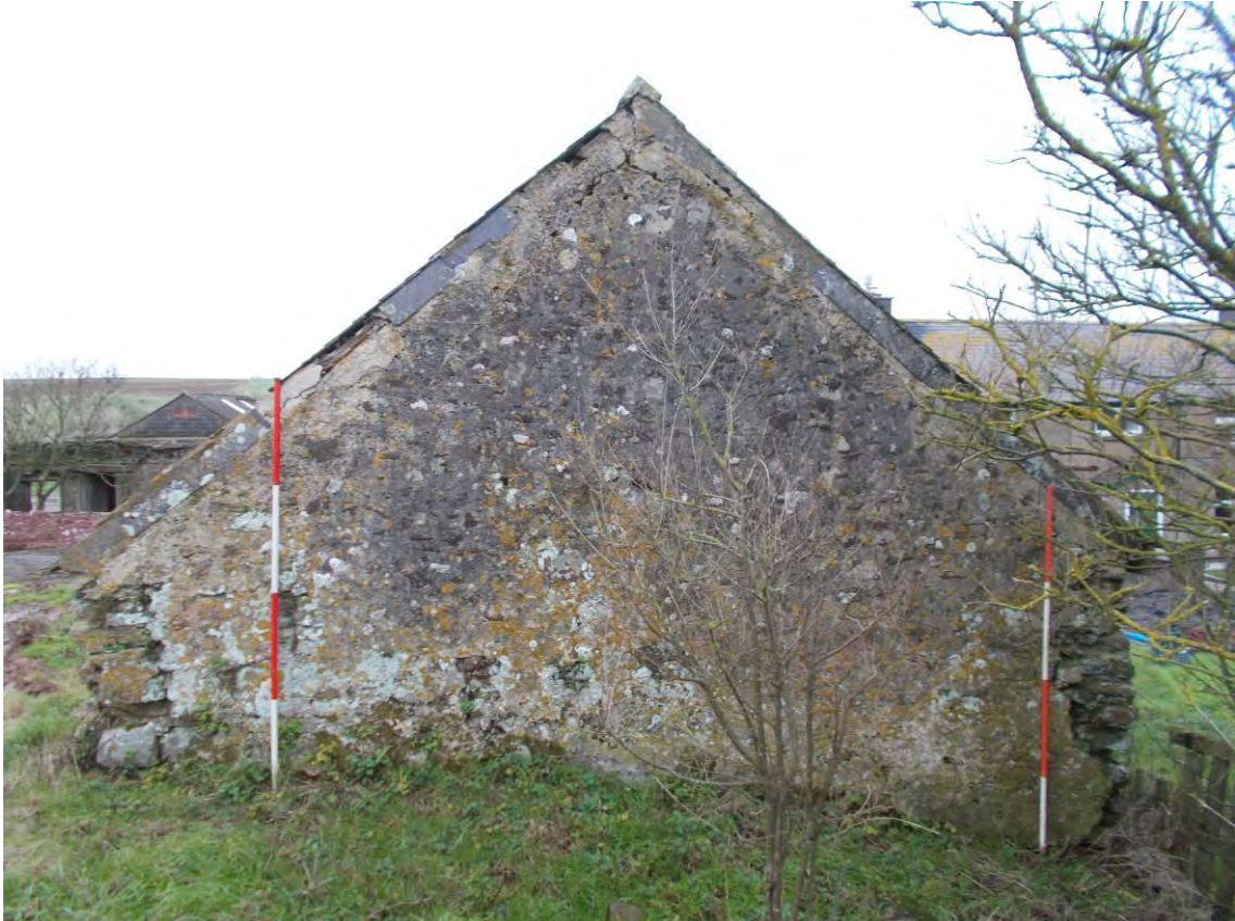
Photo 66: The Cart Shed, southern (gable) elevation. Looking North. 2m scales.
