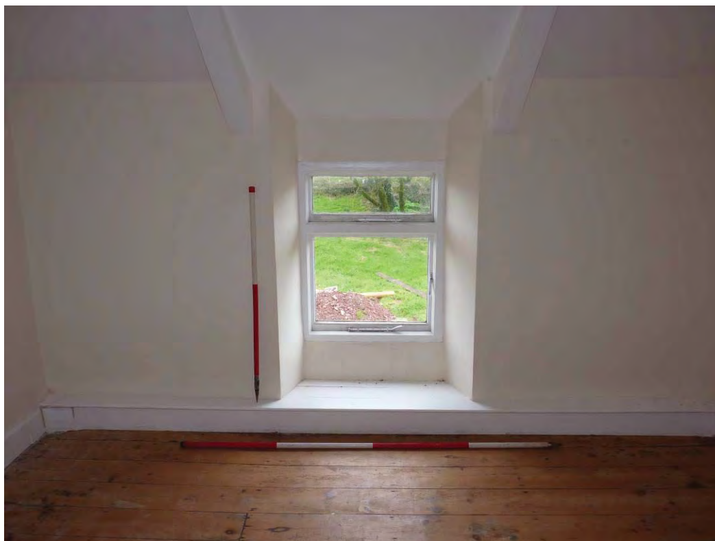
Photo 24: The Farmhouse interior, 1 st floor, Room 7. Looking South. 1m & 2m scales.
