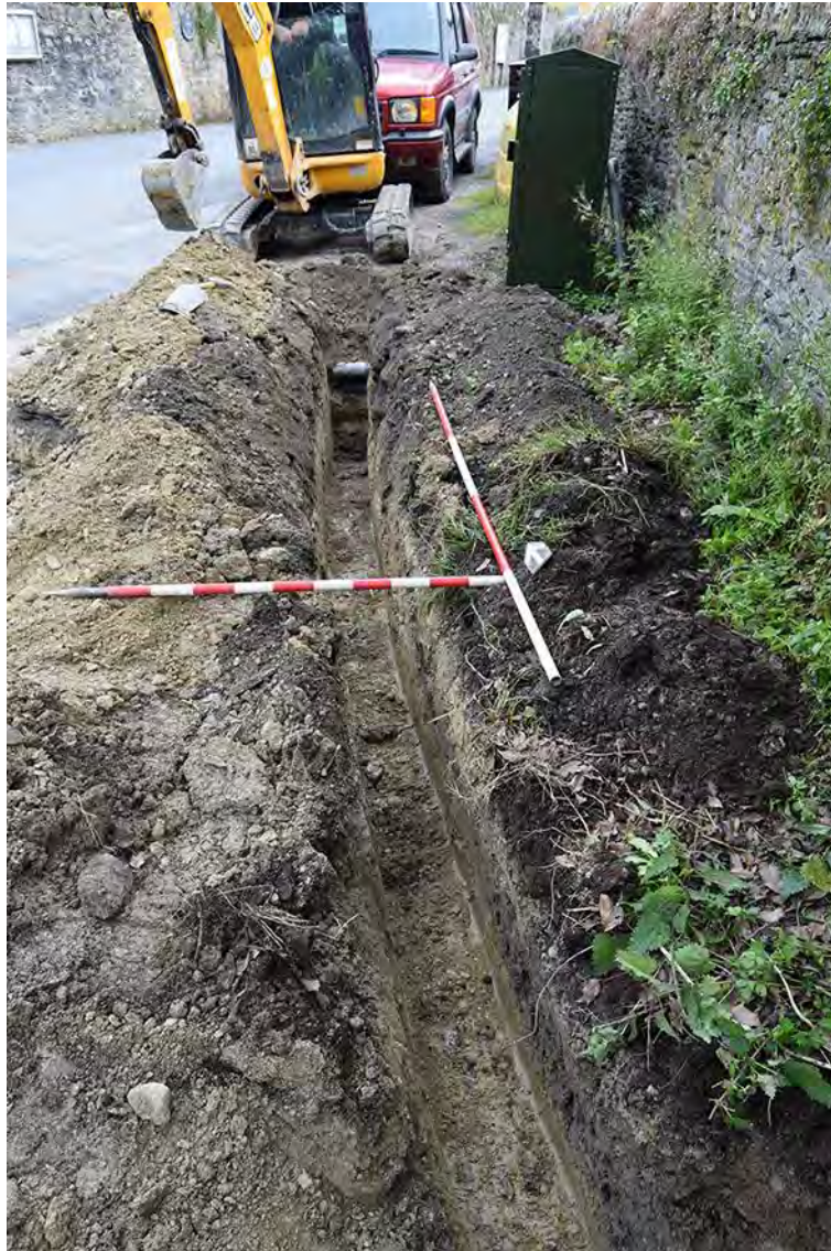
Plate 4: View north of fully excavated trench (1m and 2m scale).
