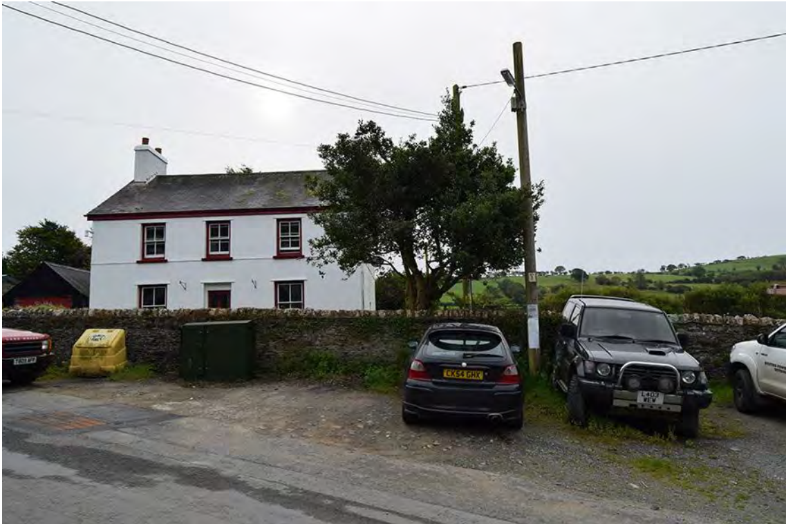
Plate 1: General shot of site from Church Street, facing southeast. Prior to commencement of groundworks.
