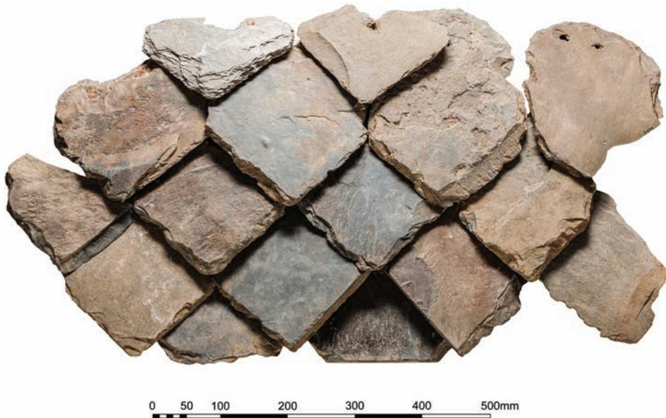
Fig. 22. Reconstructed section of the slated Roman roof from Abermagwr villa. Note the two triangular ridge-top slates, and the flat-edged slates at the base of the roof. Scale 1:8. Photograph by Iain Wright, © Crown copyright, RCAHMW.
