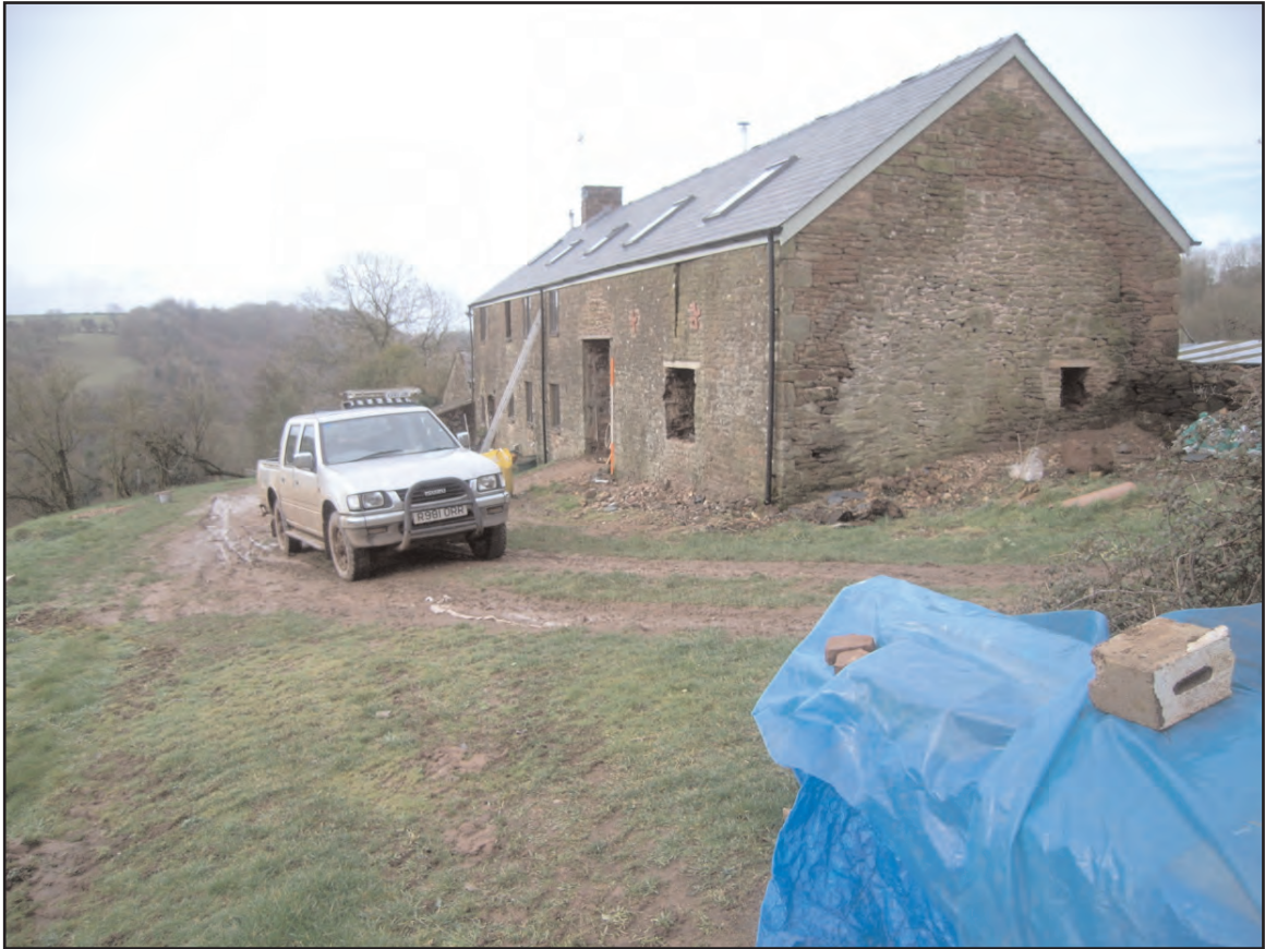
Plate 3 Llwyna farm barn, looking west
