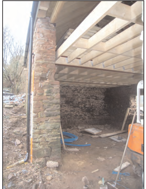
Plate 14 North-western wall showing differing thickness of upper & lower storeys, looking north-east
