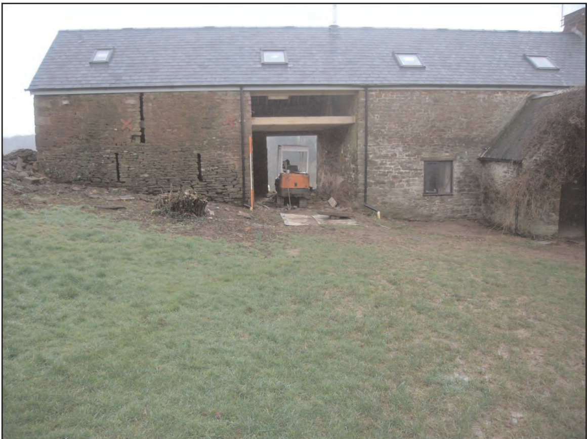
Plate 4 Llwyna farm barn, looking south-east
