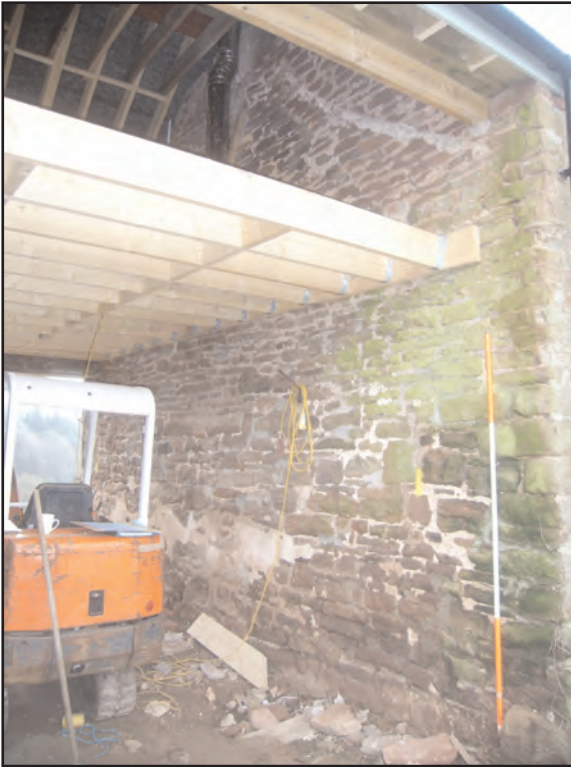
Plate 13 Southern gable showing roofline scar, looking south
