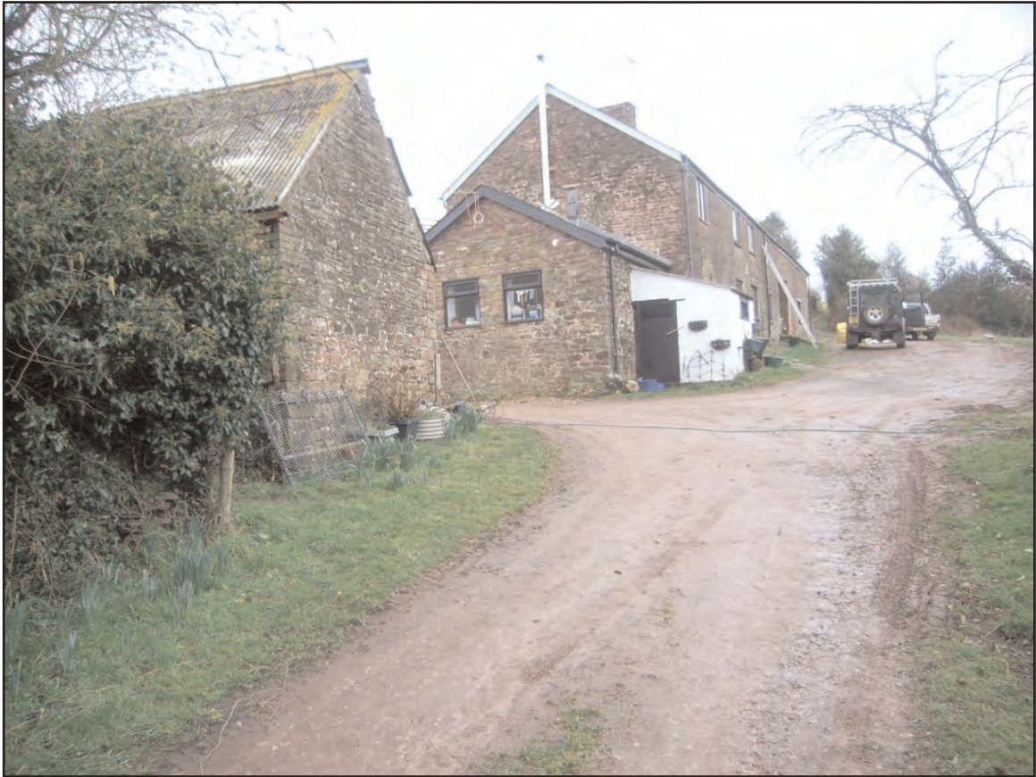
Plate 1 Llwyna farmhouse, attached barn and single-storey outbuilding, looking north
