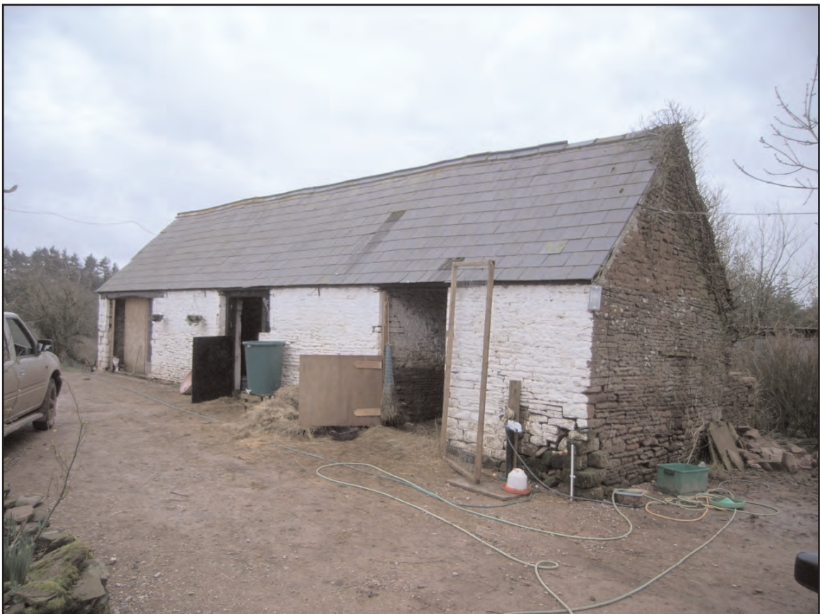
Plate 2 Stable block, looking south
