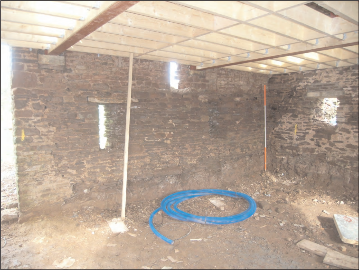
Plate 11 Interior of barn, showing window in gable wall and surviving timber lintel of ventilation slit, looking north
