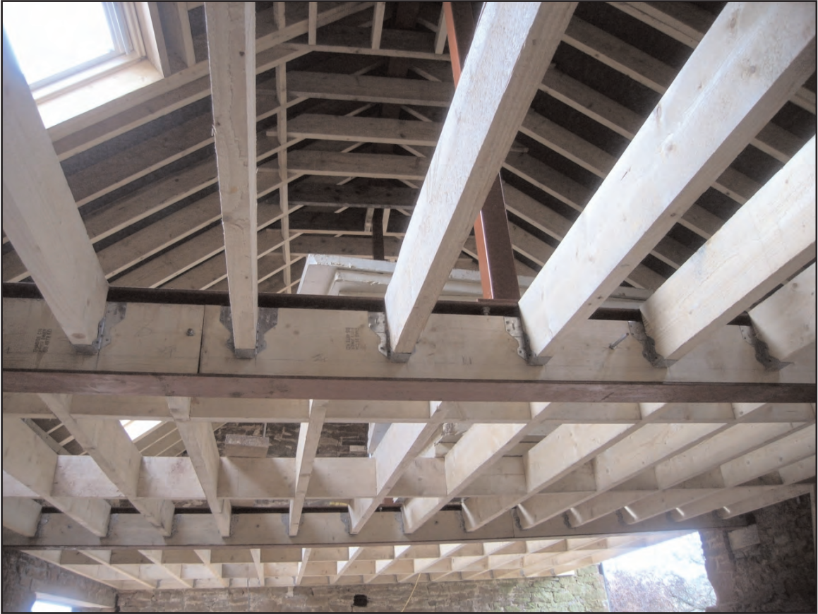
Plate 5 Modern roof and floor joists, looking south-west
