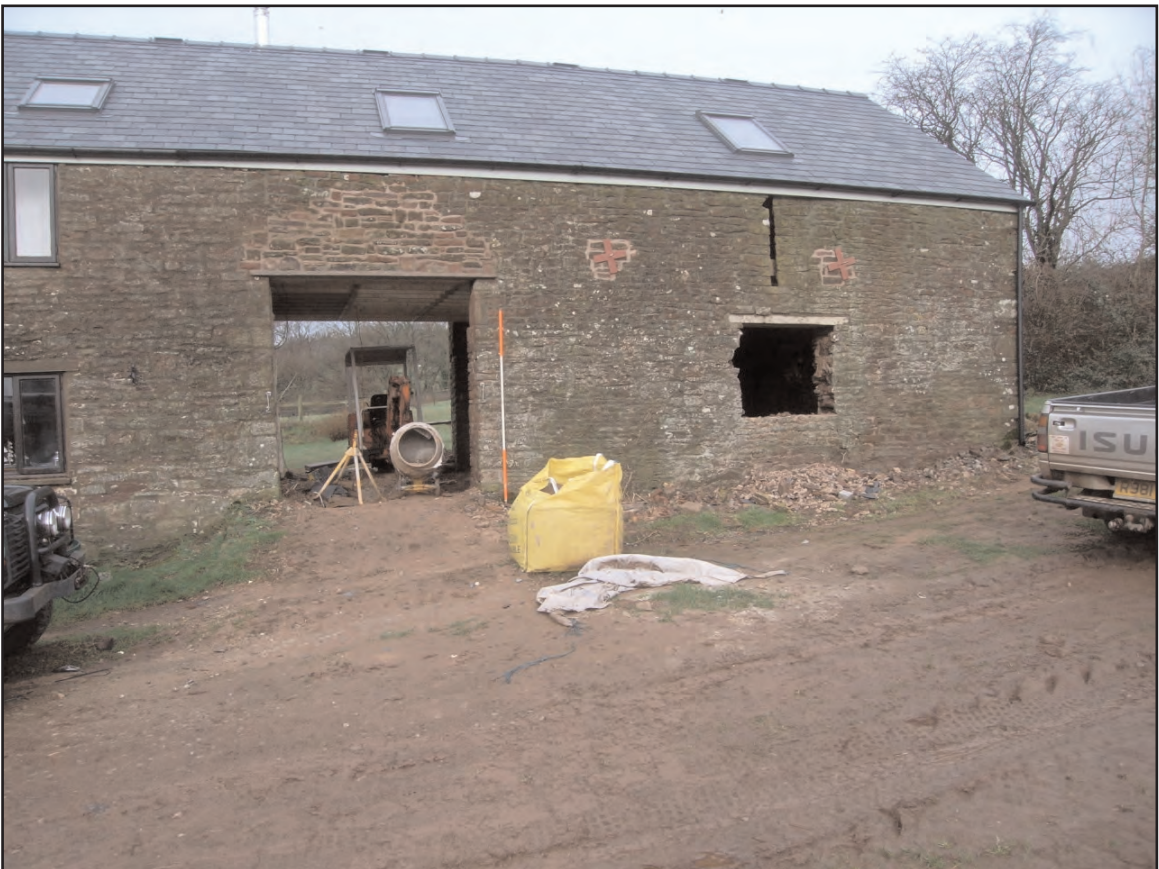
Plate 6 South-eastern side of barn, looking north
