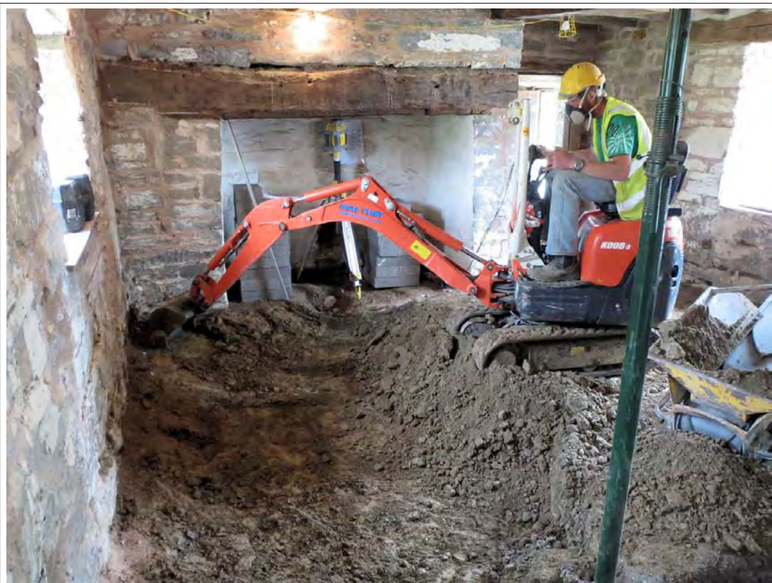
Plate 17. Excavation of internal floor levels (203) (204) within the former hall to allow for a new floor slab. Looking East.
