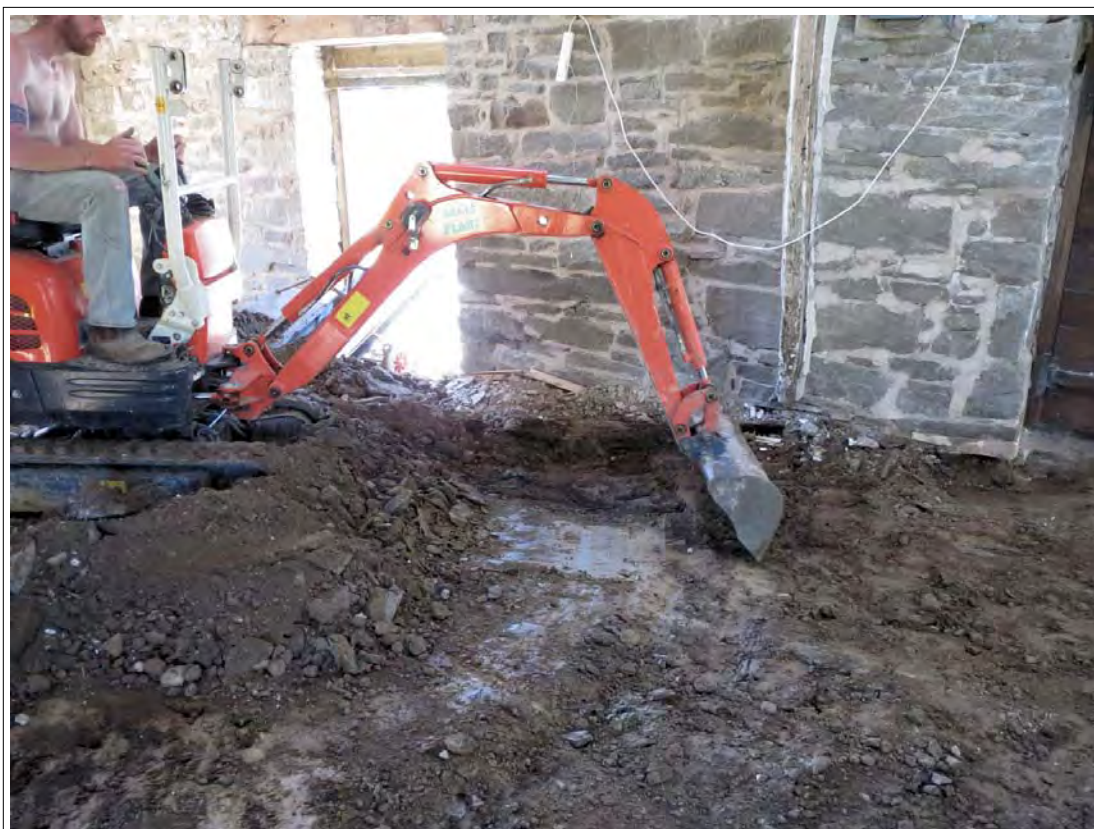
Plate 28. Excavation of internal floor levels (306) (307) within the former barn to allow for a new floor slab. Looking South-South-East.
