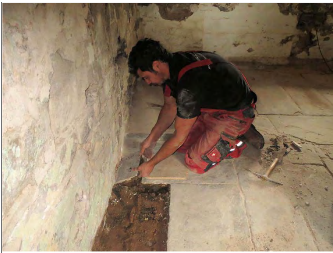
Plate 3. Working shot of the stone flags being lifted within the 'inner-room' (west wall) of the former hall-house. The flagstones (100) were bedded on lime mortar (101), above blinding material (102). Looking North.
