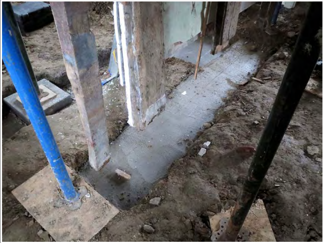
Plate 15. Foundations for the western timber partition supporting the staircase (as located within the 18 th century farmhouse). A partition at this location formerly divided the 15 th century hall and the 'inner-room'). Looking South-East.
