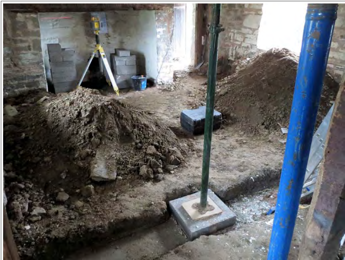
Plate 16. Foundations for the eastern timber partition supporting the staircase (as located within the 18 th century farmhouse). This area was formerly located within the 15 th century hall. Looking South-East.
