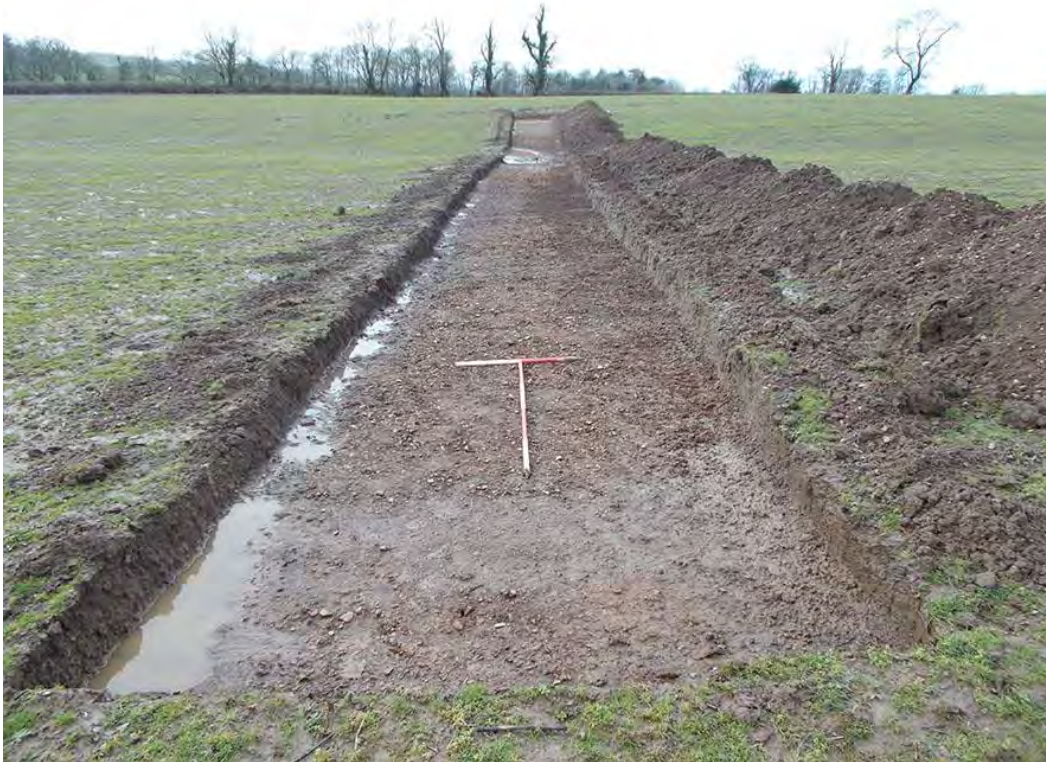
Photo 47: Looking west along Trench 7. 2m & 1m scale.
