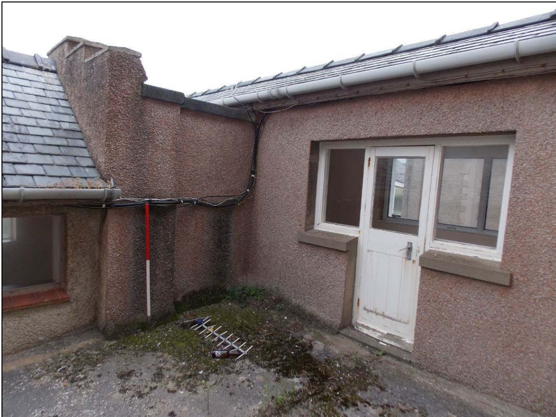
Plate 32: Walkway between Buildings A and B, looking south-west (scale 1m).
