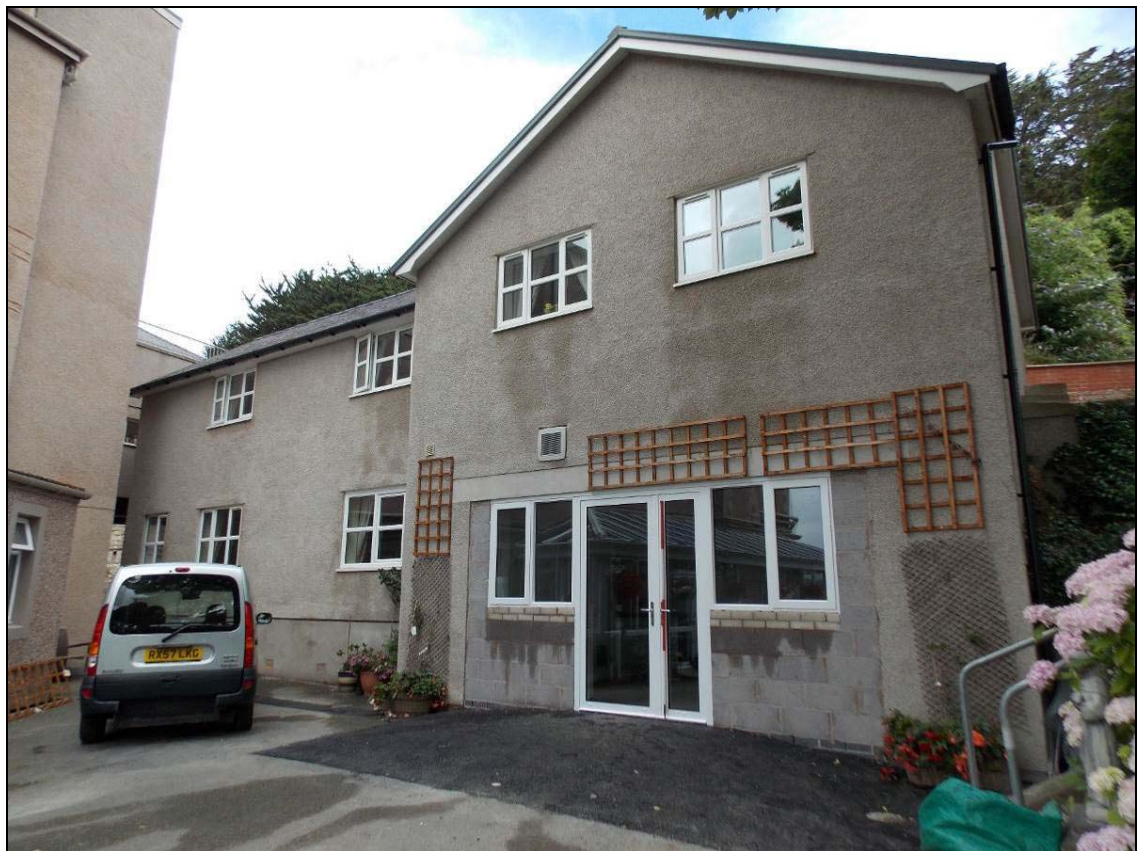
Plate 57: South elevation, looking north-west (scale 2m).
