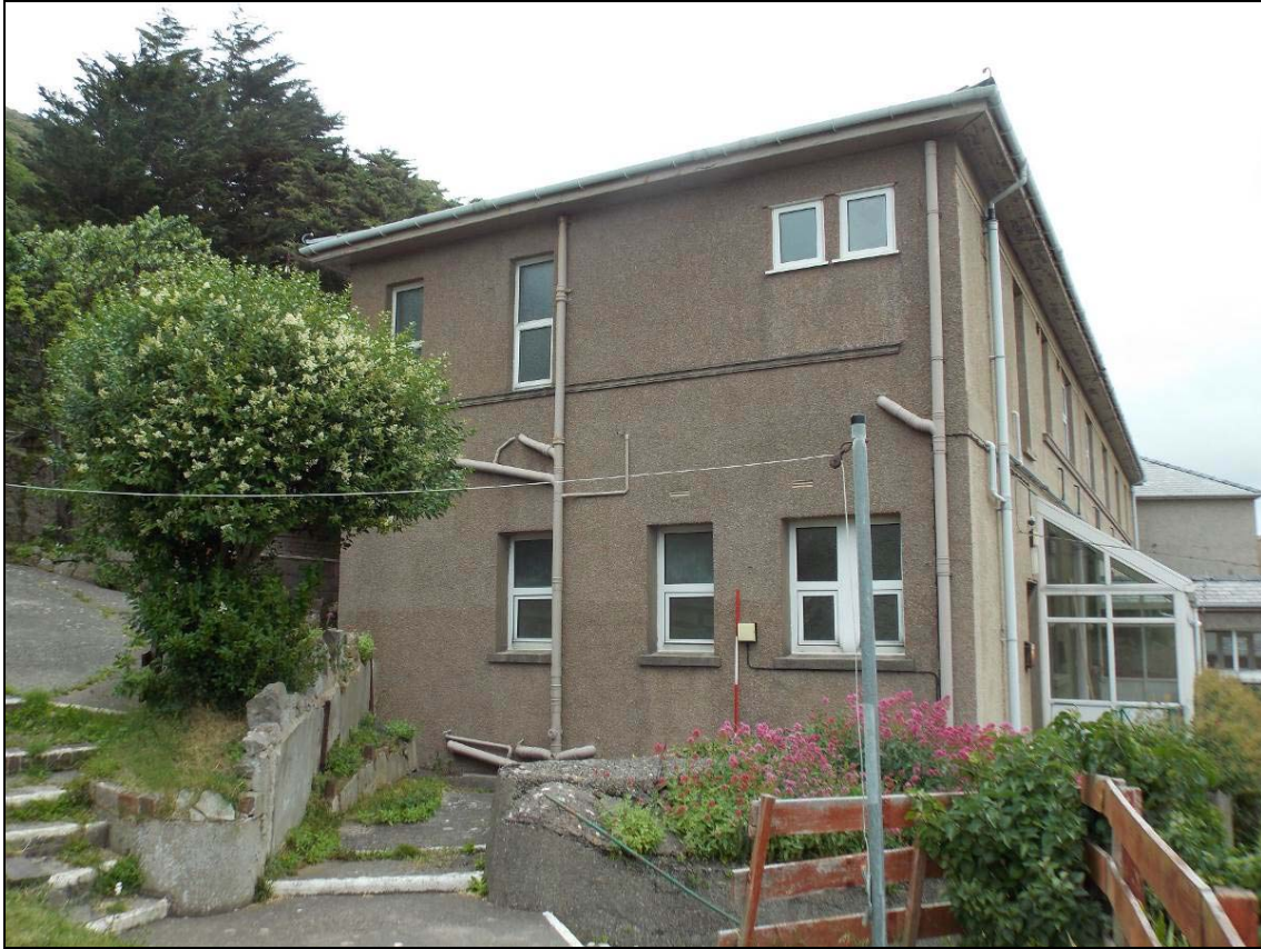
Plate 4: West elevation of Building A, looking east (scale 2m).
