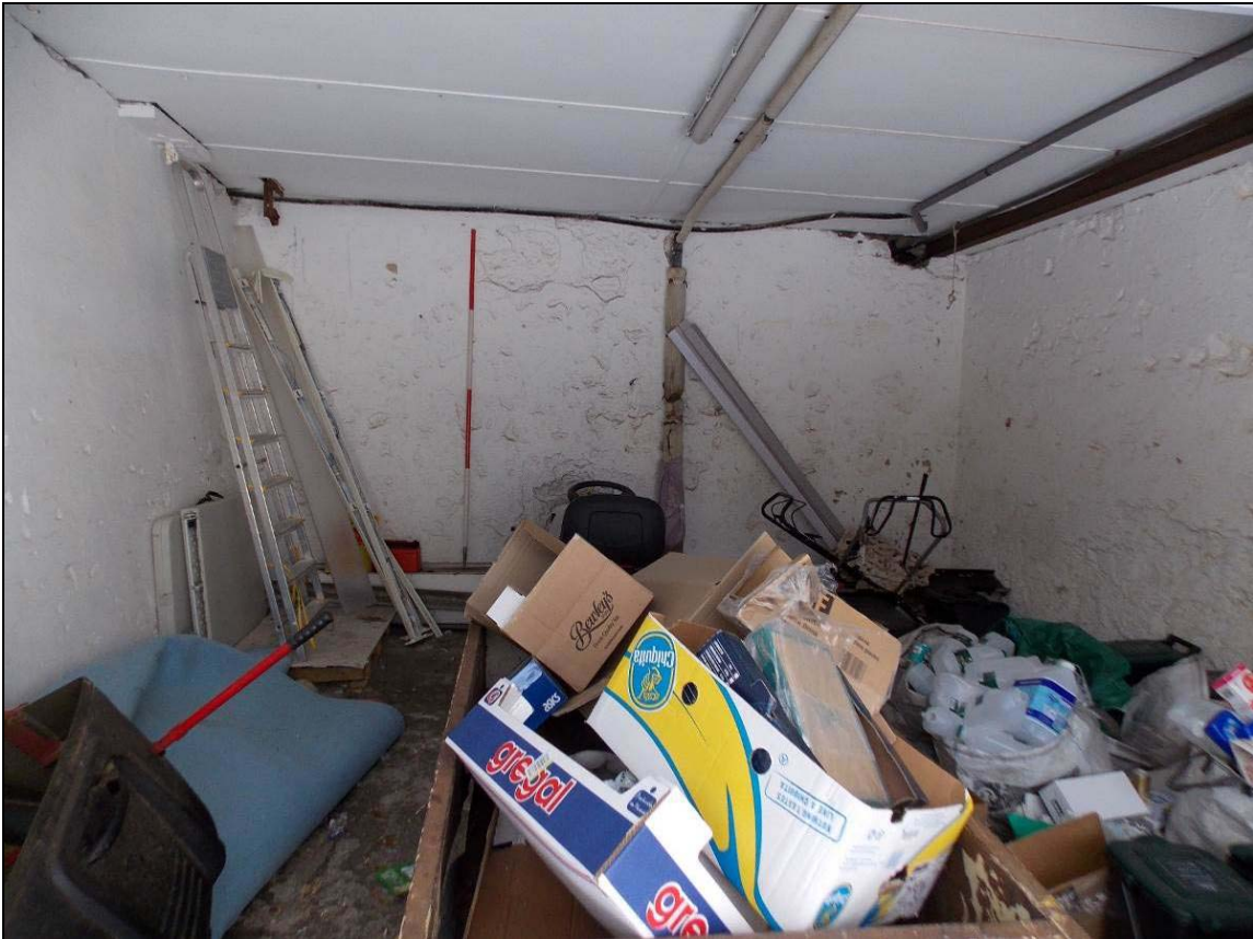
Plate 45: Internal view of the garage, looking west (scale 2m).
