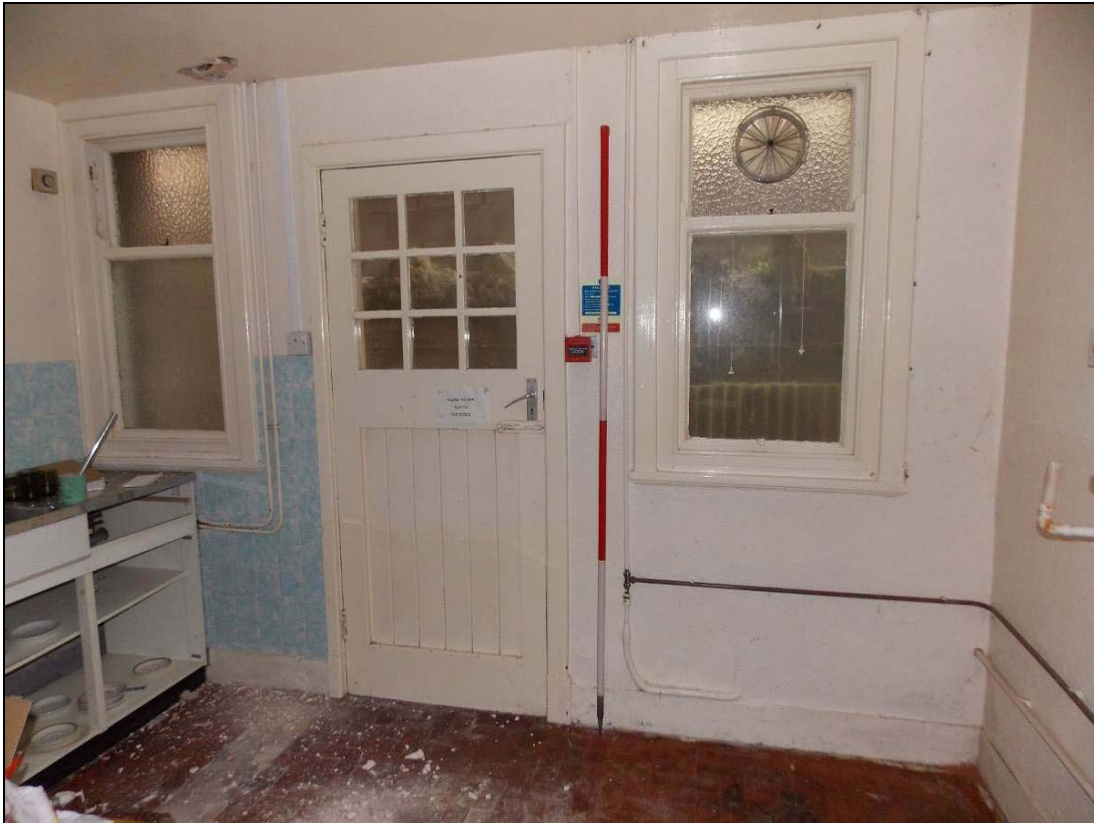
Plate 16: Kitchen room, looking north-west (scale 2m).
