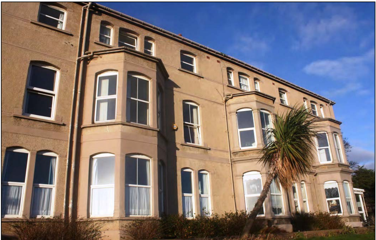
Plate 75: Detail of bay windows within the front façade of Loreto Convent, looking north-east.
