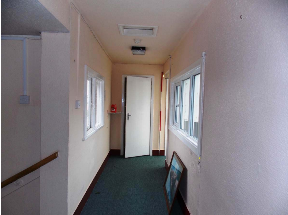
Plate 36: Inside walkway between Buildings A and B, looking south (scale 2m).
