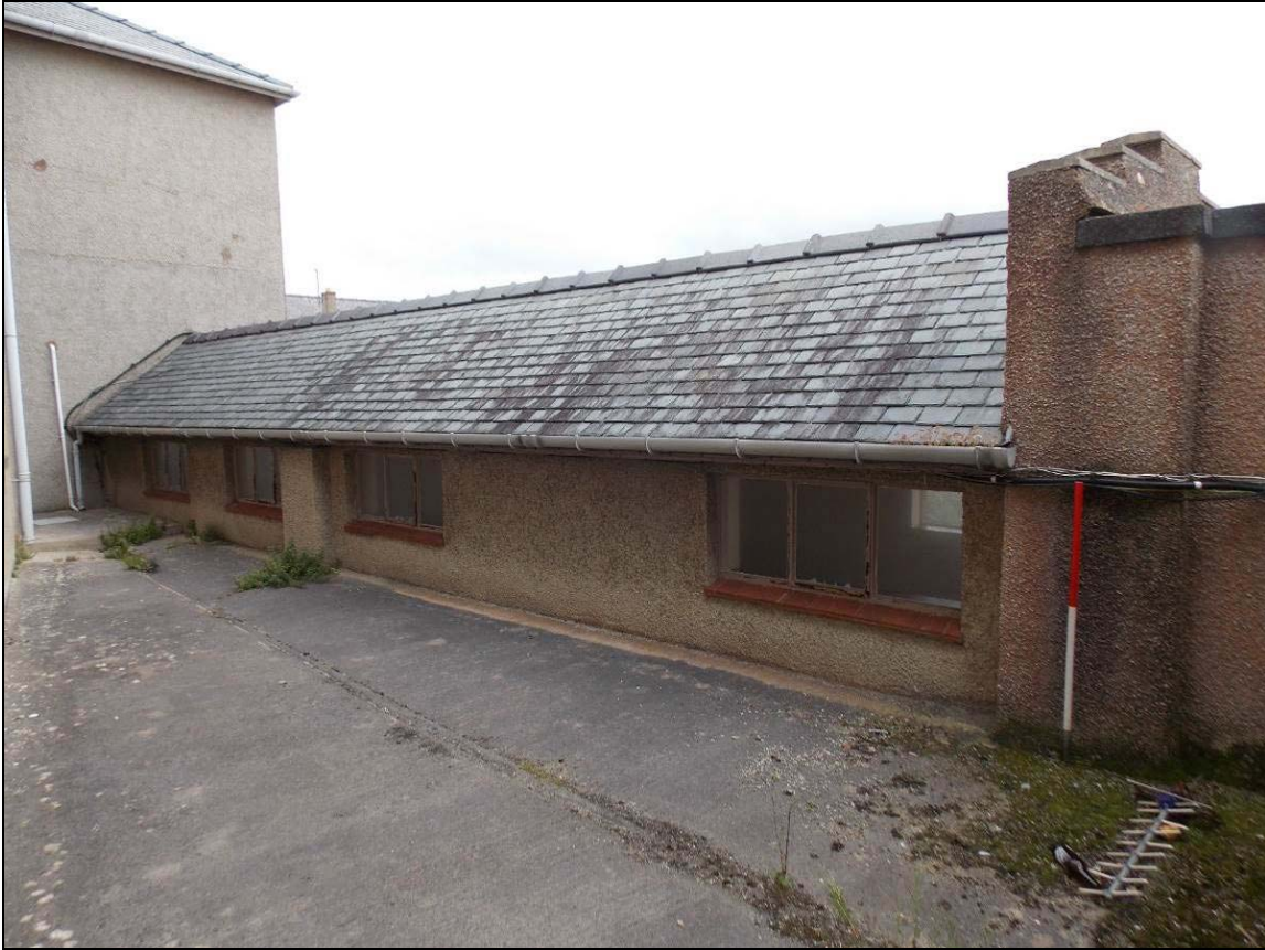
Plate 31: North elevation of Building B, looking south-east (scale 1m).
