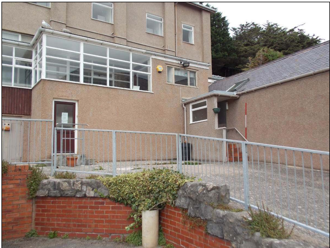
Plate 40: Projecting staircase porches, looking north-east (scale 2m).
