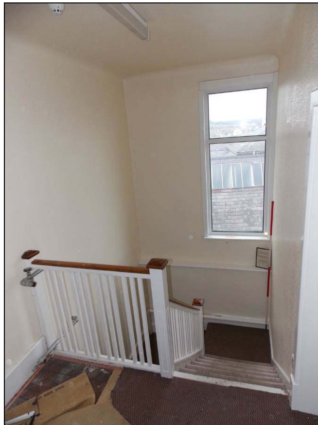
Plate 21: General view of the staircase's lobby, looking south (scale 2m).
