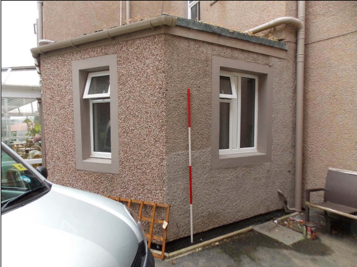
Plate 68: Detail of single-storey lavatory block, looking south-west (scale 2m).
