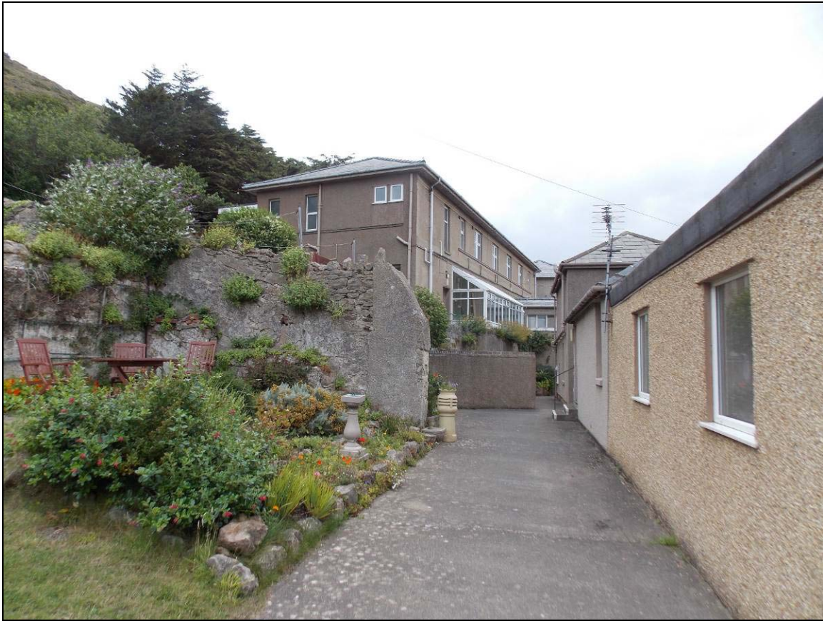
Plate 2: Front south elevation viewed from an alleyway behind the Hall, looking east.
