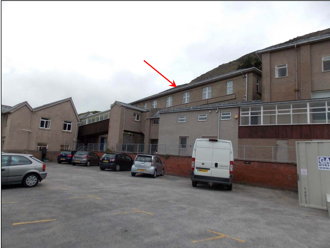
Plate 1: General view of Building A (arrow) facing onto the delivery car park, looking north-west.
