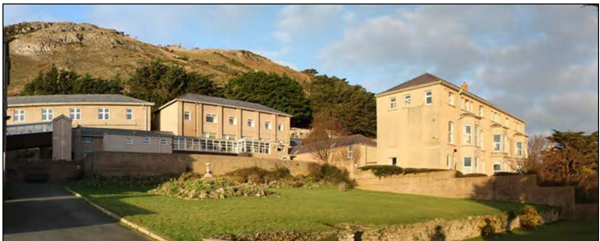
Plate 71: Front terrace to the west of Loreto Convent, looking north-east.
