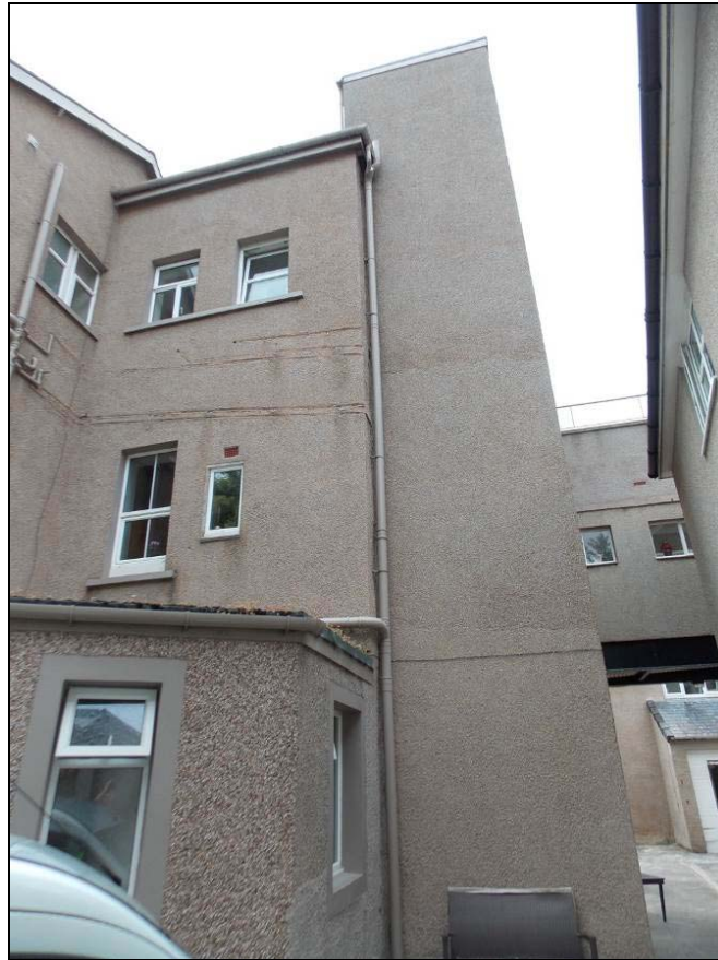
Plate 69: Projecting lift tower, looking west.
