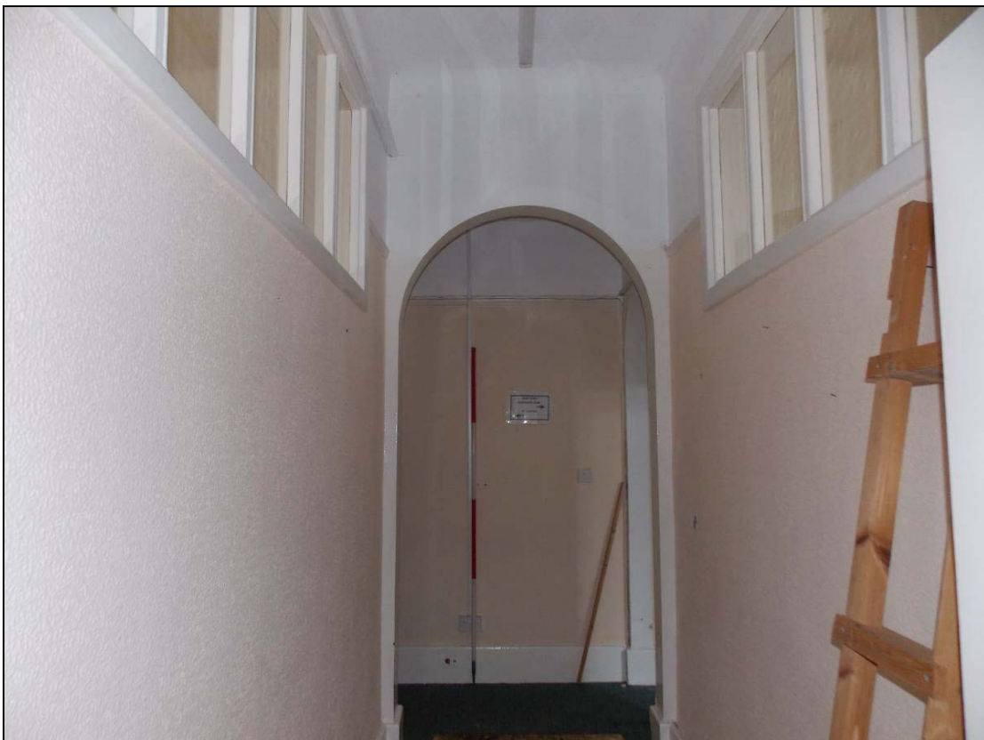
Plate 11: Principal arched doorway of the ground floor, looking north (scale 2m).
