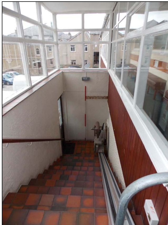
Plate 44: Staircase leading to Our Lady's Centre, looking west (scale 2m).
