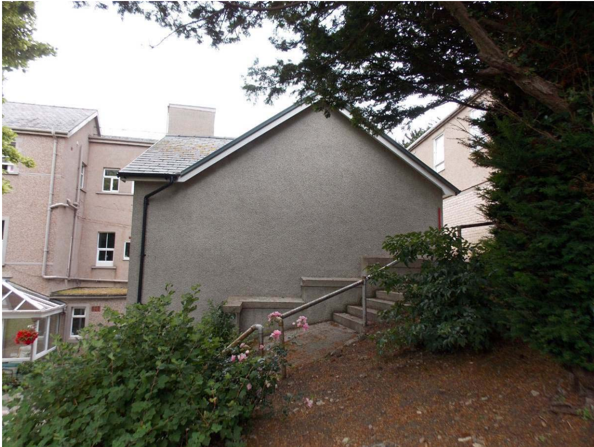
Plate 58: East elevation, looking west (scale 2m).
