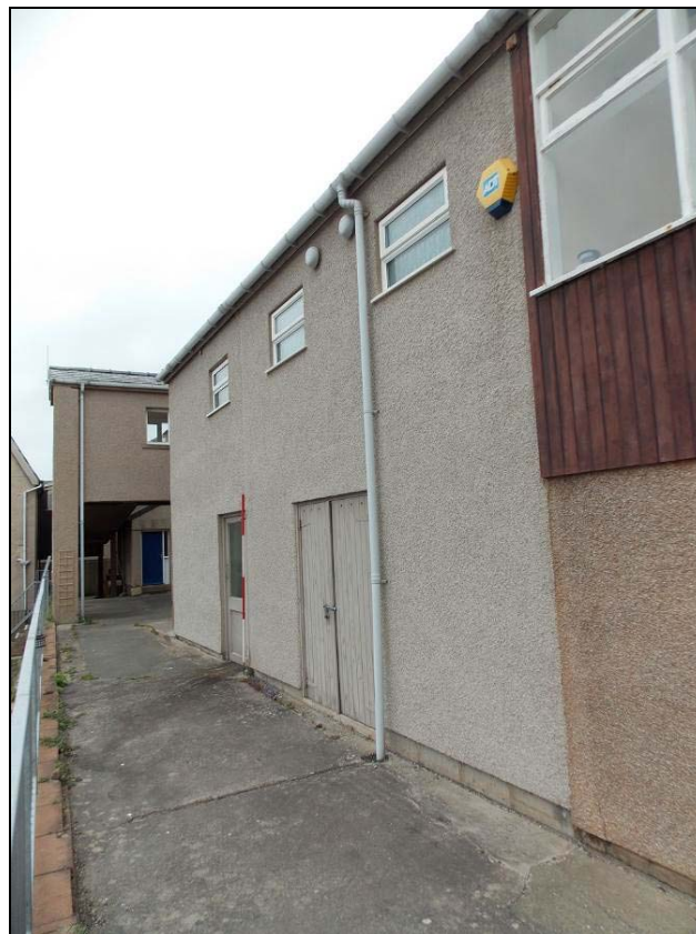
Plate 30: South elevation, looking west (scale 2m).
