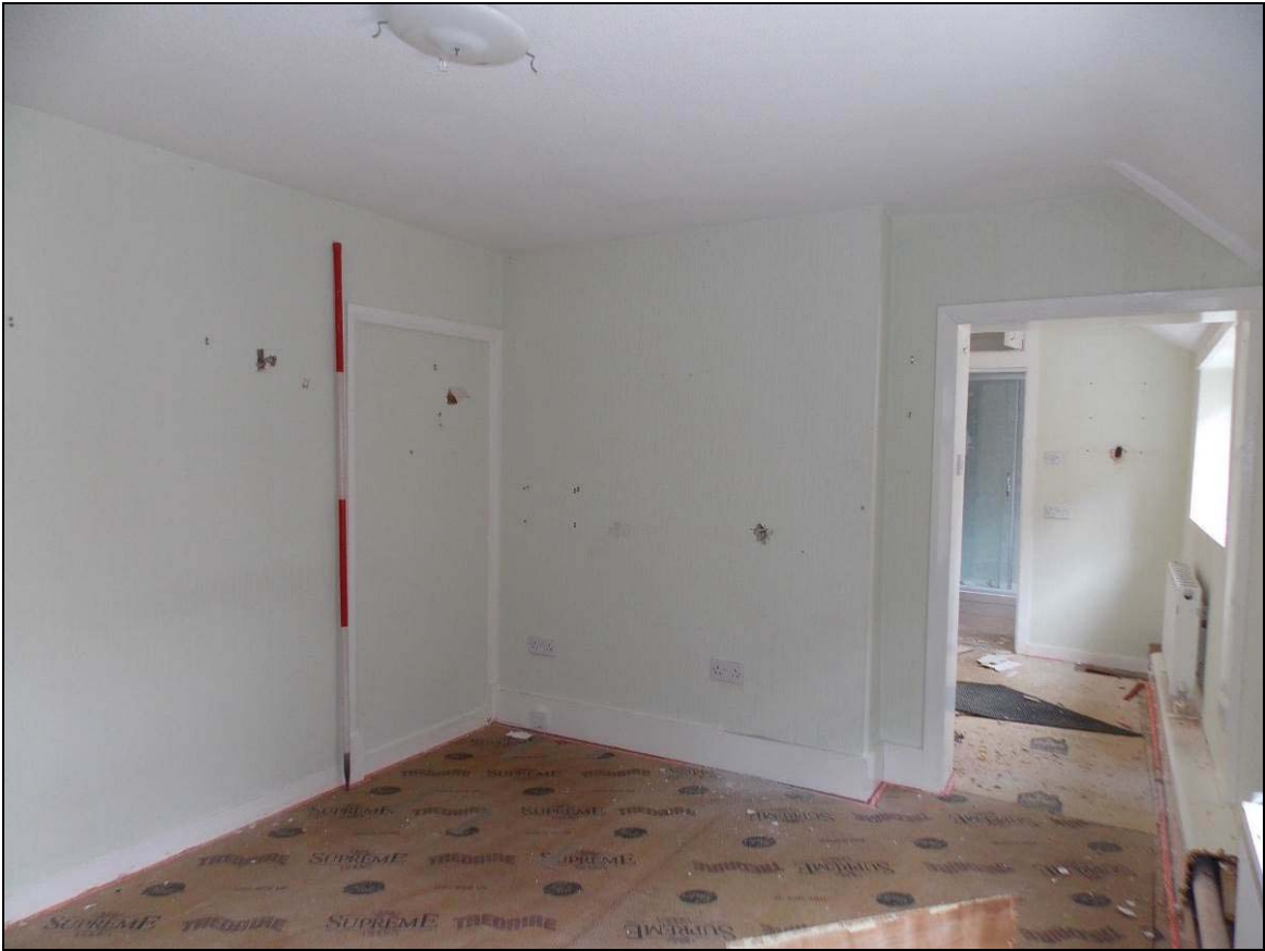
Plate 51: Central room, looking north-west (scale 2m).
