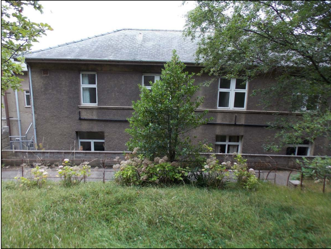
Plate 6: Rear north elevation of Building A, looking south.
