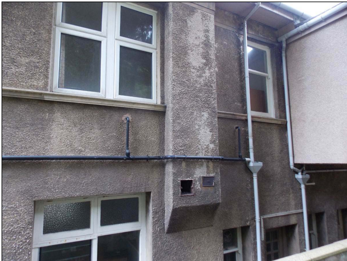
Plate 7: Detail of projecting chimney stack within the north elevation, looking south-west.
