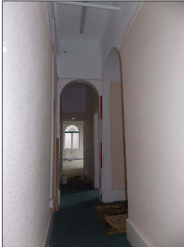
Plate 12: General view of the central corridor, looking east (scale 2m).
