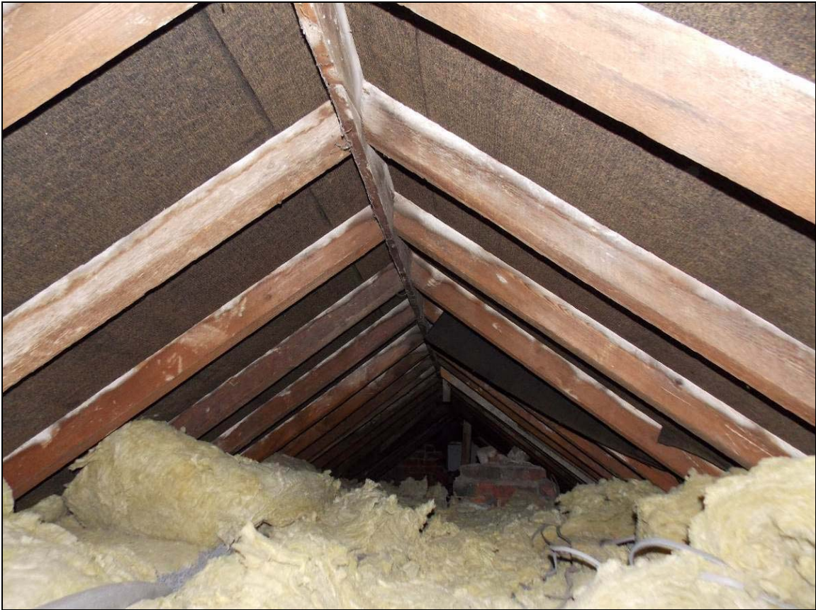
Plate 53: Roof structure within the loft northern area, looking south.
