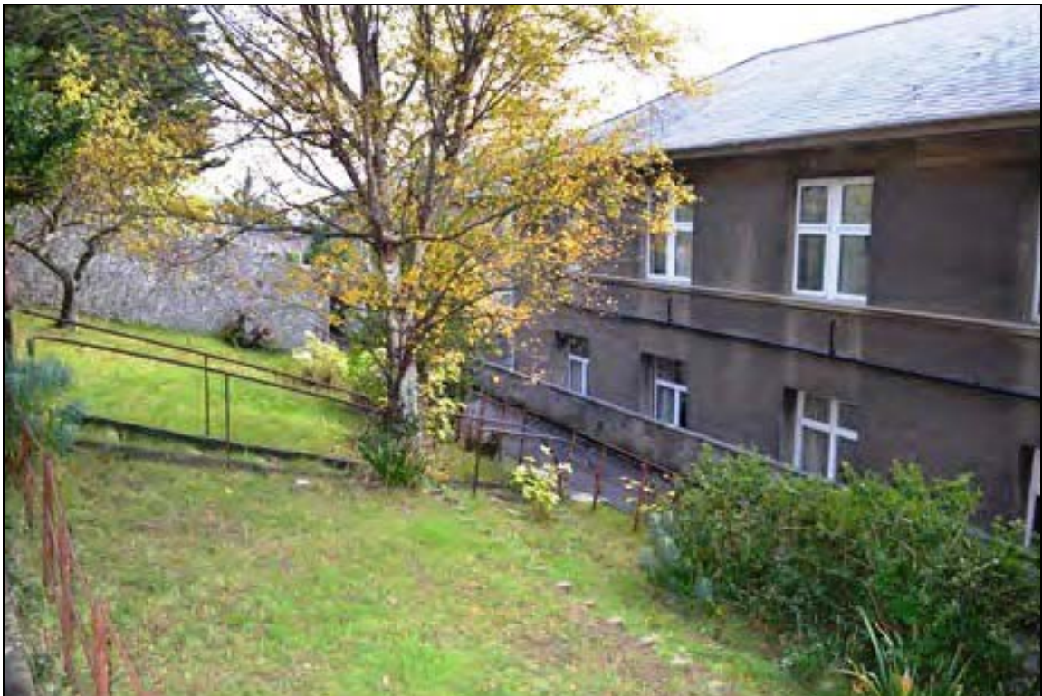
Plate 79: Terraced garden area to the rear of St Joseph's Centre (Building A), looking east.
