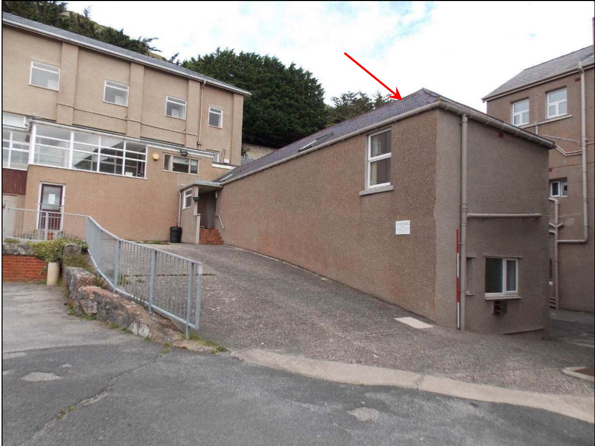
Plate 39: Building C (arrow) viewed from the delivery car park, looking north-east (scale 2m).
