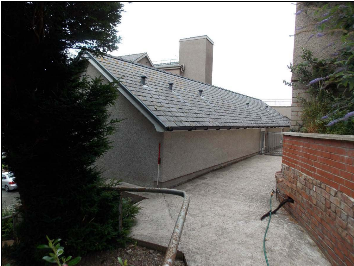
Plate 59: North elevation, looking west (scale 1m).
