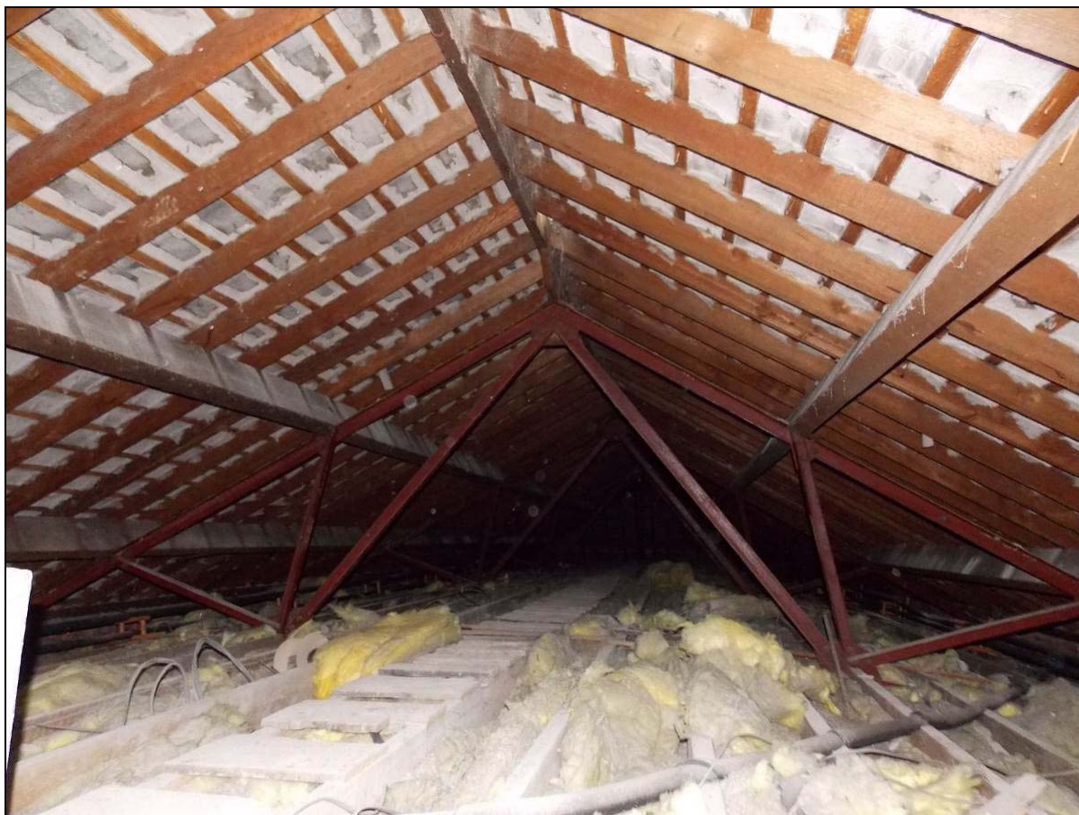
Plate 28: Roof structure inside the loft, looking east.
