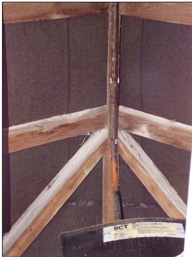
Plate 54: Hipped roof structure within the southern end, looking south.
