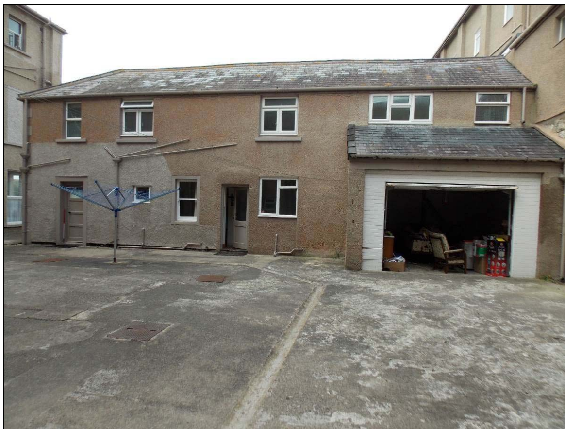
Plate 42: East elevation with projecting garage block, looking west (scale 1m).
