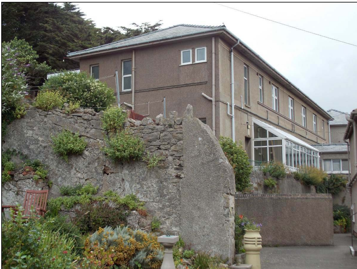
Plate 3: West and south elevations, looking north-east.
