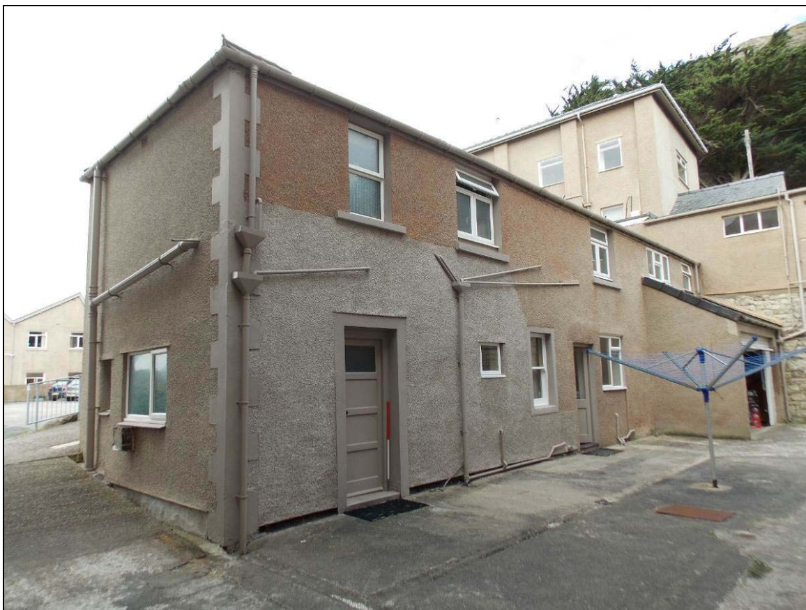
Plate 41: South and east elevations of Building C, looking north-west (scale 1m).
