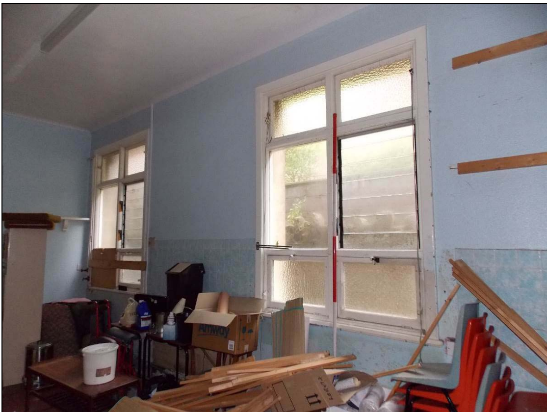
Plate 15: Northern meeting room, looking north-west (scale 2m).
