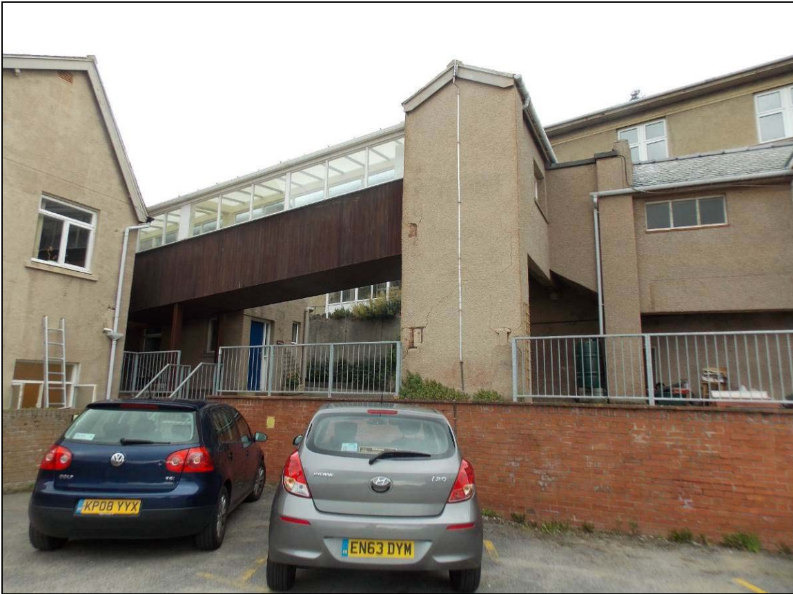
Plate 33: Walkway to the rear of Clifton centre, looking north-west.
