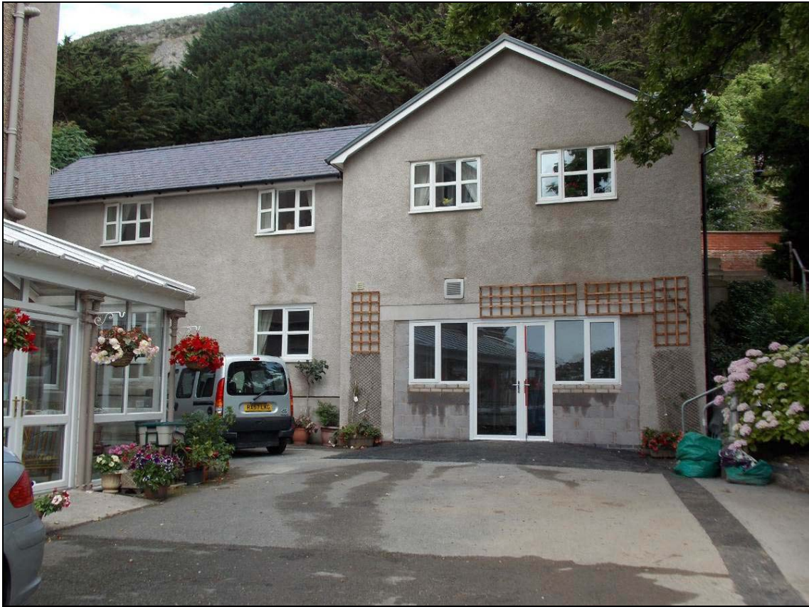
Plate 56: Front south elevation, looking north (scale 2m).
