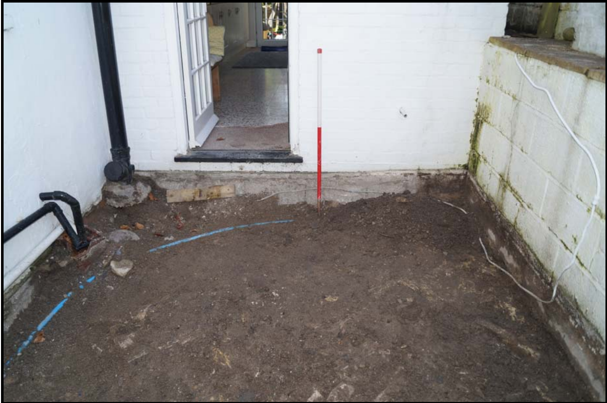
Plate 13: RCL2017_113, general view, looking southwest.
