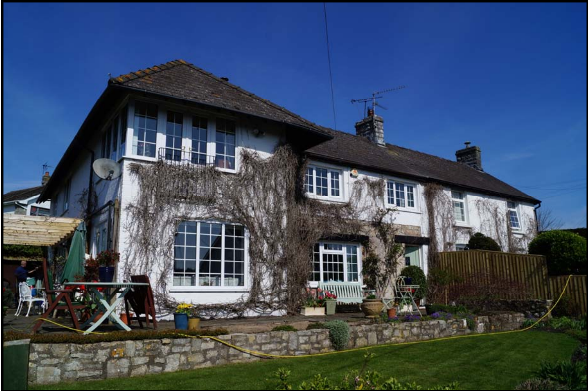
Plate 1: RCL2017_101, The front of Rose Cottage, Llancadle, the southwestern part of the whole building, looking north.
