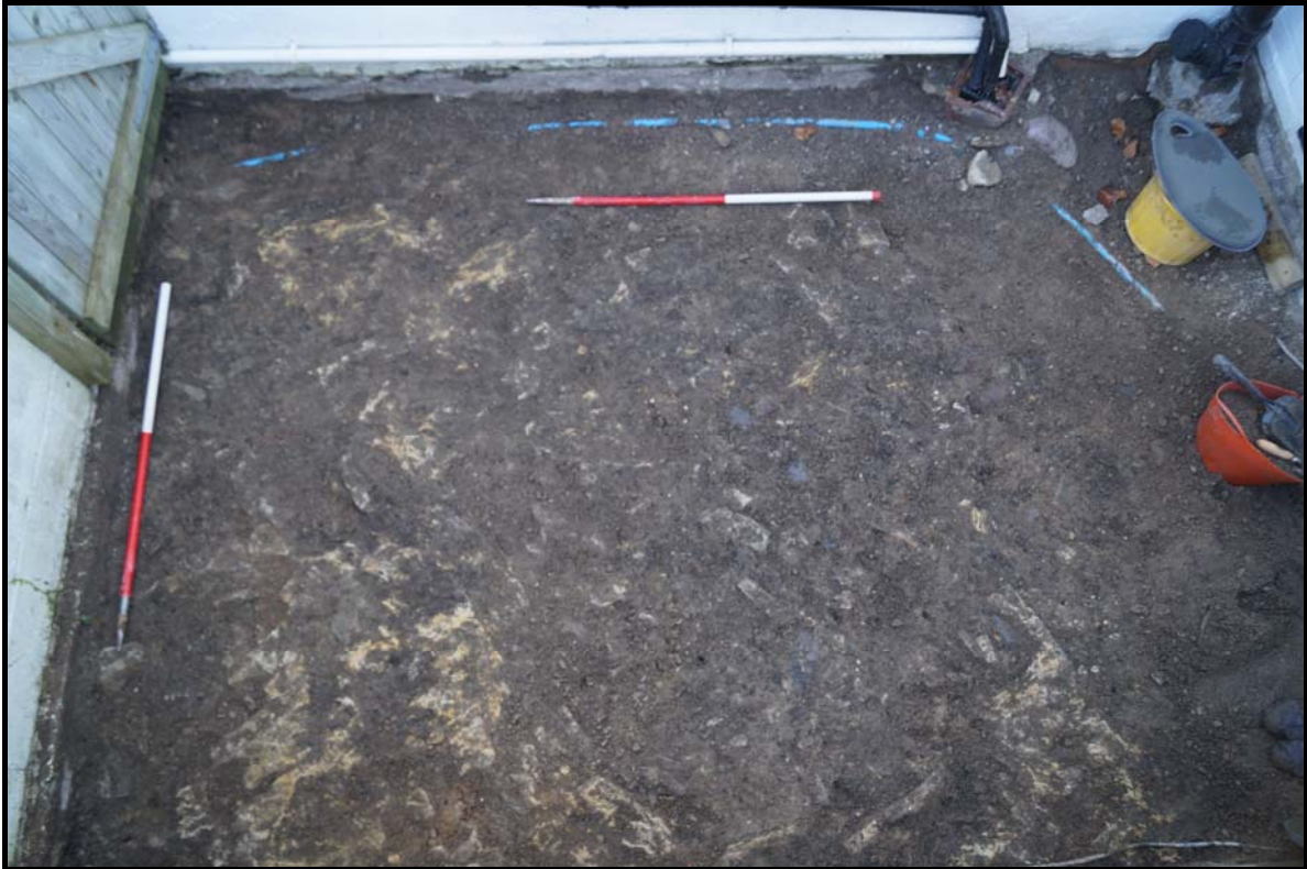
Plate 3: RCL2017_103, after removal of (001) and (005) showing (002)/[003], the modern water pipe trench, and (004) material filling a hollow in (006) natural bedrock, looking southeast..
