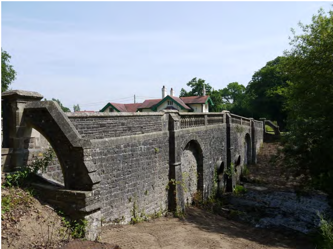
Photo 8. Bridge looking northeast
