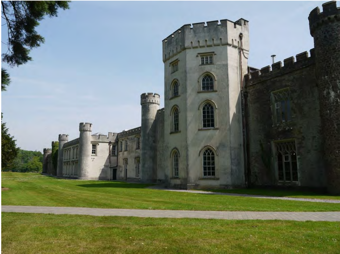
Photo 13. West side of Hensol Castle looking north
