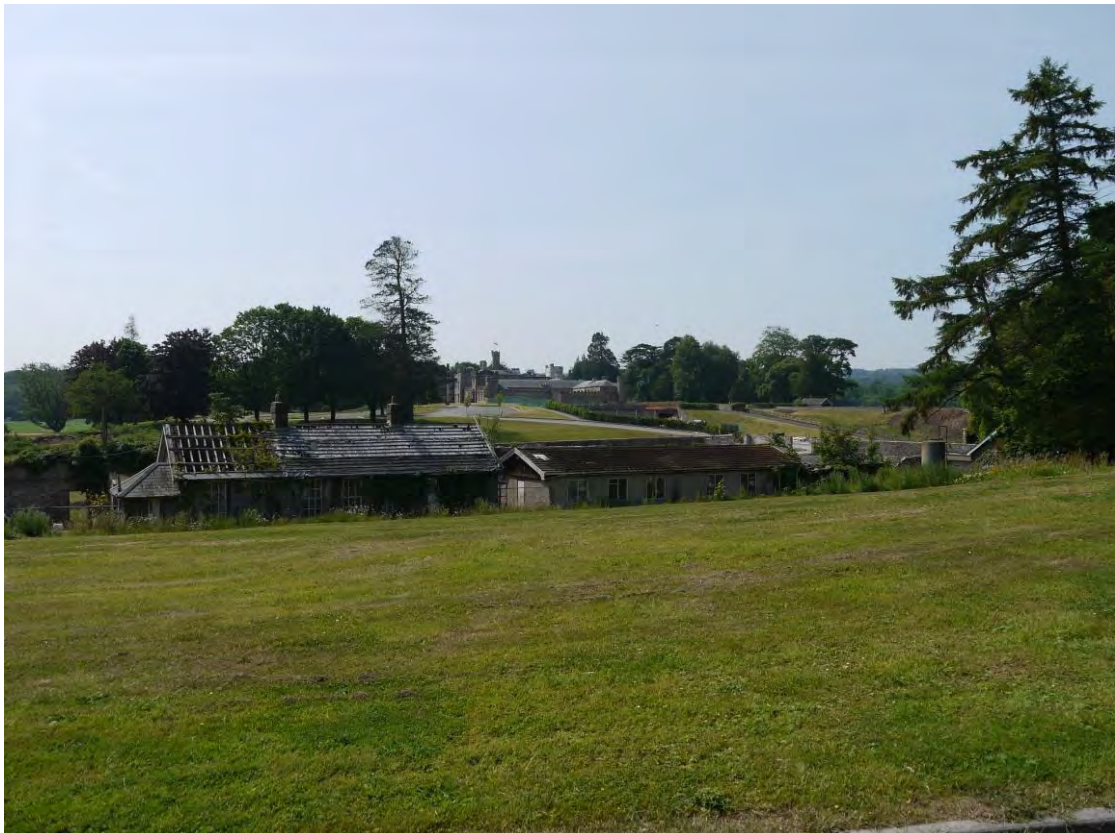
Photo 6. View of Gardeners Mews from road looking south
