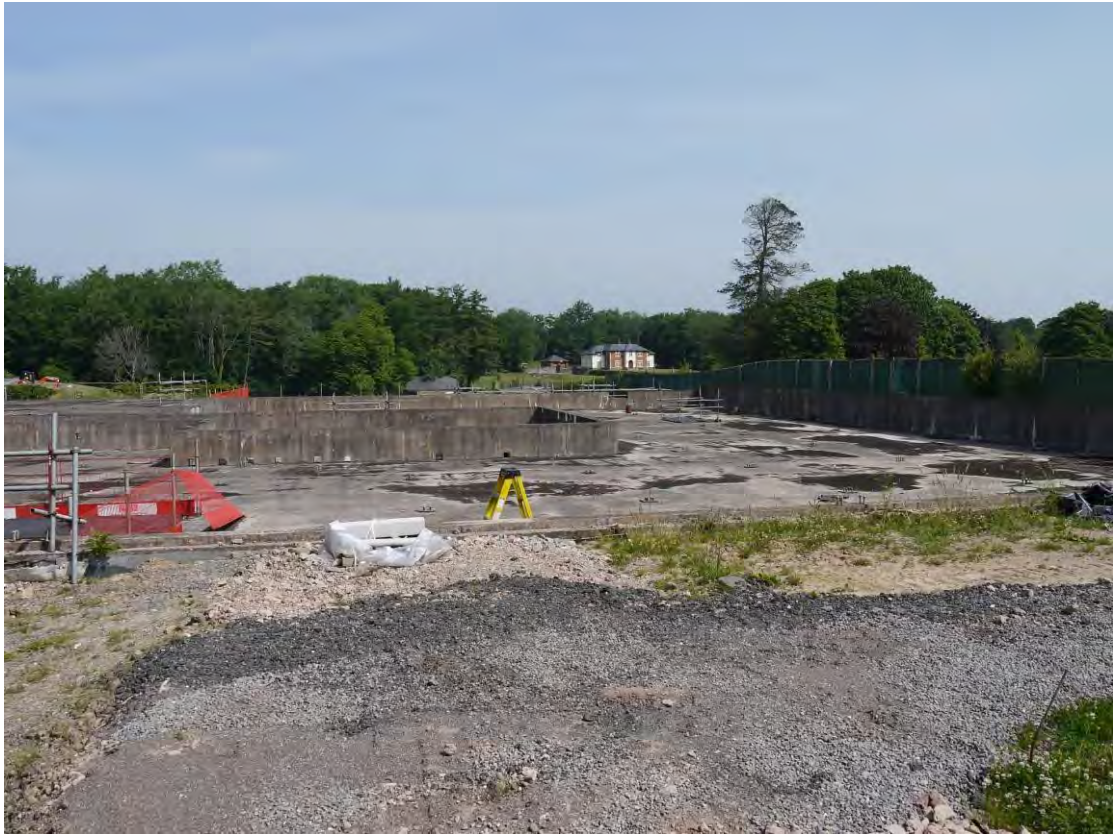
Photo 1. View from rear of Hensol Castle to north
