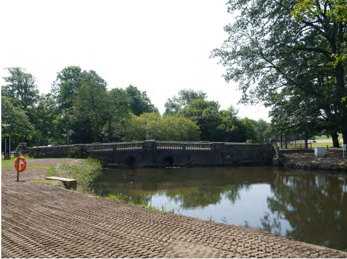
Photo 7. Bridge looking south
