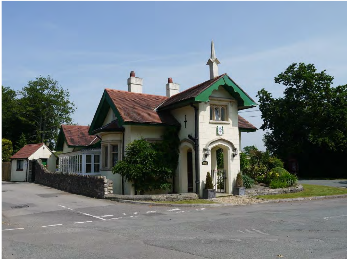
Photo 9. Hafod Lodge looking west
