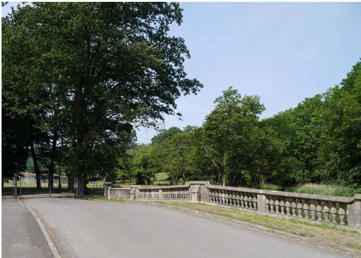
Photo 10. View across bridge looking west to Gardeners Mews
