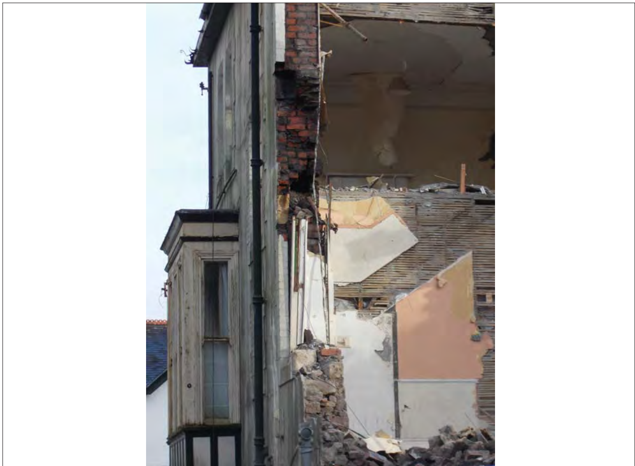
Plate 27: View of external walls during demolition works, showing upper section built in brick. Looking east.
