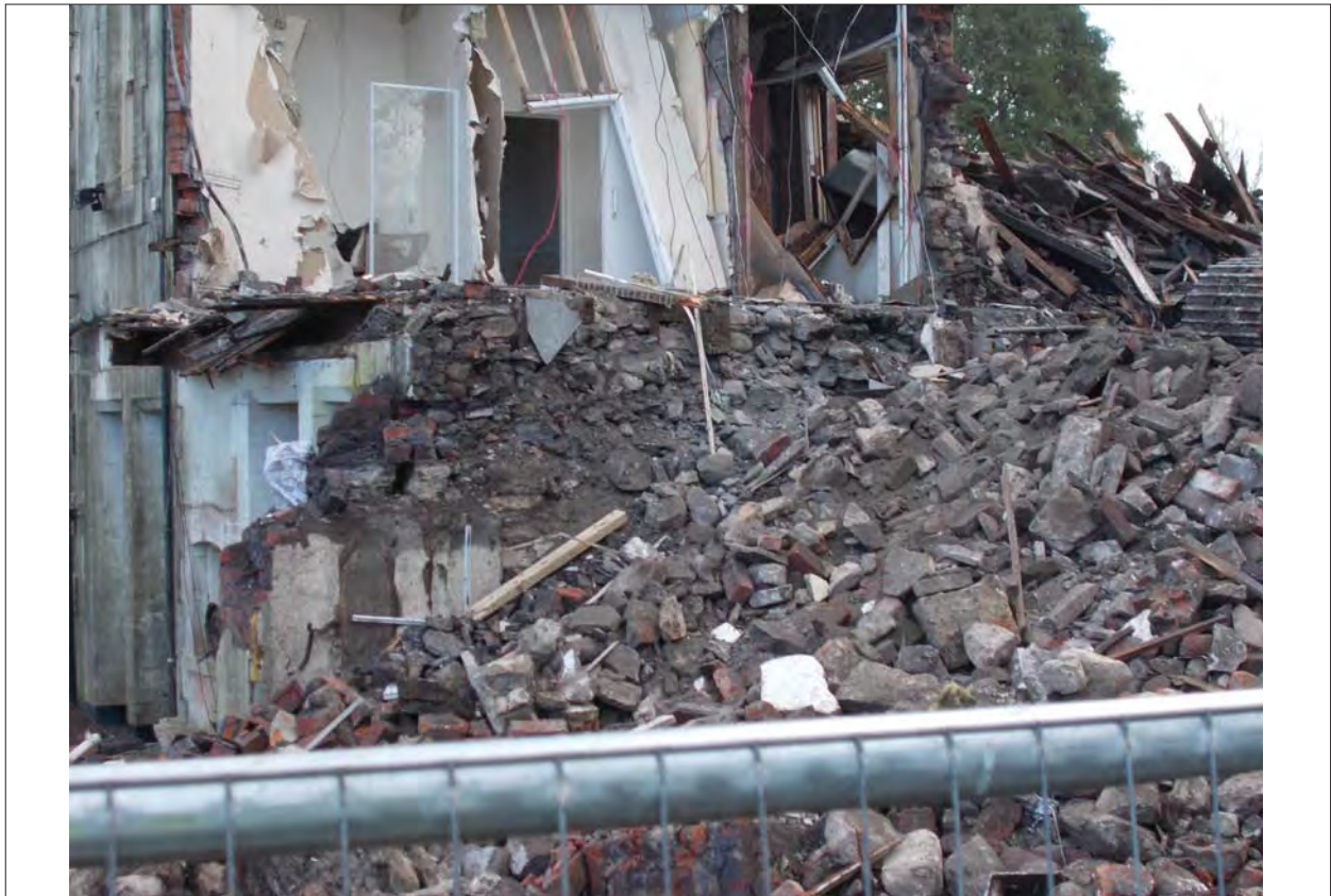
Plate 25: The demolition of the ground floor level of Sketty Isaf House, showing a high concentration of stone in the construction.
