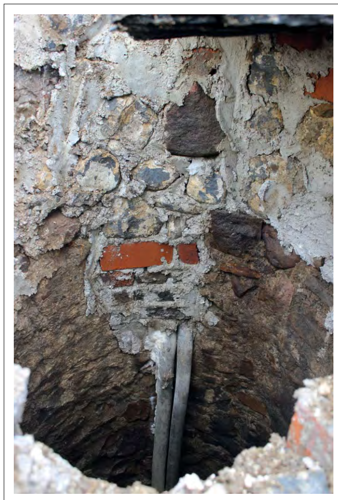
Plate 12: Internal view of upper rebuild [116] (112) of Well 115 and contemporary lead pipework.
