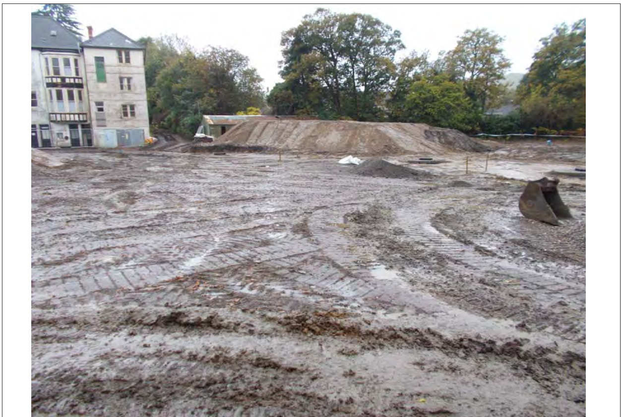
Plate 14: VGeneral shot of soil strip down to natural subsoil (102) in the western part of the site. 2m scale. Looking west.
