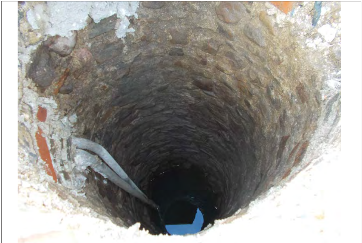
Plate 13: View down well 115, showing lead water pipes to draw water.
