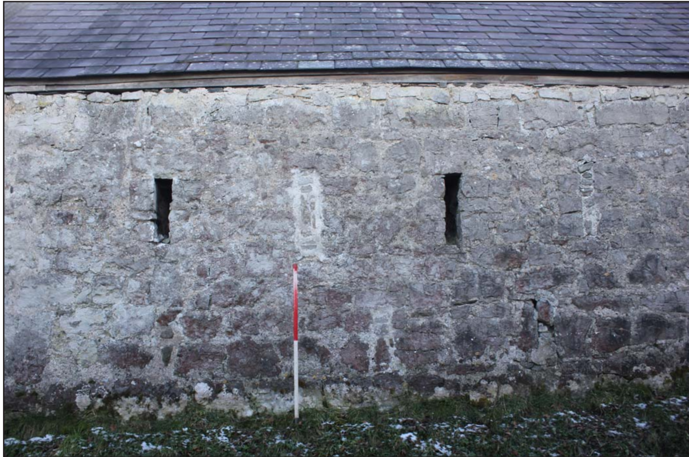
Plate 07: Plas Yn Llan, Cilcain, Flintshire. External shot - central portion of northern elevation - From the north - 1m scale
