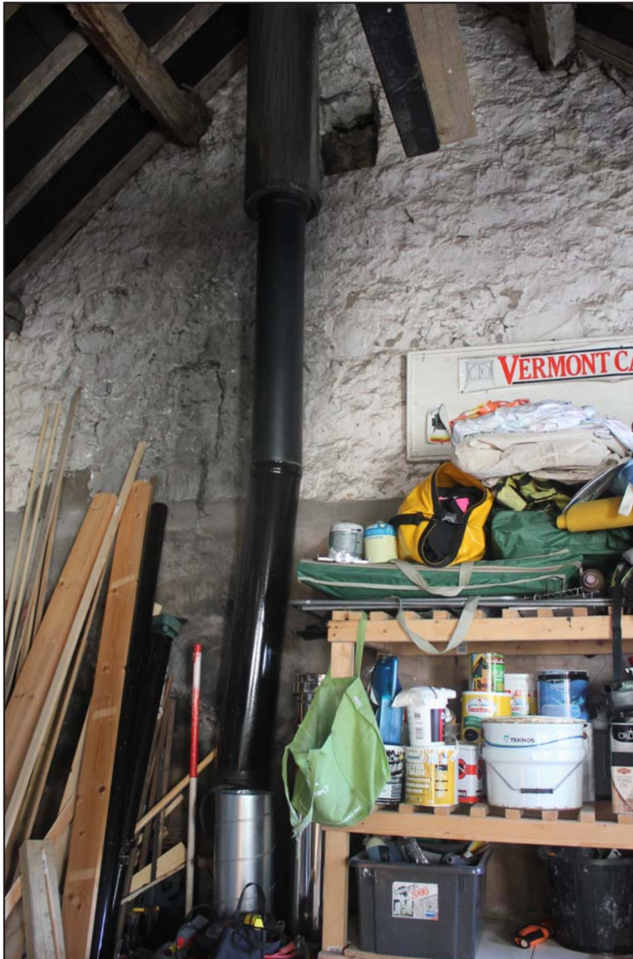
Plate 18: Plas Yn Llan, Cilcain, Flintshire. Internal shot - eastern elevation - from the southwest - 1m scale
