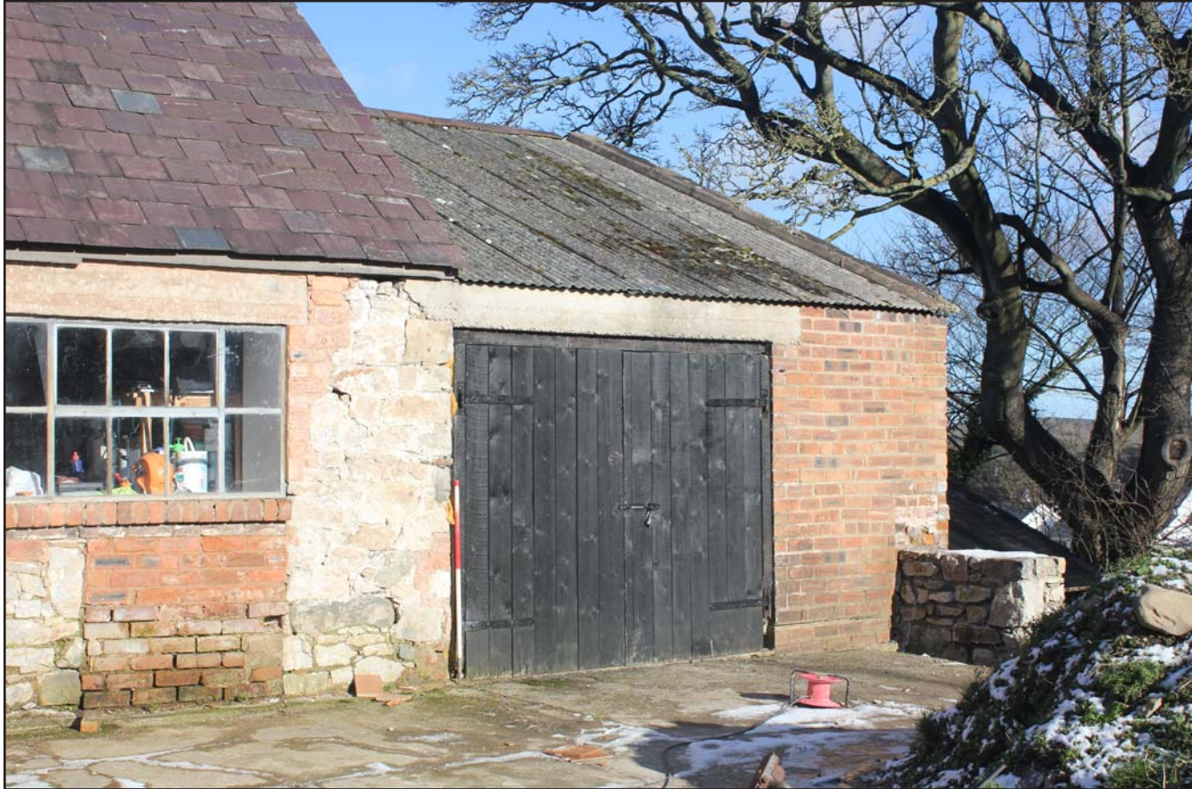
Plate 03: Plas Yn Llan, Cilcain, Flintshire. External shot - right hand end of southern elevation (Stores) - From the south - 1m scale
