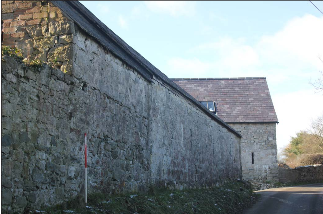
Plate 06: Plas Yn Llan, Cilcain, Flintshire. External shot - left hand end of northern elevation - From the northeast - 1m scale
