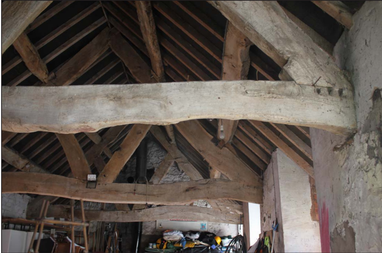
Plate 23: Plas Yn Llan, Cilcain, Flintshire. Internal shot - Queen truss timber frame context shot from below (southern) - from the west - no scale
