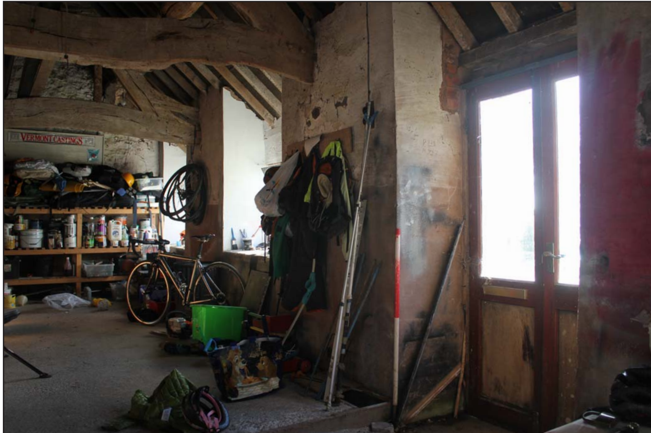
Plate 16: Plas Yn Llan, Cilcain, Flintshire. Internal shot - oblique shot of southern elevation - from the northwest - 1m scale
