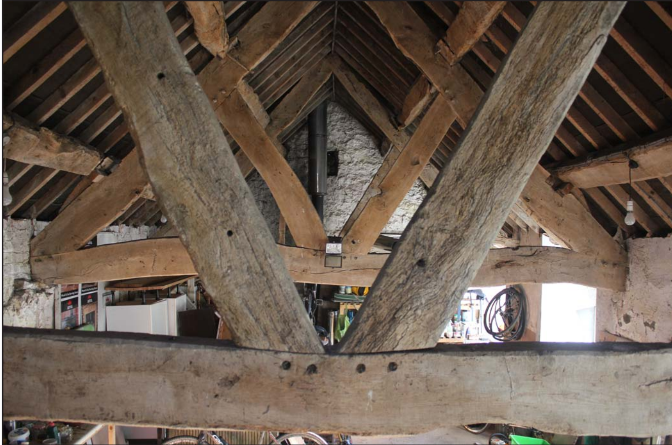
Plate 22: Plas Yn Llan, Cilcain, Flintshire. Internal shot - Queen truss timber frame context shot from above (central) - from the west - no scale
