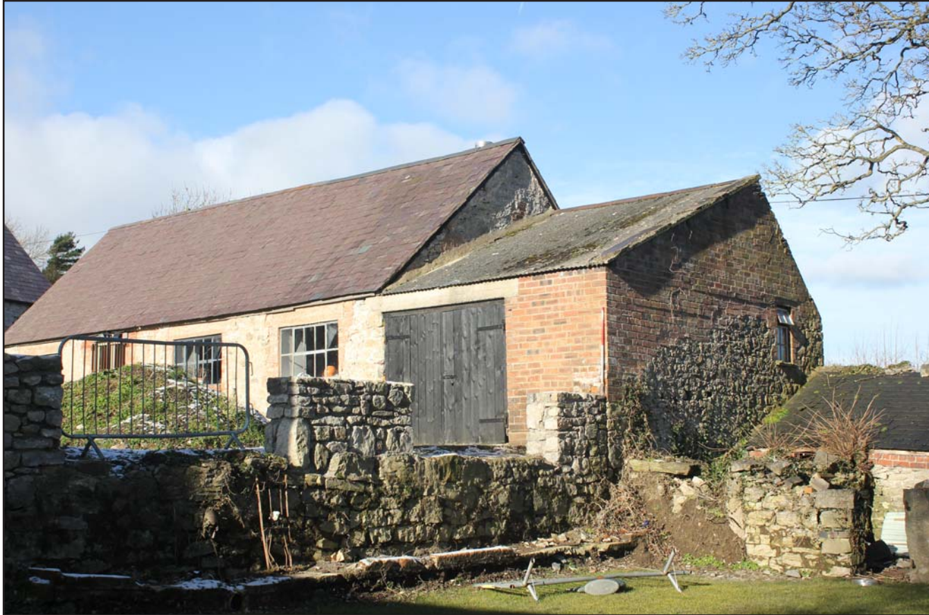
Plate 04: Plas Yn Llan, Cilcain, Flintshire. External shot - oblique shot showing southern & eastern elevations - From the southeast - 1m scale
