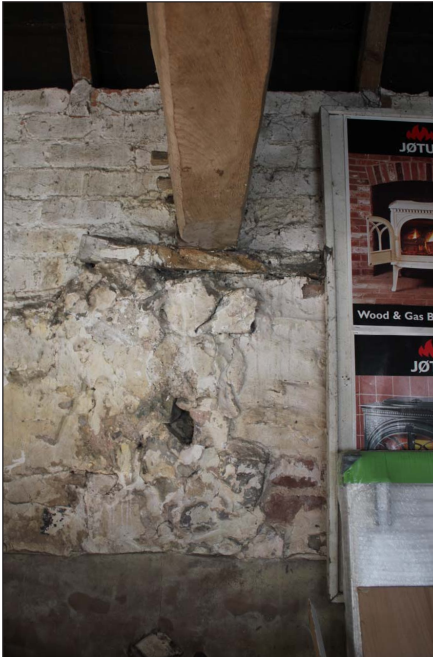
Plate 25: Plas Yn Llan, Cilcain, Flintshire. Internal shot - another example of corble table on northern elevation - from the south - no scale
