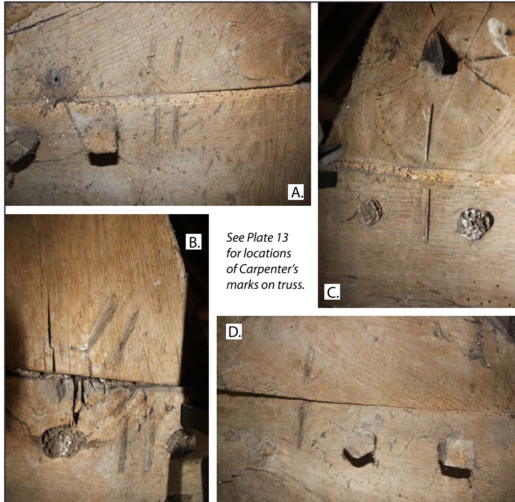
Plate 12: Plas Yn Llan, Cilcain, Flintshire. Carpenter's marks on the central timber truss inside the former workshop - From the west - no scale
