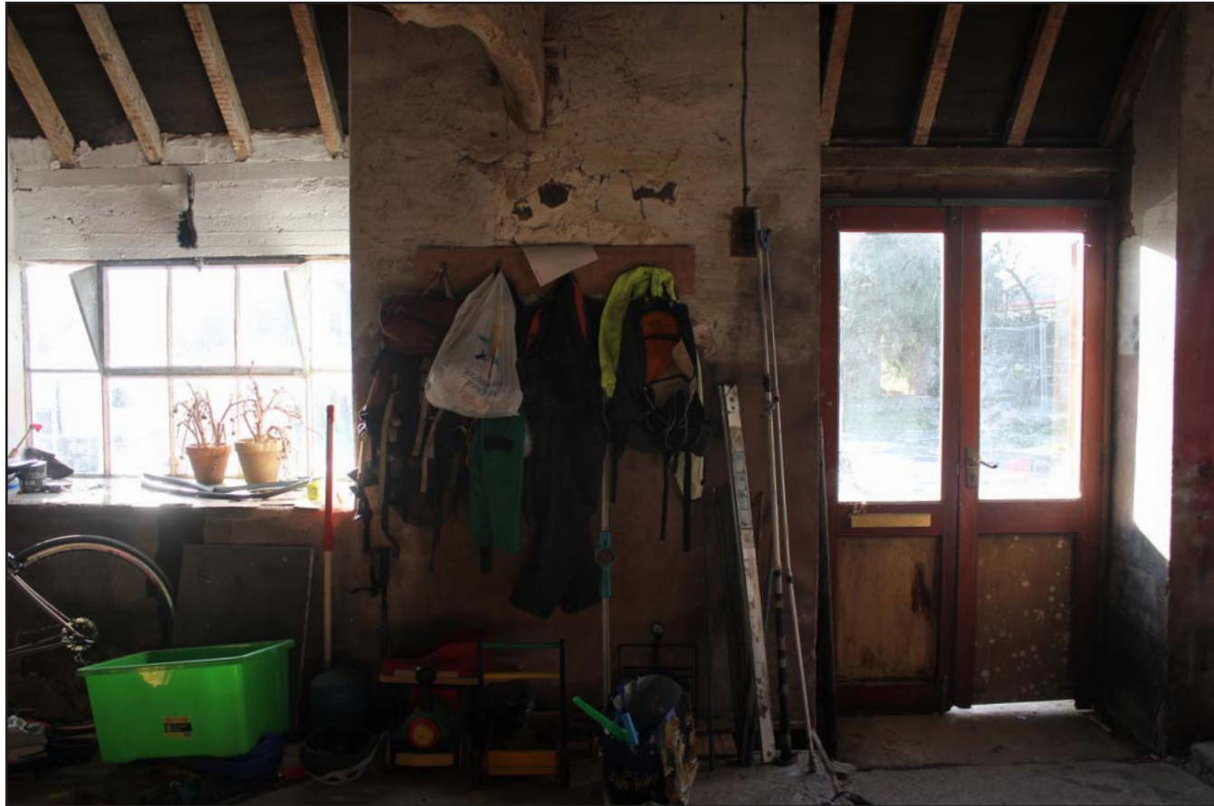
Plate 17: Plas Yn Llan, Cilcain, Flintshire. Internal shot - example section of southern elevation - from the north - 1m scale
