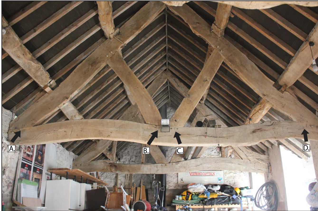
Plate 13: Plas Yn Llan, Cilcain, Flintshire. Internal shot - west facing side of central timber truss inside the former workshop, showing locations of the Carpenter's marks - From the west- no scale
