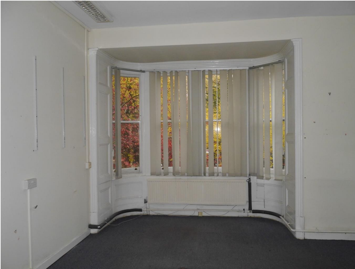
Plate 22: F1 [above] curved bay with original windows, cornice detail, architrave and panelling.
