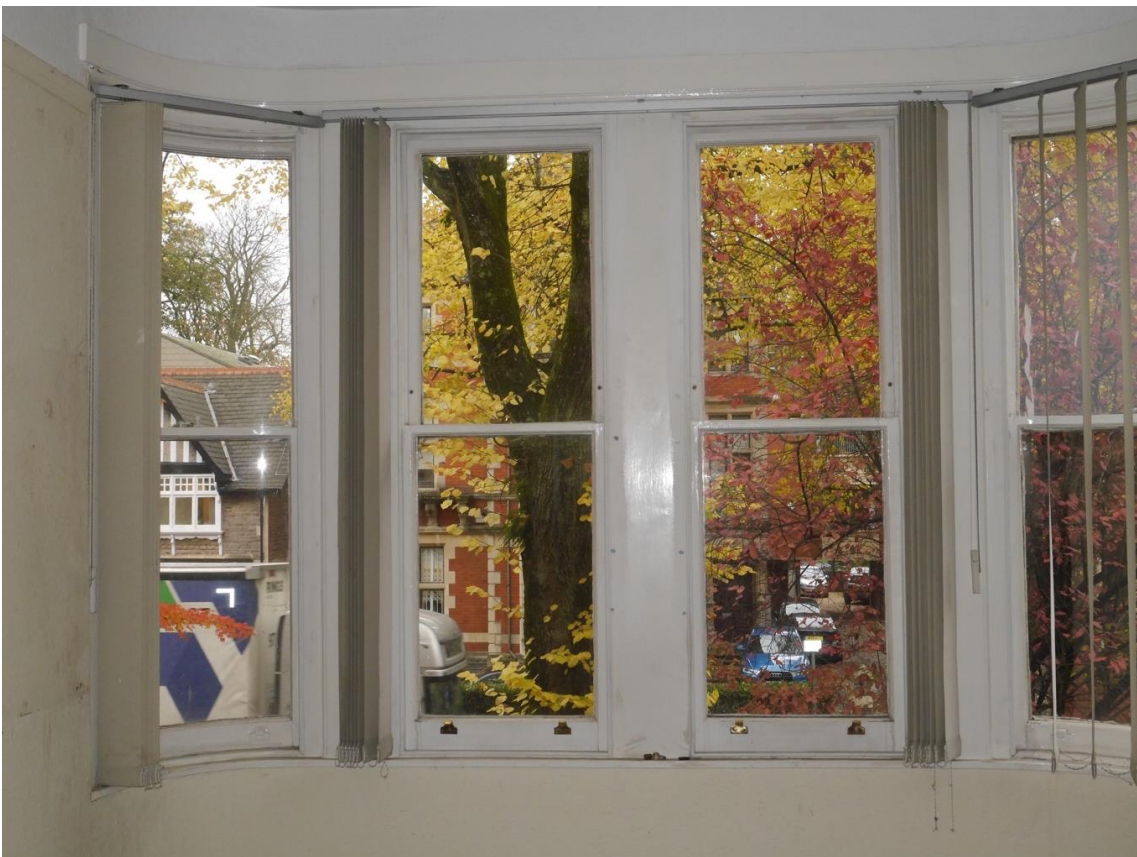
Plate 23: F3 [above] curved bay with original windows.
