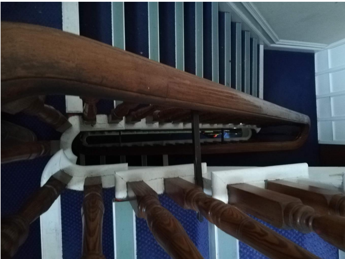
Plate 27: Open stair with continuous hand rail
