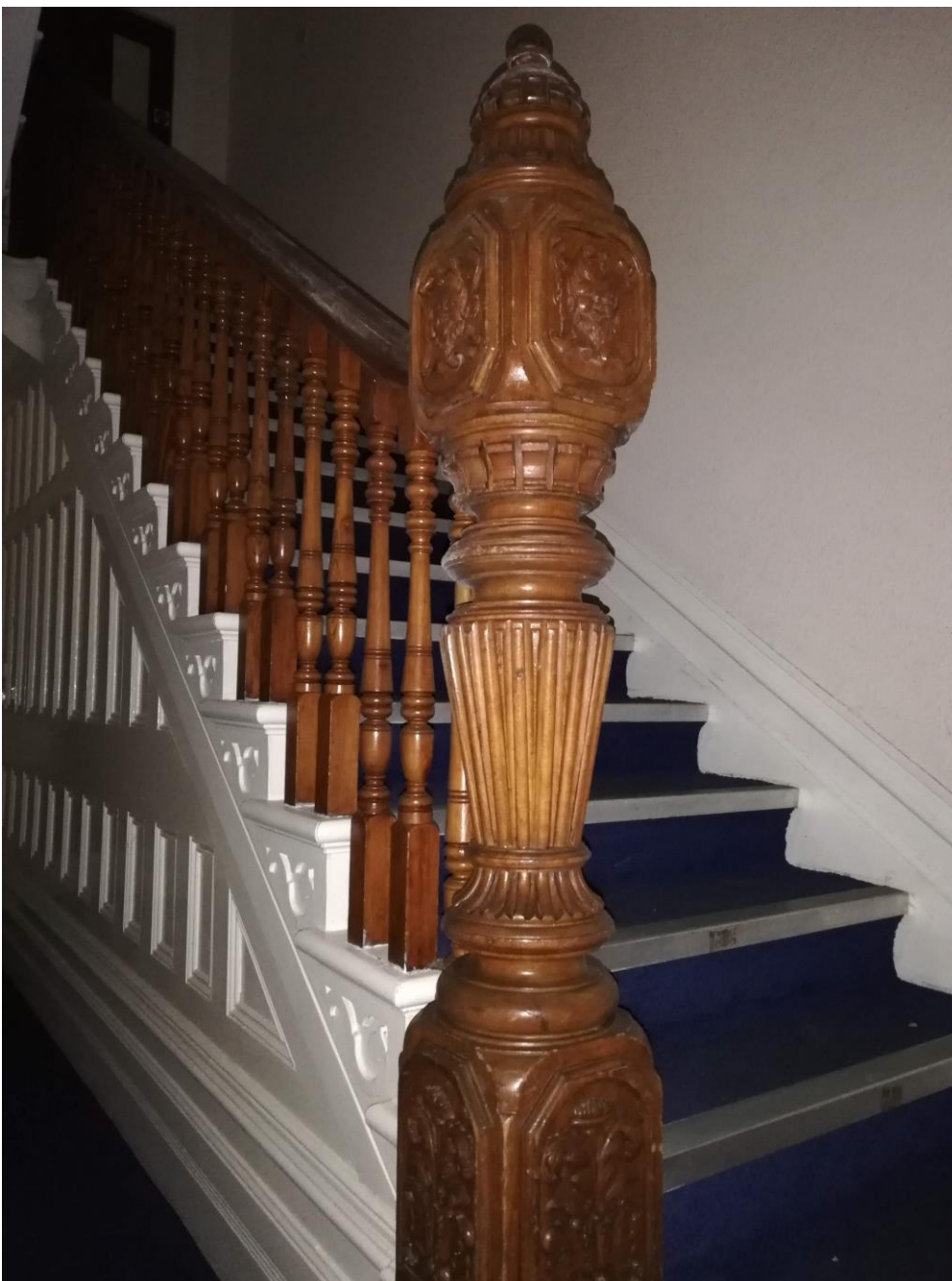
Plate 24: base of stair showing substantial newel post, open risers, panelling and detailed treads.
