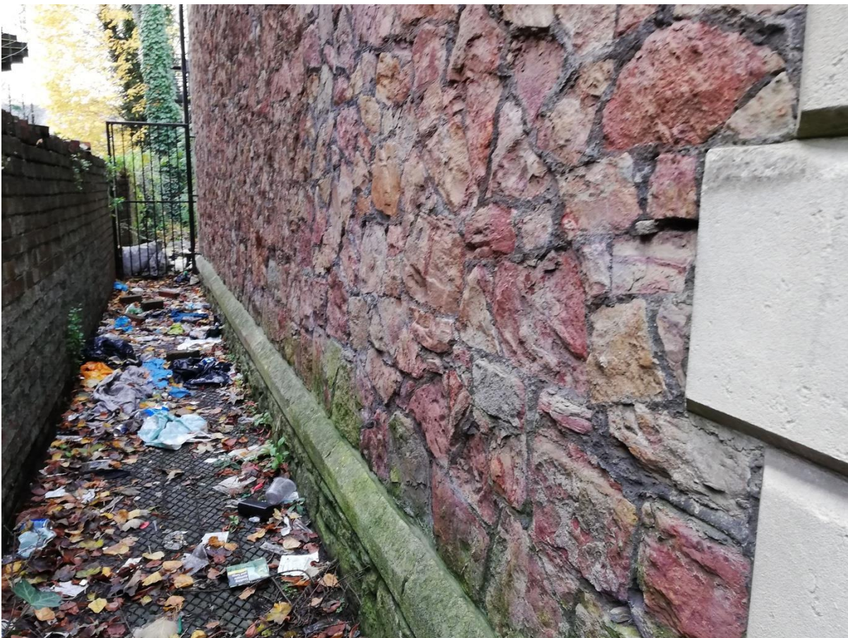
Plates 9 & 10: Detail of stonework to S elevation 29 Cathedral Road
