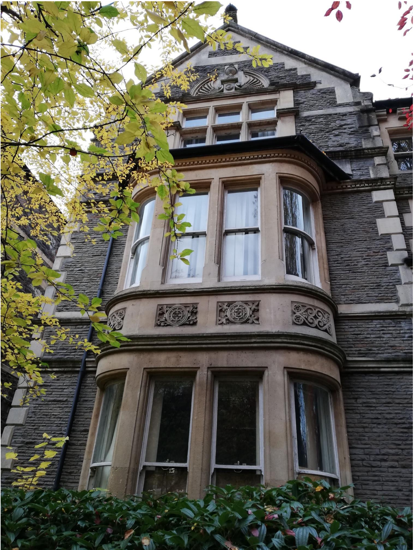
Plate 1: 27 Cathedral Road: two Storey Bays with curved glass and frieze
