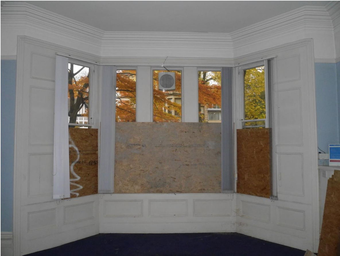
Plate 20: G4 Deep cornice, panelling and skirting to No. 29 Cathedral Road.
