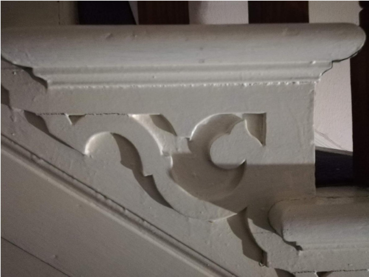
Plate 26: Open string with bracket detail
