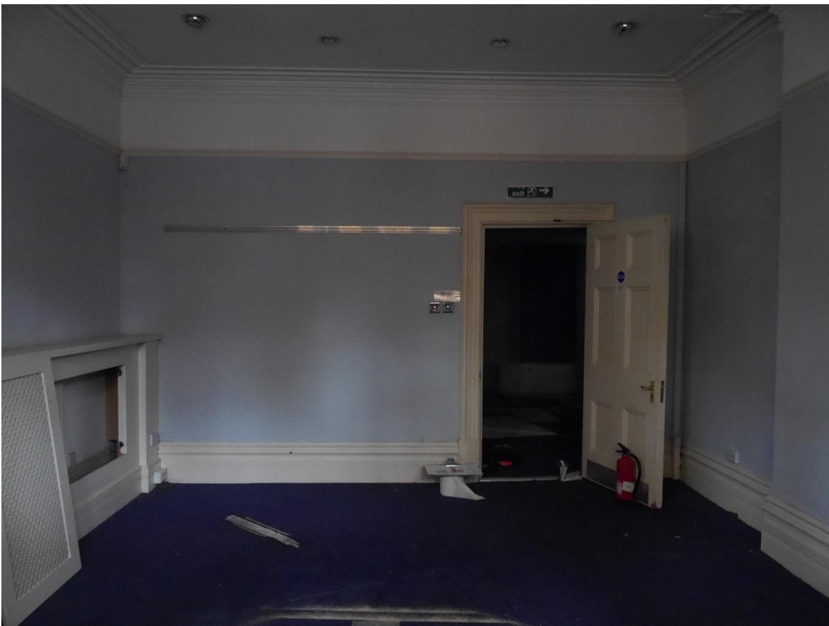
Plate 21: G4 Deep cornice, panelling and skirting to No. 29 Cathedral Road
