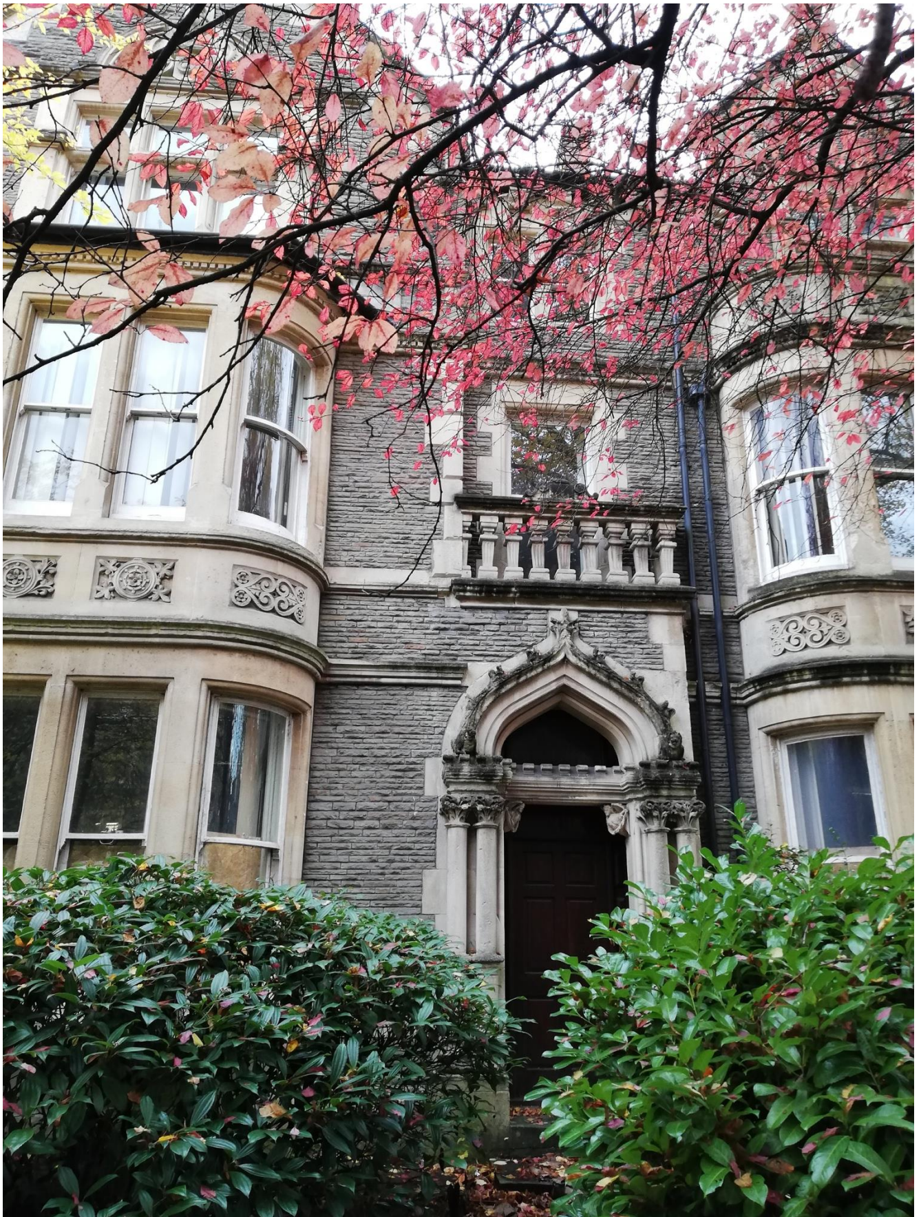
Plate 2: 27 Cathedral Road: original entrance including balcony and ogee arch
