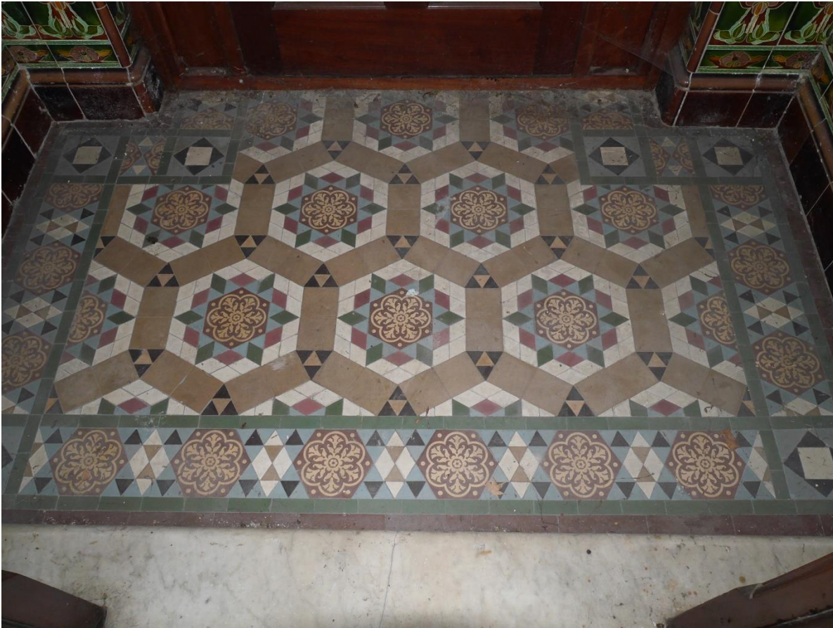
Plate 15: Original Mosaic Tiles to No. 27 Entrance Lobby
