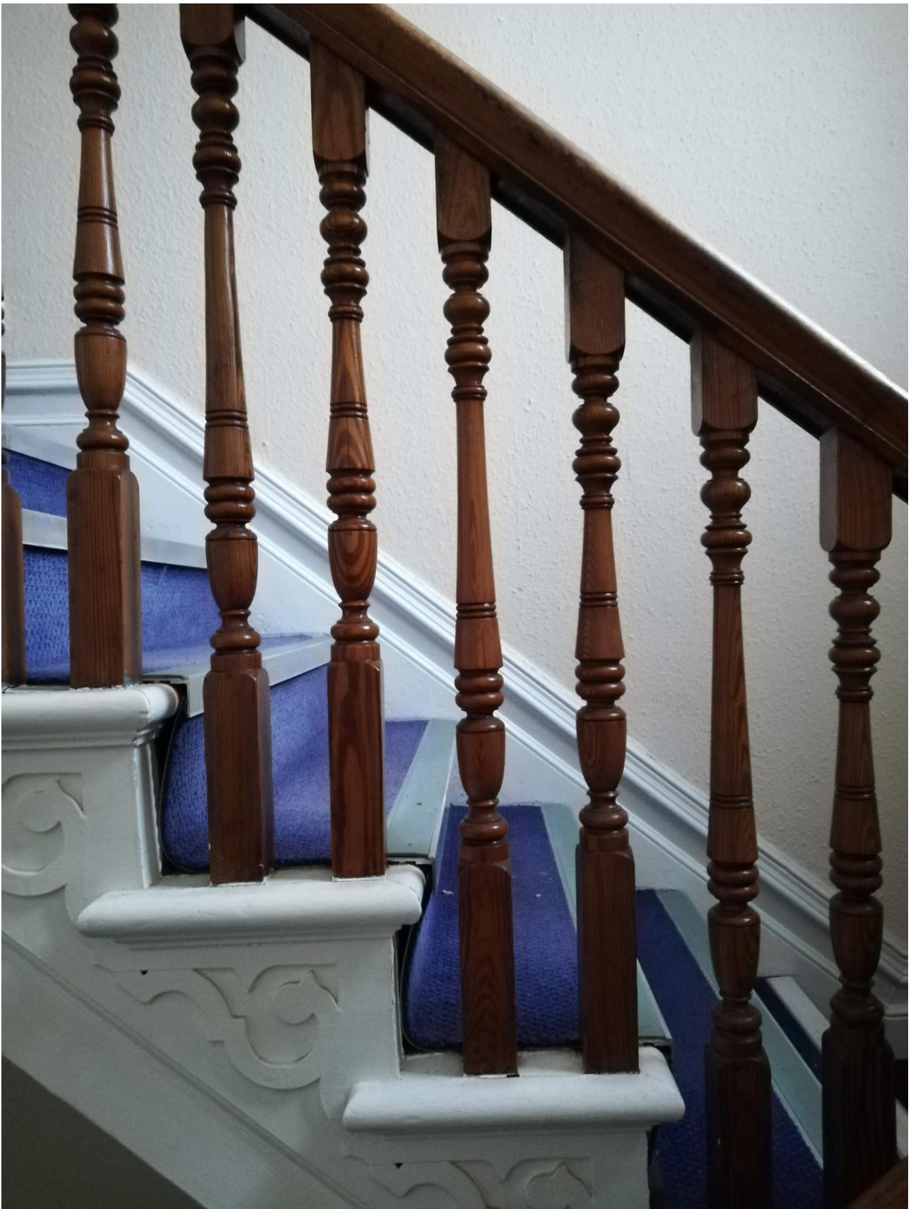
Plate 25: decorative open treads and alternating ballusters
