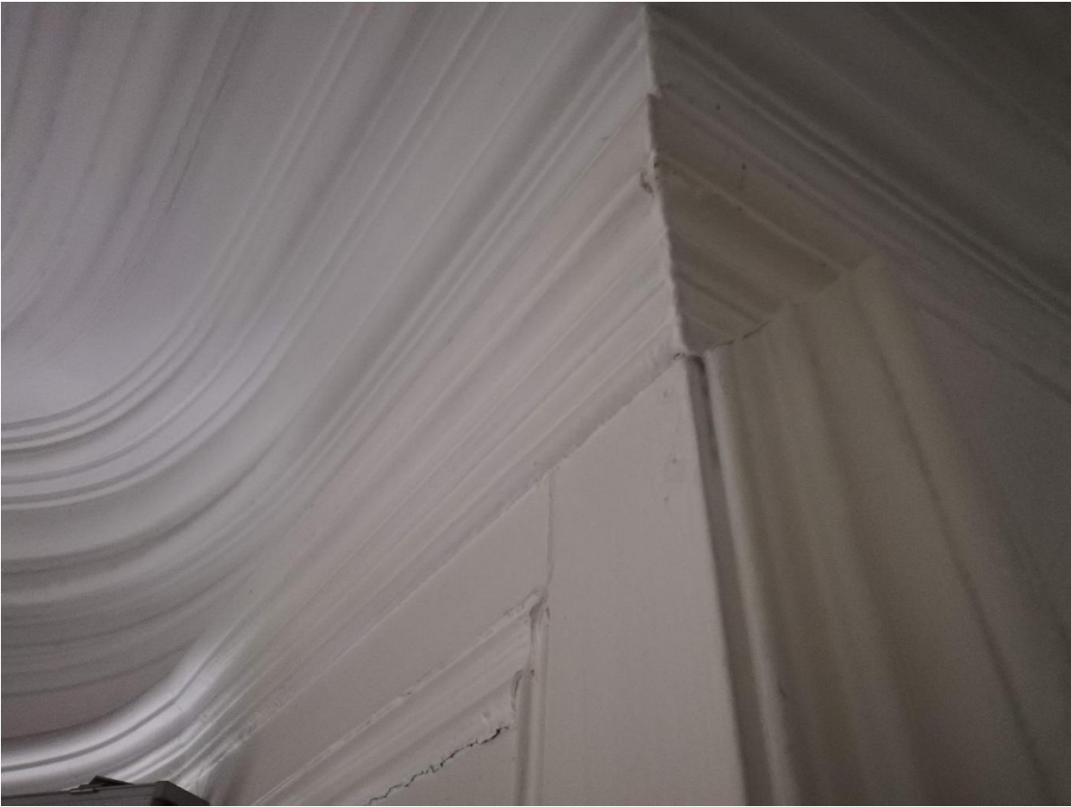
Plate 19: G3 Detail of curved cornice wrapping around bay.
