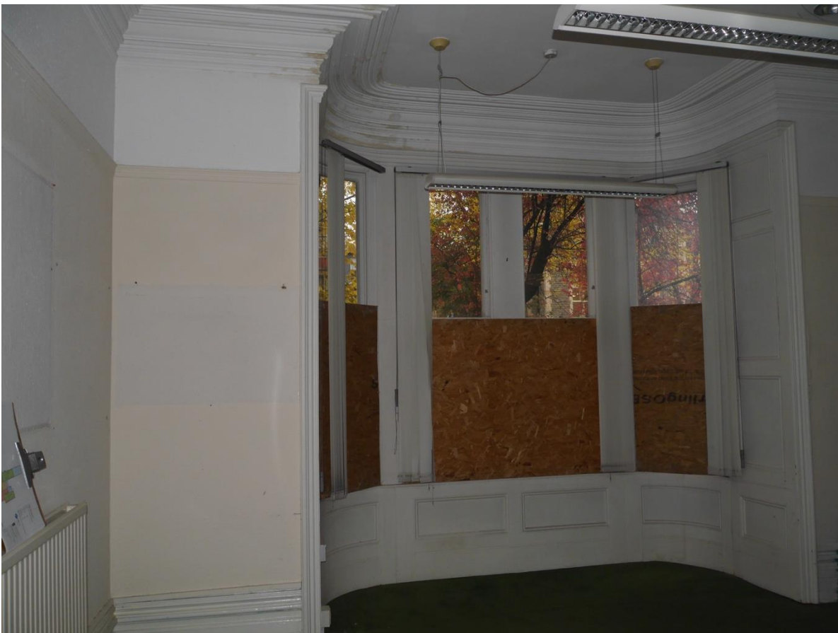
Plate 16: G3 deep curved cornice and skirting [see Appendix D Drawing 1] for dimensions
