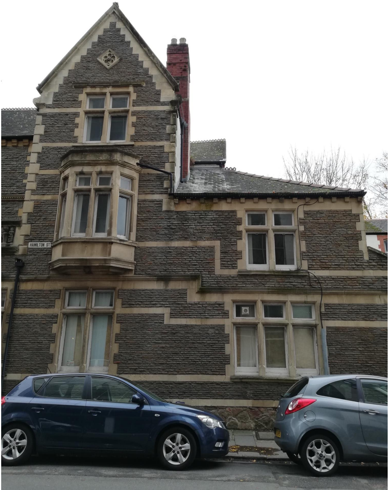
Plate 7: Hamilton Street: variety of stone detailing used including rubble plinth, ashlar coursing and window detail and small pennant blockwork
