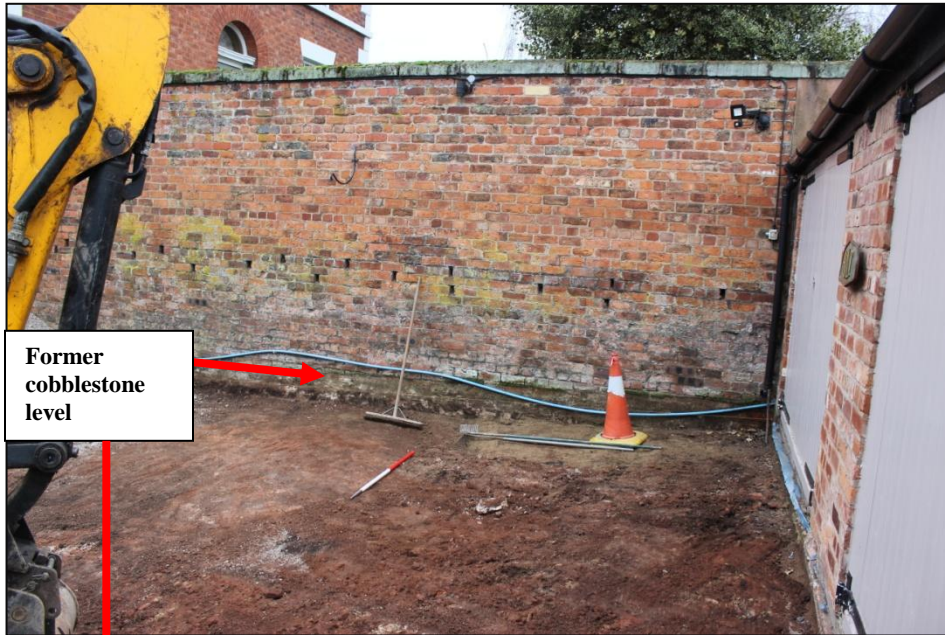
Plate 2: Southwest corner of the courtyard, excavated to 300mm below former finished level of the cobbles. 1m scale shows the bedrock outcrop
