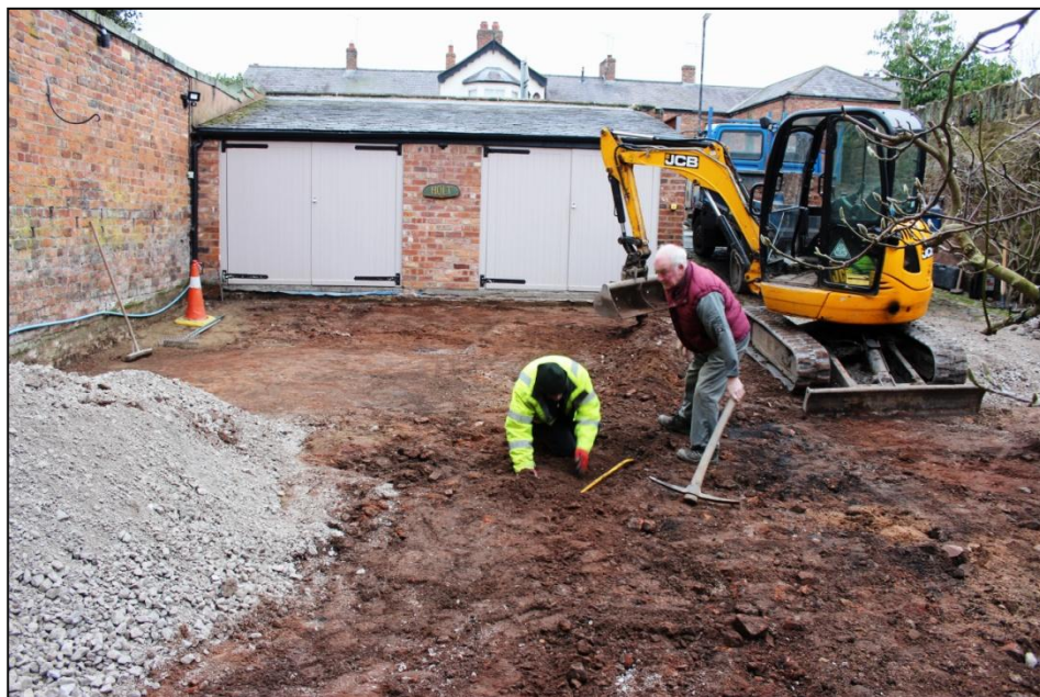
Plate 4: Investigating the gas main, view from the west
