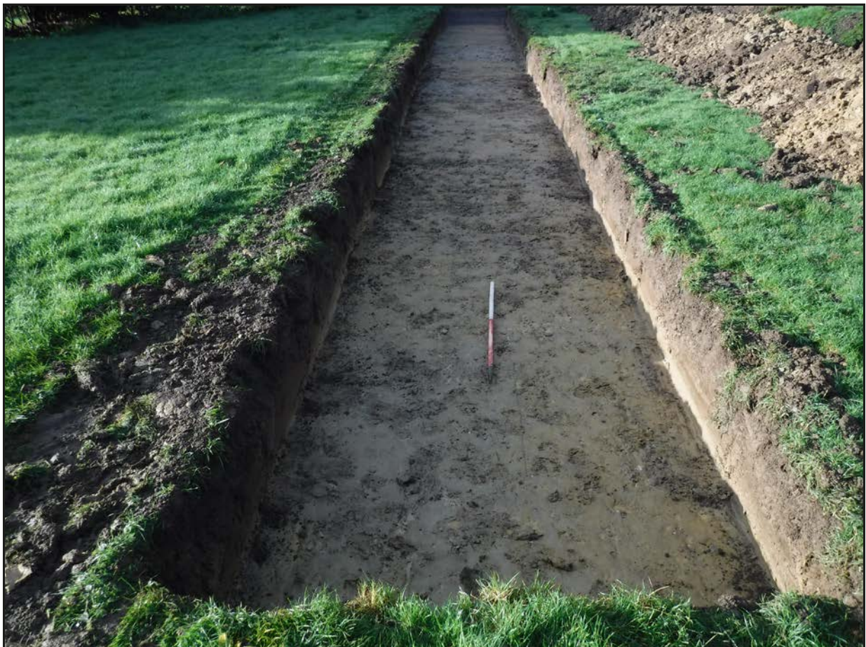
Plate 8 : Trench 8 looking south-west.
