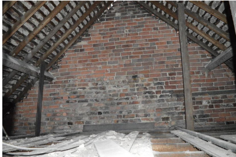
Fig. 8 Internal view of southern gable, showing the original roof line. CPAT image 4701-0042
