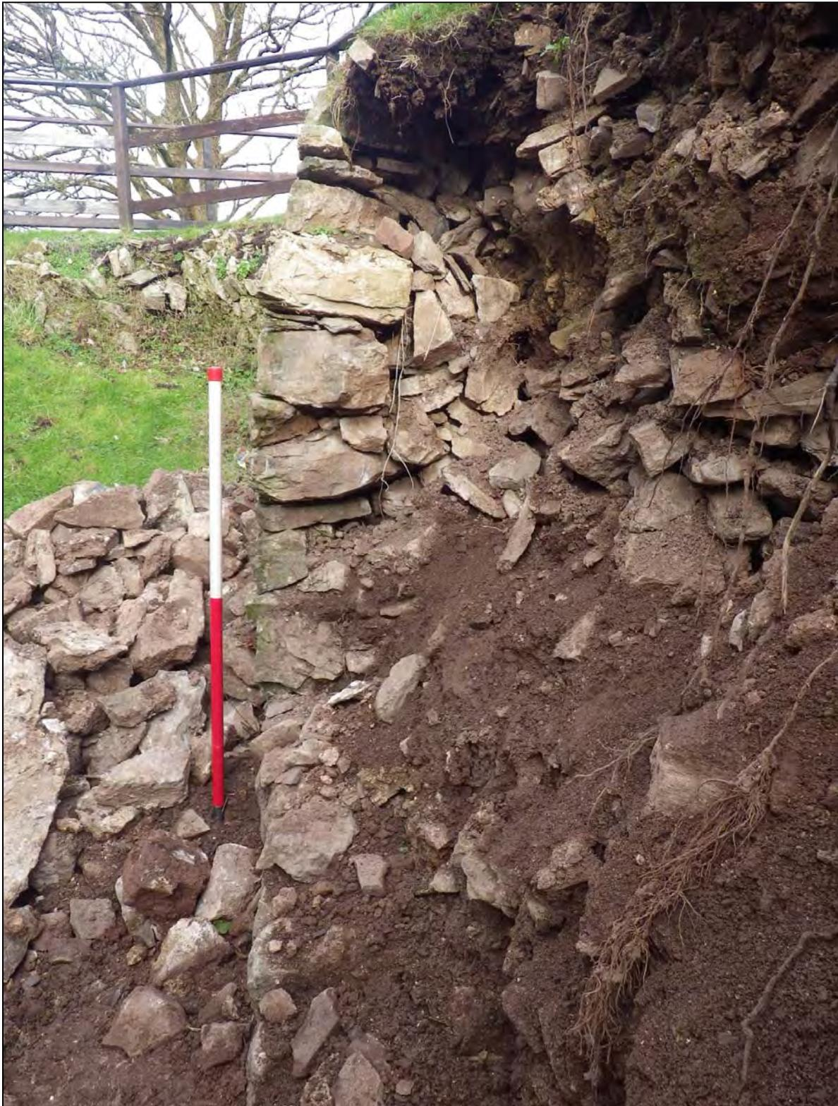
*Plate 8: MBC2015\_108, the northwestern part of the collapsed section of revetment after cleaning. This section did not need a new foundation trench as the lower part of the revetment was still in situ, looking northwest.*
