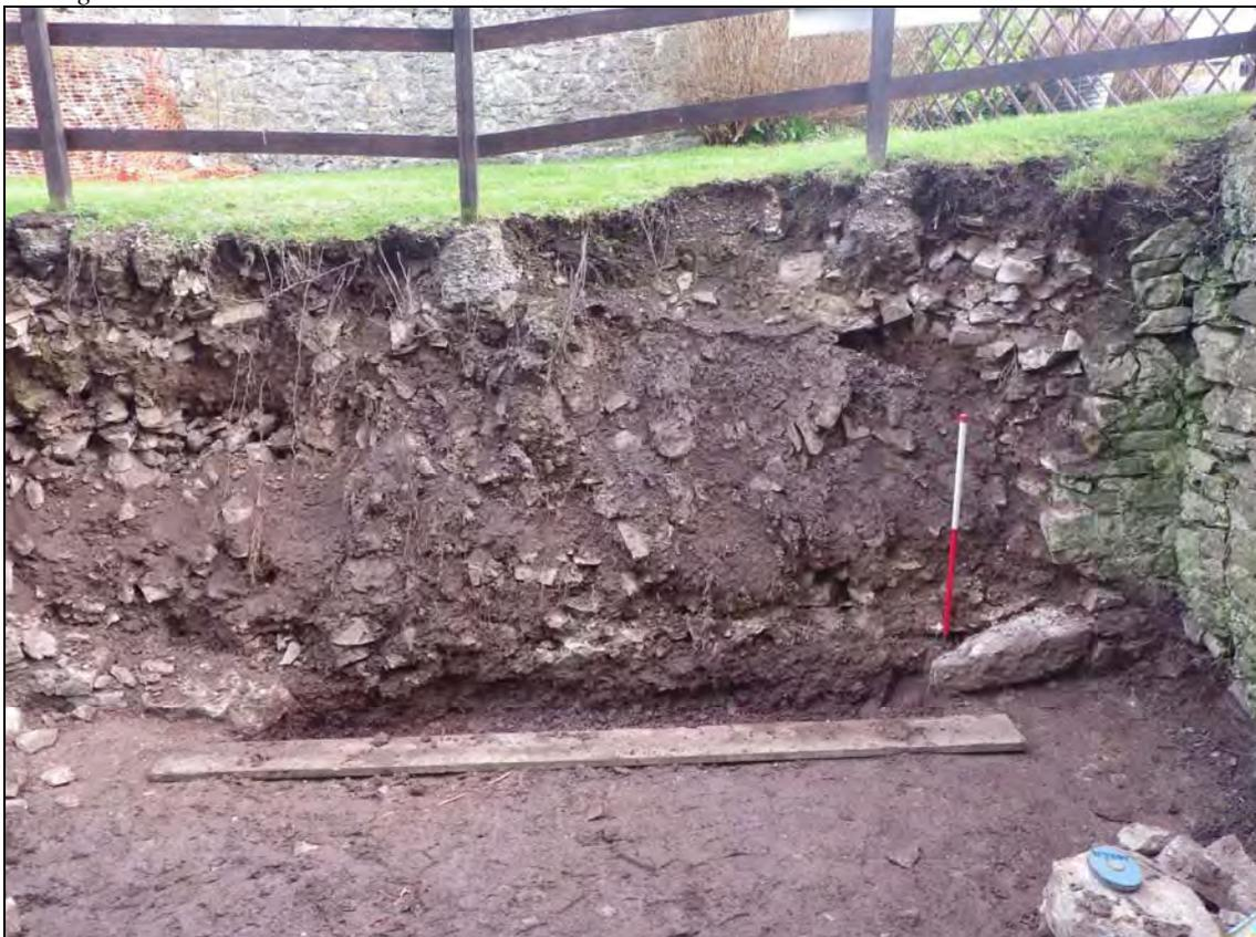
*Plate 4: MBC2015\_104, the section of collapsed revetment after cleaning and foundation trench excavated, looking northeast.*
