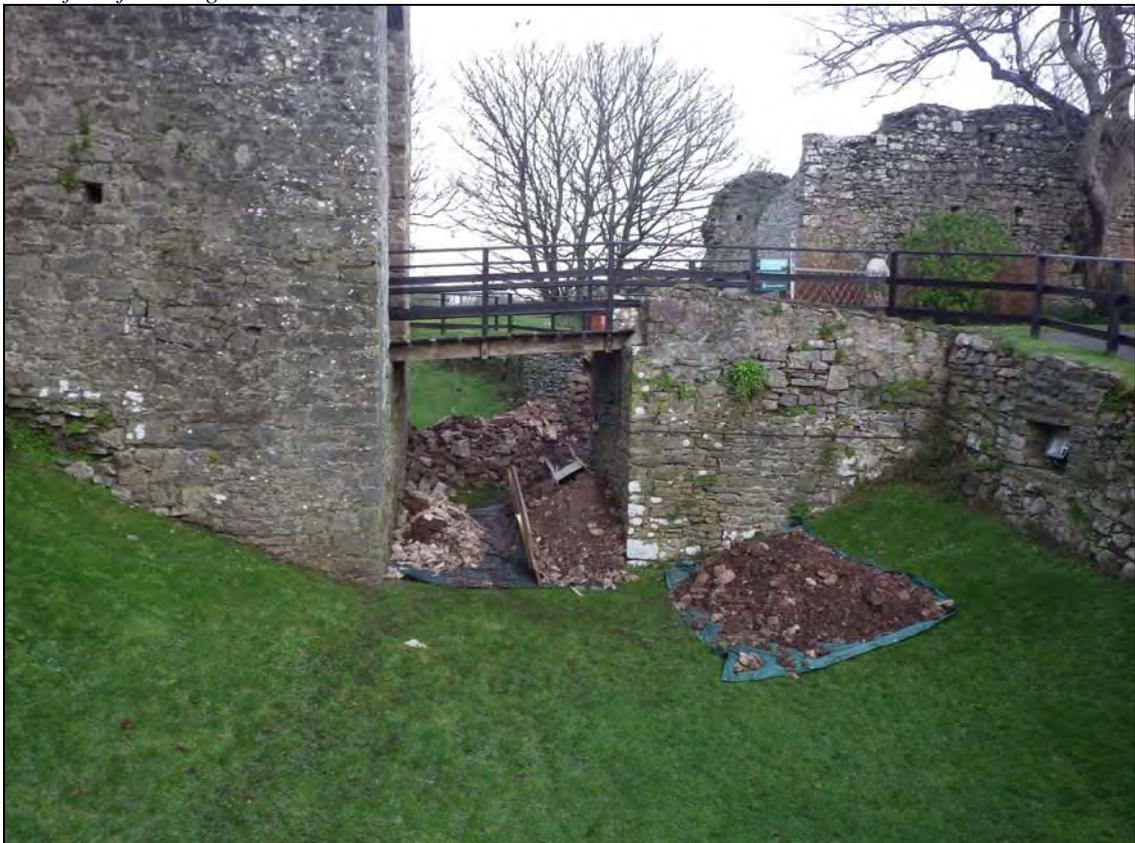
*Plate 2: MBC2015\_102, looking north in the ditch to the east of the castle, south of the footbridge crossing into the gatehouse. Collapsed revetment wall to the north of the footbridge.*
