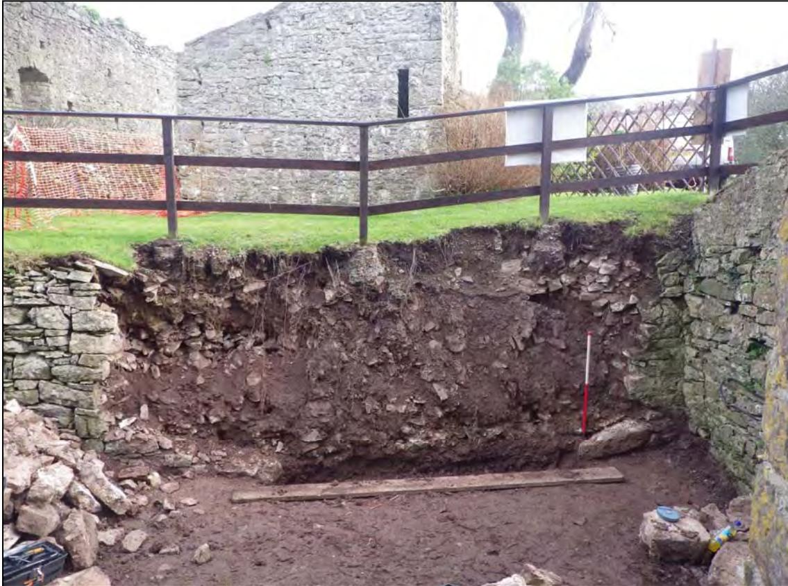
*Plate 3: MBC2015\_103, the area of collapsed revetment after cleaning and foundation trench excavated, looking northeast.*
