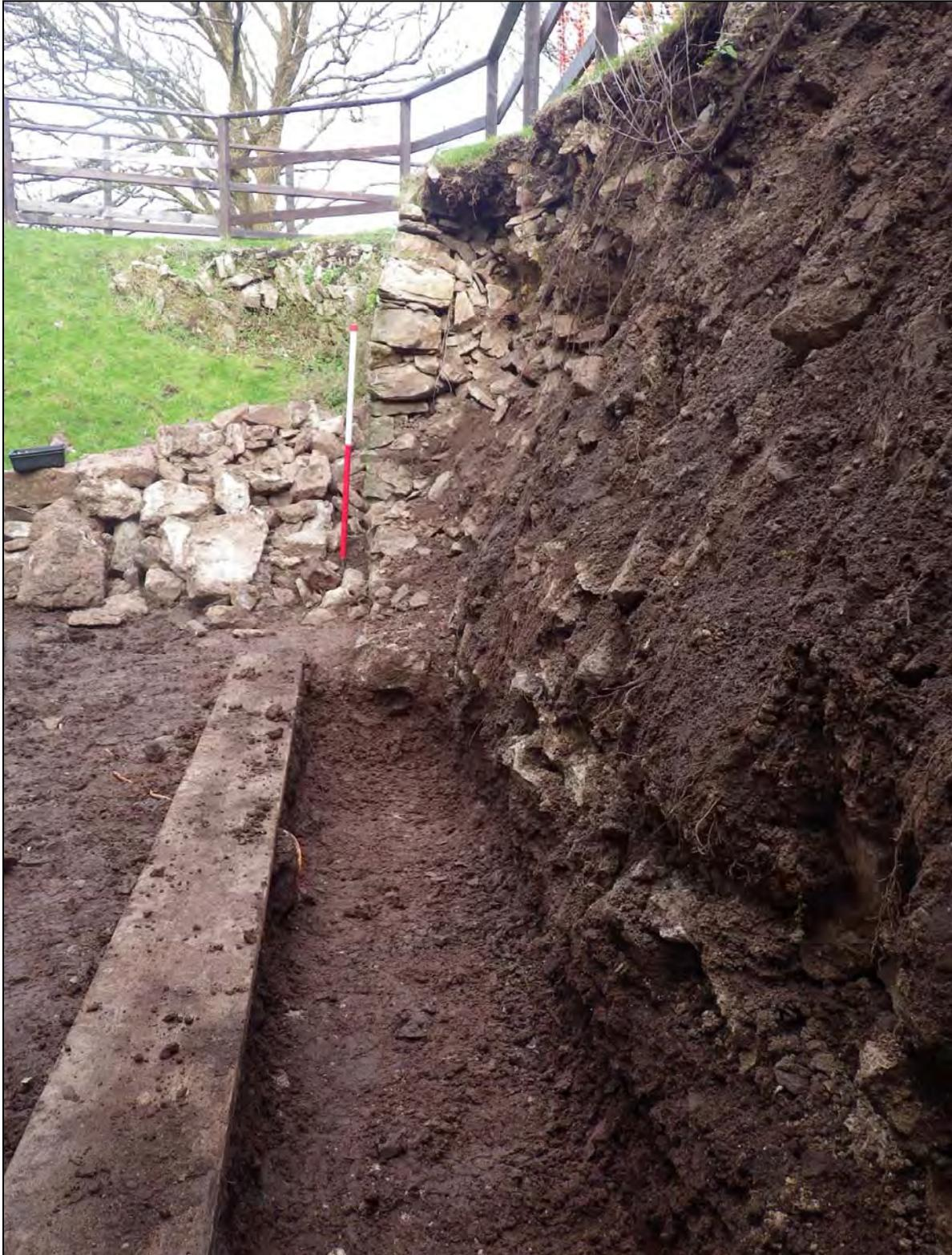
*Plate 7: MBC2015\_107, the collapsed revetment after cleaning and foundation trench excavated, looking northwest.*
