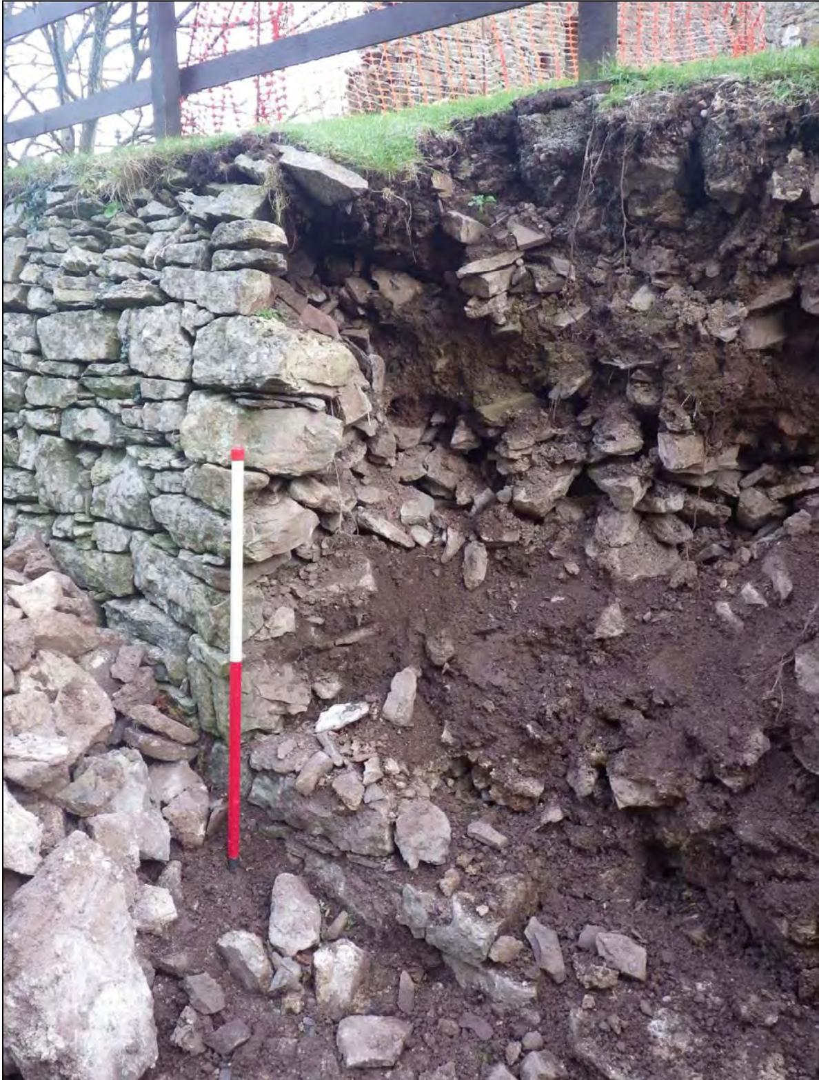
*Plate 6: MBC2015\_106, the northwestern end of the collapsed section of revetment wall, looking north northeast.*
