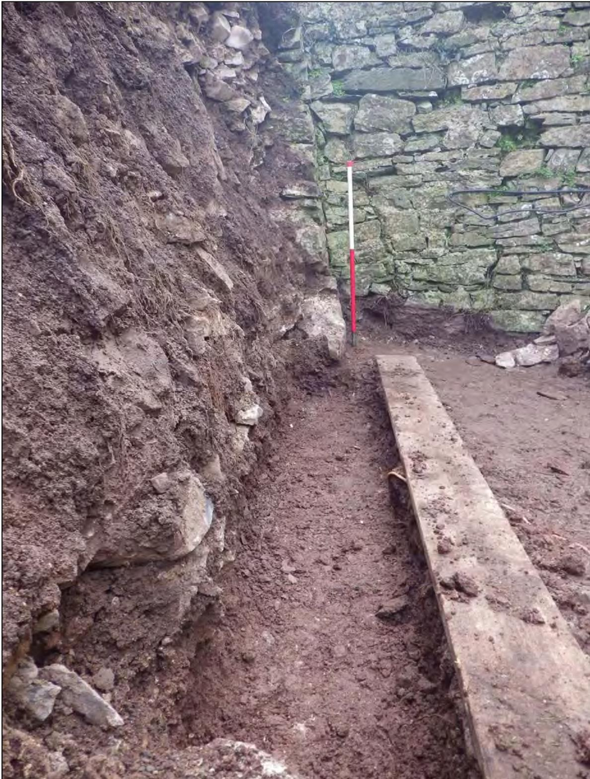
*Plate 5: MBC2015\_105, the collapsed revetment after cleaning and foundation trench excavated, looking southeast.*
