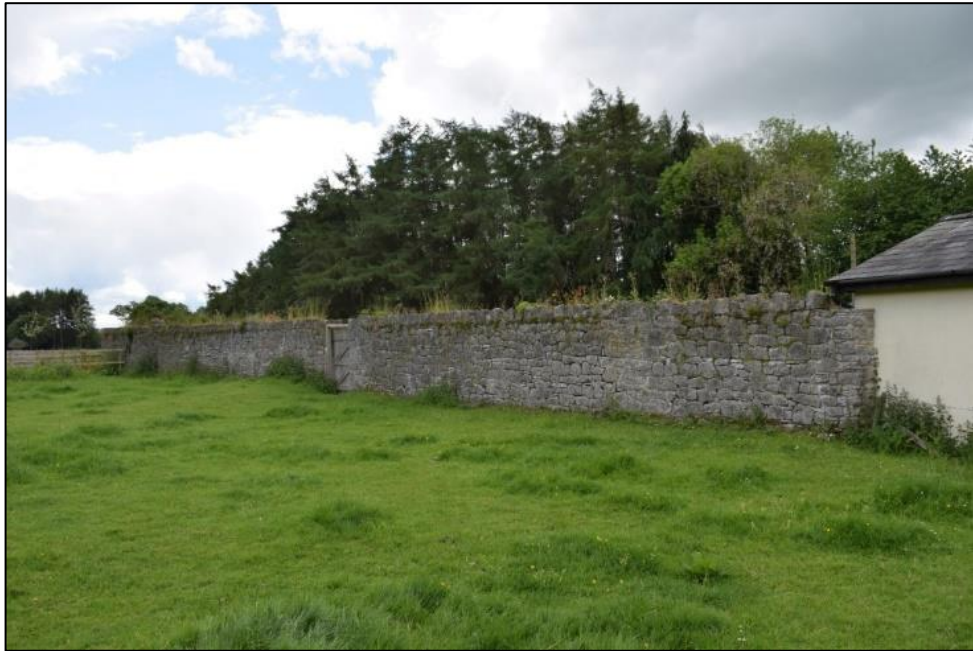
Fig. 7: The eastern side of the former walled garden. Photo CPAT 4653-0057
