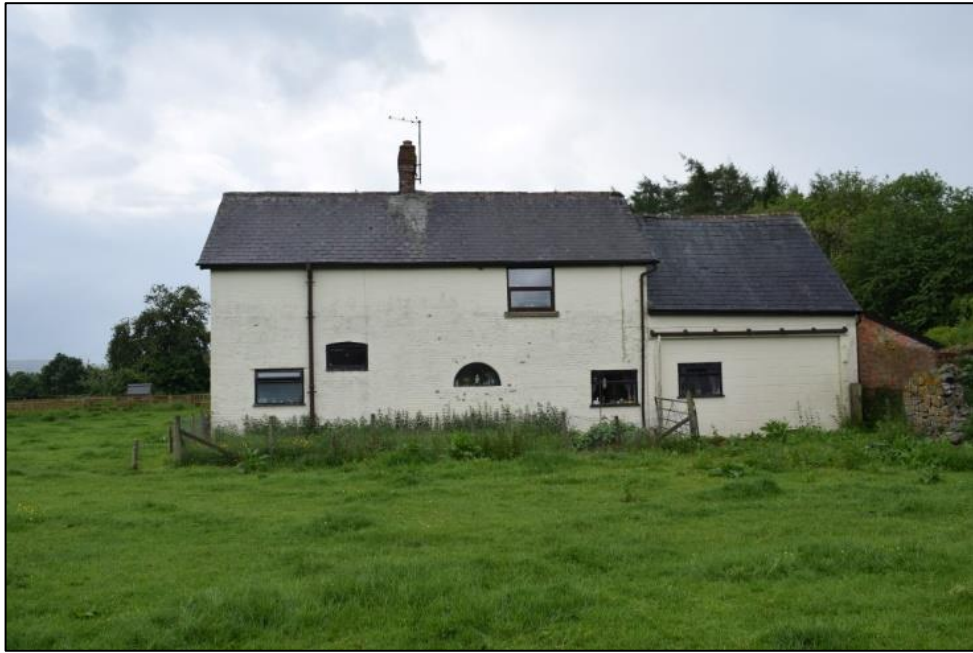
Fig. 11: The north side of the cottage, with slate roof and random windows. Note the lower section to the right which probably indicates the original roof line and pitch. Photo CPAT 4653-0002
