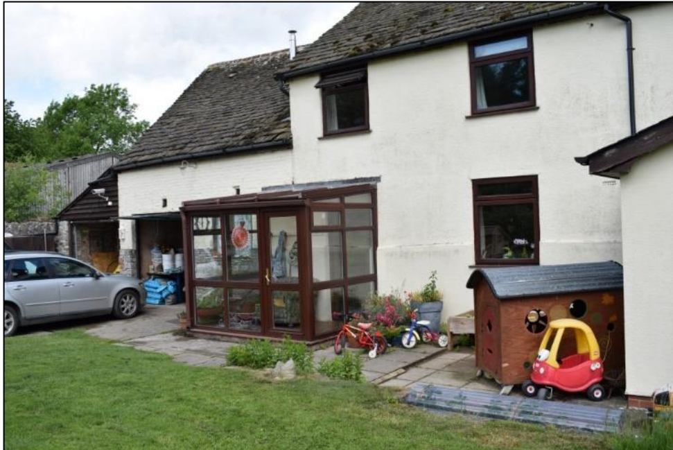
Fig. 5: The stone wall of the kitchen garden predating the cottage, seen as a step in the wall halfway up the conservatory and between the two garages to its left. Photo CPAT 4653-0042
