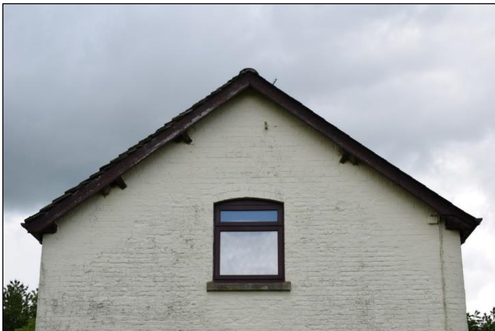
Fig. 8: The eastern gable of the cottage showing the former roof level. Photo CPAT 4653-0056
