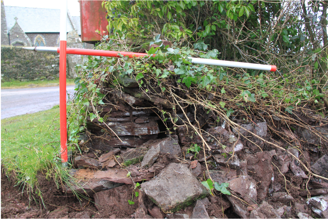
Plate 5 - AD003-D1-005 - Partial removal of stone dry wall to widen site entrance.
