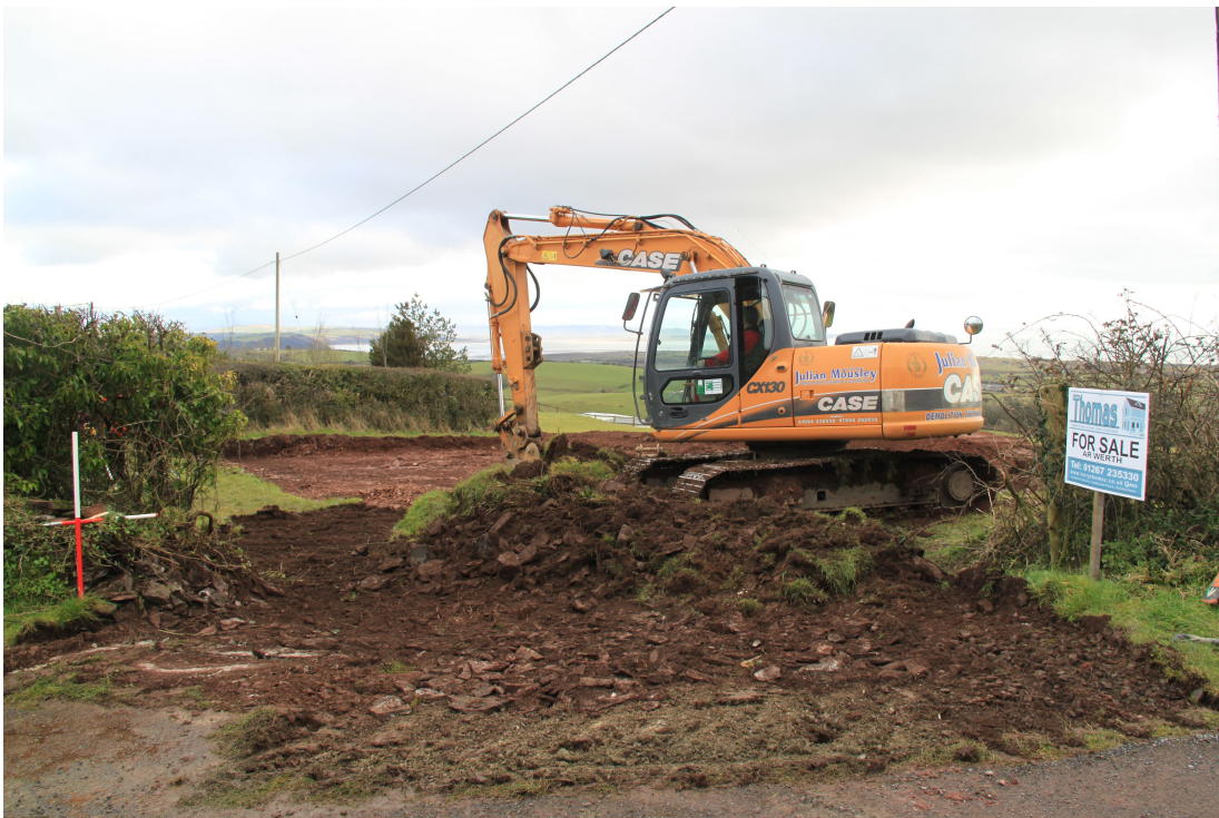
Plate 6 - AD003-D1-006 - Widening and landscaping to create entrance to site.
