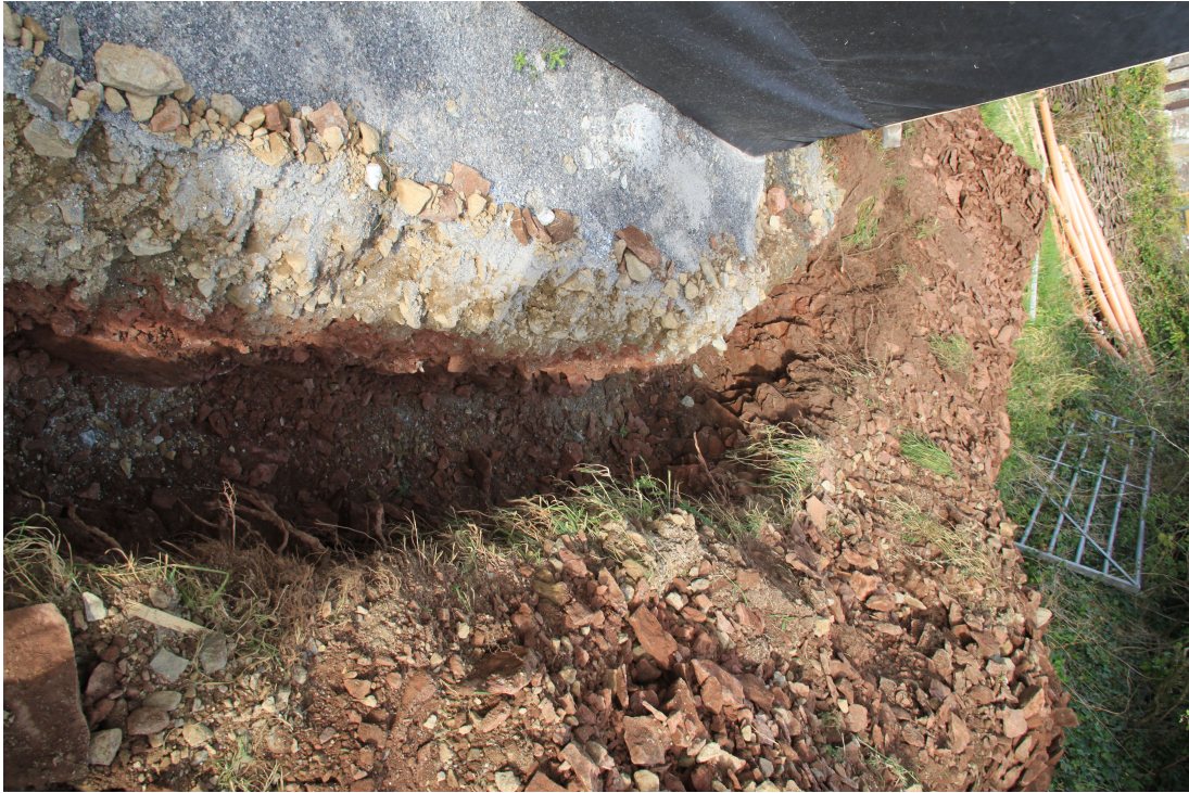
Plate 11 - AD003-D2-011 - Service trench turning south, along east edge of plot.
