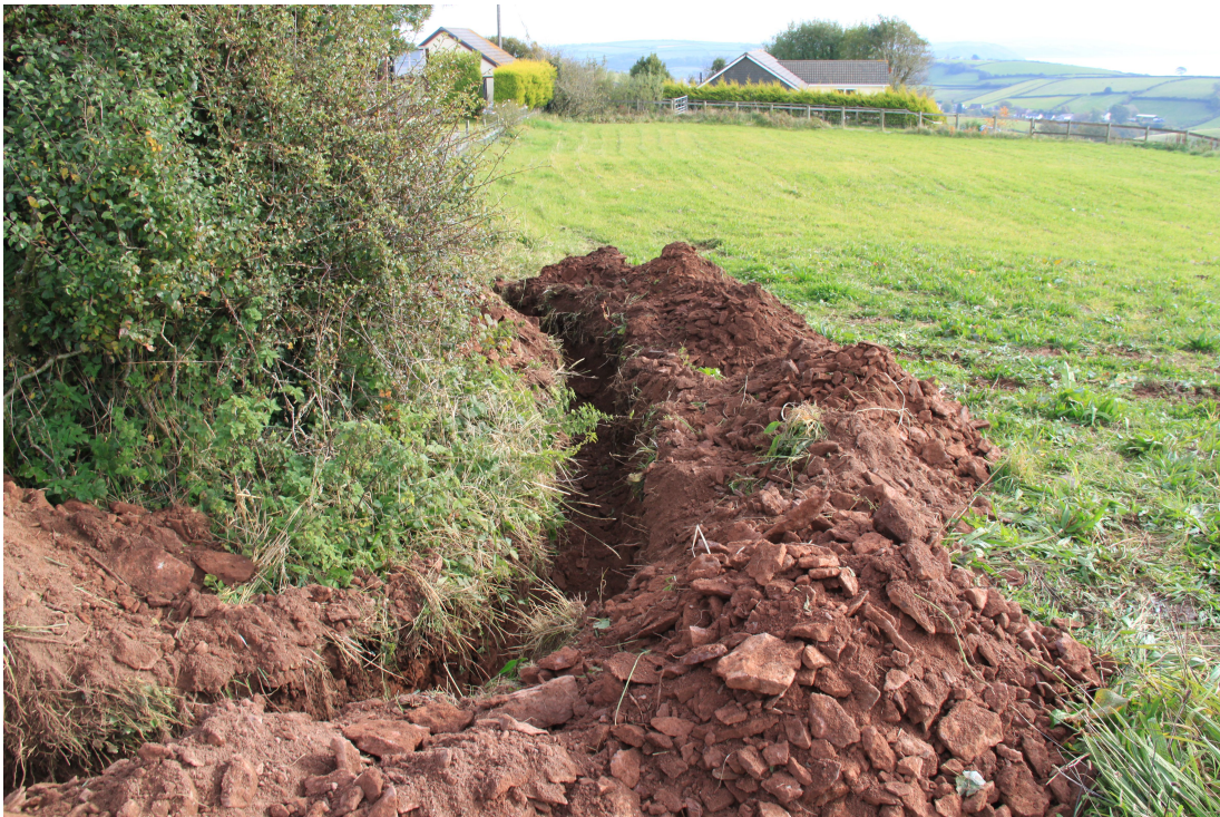
Plate 14 - AD003-D2-014 - Service trench turning east, along north edge of plot.
