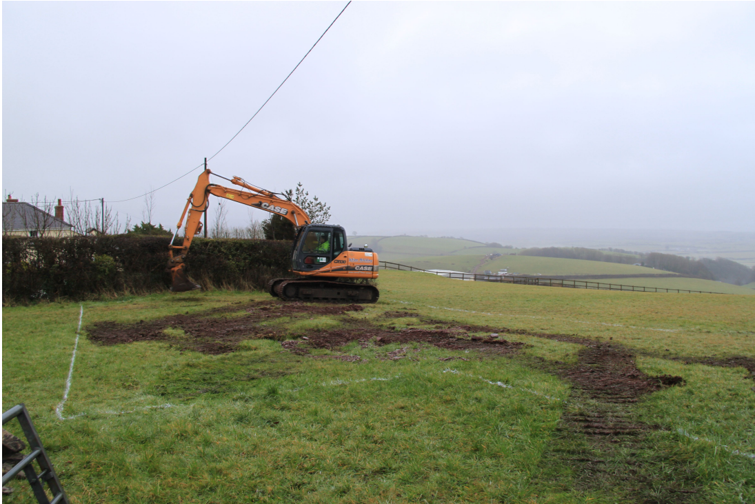
Plate 1 - AD003-D1-001 - Site on arrival, view toward the south-east.
