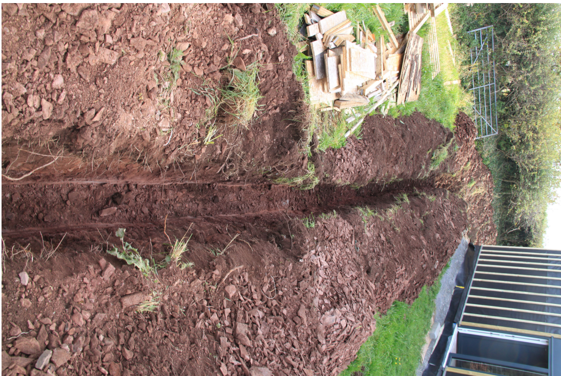
Plate 8 - AD003-D2-008 - Service trench across north of site.
