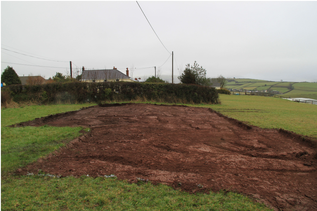
Plate 2 - AD003-D1-002 - After humus and topsoil removal, view toward the east.
