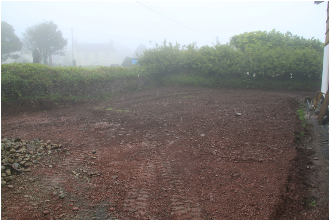
Plate 19 - AD003-D3-019 - Completed levelling and landscaping at front of house.
