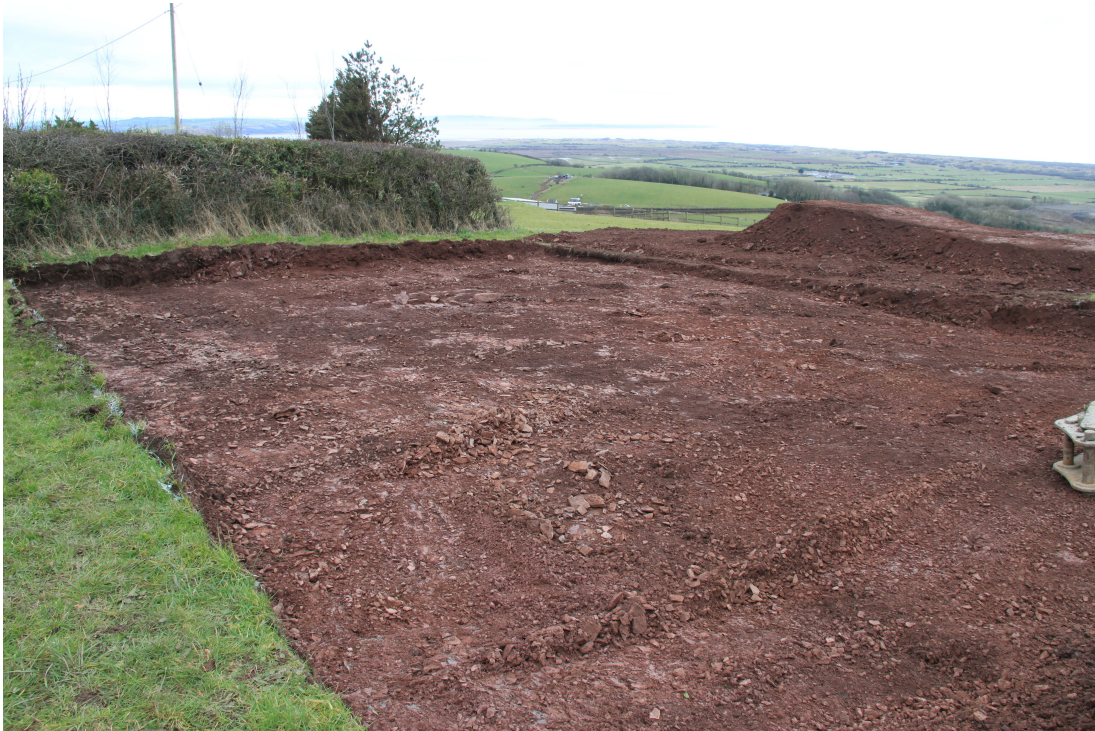
Plate 7 - AD003-D1-007 - Completion of excavations for foundation raft.
