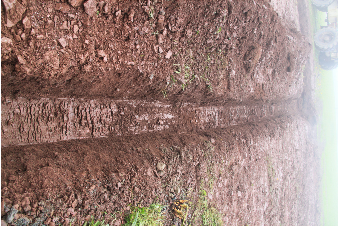
Plate 17 - AD003-D3-017 - Service trench to septic tank, running south.
