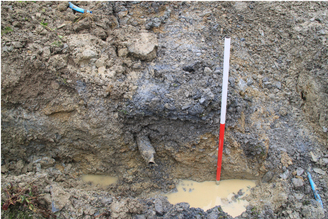
Plate 6 - AD007-1_006 - Cut of existing, disused service conduit.
